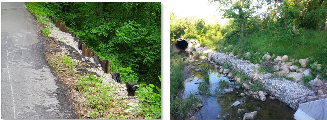
Figure 18: Examples of Cribbing (left) and Gabions (right)
