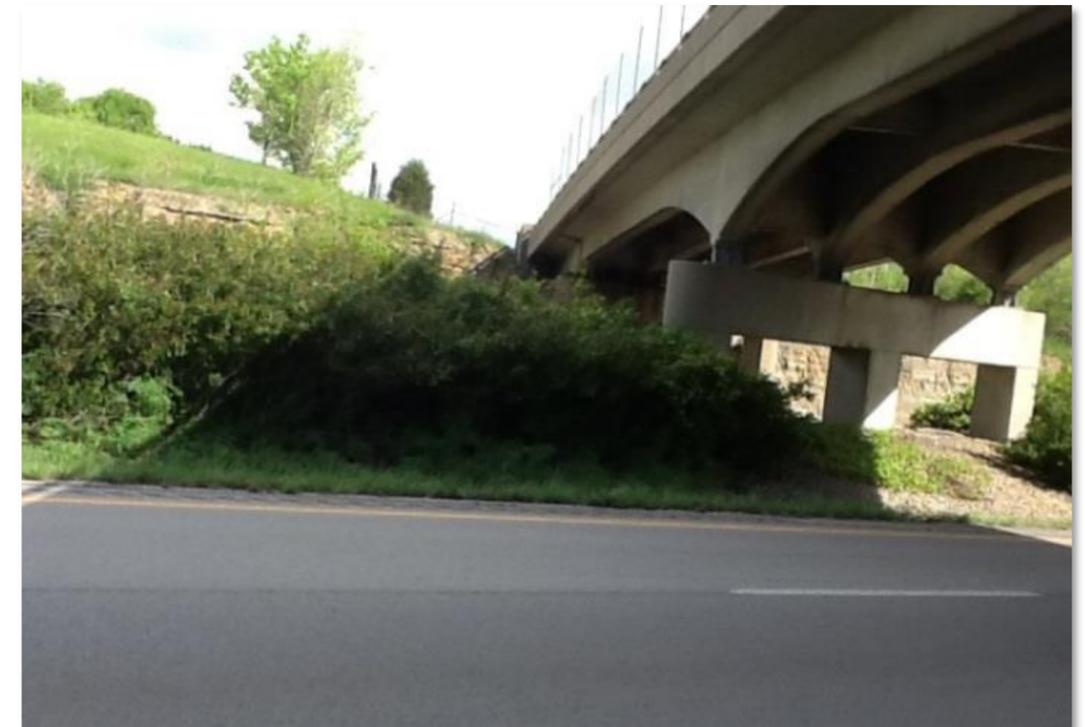
**Photo 3: Pier protection that does not meet standards**
