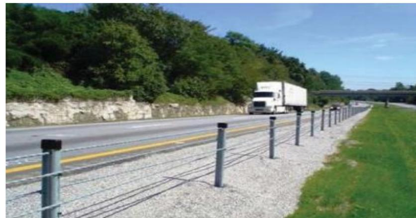
Photo 6: Cable Guardrail
