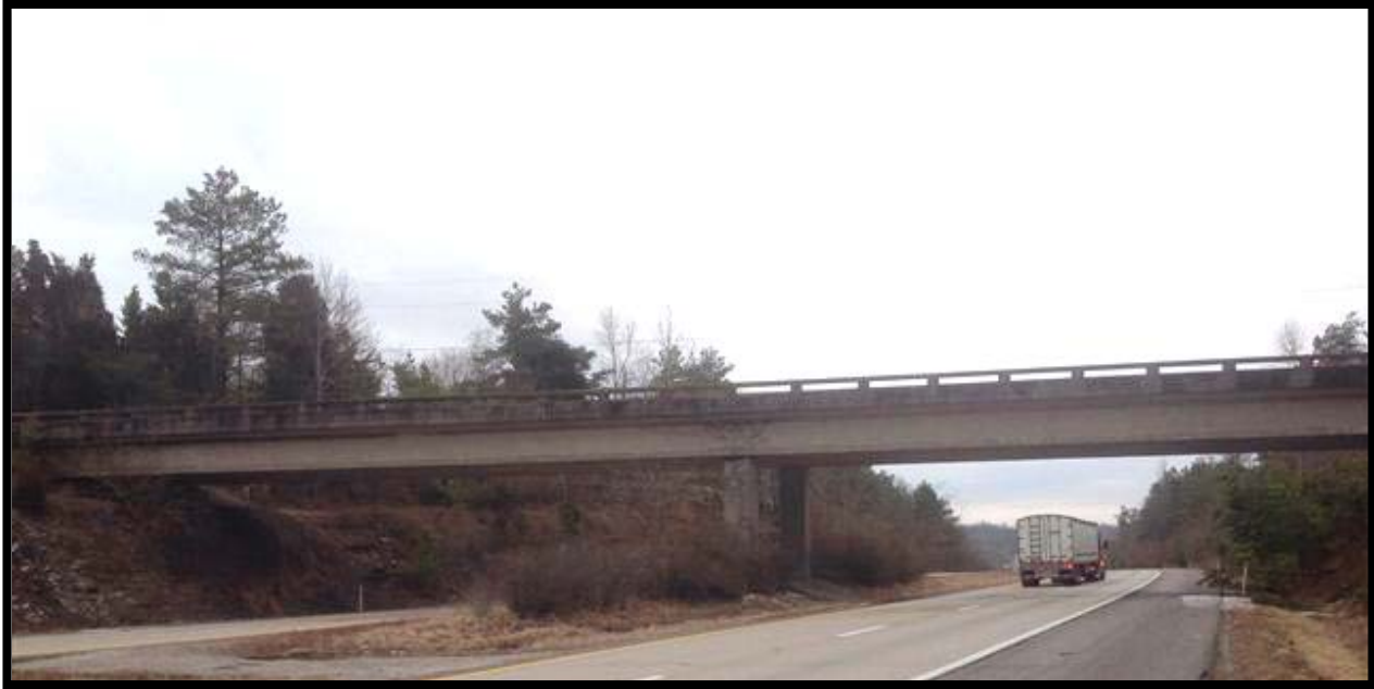
Figure 8: Inadequate Pier Protection - MP 18.474 Cavanaugh Lane (KY 2636)
