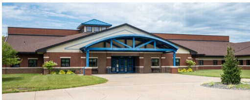
Figure 28: Milton Elementary School
