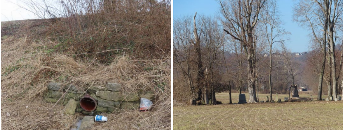
Figure 30: Potentially Historic CRA 1 culvert (left) and CRA 2 cemetery (right)
