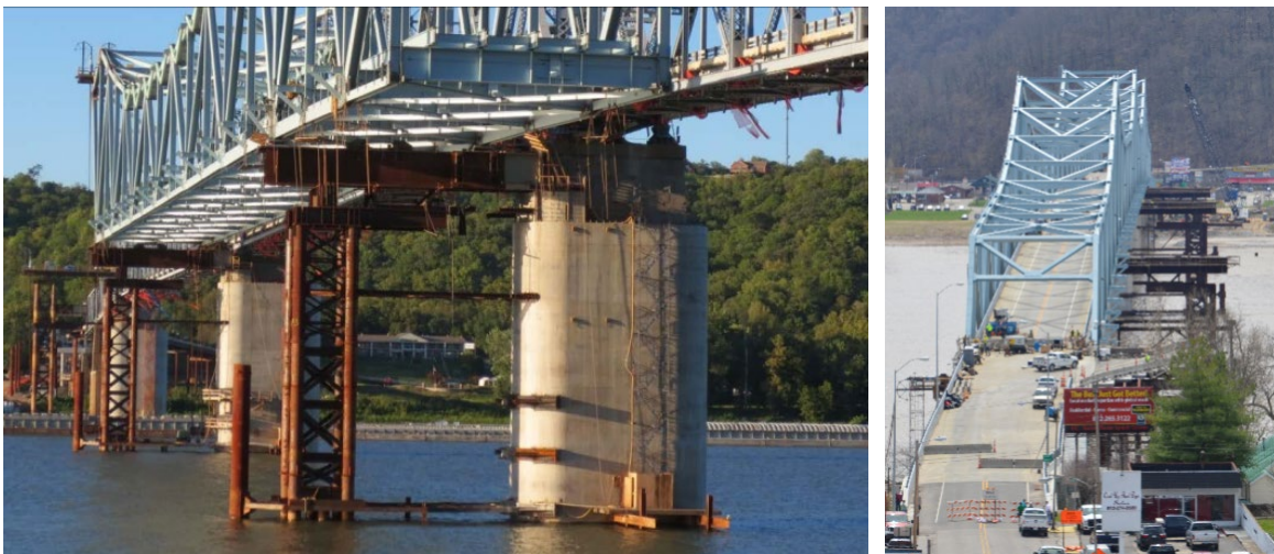
Figure 4: 2012 Bridge Slide, Before and After
