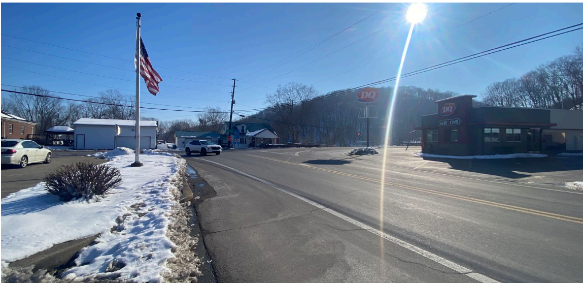
Figure 20: Eastbound US 421 approaching KY 36
