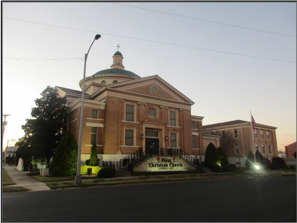
Figure 56. GVM 172: Façade and south elevation of church, looking west-northwest.
