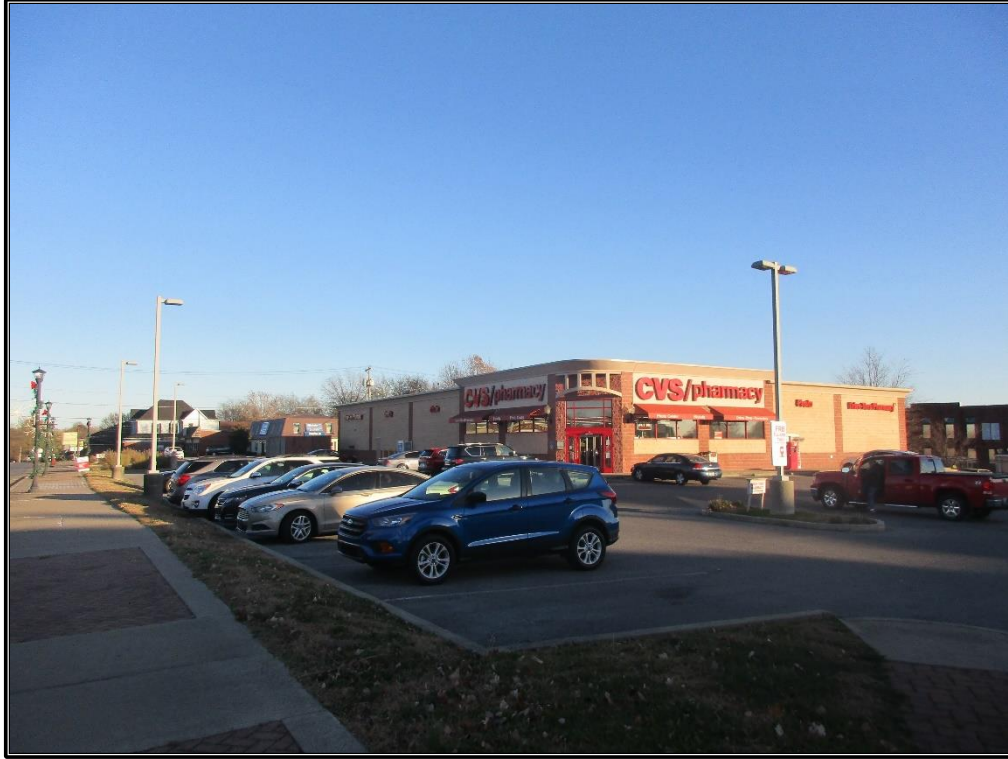
Figure 29. Mayfield Downtown Commercial Historic District: Overview of commercial infill on East Broadway Street, looking south-east.
