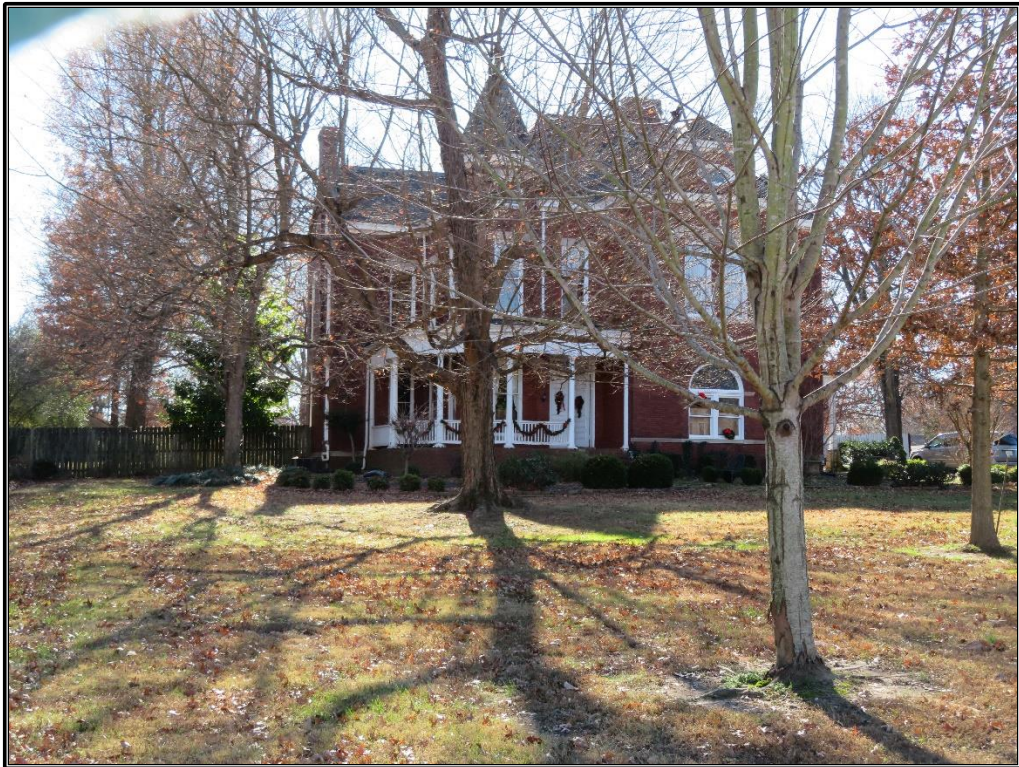
Figure 42. CRA 6: Façade and east elevation of residence, looking west-southwest.
