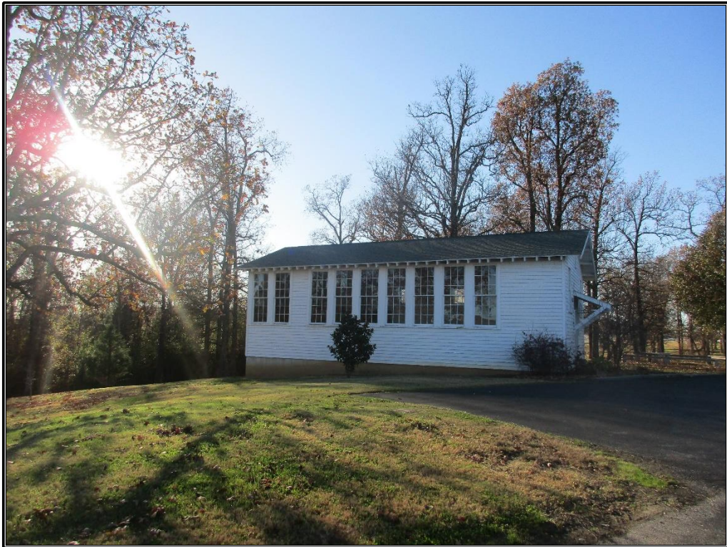
Figure 44. GV 199: Façade and east elevation of former school, looking north-northwest.
