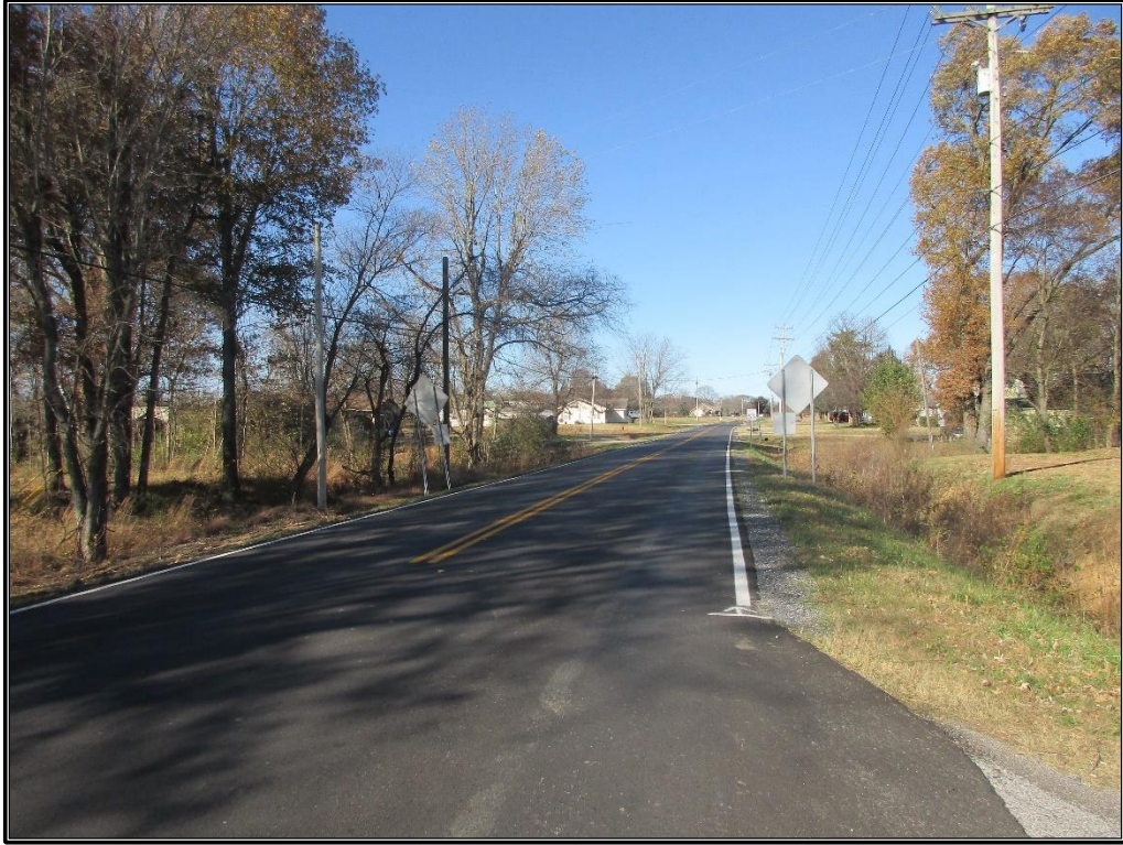
Figure 5. Overview of KY 1241, looking north-northeast.
