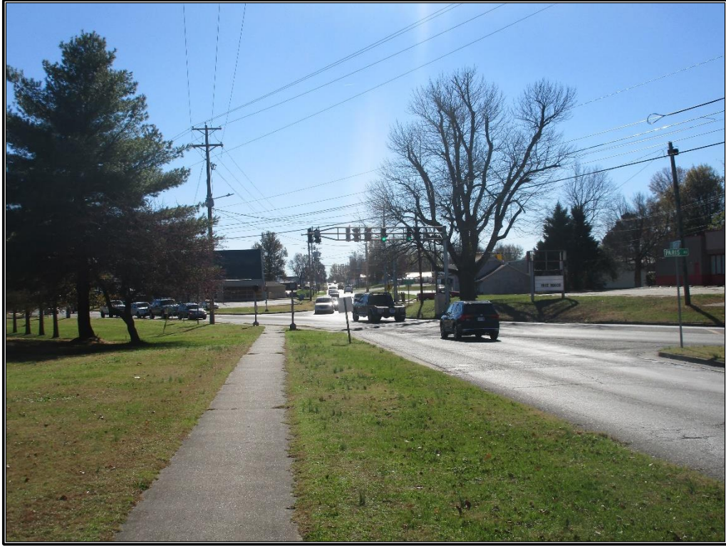
Figure 11. Overview of Cuba Road (KY 303) and Paris Road (KY 121) intersection, looking south.
