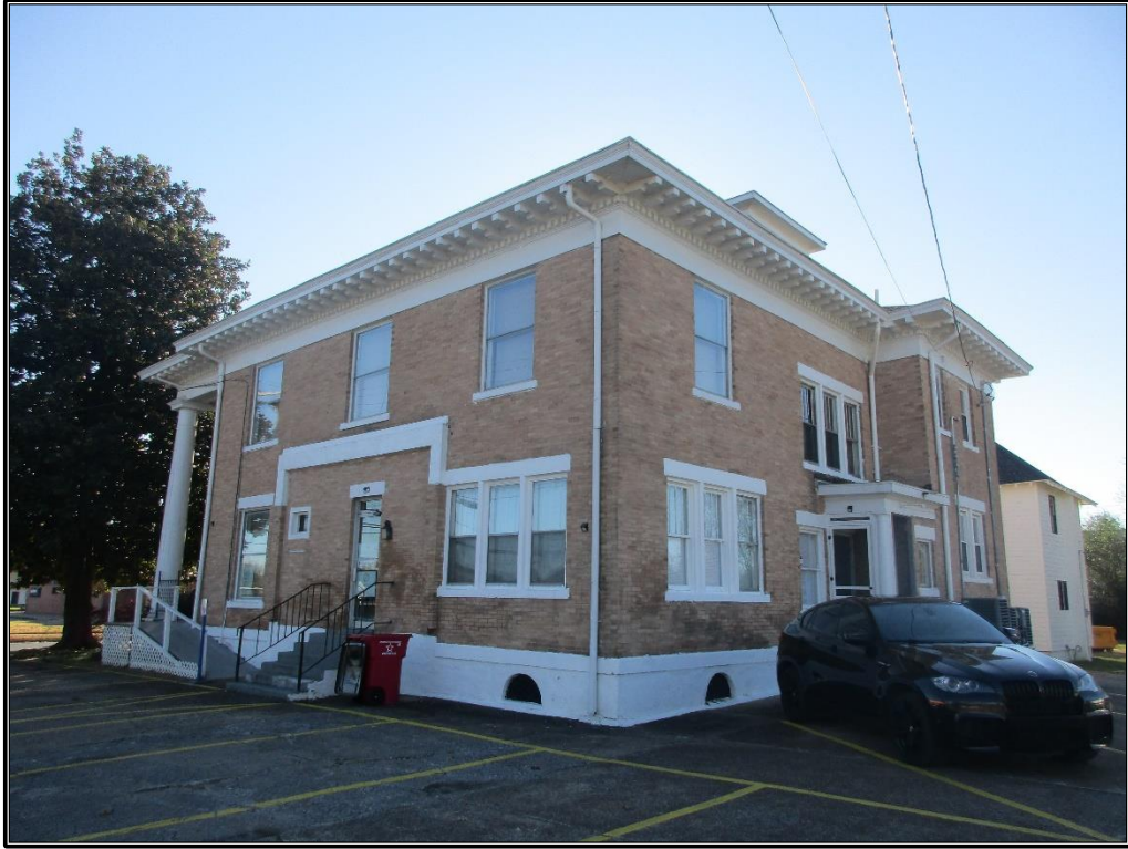
Figure 55. GVM 71: North and rear elevations of residence, looking south-southeast.
