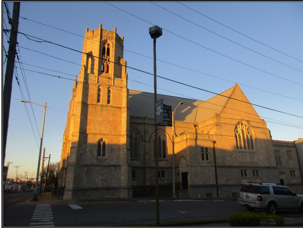
Figure 51. GVM 57: Façade and south elevation of church, looking east-southeast.
