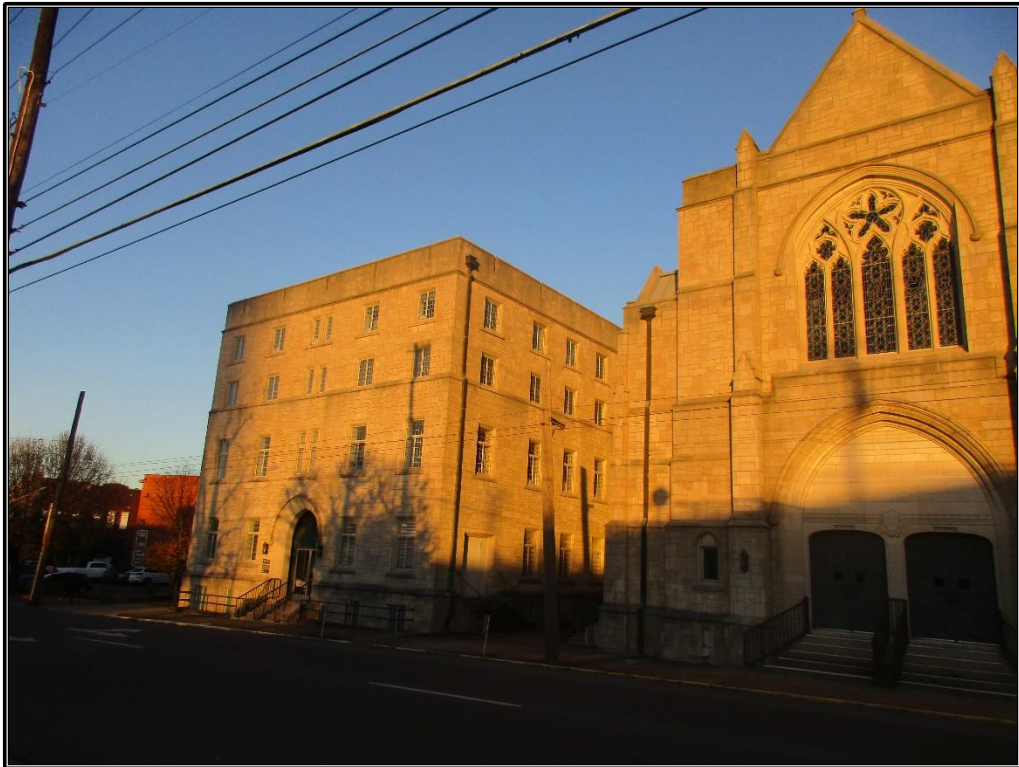
Figure 48. GVM 56: Façade and south elevation of education building, looking east-northeast.
