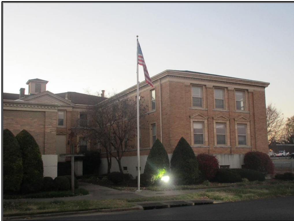
Figure 58. GVM 172: Façade and south elevation of church annex, looking west-northwest.
