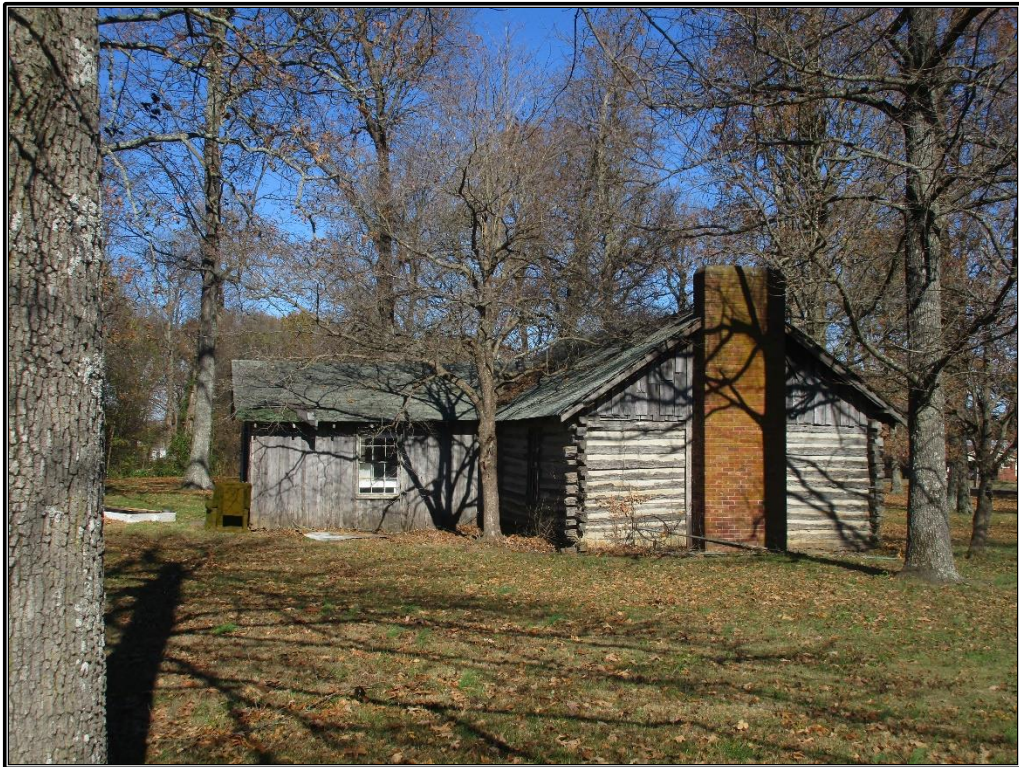
Figure 38. CRA 4: South and rear elevation of residence, looking north-northeast.
