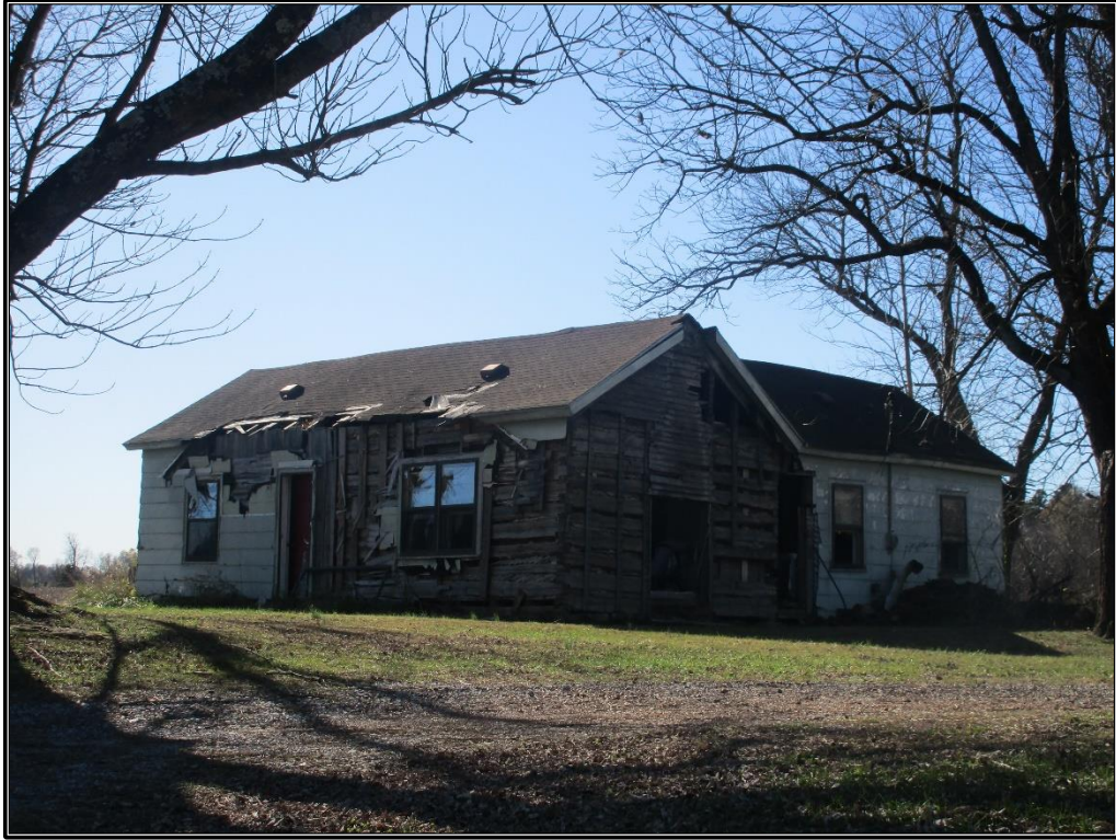
Figure 31. CRA 1: Façade and north elevation of residence, looking south-southwest.
