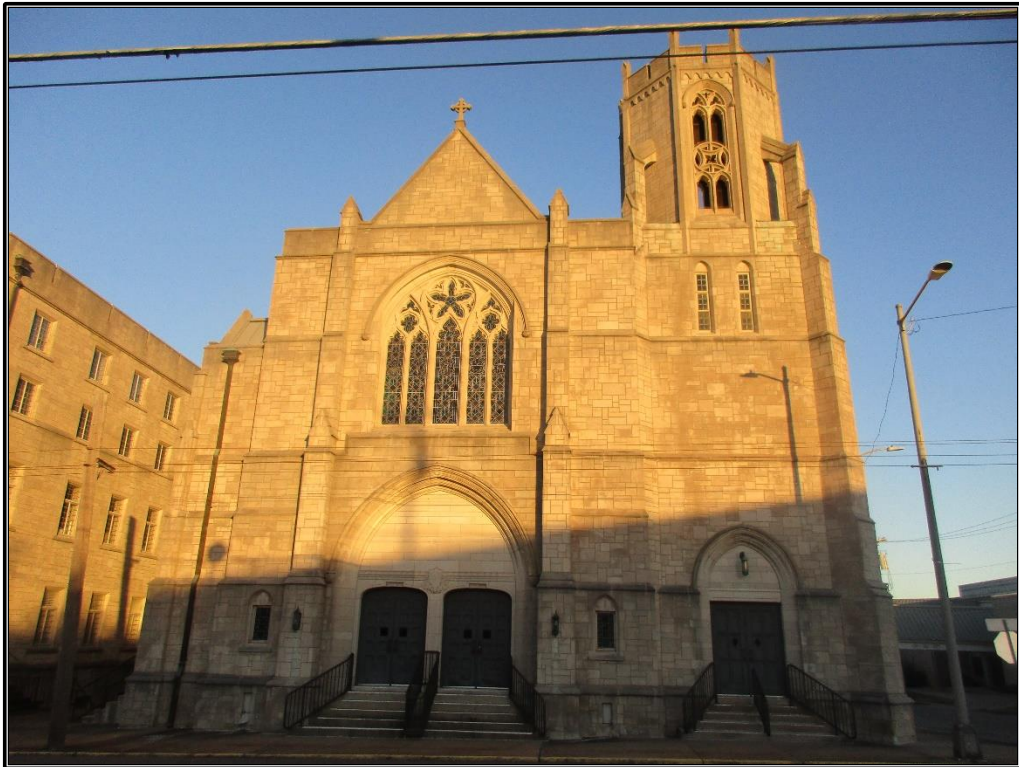
Figure 50. GVM 57: Façade of church, looking east.
