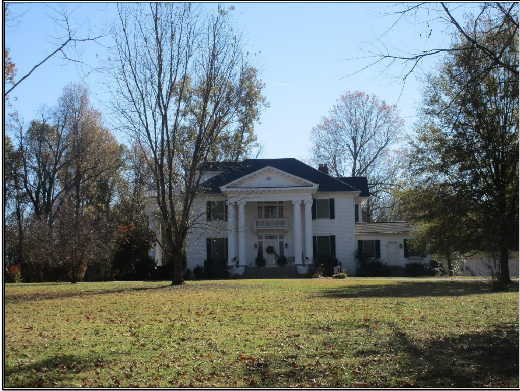
Figure 39. CRA 5: Façade of residence, looking south.
