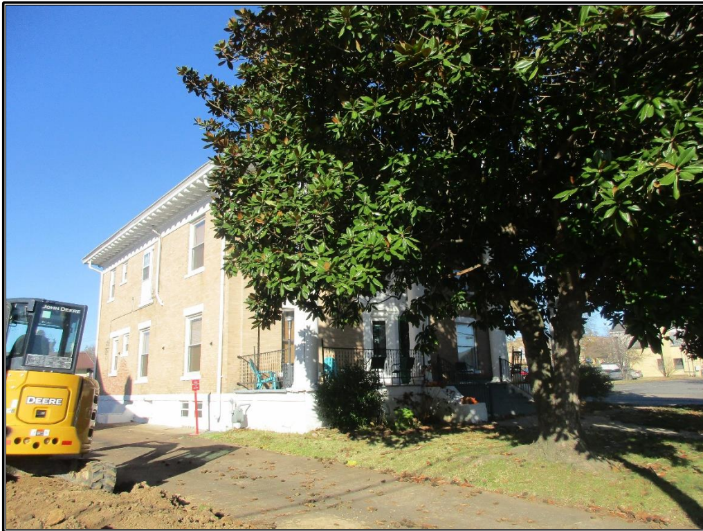
Figure 54. GVM 71: Façade and south elevation of residence, looking west-northwest.
