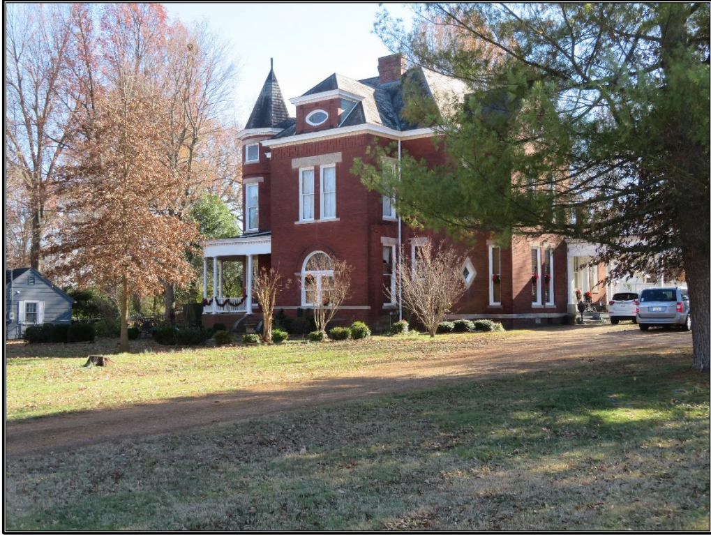
Figure 41. CRA 6: Façade and west elevation of residence, looking south-southeast.
