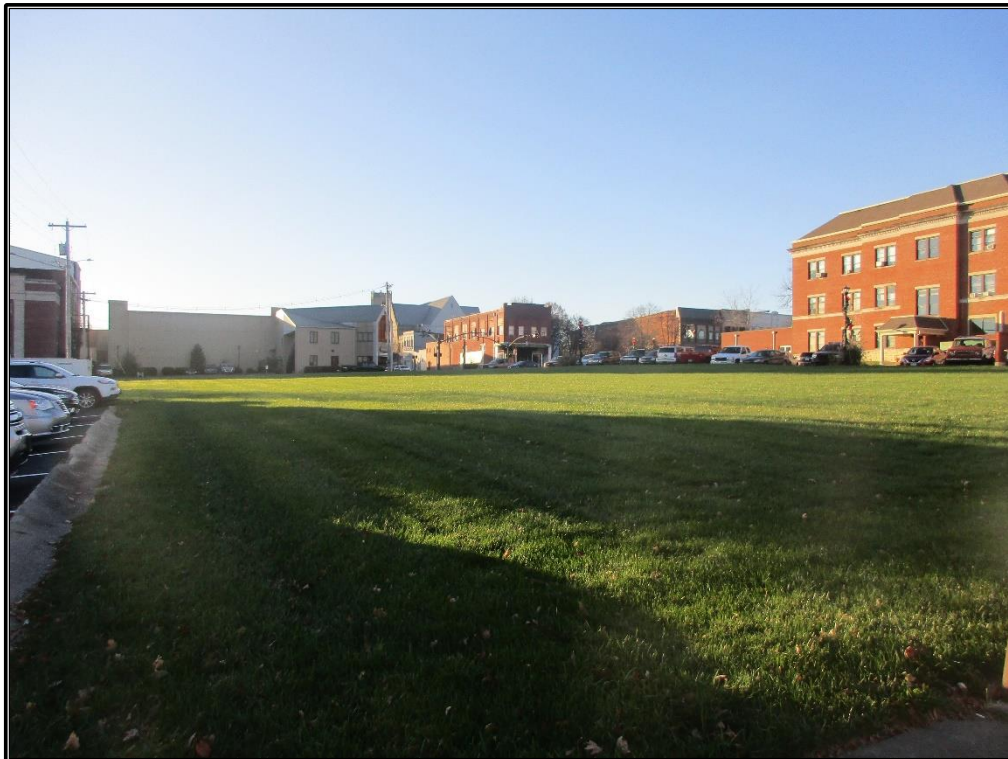
Figure 30. Mayfield Downtown Commercial Historic District: Overview of demolished properties on East South Street, looking west-northwest.
