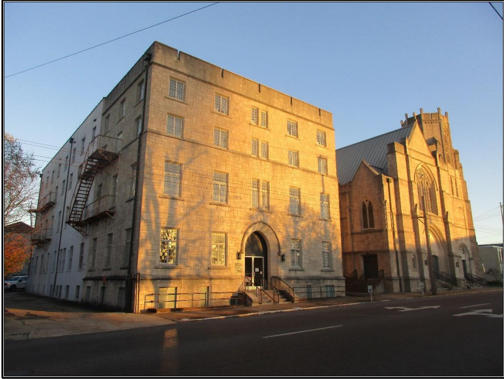
Figure 49. GVM 56: Façade and north elevation of education building, looking southeast.
