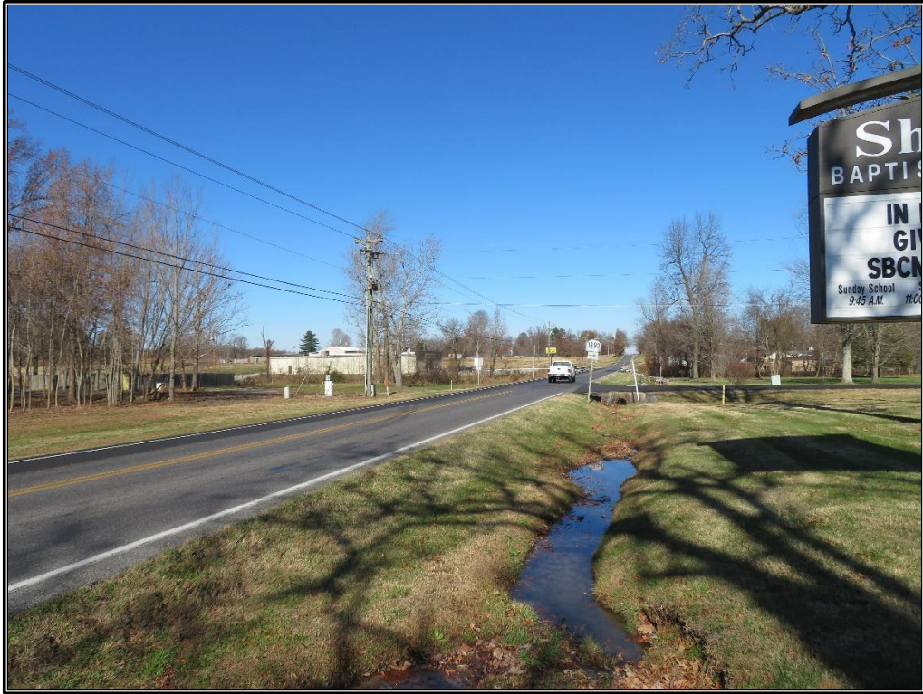
Figure 12. Overview of Cuba Road (KY 303) and KY 1890 intersection, looking northwest.
