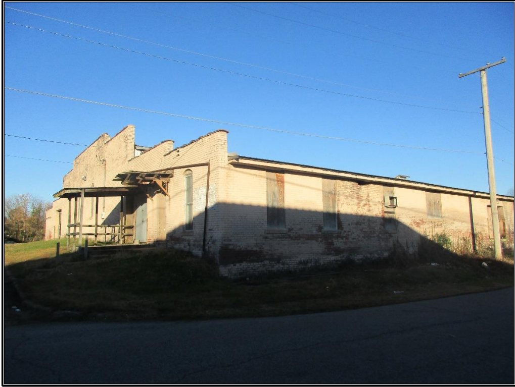
Figure 21. GVM 376: Façade and east elevation of warehouse, looking north-northwest.
