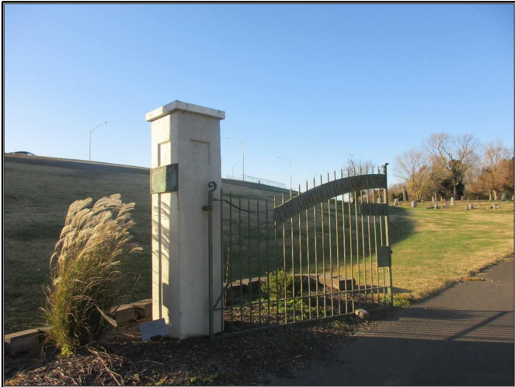
Figure 20. GVM 70: View of west gate, looking south-southwest.
