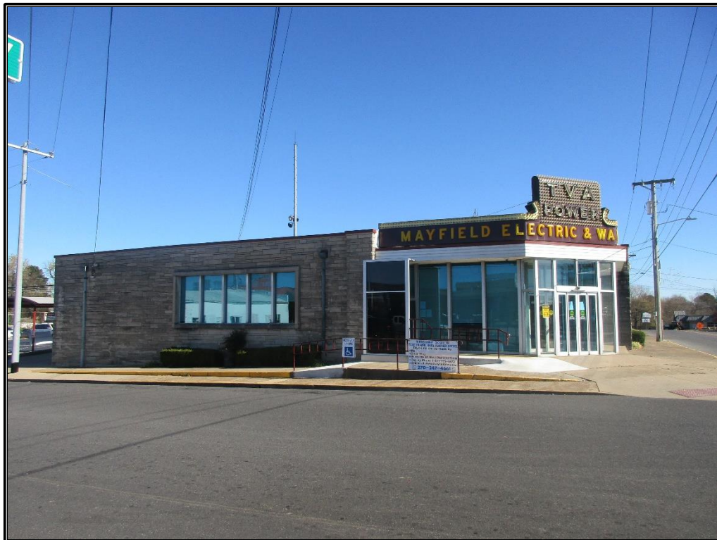
Figure 36. CRA 3: Façade and west elevation of building, looking east-northeast.
