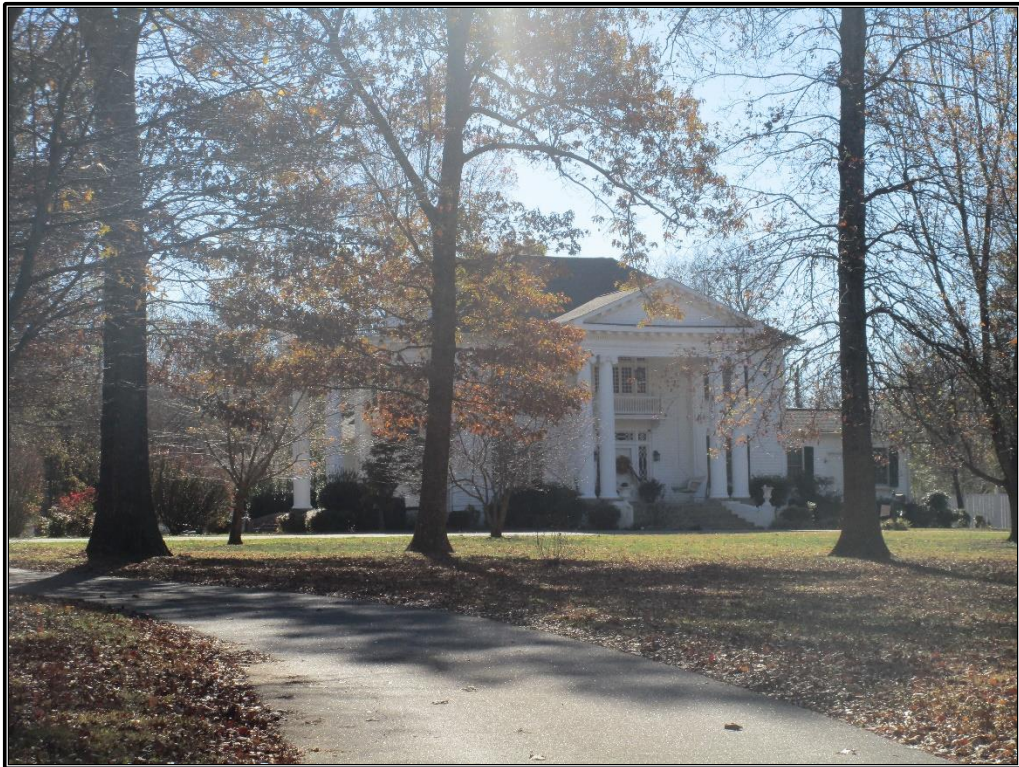
Figure 40. CRA 5: Façade and east elevation of residence, looking south-southwest.
