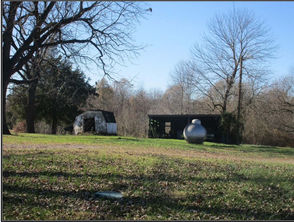
Figure 33. CRA 1: Overview of outbuildings (Resources A and B), looking west.
