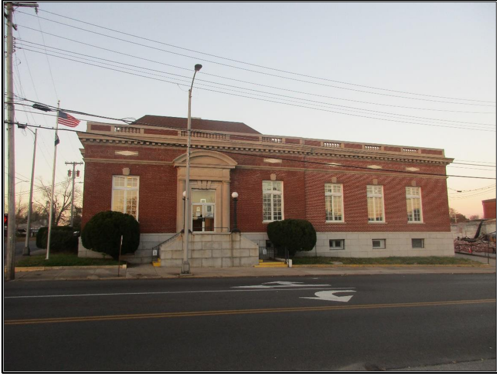
Figure 15. GVM 2: Façade of post office, looking north.
