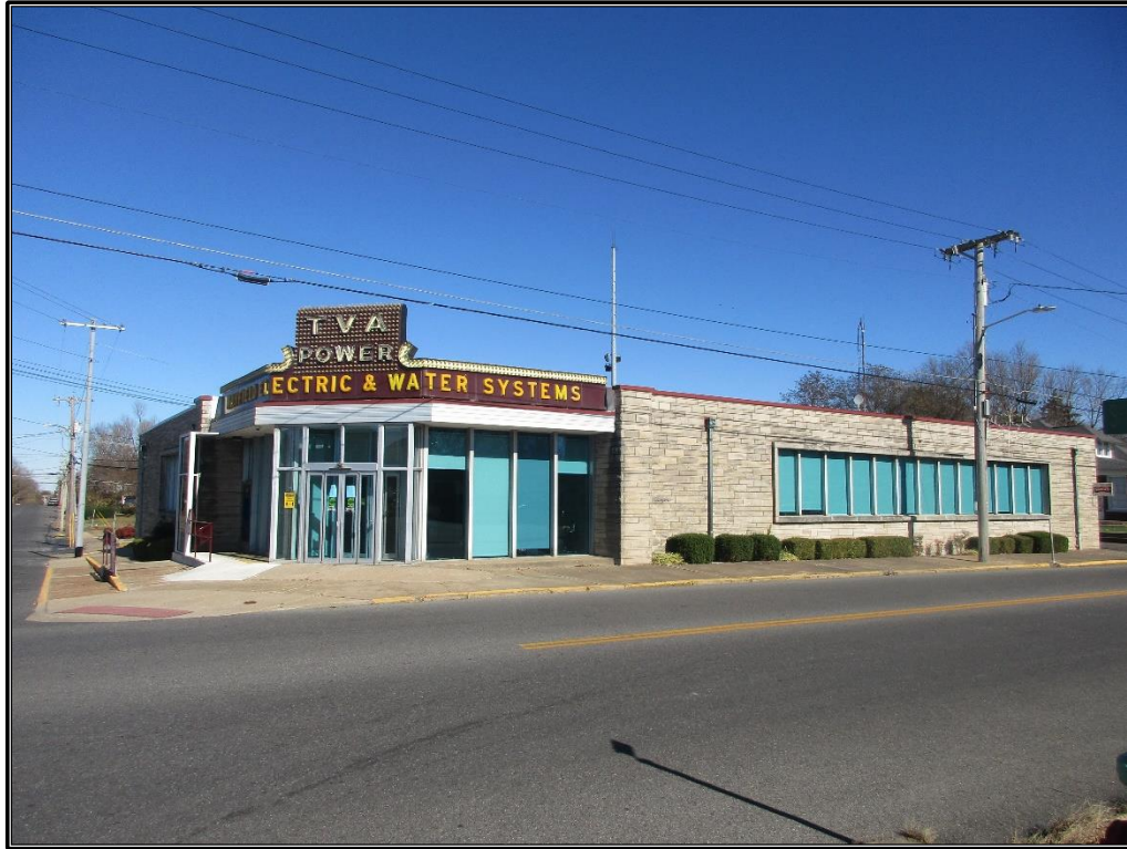
Figure 35. CRA 3: Façade and south elevation of building, looking north-northeast.
