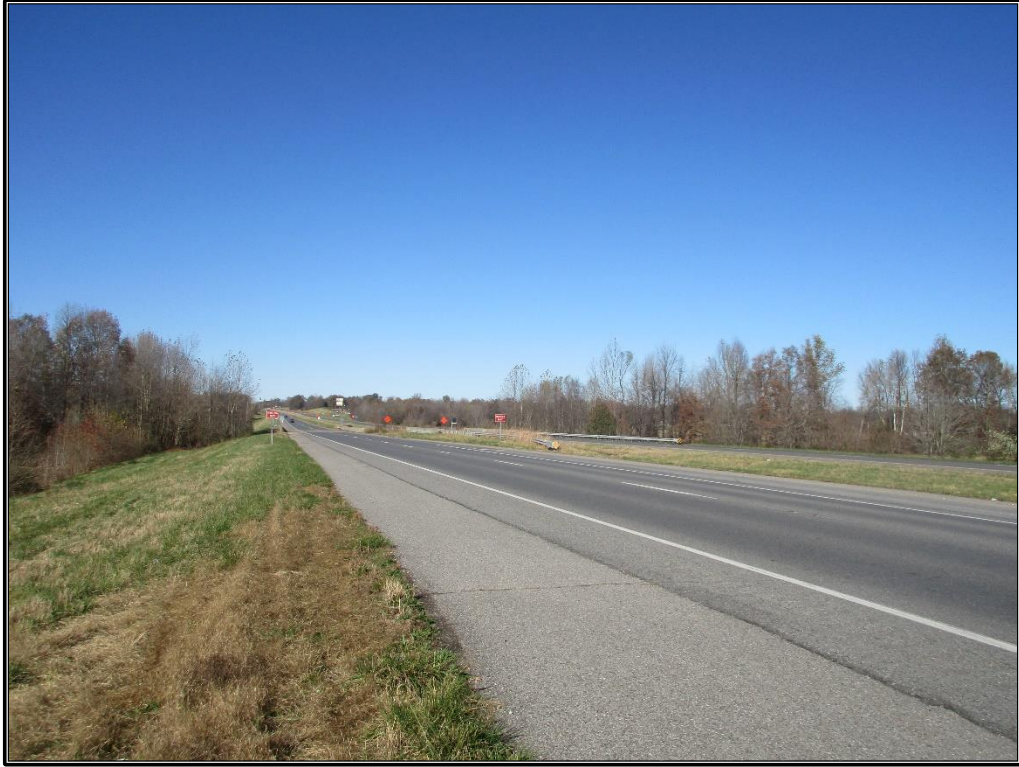
Figure 3. Overview of US 45 from KY 2195 intersection, looking north-northwest.
