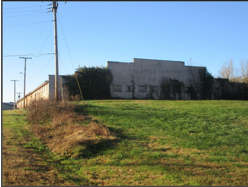
Figure 23. GVM 376: Rear elevation of warehouse, looking south-southwest.
