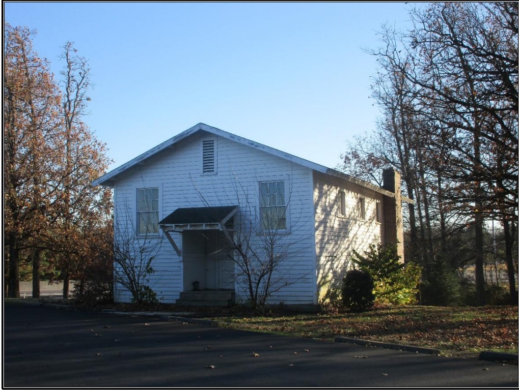
Figure 43. GV 199: Façade and west elevation of former school, looking south-southeast.
