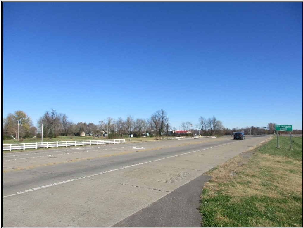
Figure 10. Overview of KY 121, looking south.
