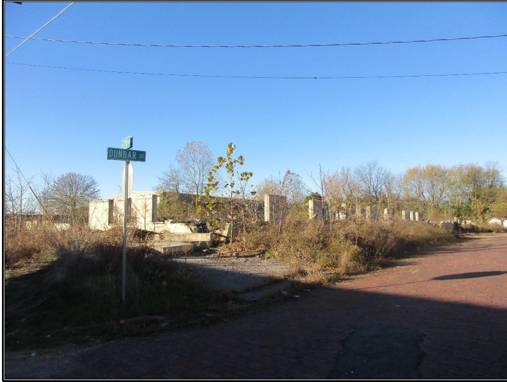
Figure 75. Potential Tobacco Warehouse Historic District: View of demolished warehouse on Dunbar Street, looking southwest.
