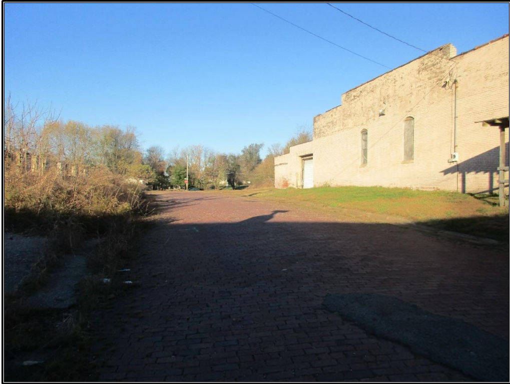
Figure 72. Potential Tobacco Warehouse Historic District: Overview of Dunbar Street, looking west.
