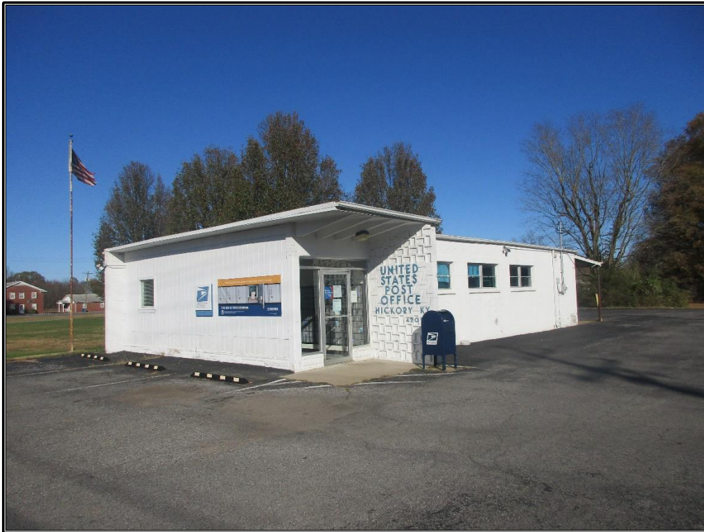
Figure 34. CRA 2: Façade and south elevation of post office, looking north-northeast.
