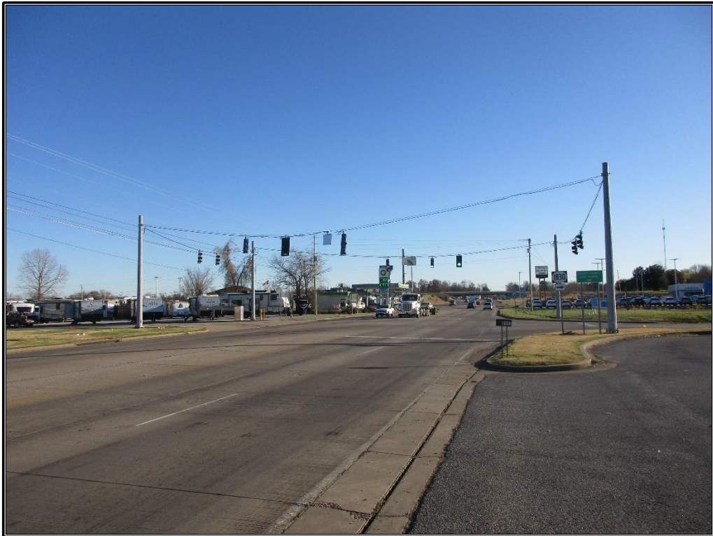
Figure 4. Overview of US 45 and KY 1830 intersection, looking south.
