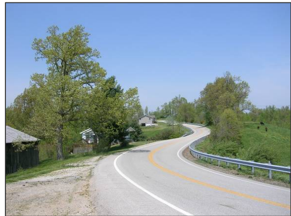
Typical Corridor View along KY 32
