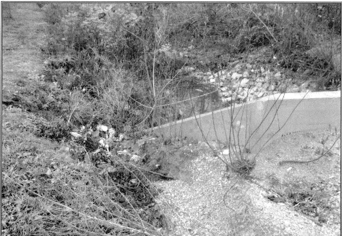
Photograph 8: View of an unnamed ephemeral stream crossing, west of 7031 Southside Drive. The stream emerges from a culvert on the south side of the road but lacks an aboveground channel on the north side of the road. Southside Drive Widening. December 6, 2004.
