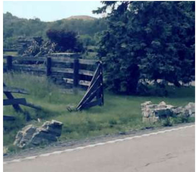
Fence and mailbox damaged by CMV crash in 2016
