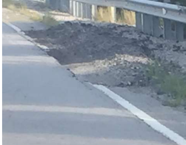
Shoulder failure
