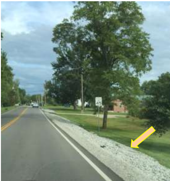
Shoulder widening in Alton area
