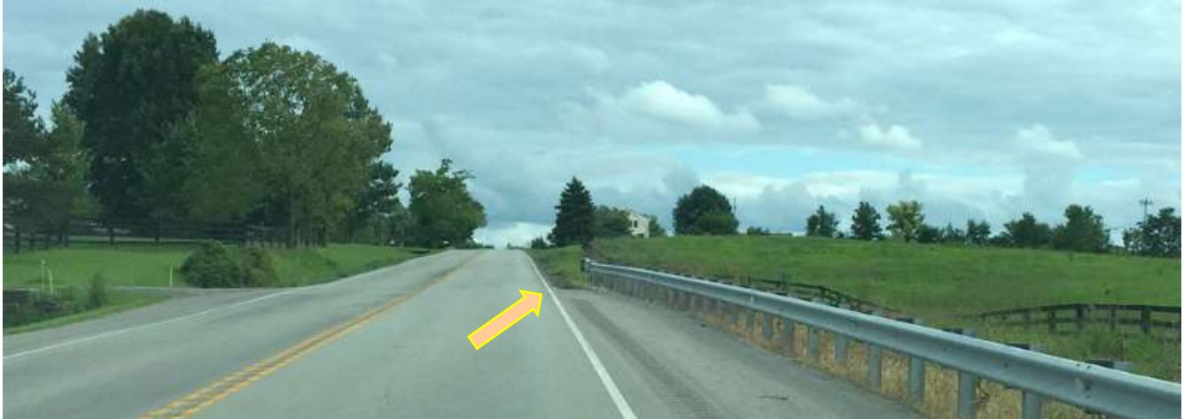
Change in paved width at MP 4.1, Anderson County, looking southbound
