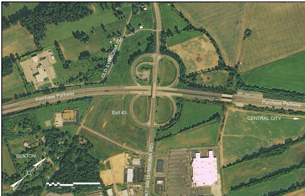
Exit 43 – Purchase Parkway / KY 348 Previous Toll Plaza
