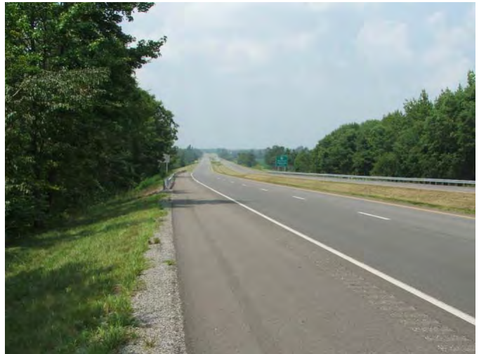
Clear zones may require guardrail placement or extensions to meet current standards.
