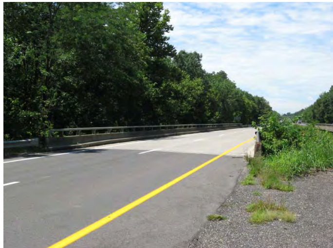
The mainline bridges that do not meet minimum lateral clearance are greater than 200 ft long.
