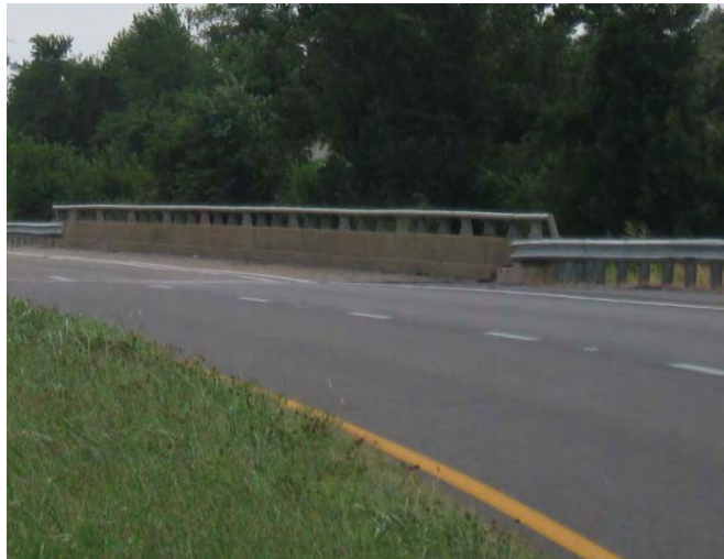
All of the Purchase Parkway mainline bridges have side railings/barriers that do not meet current standards.
