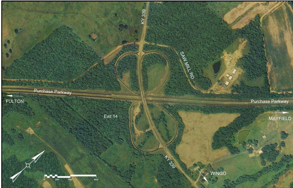
Exit 14 – Purchase Parkway / KY 339 Previous Toll Plaza
