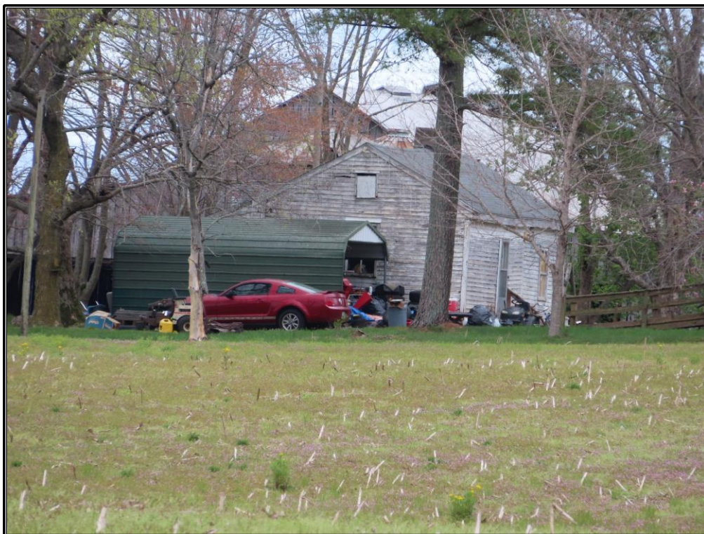
Figure A-12: TR 86: Façade and south elevation of the tenant house, looking north-northwest.
