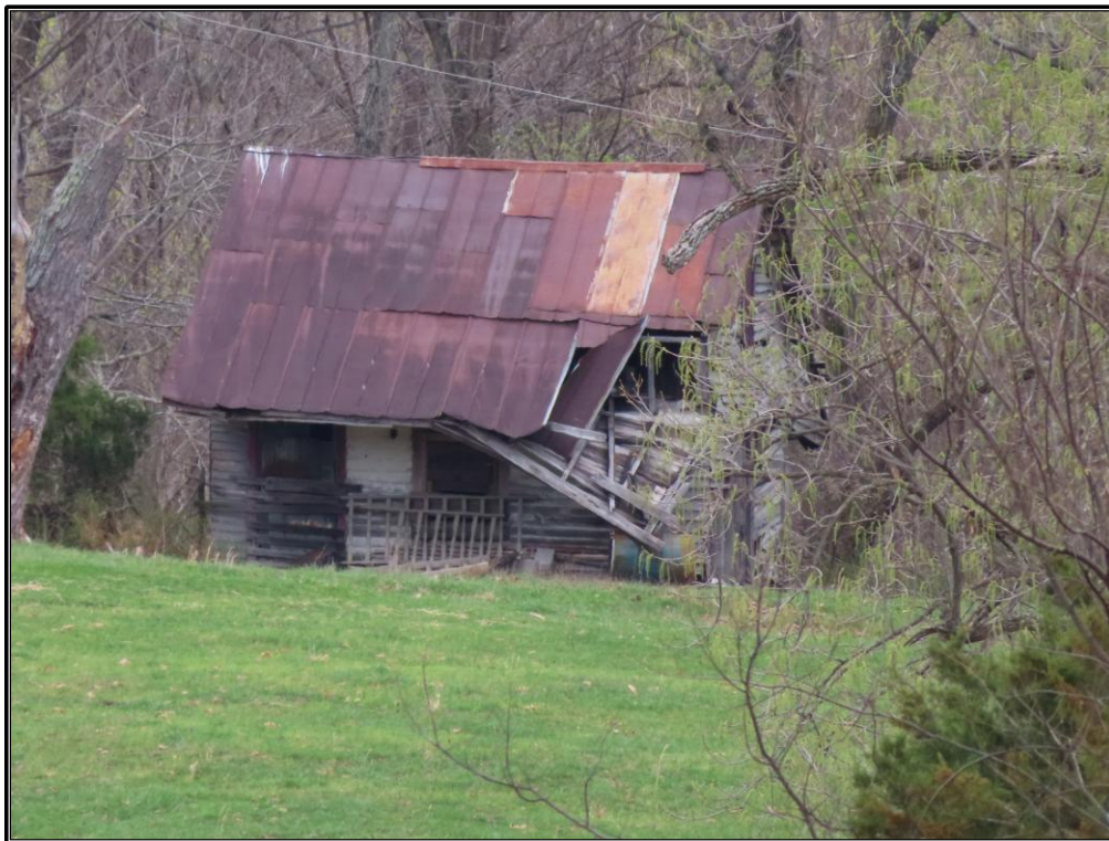
Figure A-11: TR 85: Façade and southwest elevation of the residence, looking east.
