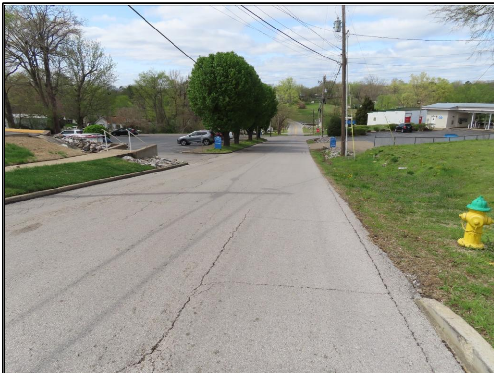
Figure 9. Overview towards the study area from the southwestern limit of the Cadiz Residential Historic District, looking northwest.
