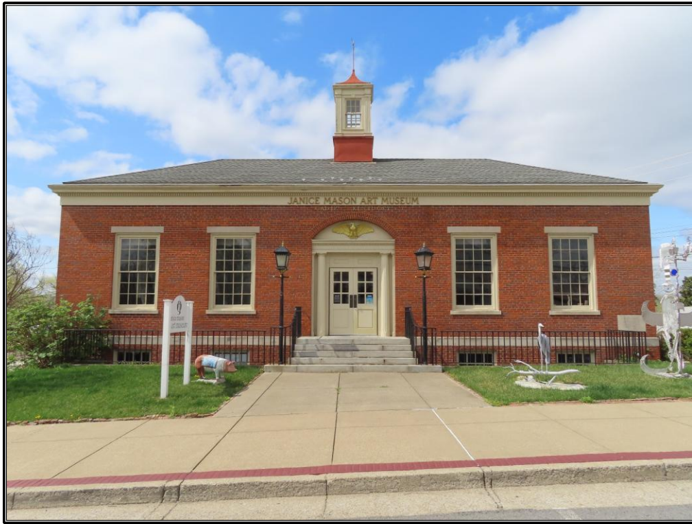
Figure A-29. TRC 41: Façade of the former post office, looking northwest.
