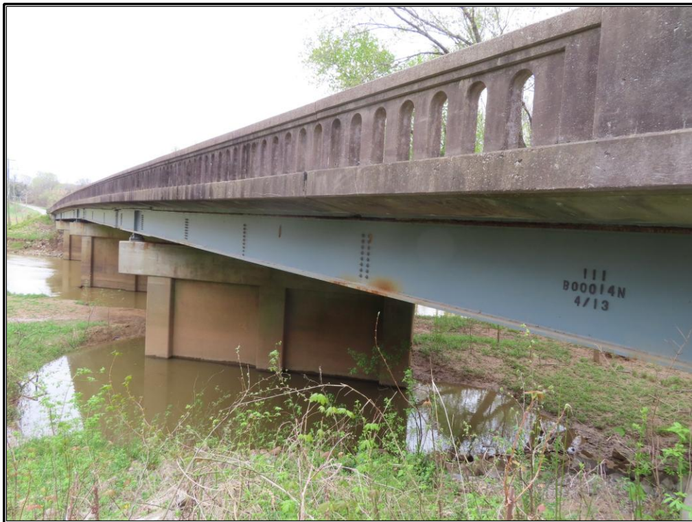
Figure 32. CRA 14: Overview of the bridge piers and railing, looking southeast.
