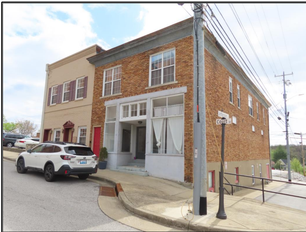
Figure 28. CRA 11: Façade and northwest elevation of the commercial buildings at CRA 11 and CRA 12, looking southwest.
