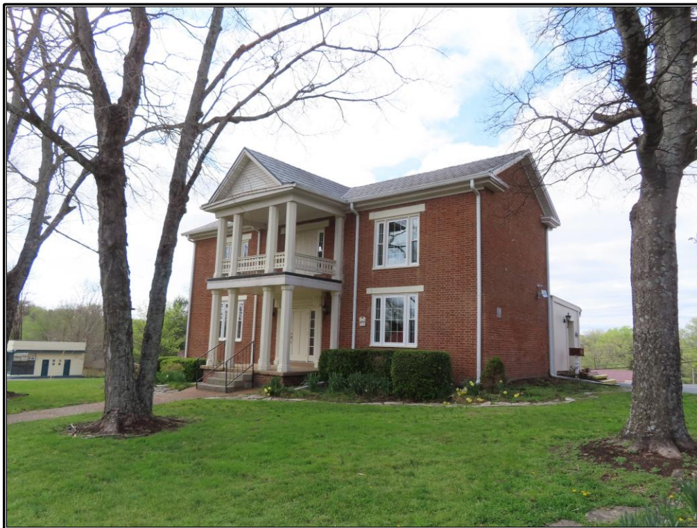
Figure A-37. TRC 71: Façade and northeast elevation of the residence, looking southwest.
