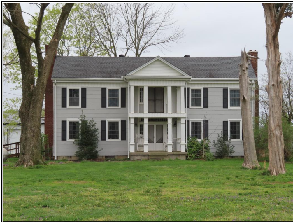
Figure A-1. TR 78: Façade of the residence, looking southwest.
