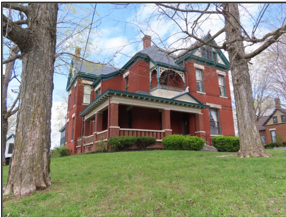
Figure A-28. TRC 54: Façade and southwest elevation of the residence, looking north-northwest.
