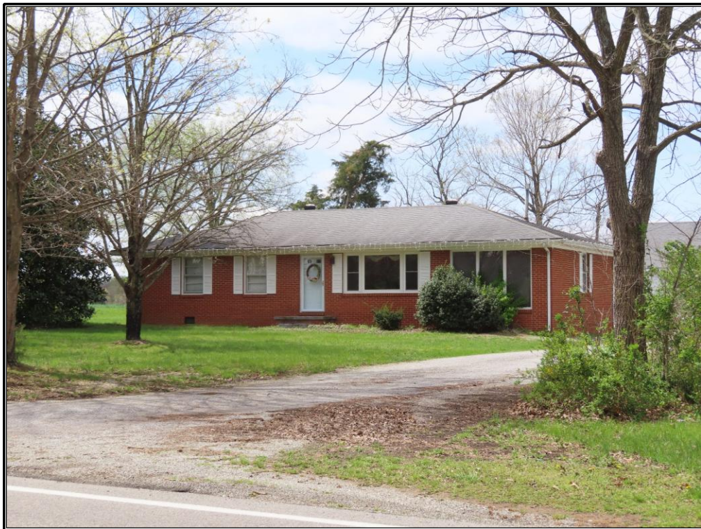
Figure A-16. TR 238: Façade and northeast elevation of the residence, looking southwest.
