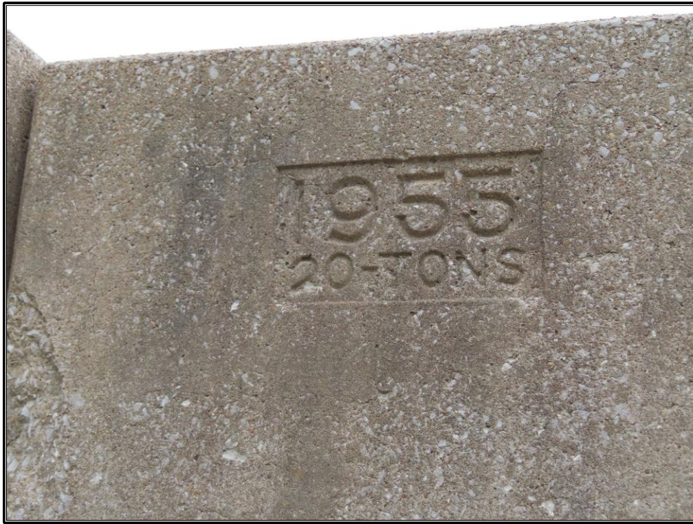
Figure 33. CRA 14: Date stamp located on the southeast abutment, looking northwest.
