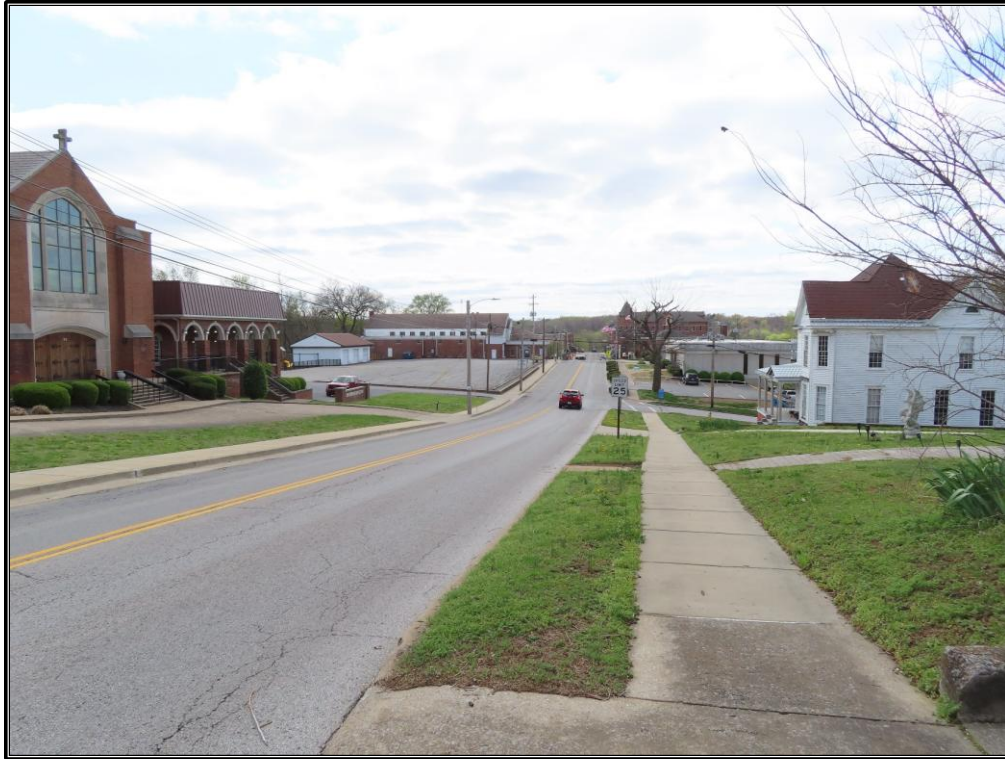
Figure 8. Overview of the Cadiz Residential Historic District near the intersection of Main and Brown Streets, looking southwest.
