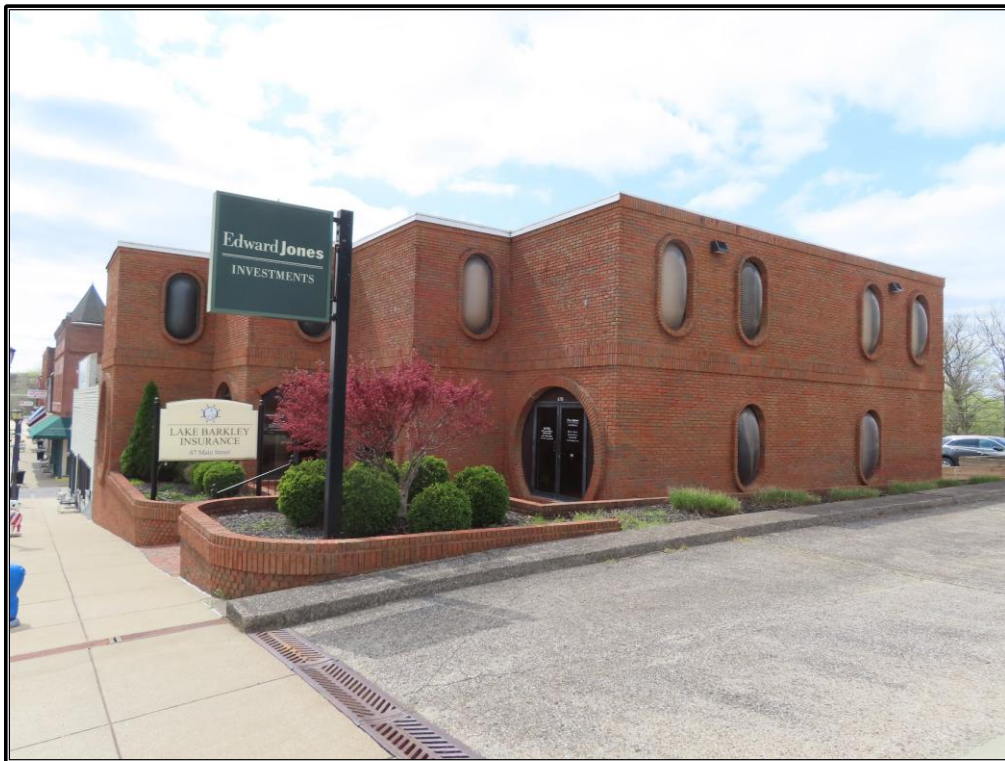
Figure 22. CRA 9: Façade and northeast elevation of the commercial building, looking west-northwest.
