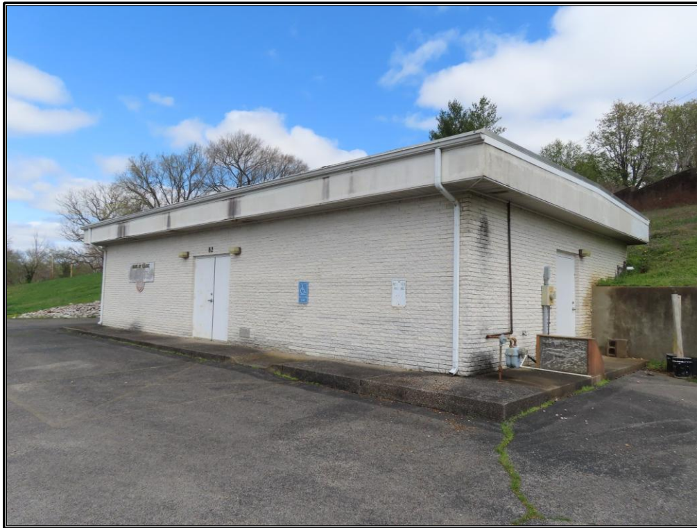
Figure A-25. TRC 4: Overview towards the razed structure showing the 1980s building, looking northeast.
