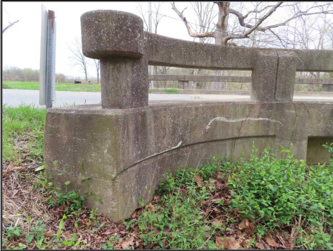
Figure 14. CRA 3: Detail of the bridge's railing and curved ends, looking southwest.
