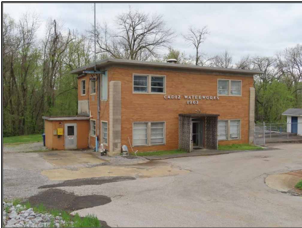
Figure 30. CRA 13: Façade and northeast elevation of the Cadiz Waterworks building, looking south.
