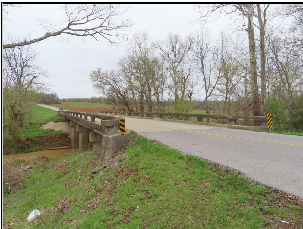
Figure 13. CRA 3: Overview of the bridge carrying KY 276 over Kenady Creek, looking northwest.
