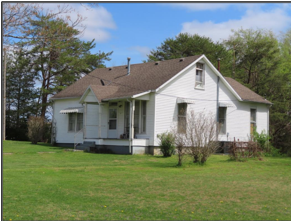
Figure A-21. TR 244: Façade and southwest elevation of the residence, looking northeast.
