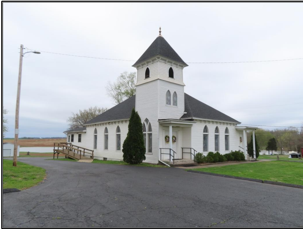
Figure A-5. TR 95: Northwest and northeast elevations of the Wallonia Baptist Church, looking southeast.
