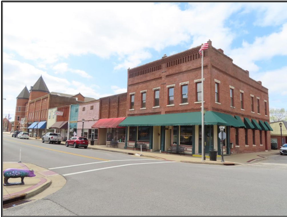
Figure A-31. TRC 7, TRC 24, TRC 68, and TRC 69: Overview of the commercial buildings in Cadiz, looking southwest.
