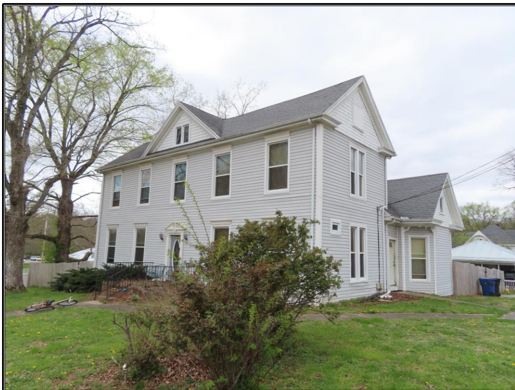
Figure A-38. TRC 9: Façade and northeast elevation of the residence, looking southwest.
