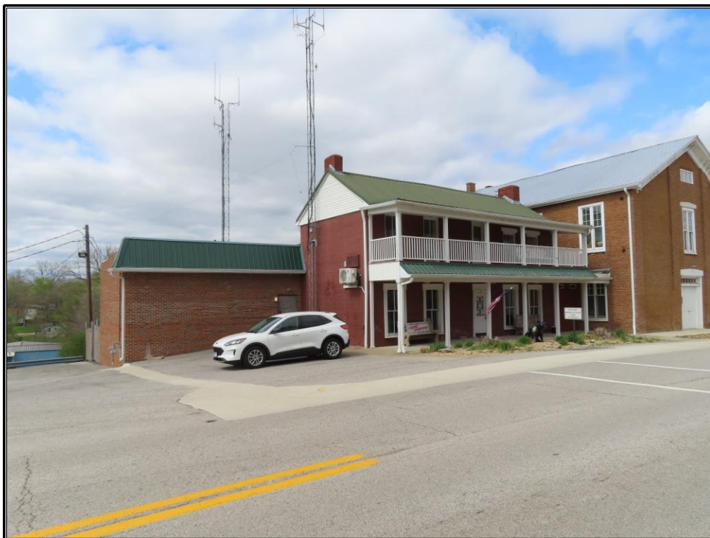
Figure A-42. TRC 8: Façade and southwest elevation of the residence, looking northeast.
