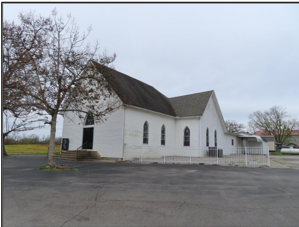
Figure A-8. TR 89: Façade and northeast elevation of the Wallonia Christian Church, looking southwest.
