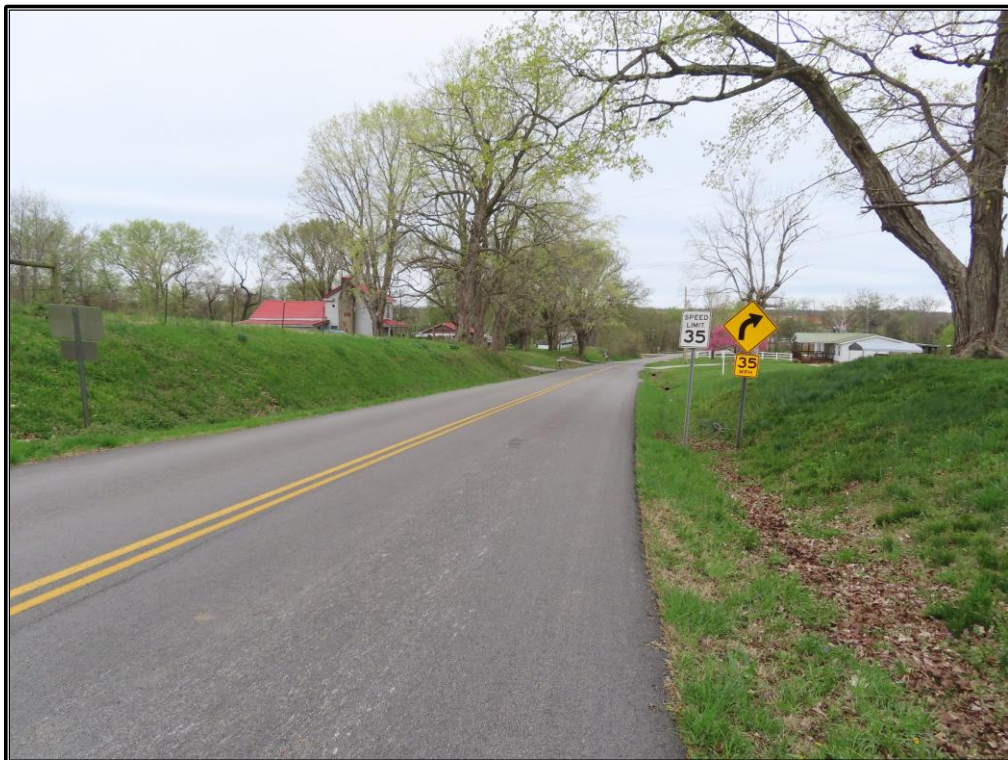
Figure 36. Overview of the study area at the intersection of KY 276 and KY 128 in the community of Wallonia, looking northwest.
