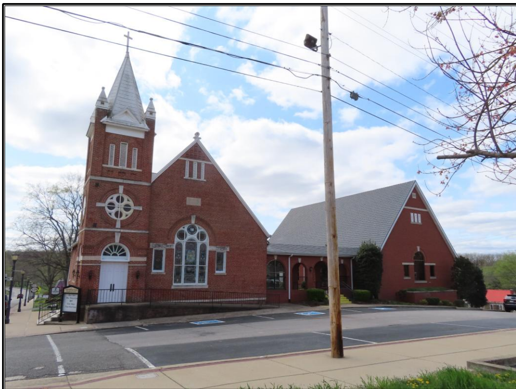
Figure A-36. TRC 27: Northeast elevation of the Cadiz Christian Church, looking southwest.
