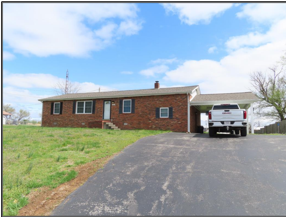
Figure A-17. TR 239: Façade and southwest elevation of the residence, looking east-northeast.
