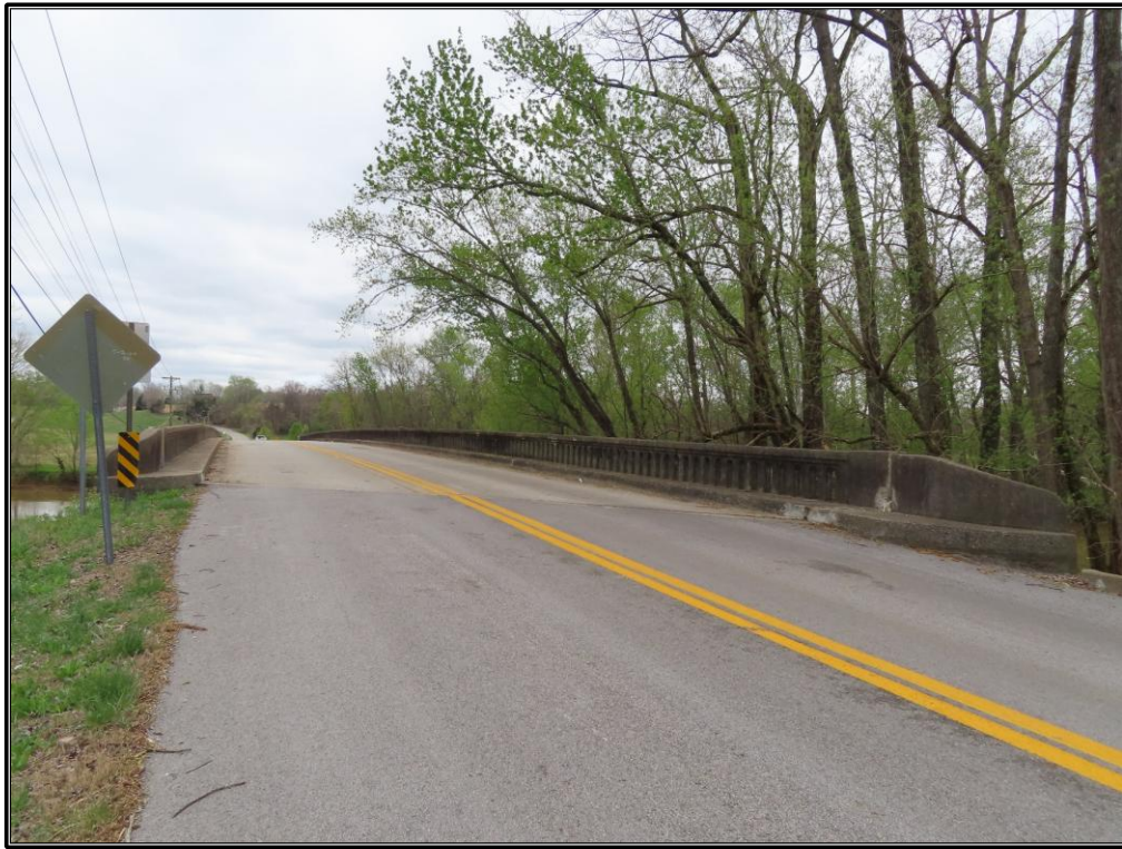
Figure 31. CRA 14: Overview of the bridge, looking south.
