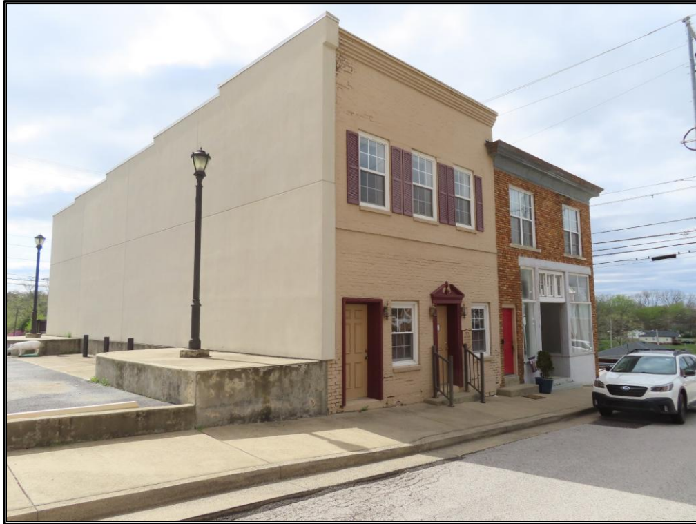
Figure 29. CRA 12: Façade and southeast elevation for the commercial buildings at CRA 11 and CRA 12, looking west-northwest.
