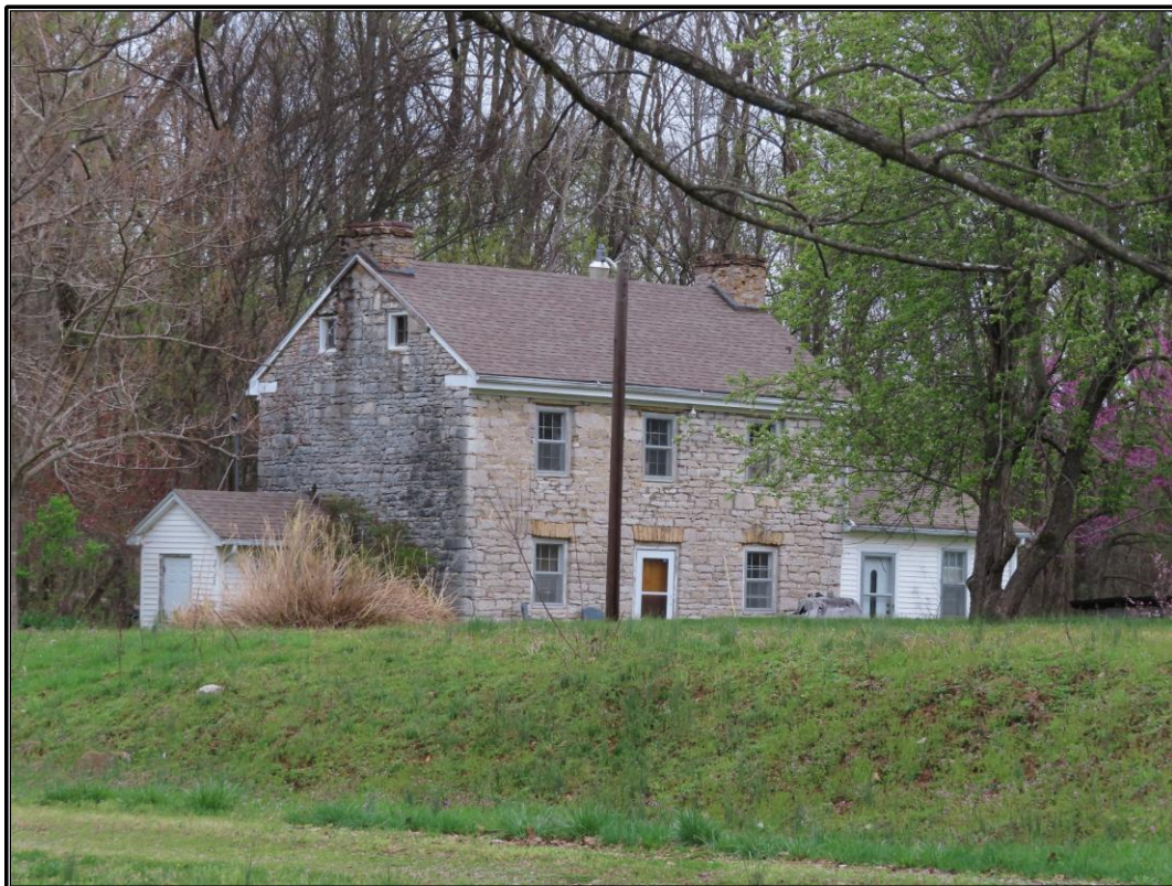
Figure 3. Site TR 22: Façade and northwest elevation of the residence, looking northeast.
