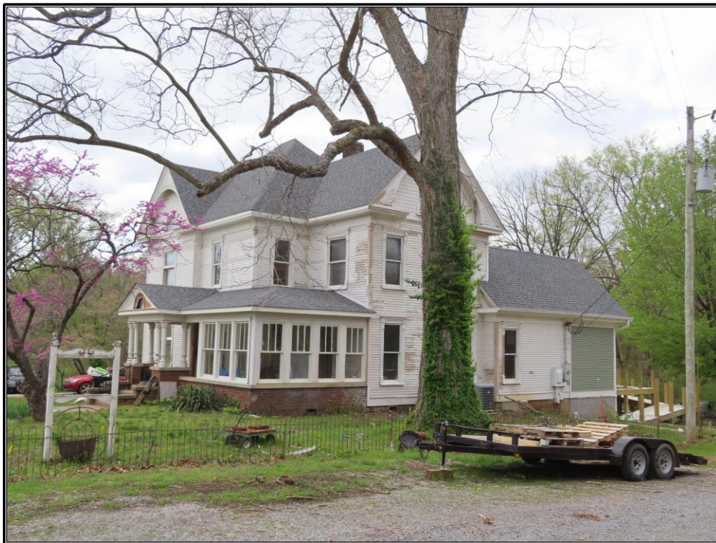
Figure A-39. TRC 11: Façade and northeast elevation of the residence, looking southwest.
