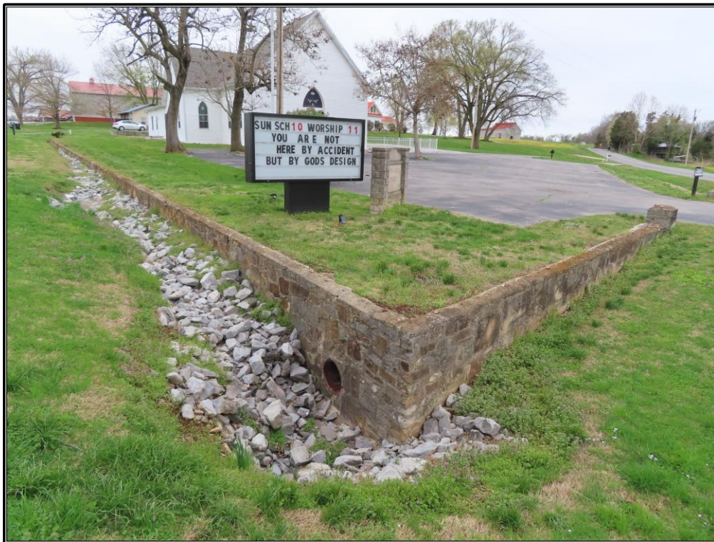
Figure A-9. TR 89: Overview of the stone retaining wall at the Wallonia Christian Church, looking northwest.
