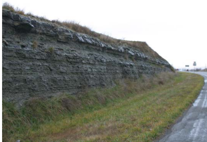
Photo 2. Typical Outer Blue Grass Stratigraphy Along Existing KY 555 Road Cut Showing Interbedded Limestones and Shales
