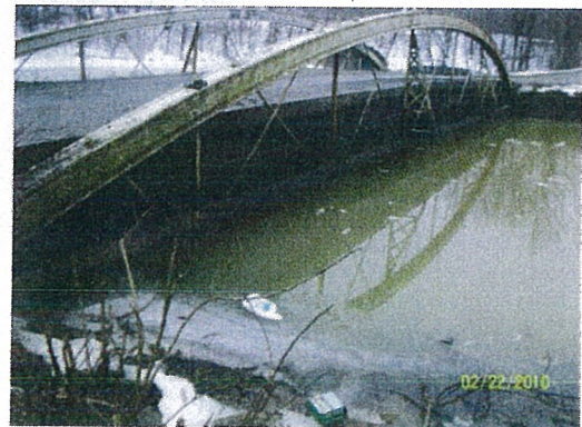
Right side view of structure, note clearance between lower chord and surface of stream
