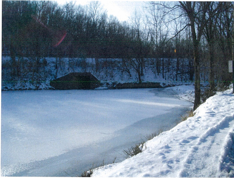
Estimated Single 12 ft X 12 ft Reinforced Concrete Culvert and Double 14 ft X 14 ft Reinforced Concrete Culvert at KY 8
