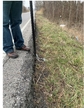
Figure 31: Pavement Drop
