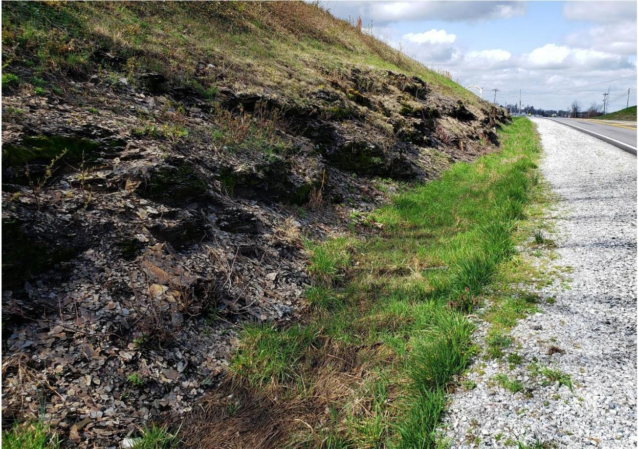
*Image 1: East Lebanon, looking West along US 68. Note the poor quality and natural slope of the shale.*
