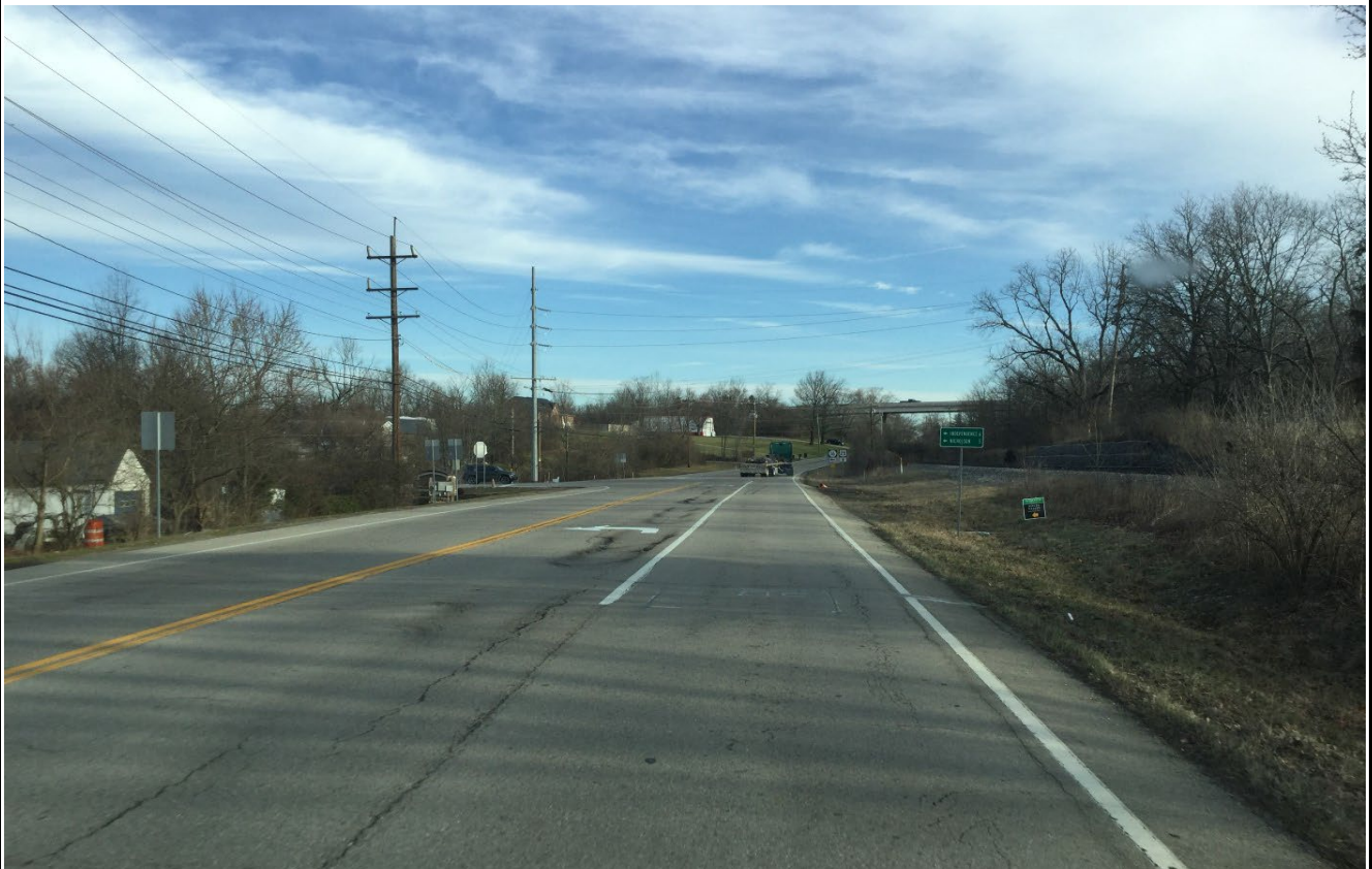
Exhibit 12: US-25 (Looking Northeast) Approaching Intersection with KY-16
