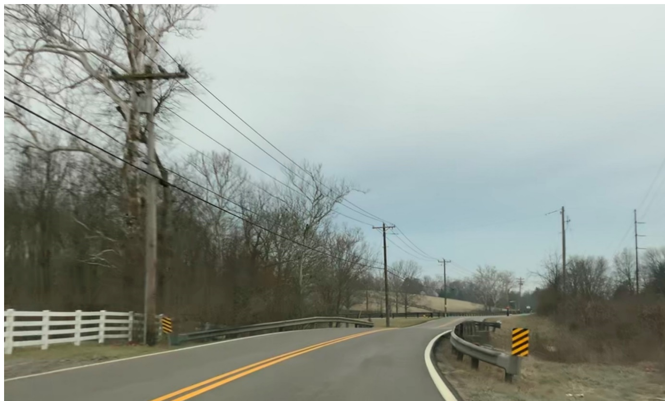
Exhibit 6: Culvert near Mile Point 1.3
