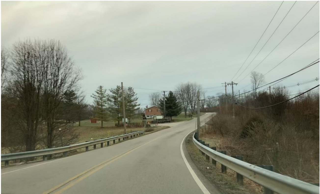
Exhibit 15: Hicks Pk Facing West at Culvert Between Richwood Church Rd and Toll House Rd
