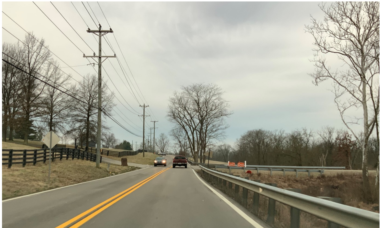
Exhibit 4: New Commercial Entrance near Mile Point 0.9
