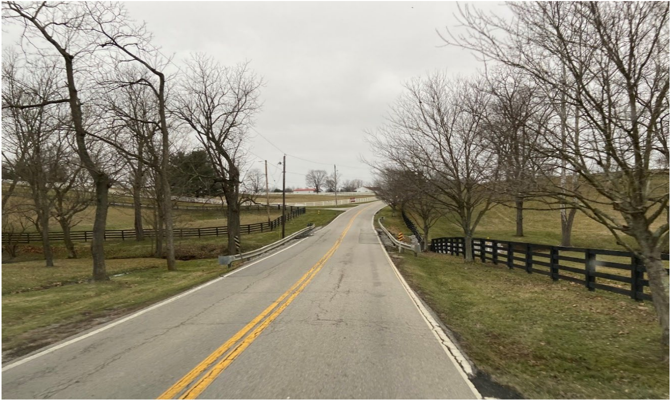
Exhibit 13: View of Narrow Bridge/Culvert and Sharp Curve on Richwood Rd near Mile Point 2.7
