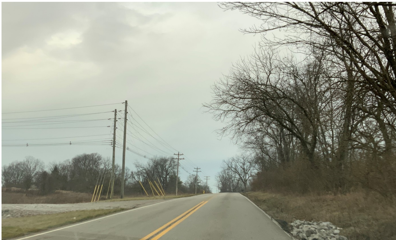
Exhibit 14: Hicks Pk Facing North near Intersection with KY-338
