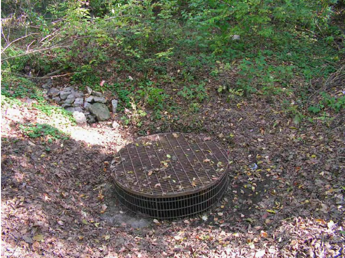
Sinkhole East of Chestnut Street
