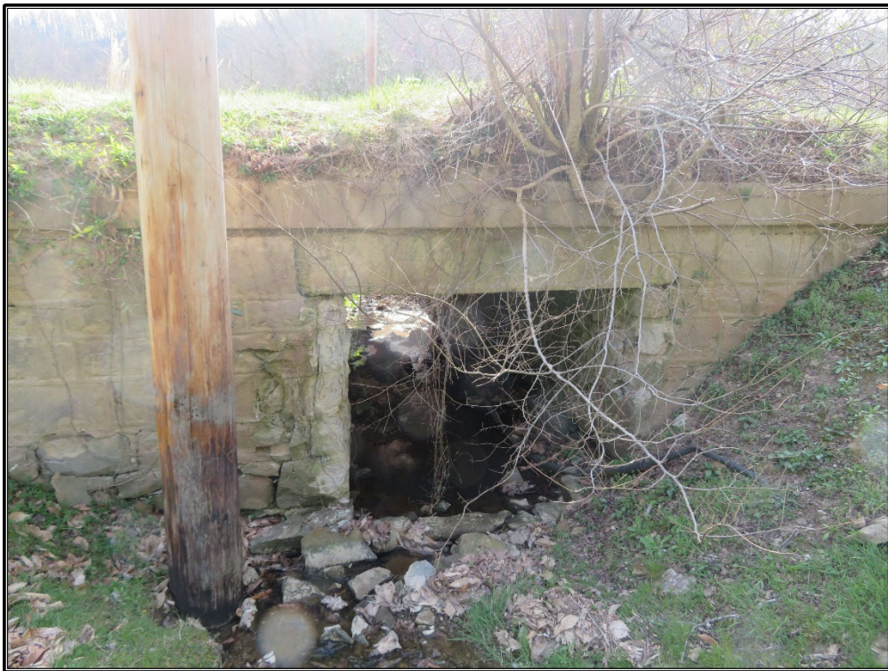
Figure A40. CRA E: Northeast elevation of the stone box culvert, looking west-southwest.
