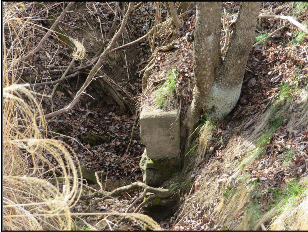
Figure A37. CRA B: East elevation of the concrete pipe culvert with mortared stone headwalls, looking south-southeast.
