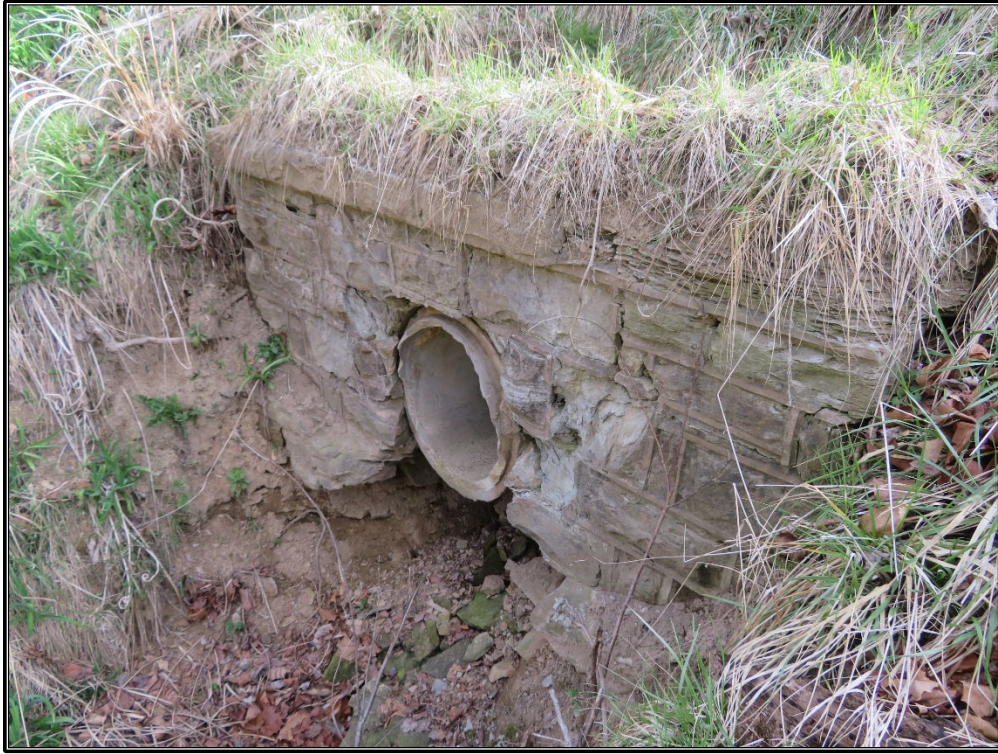
Figure A39. CRA C: West elevation of the concrete pipe culvert with mortared stone headwalls, looking northeast.
