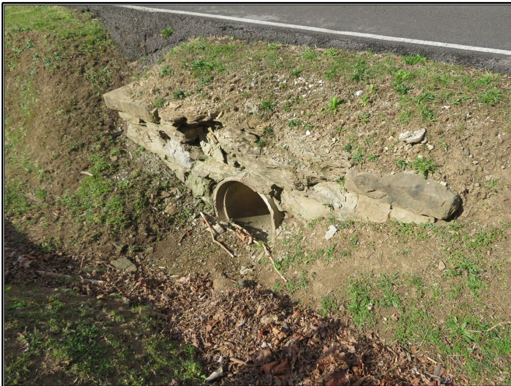
Figure A38. CRA C: East elevation of the concrete pipe culvert with mortared stone headwalls, looking west-southwest.
