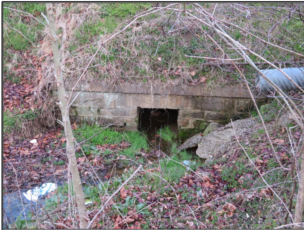
Figure A42. CRA E: Northeast elevation of the stone box culvert, looking west-northwest.
