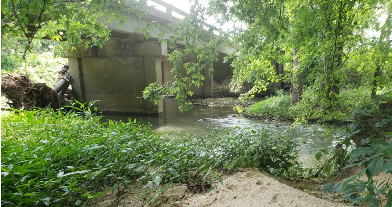
Figure 4: Looking east along KY 222, beneath 047B00046N. Note the sandy embankment (foreground), the lack of bedrock in the east embankment, and the fallen tree with roots intact against the north side of the central pier.
