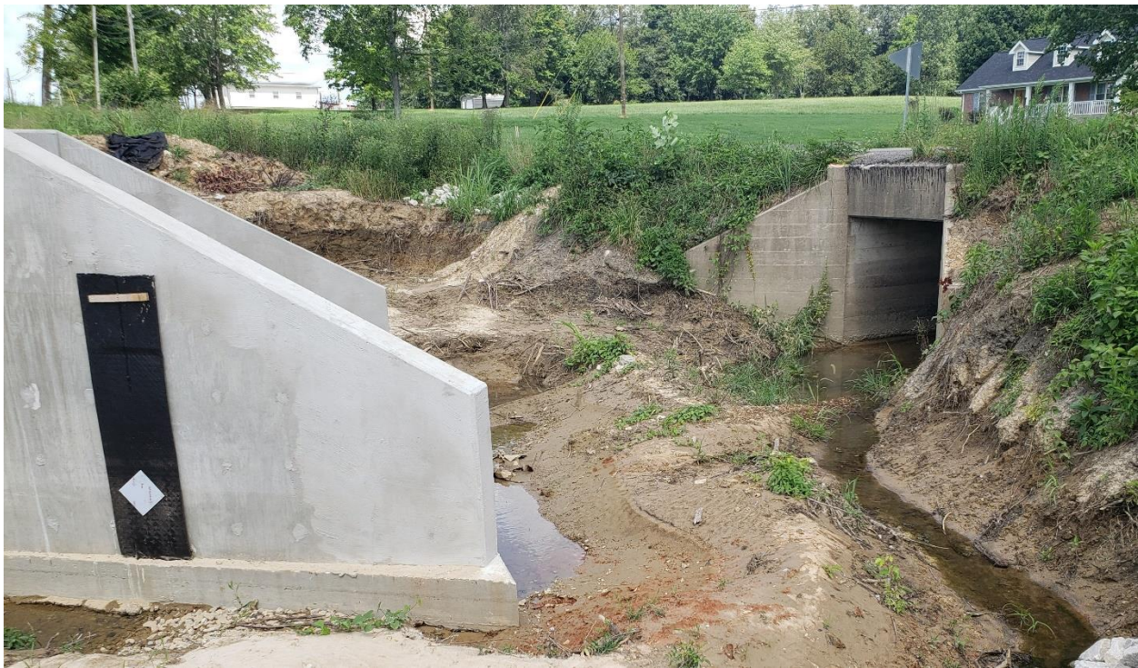
Figure 5: New culvert construction adjacent existing culvert under KY 222, both built on soil (slumped material).
