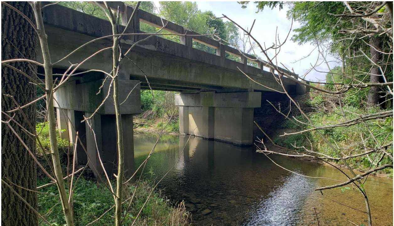
Figure 3: Underneath 047B00091N on KY 1904, looking south toward KY 222. Note the lack of bedrock in the south embankment.
