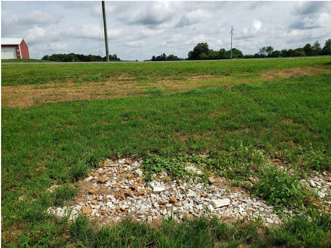
Figure 6: Repaired sinkhole along Bacon Creek Road, south of KY 222, in the project area.
