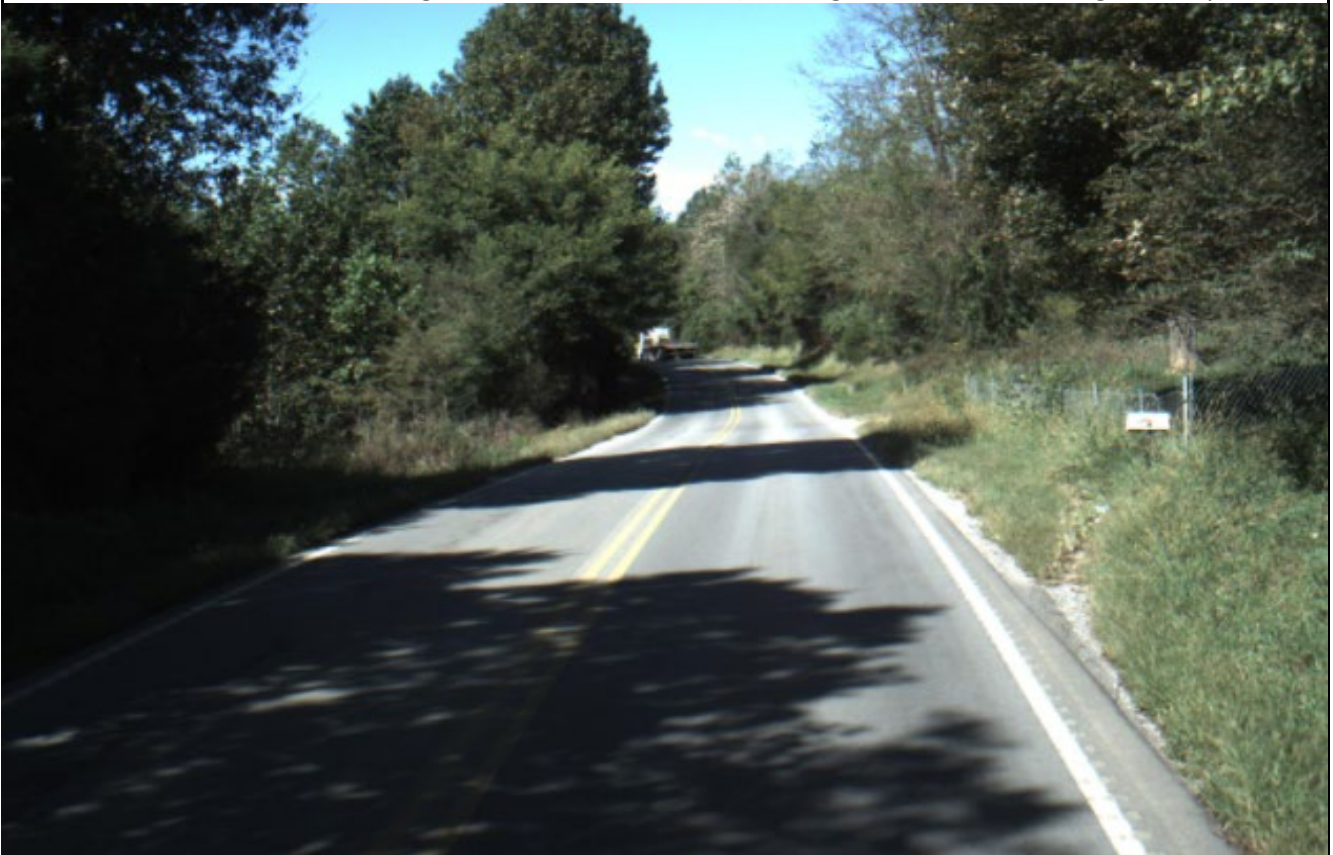
Photo 4: Near the end of the project area facing north toward Scottsville
