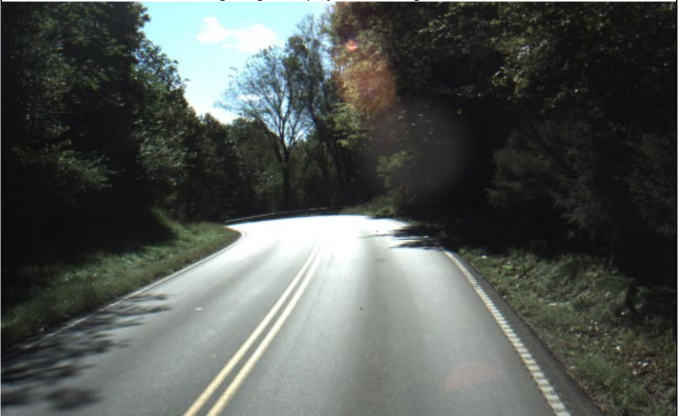
Photo 2: Main curve facing south toward Fountain Run (showing the vertical curvature)
