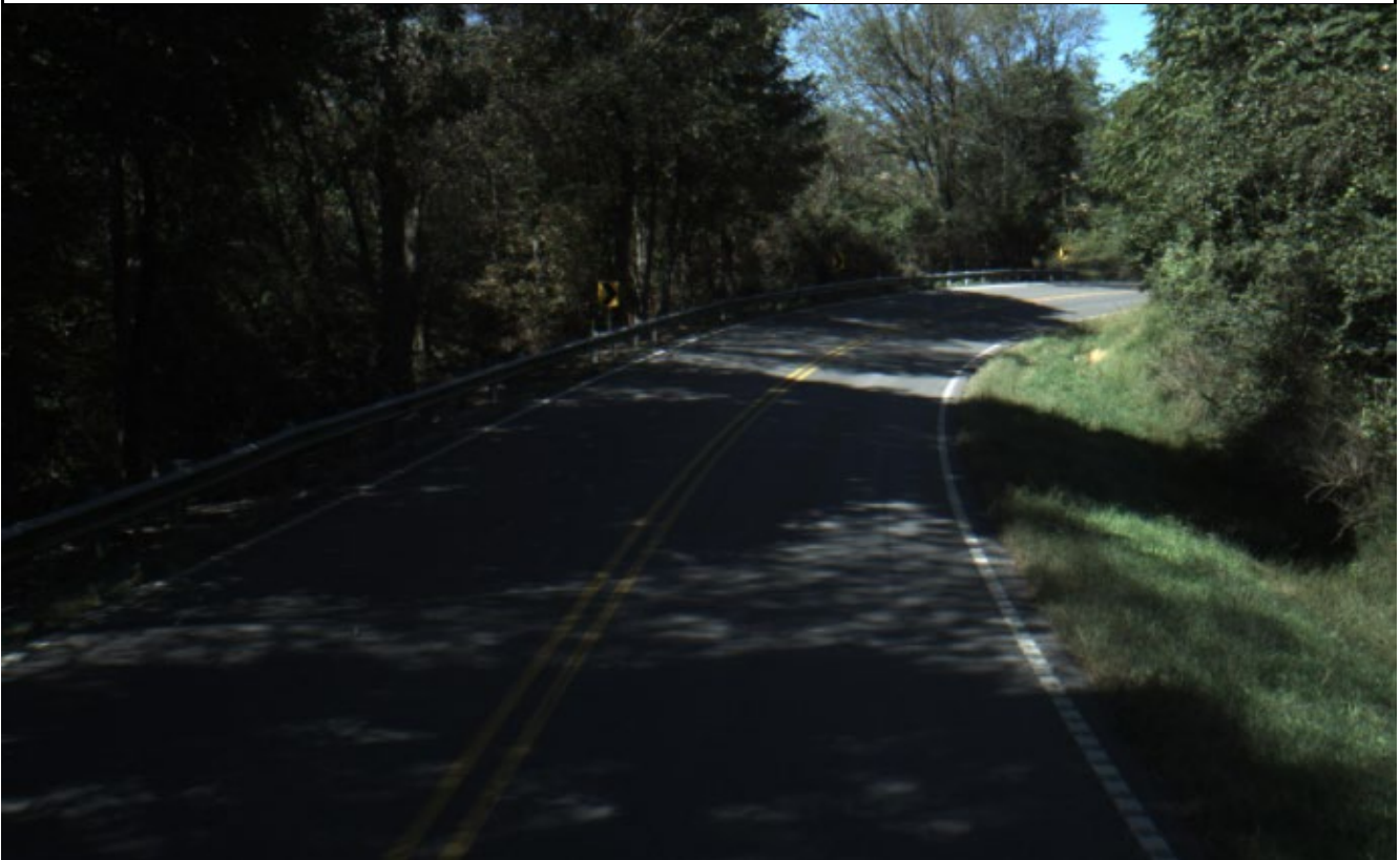
Photo 3: Main curve facing north toward Scottsville (showing issue of trees shading roadway)
