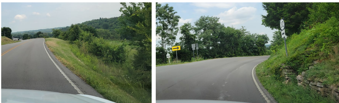
Figure 10: Steep Topography beyond Shoulders
