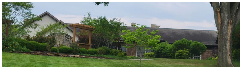
Figure 22: Hospice Care Center
