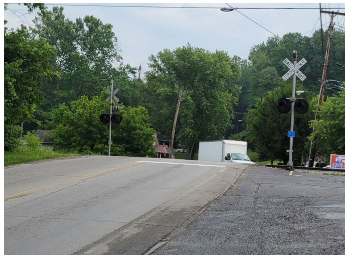
Figure 7: Steep Vertical Curve Limits Visibility
