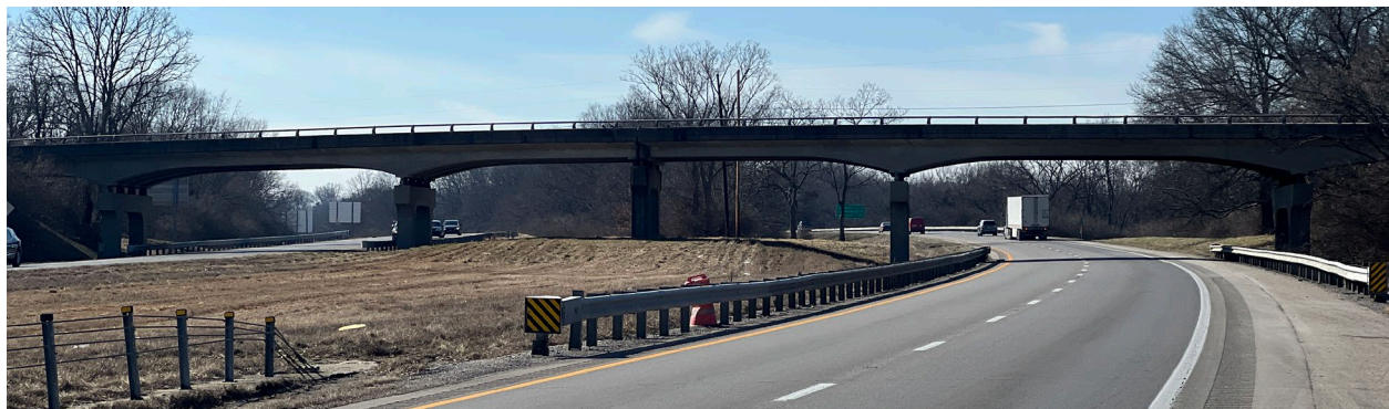
Figure 6: KY 2821 Overpass seen from Westbound I-64
