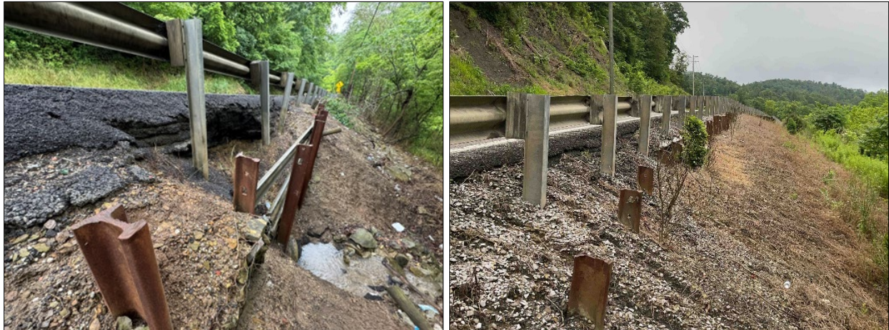
Figure 38. Representative Cribbing Not Meeting Modern Design Guidelines
