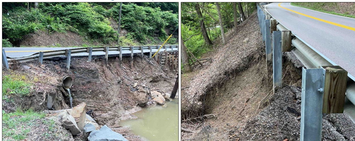
Figure 40. Representative Unstable Slopes
