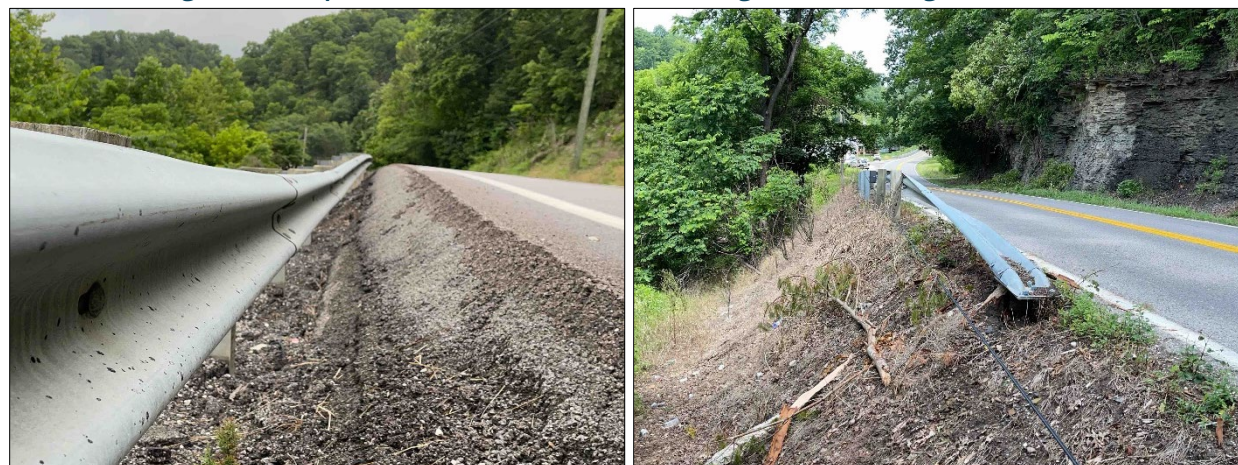
Figure 36. Representative Guardrail Not Meeting Modern Design Guidelines
