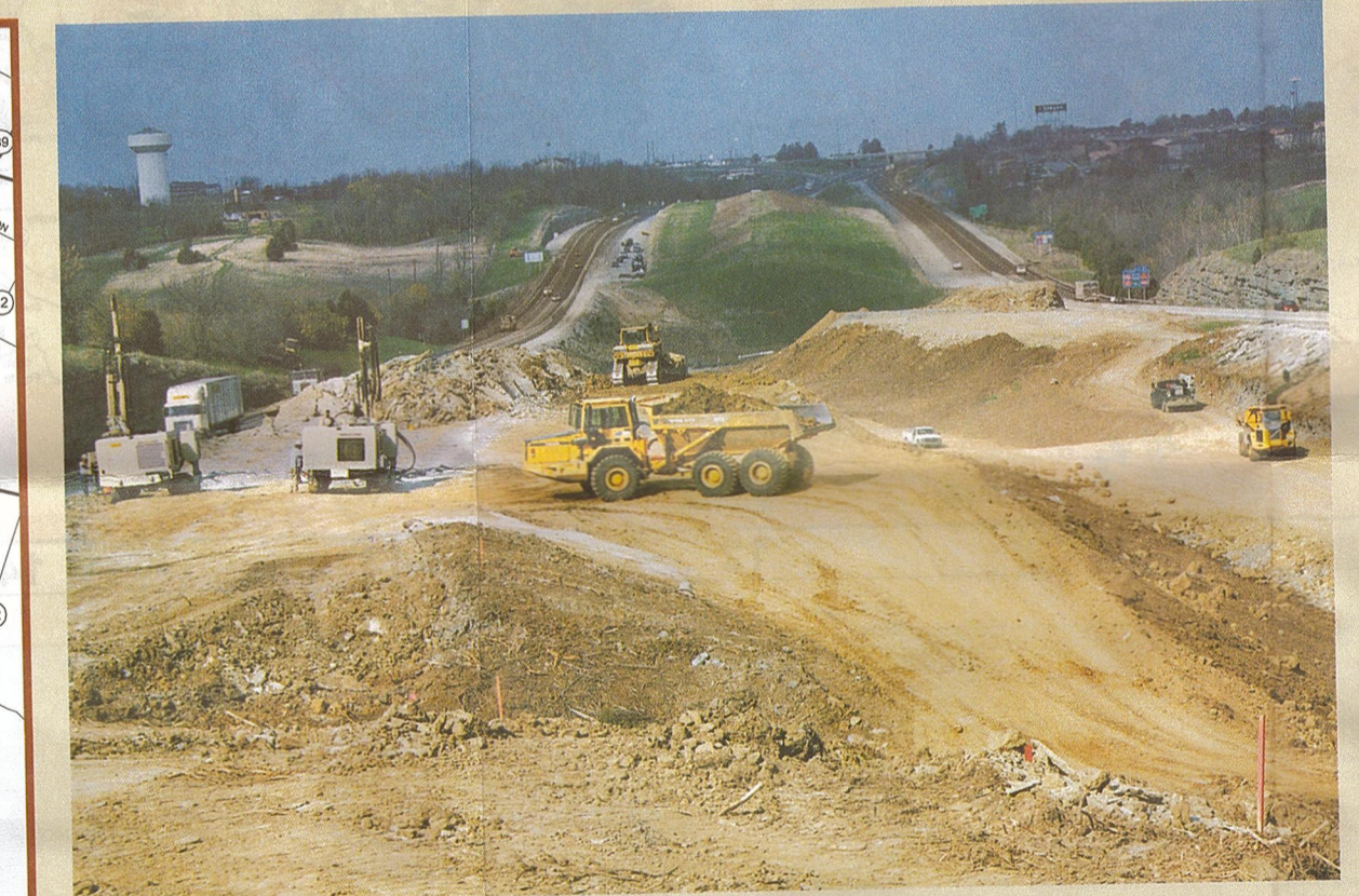
Reconstruction on I-75 in Madison County
