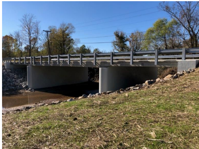
A new bridge on KY 339 over Massac Creek reopened to traffic on Nov. 1.
