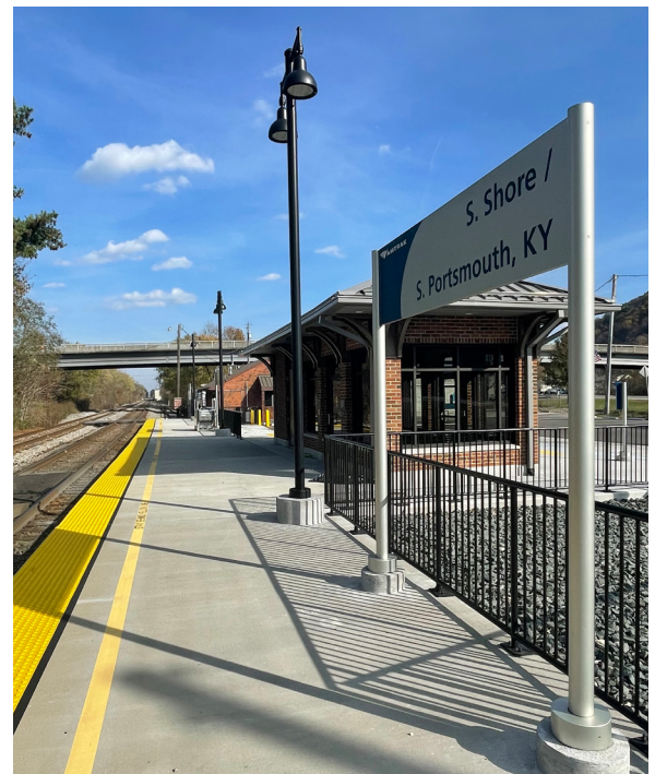
Source: Kentucky Transportation Cabinet
