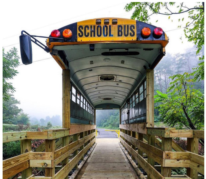
Source: Kentucky Transportation Cabinet
