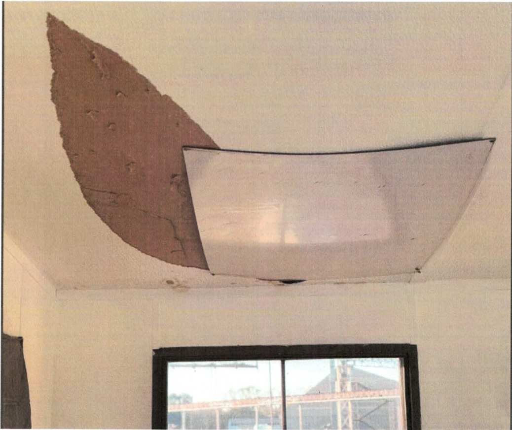
Deteriorated Ceiling – Above Scale Operator Desk
