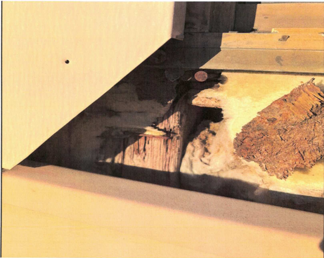
Deteriorated Window Frames
