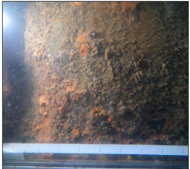
Photograph 12 Underwater view of typical condition of sheet piles.
