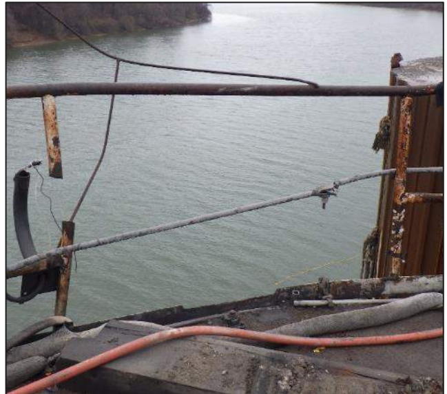
Photograph 8 View of broken guardrail.
