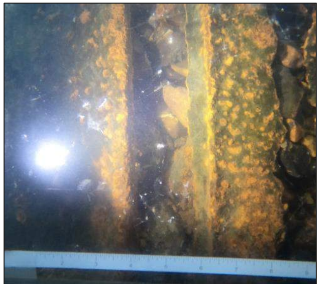
Photograph 12 Underwater view of split interlock between Sheet 2 and Sheet 3.
