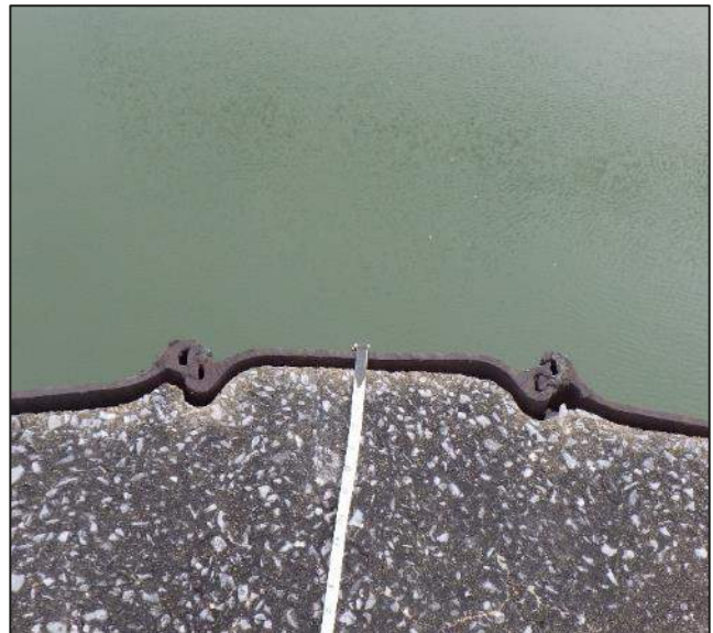
Photograph 8 View of the gap between the cap and the sheets at Sheet 10 through Sheet 12.
