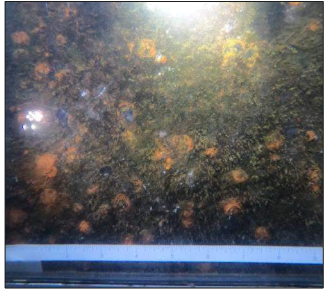
Photograph 14 Underwater view of typical sheet pile condition.
