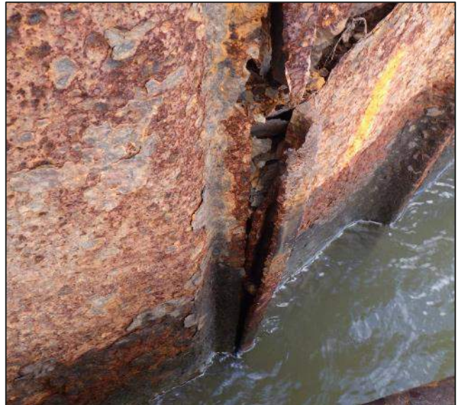
Photograph 8 View of split interlock between Sheet 1 and Sheet 2.
