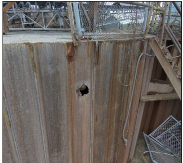
Photograph 12 View of hole on Sheet 62.
