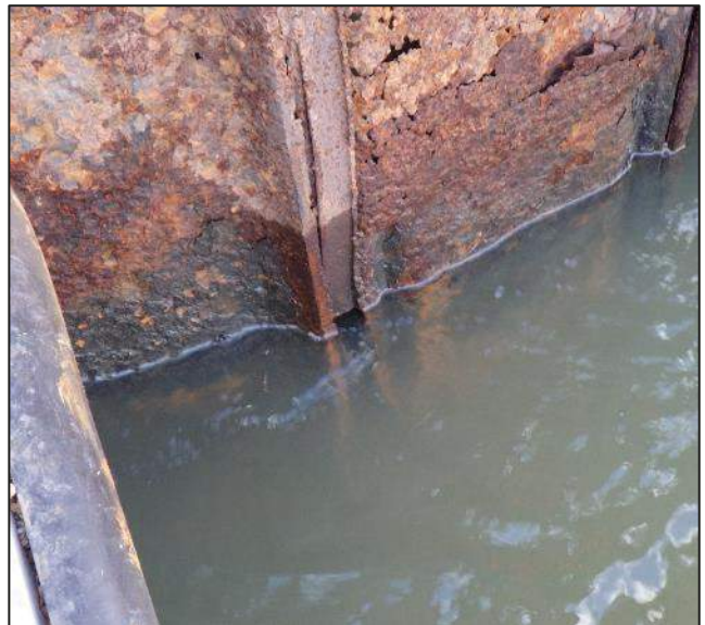
Photograph 8 View of split interlock between Sheet 2 and Sheet 3.
