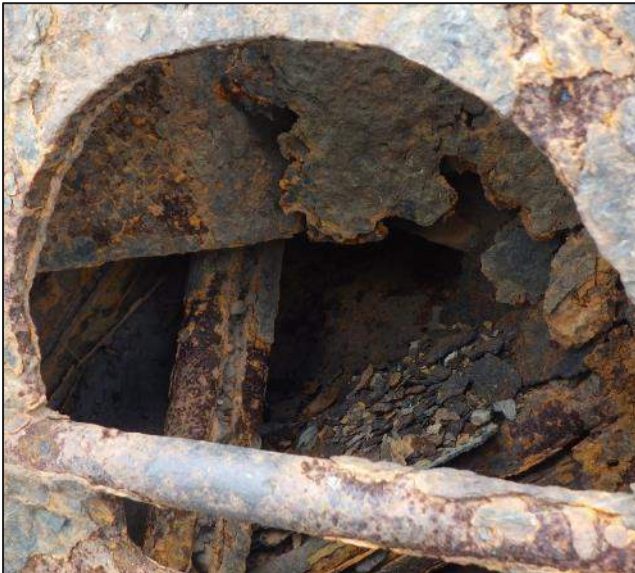
Photograph 7 View of split in pan sheet.
