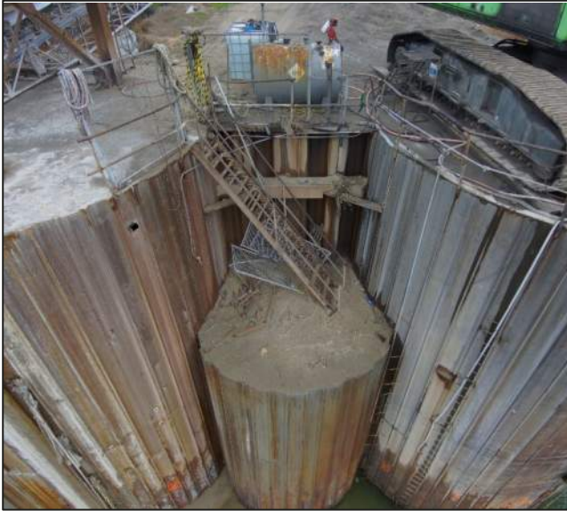
Photograph 13 View of damaged staircase centered at Sheet 56.
