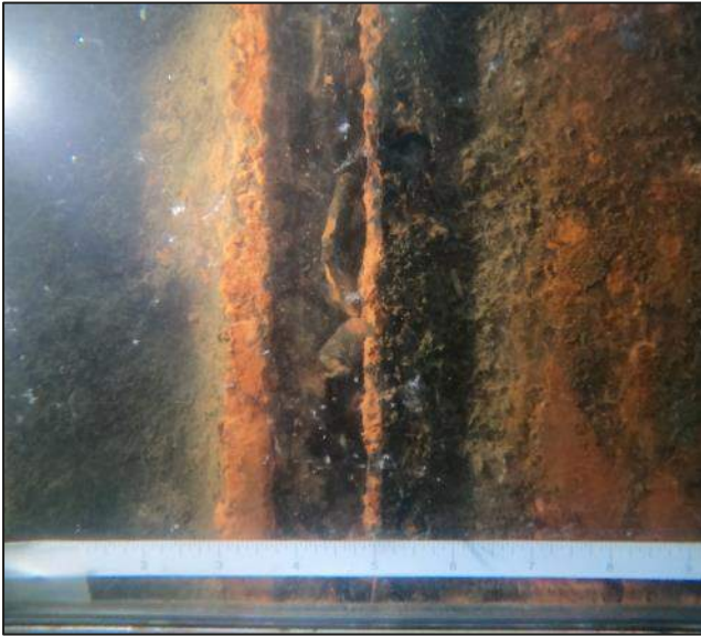
Photograph 13 Underwater view of split between Sheet 2 and Sheet 3
