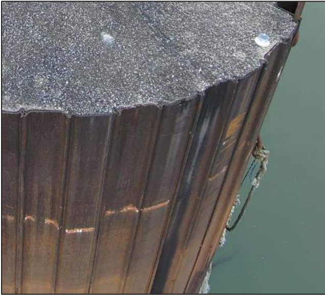
Photograph 9 View of impact damage on Sheet 5.
