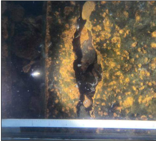
Photograph 13 Underwater view of split web on Sheet 2.
