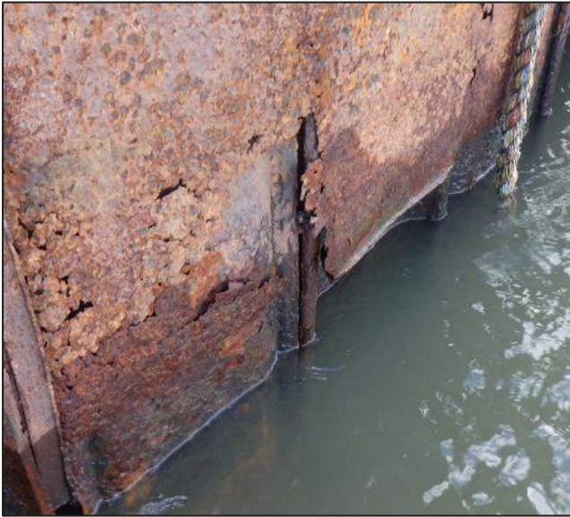
Photograph 9 View of split interlock between Sheet 1 and Sheet 2.
