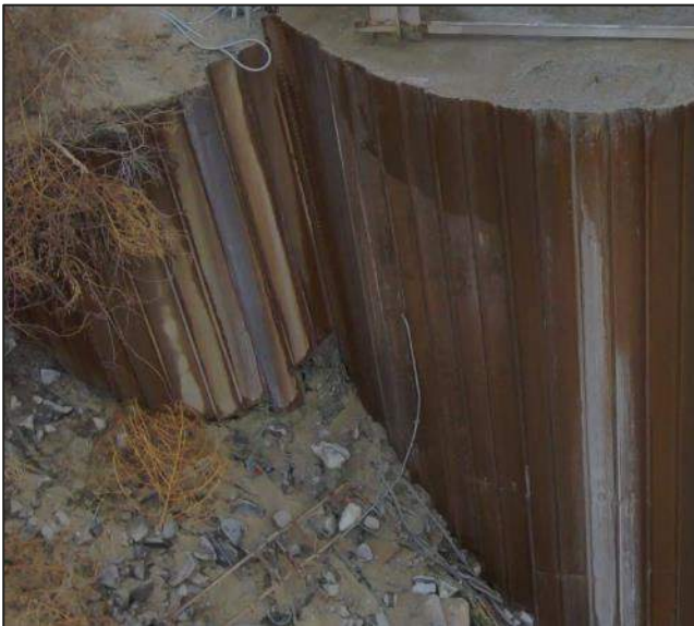
Photograph 15 View of erosion and undermining of the containment sheets attached to Sheet 31.
