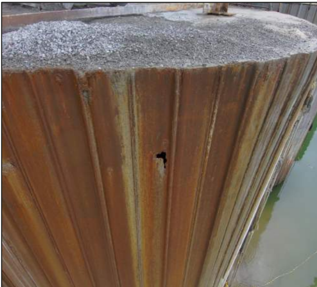
Photograph 11 View of hole on Sheet 7.
