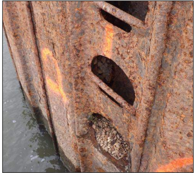
Photograph 6 View of split pan sheet with active loss of fill on Sheet 1.
