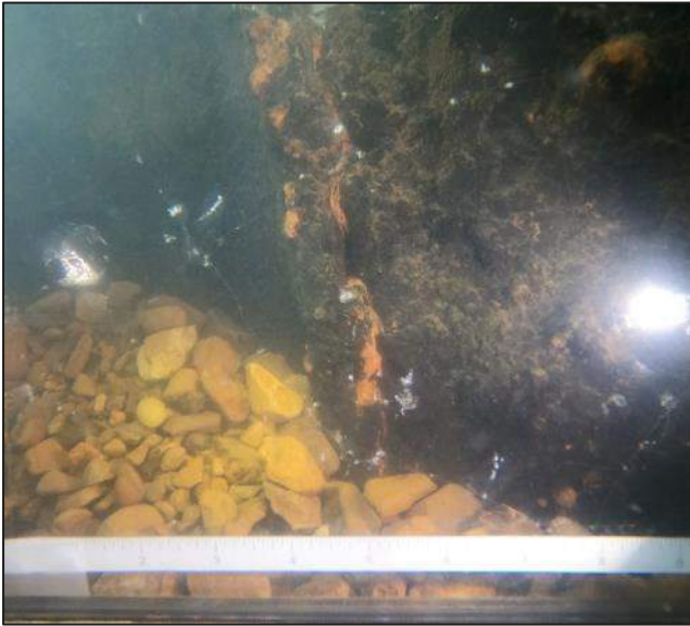
Photograph 13 Underwater view of split between Sheet 48 and Sheet 1
