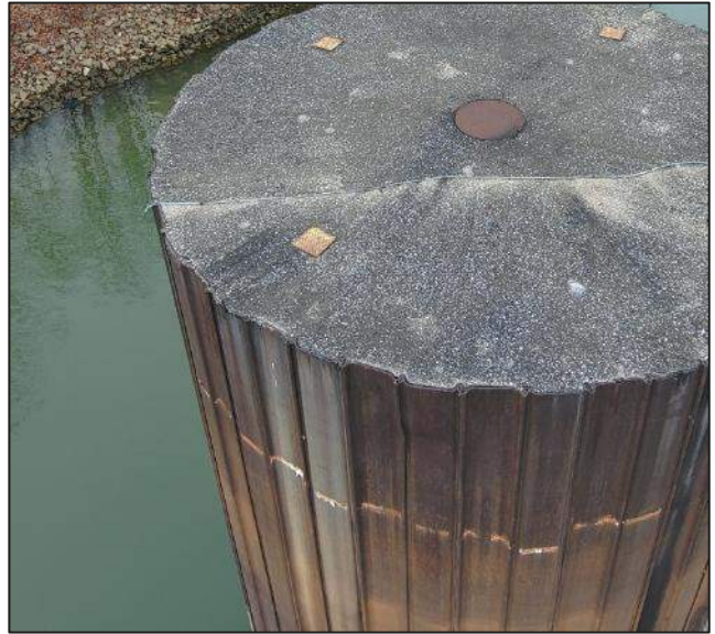
Photograph 10 View of impact damage on Sheet 10 through Sheet 12.
