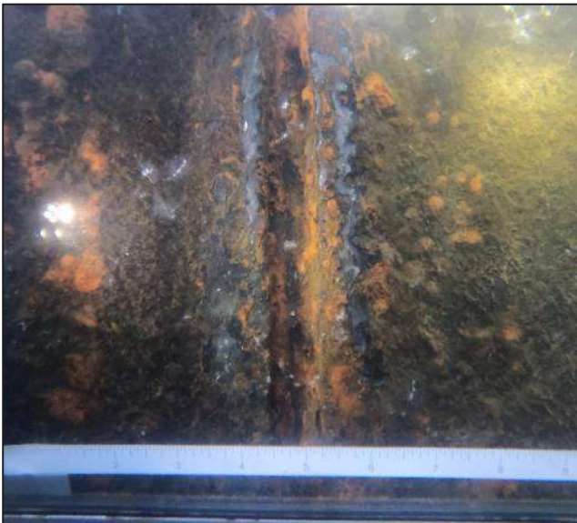
Photograph 15 View of split interlock between Sheet 72 and Sheet 1.
