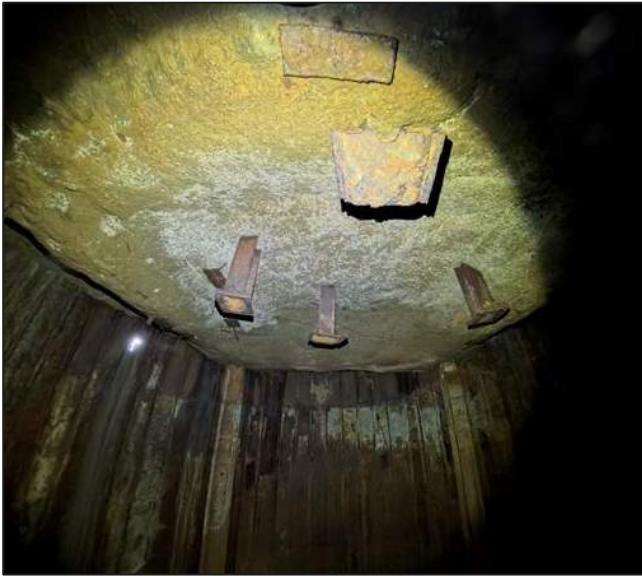
Photograph 9 View of the bottom side of the concrete cap and bases of the unloader columns.
