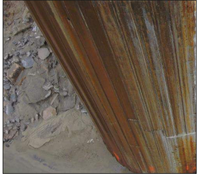
Photograph 14 View of isolated impact damage on Sheet 5 and Sheet 6.
