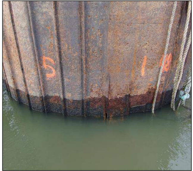
Photograph 10 View of the typical waterline condition.
