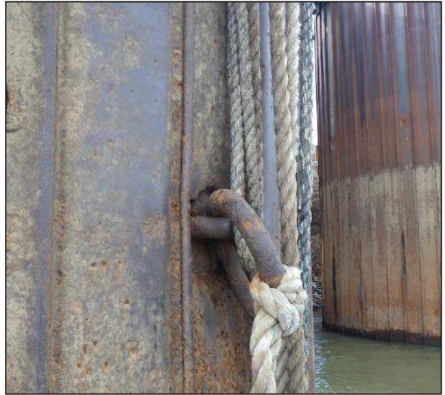
Photograph 10 View of impacted mooring ring on Sheet 37.
