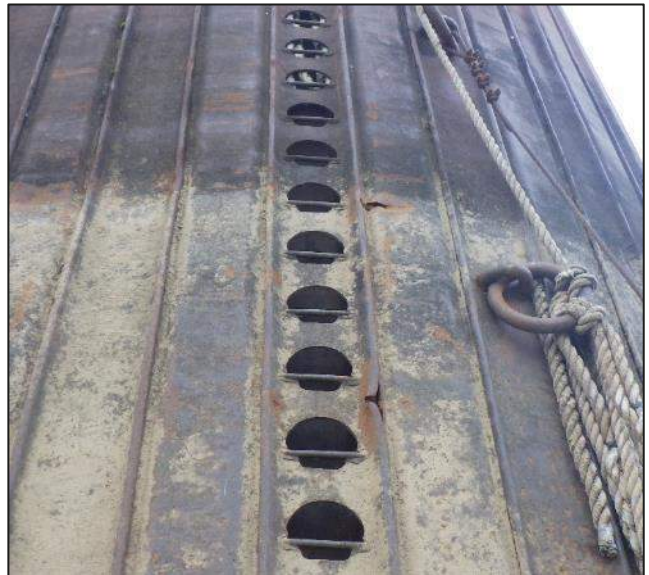
Photograph 8 View of splits on Sheet 1.
