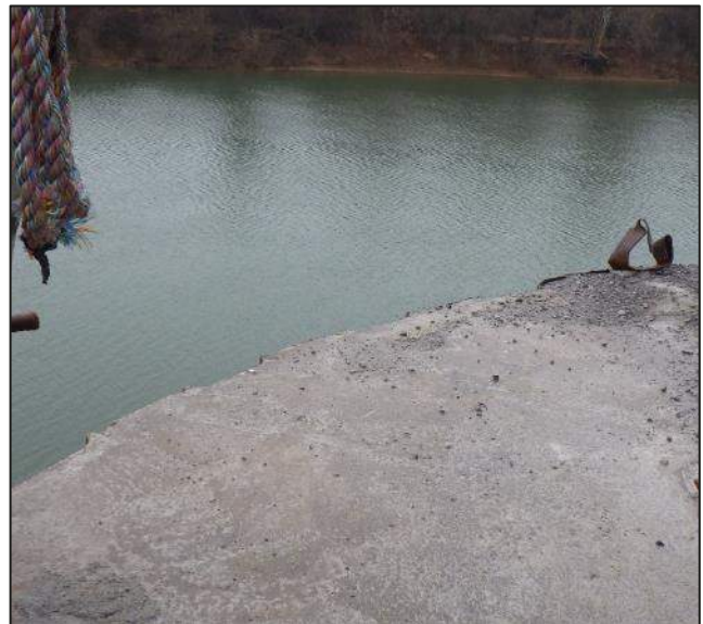
Photograph 8 View of missing guardrail on the channel side of the cell.
