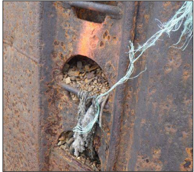
Photograph 6 View of pan sheet with active loss of fill.
