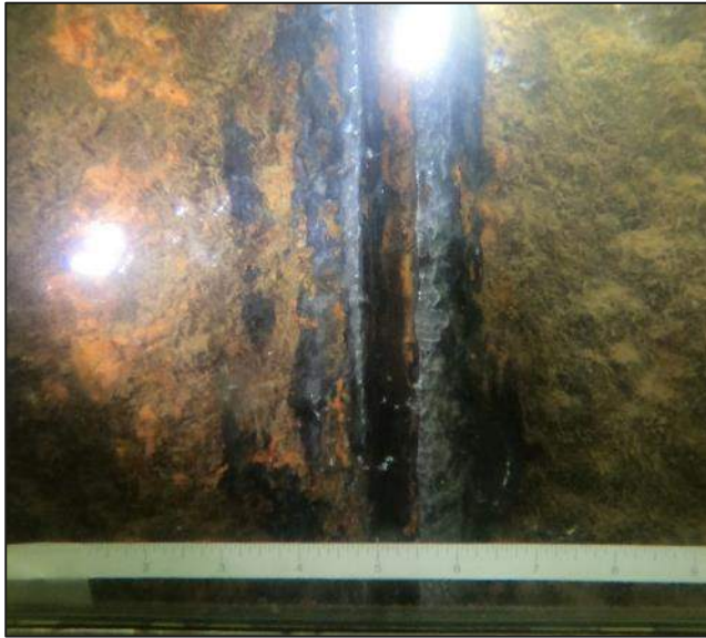
Photograph 13 Underwater view of split interlock between Sheet 1 and Sheet 2.
