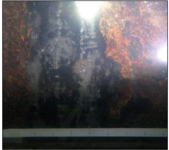
Photograph 10 Underwater view of typical sheet pile condition.
