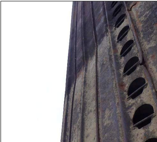
Photograph 7 View of impact damage on Sheet 3.
