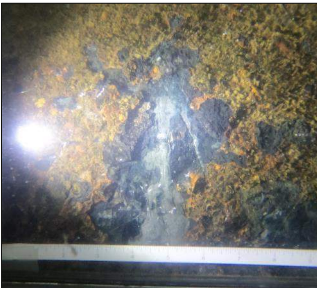
Photograph 11 Underwater view of typical sheet pile condition.
