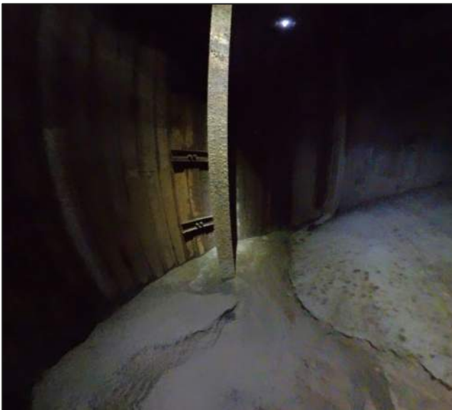
Photograph 7 View of lost ballast material inside cell.
