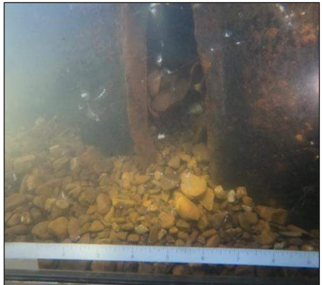
Photograph 12 Underwater view of split between Sheet 2 and Sheet 3.
