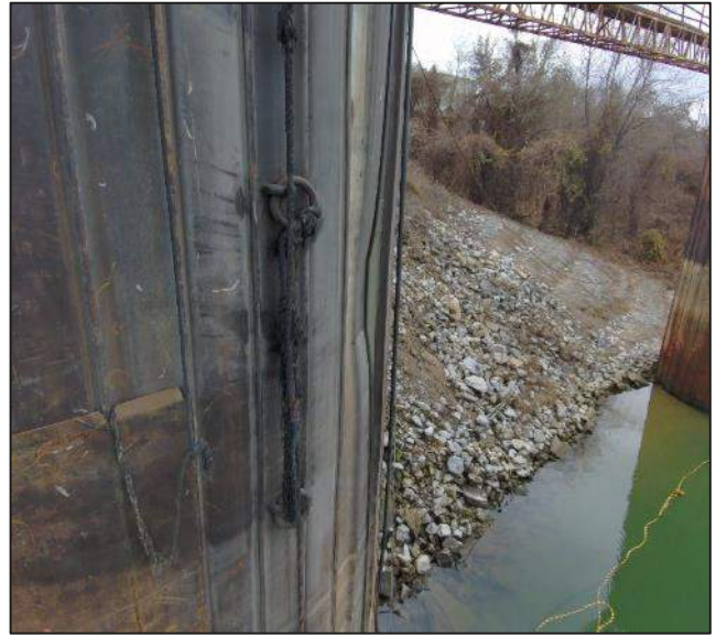
Photograph 10 View of impact damage at Sheet 67.
