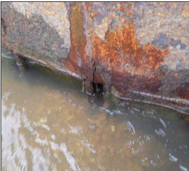
Photograph 7 View of split interlock between Sheet 2 and Sheet 3 showing exposed fill material.
