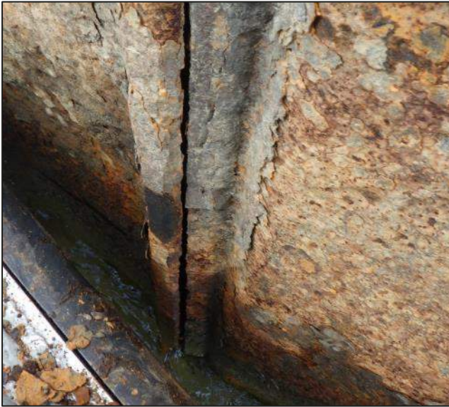
Photograph 9 View of split interlock between Sheet 2 and Sheet 3.
