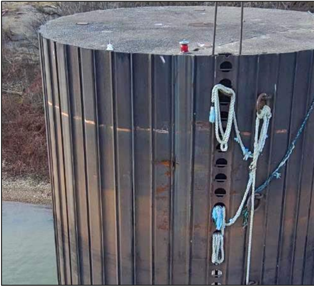
Photograph 9 View of interlock hole between Sheet 3 and Sheet 4.
