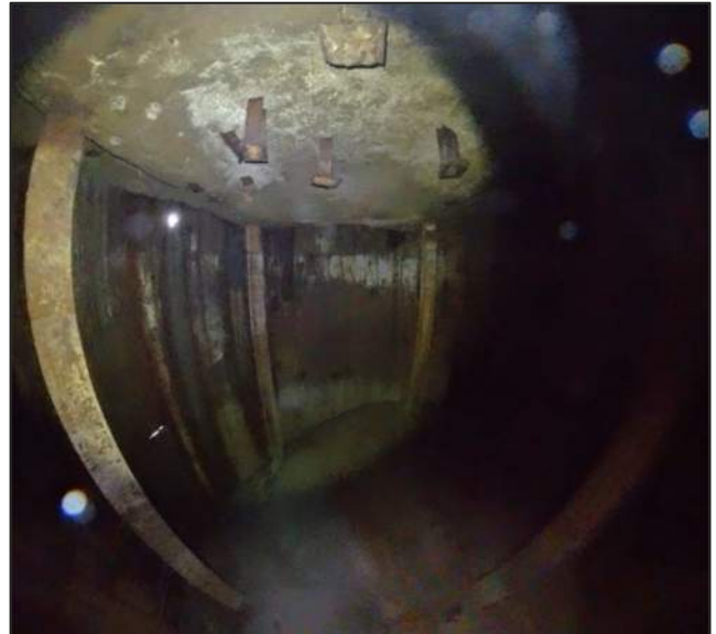
Photograph 10 View of the columns supporting the concrete cap.
