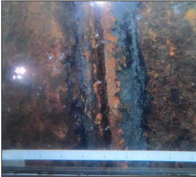
Photograph 9 Underwater view of split interlock between Sheet 37 and Sheet 38.
