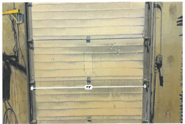
Existing dock doors 1 and 2—current door width 7'3" and dock plate width 6'1"
