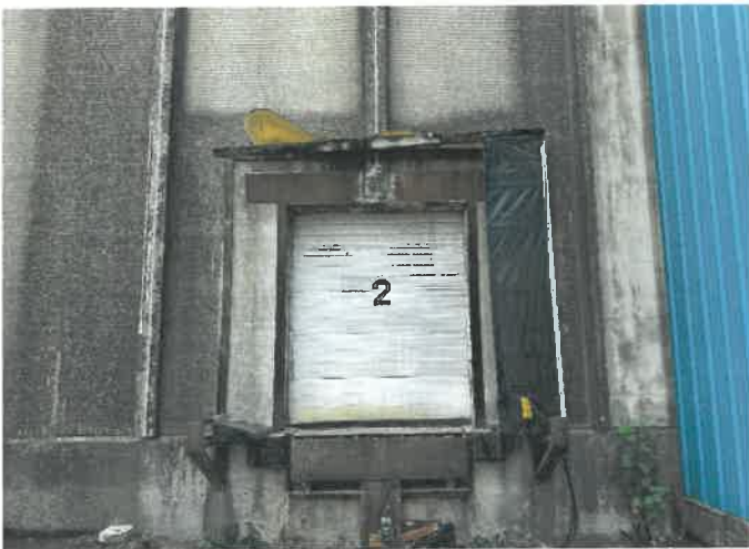
Existing dock doors 1 and 2—current door width 7'3" and dock plate width 6'1"
