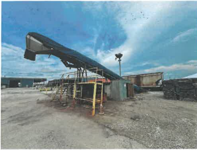
Rail-to-truck loading chute
