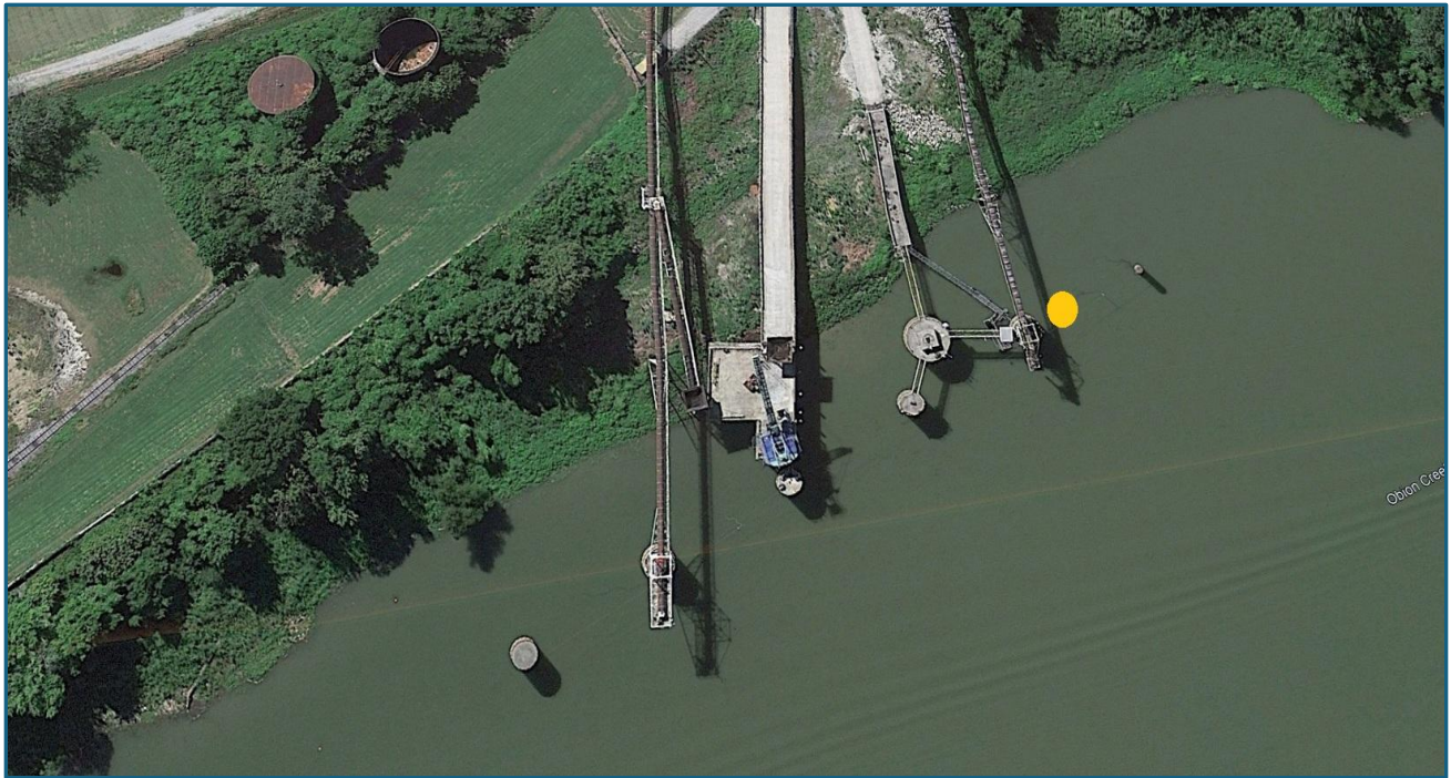
Photo # 2 - Aerial of New Cell Location
