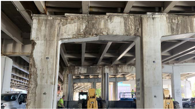
Bridge 056B00183N: Exposed rebar and concrete spalling
