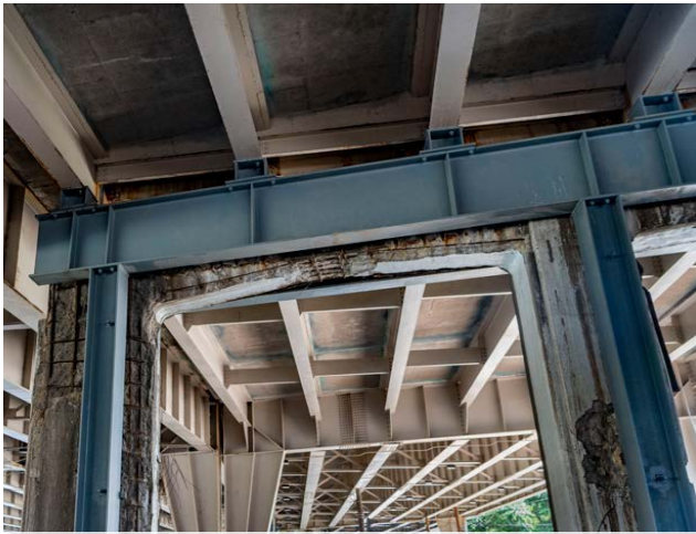
Bridge 056B00183N, E. Kentucky & S. Brook Street, temporary support for crumbling piers
