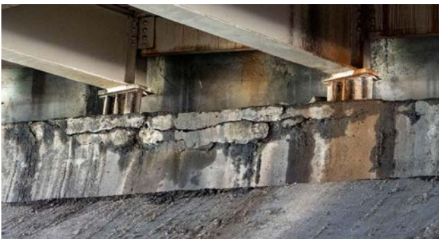
Bridge 056B00209N, Phillips Lane, deteriorating concrete abutment
