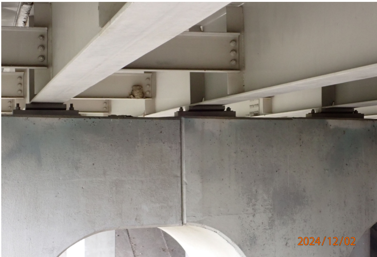
Typical fixed bearings at Pier 2
