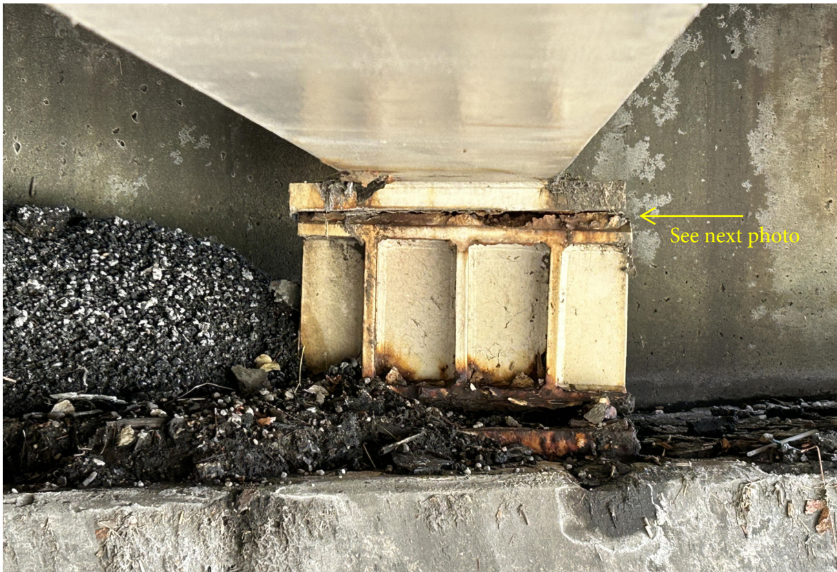
At Abutment 1-Beam 4, the rocker bearing is laterally rotated with an 11/16 " gap between the sole plate and rocker on the west side only. Note asphalt piled on seat.
