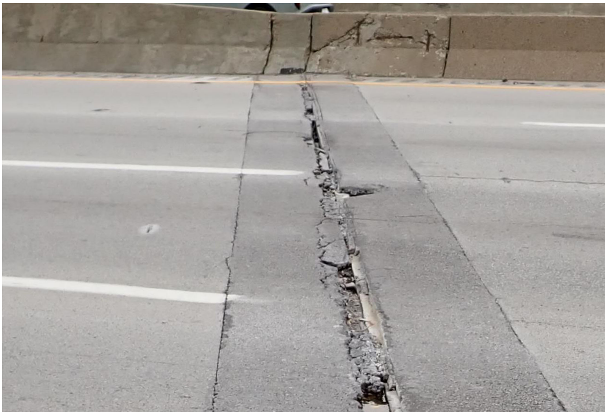
Asphalt plug joints are breaking up and/or missing throughout the traffic lanes (Abutment 4 joint shown). Note fracture in median barrier.
