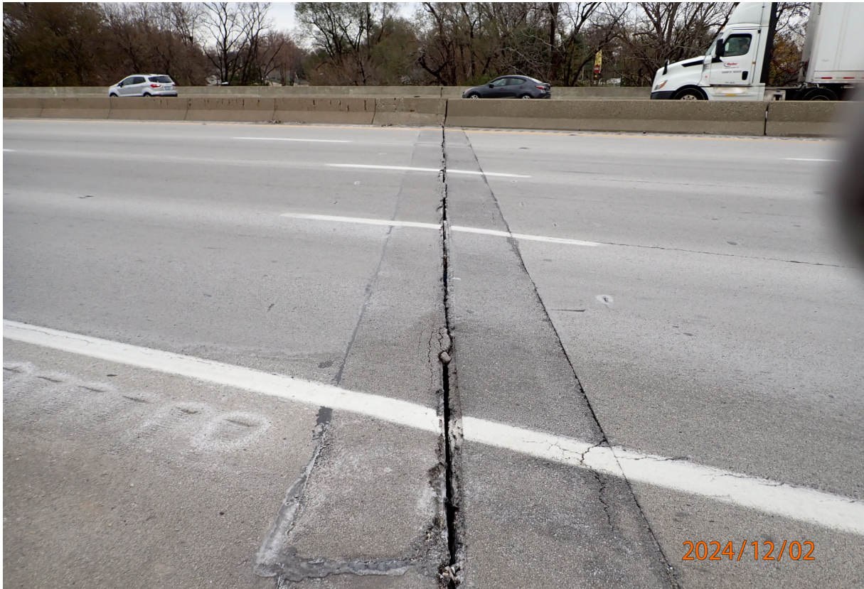
Asphalt plug joint over Abutment 1 (SB)
