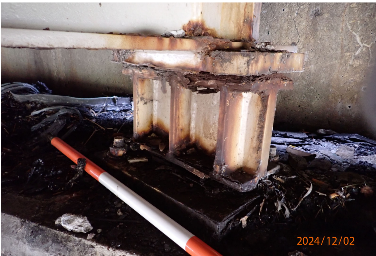
Abutment bearings have flaking corrosion and pack rust, primarily between the rockers and masonry plates, with heavier corrosion at the longitudinal joint and exterior beams (Beam 16 at Abutment 1 shown).
