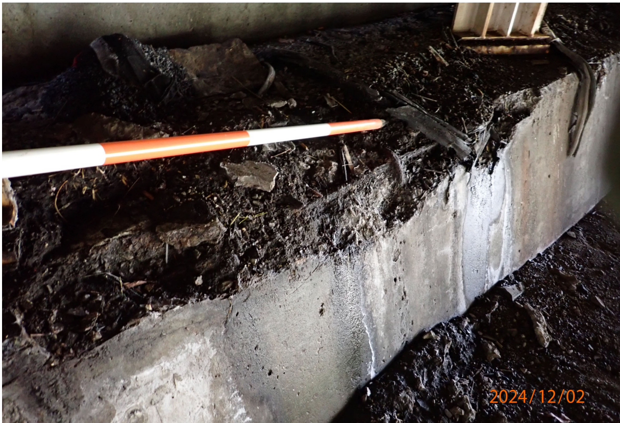
Abutment 1 cap has 6' L x 1' W x 9" H spalling with exposed rebar in Bay 8.
