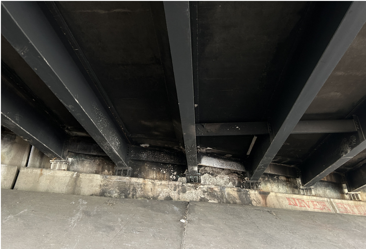
There is soot from fires on Beams 12-20 at Abutment 4.
