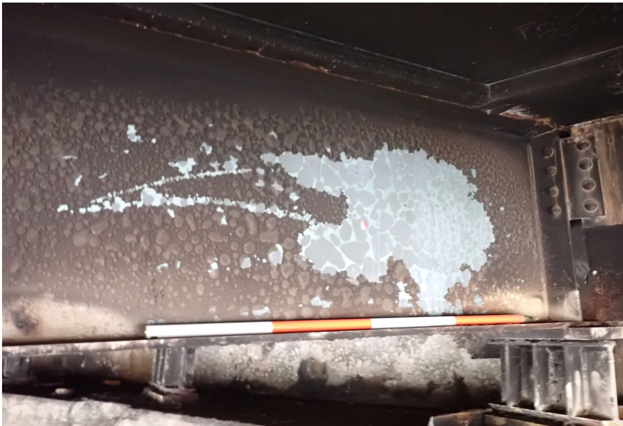
Paint bubbling and failure from fires at Beam 15
