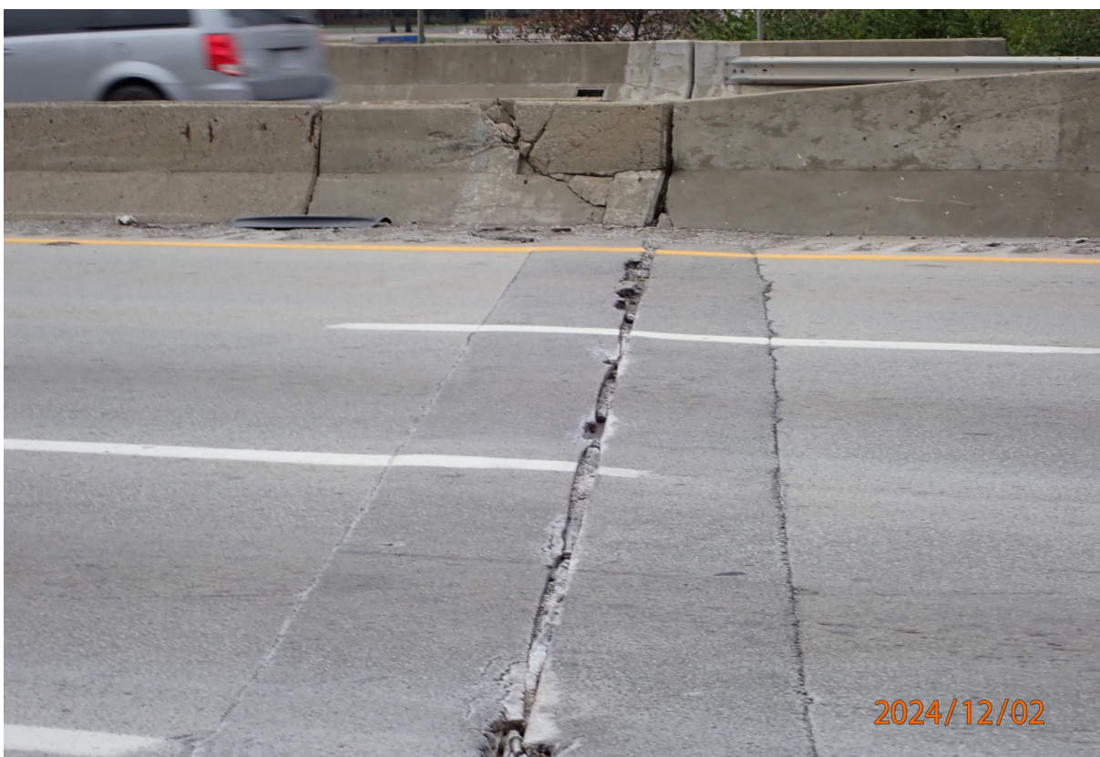
Median railing has a 5-foot-long diagonal fracture at the north end, with spalling along both faces and exposed rebar on the west face. Note failed asphalt plug joint.
