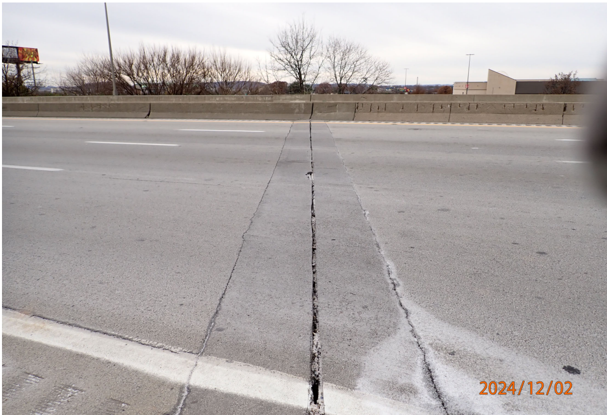
Asphalt plug joint over Abutment 1 (NB)
