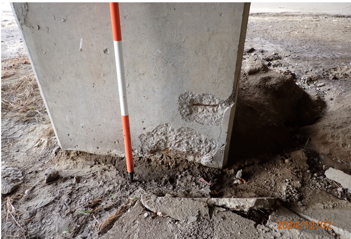
Pier 2-Column 3 has spalling with exposed rebar at the bottom of the south face, 1.5-foot-diameter by 1-inch-deep.
