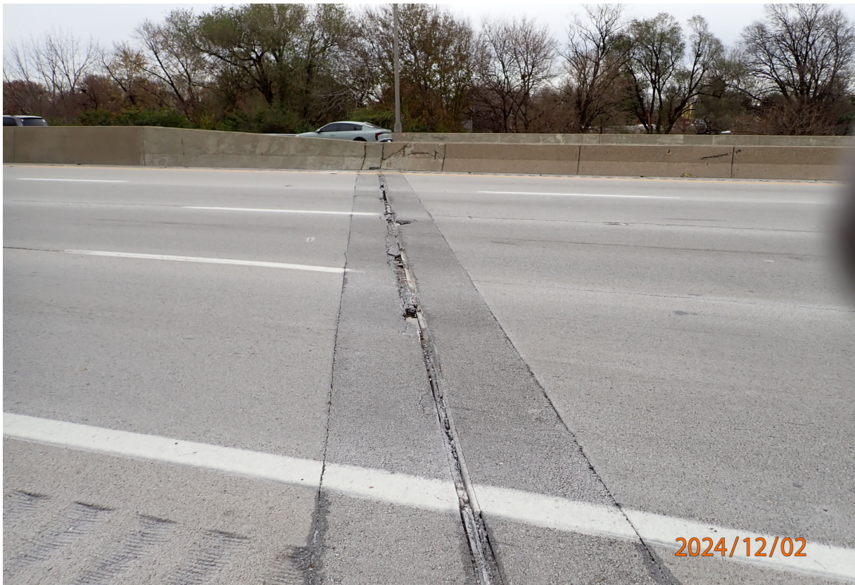
Asphalt plug joint over Abutment 4 (SB)
