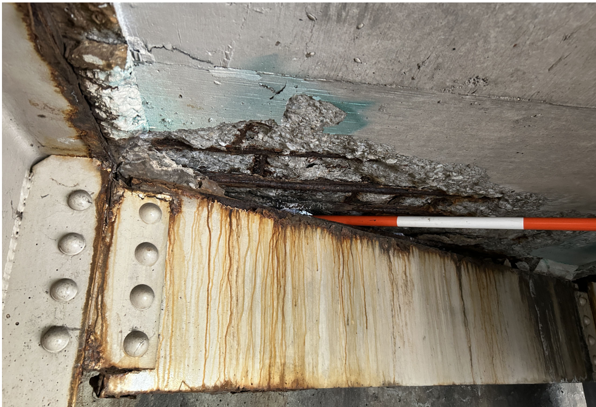
Bay 6 soffit has a 4' W x 2' L x 3" D spall at Abutment 1. Note daylight visible through failed joint.
