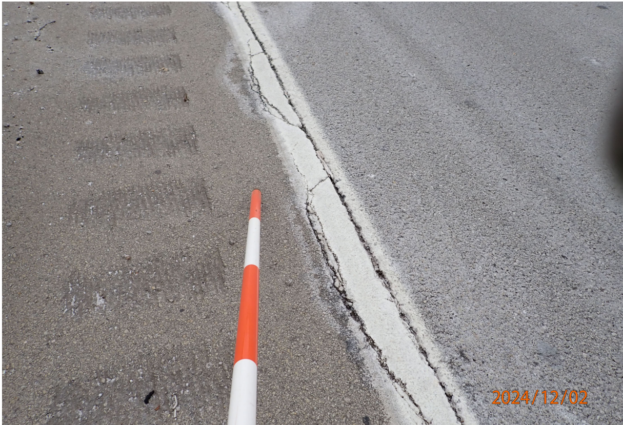
Overlay has intermittent unsealed longitudinal cracking along the right NB edge line.
