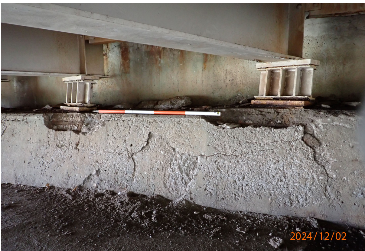
Abutment 4 cap has spalls with exposed rebar at Beams 5 and 6, each roughly 4' L x 1' H x 7" D. There are also large delaminations at this location.
