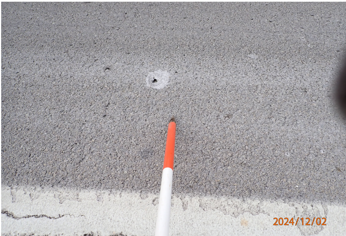
Overlay has minor wearing in the traffic lanes, plus some 1-inch-wide spalls in the NB lanes in Span 1.
