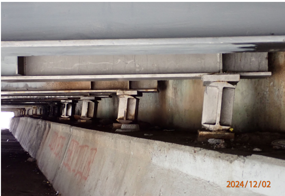
Abutment bearings are expanded at 28° F (tolerable alignment, inconsistent with temperature; looking west along Abutment 4 shown).
