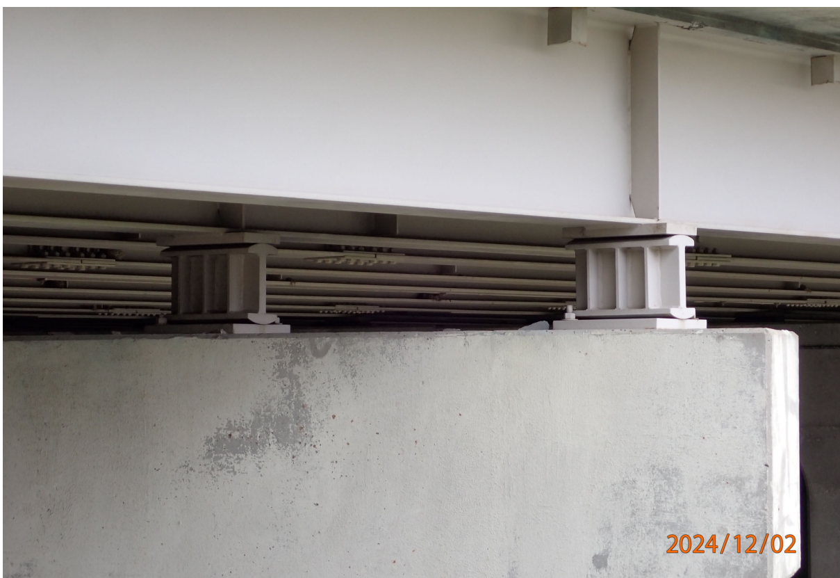
Typical rocker bearings at Pier 3
