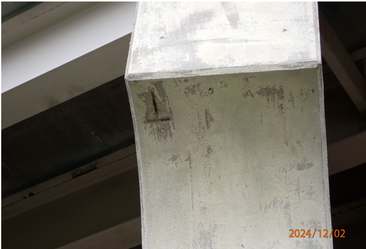
Pier 3 cap has an 8-inch-diameter spall with exposed rebar on the bottom face at the west end.
