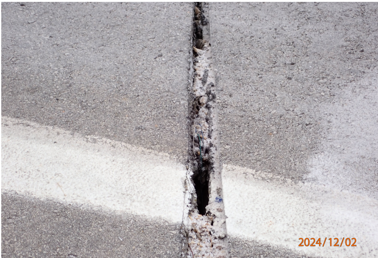
Asphalt plug joints are breaking up and/or missing throughout the traffic lanes (Abutment 1 at right NB edge line shown).
