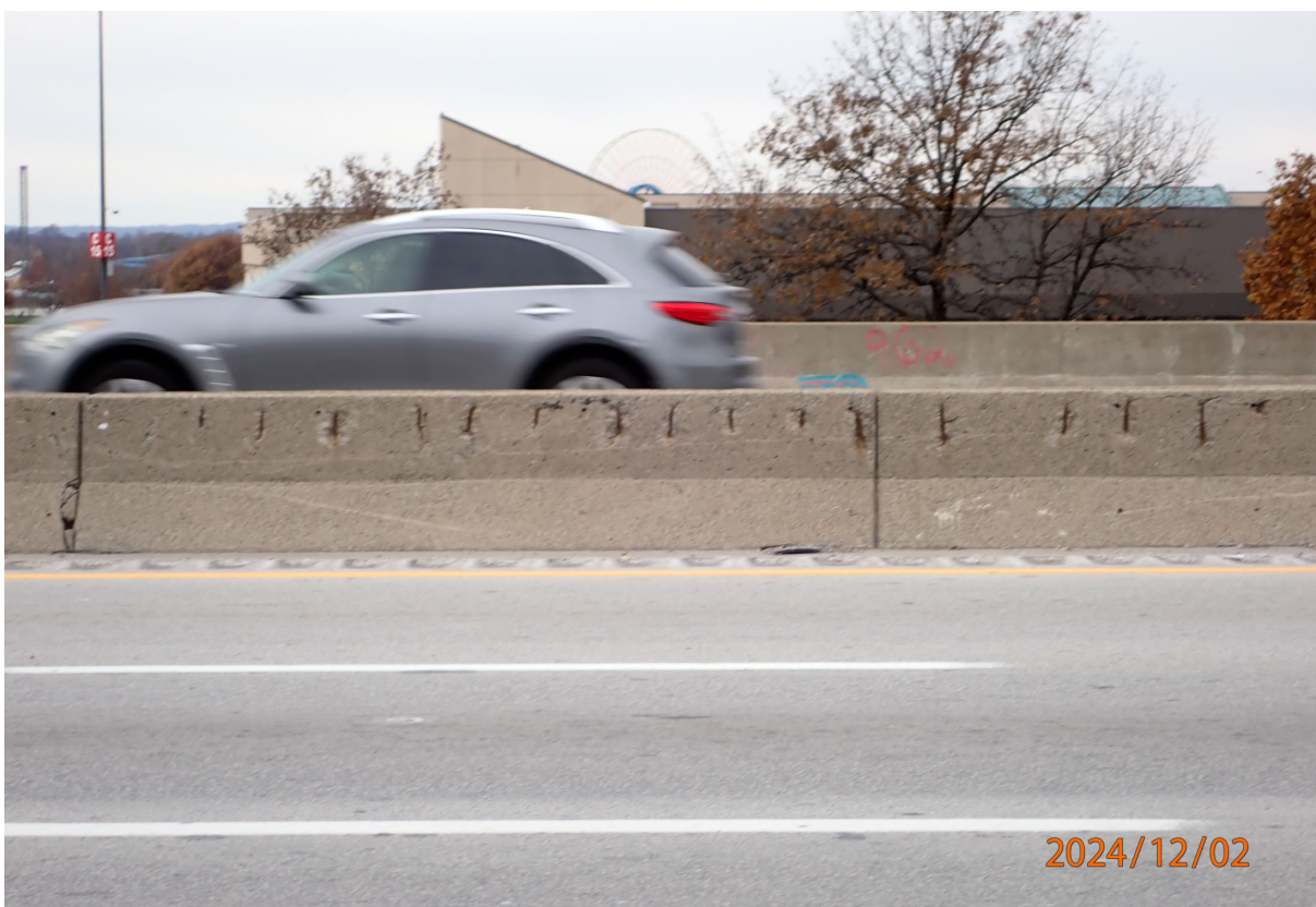
Median rails have numerous spalls with exposed rebar; spalling is more widespread on the NB rail.
