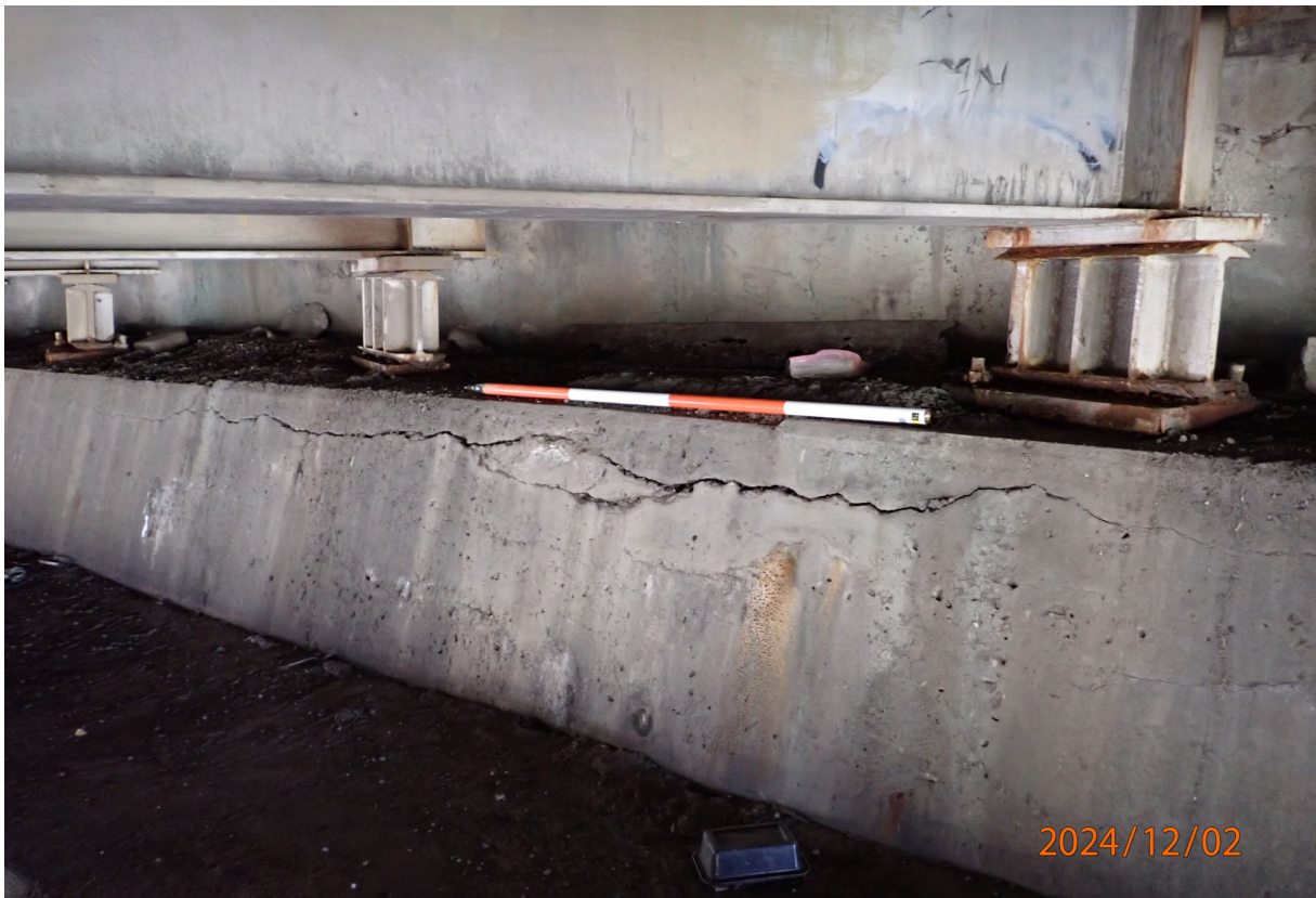
Abutment 1 has intermittent wide horizontal cracking in the NB portion.
