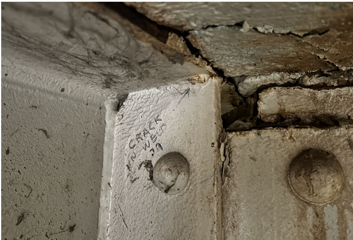
There are a few cracked tack welds at the top of the stiffeners visible near the abutments.
