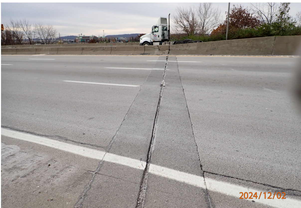
Asphalt plug joint over Abutment 4 (NB)
