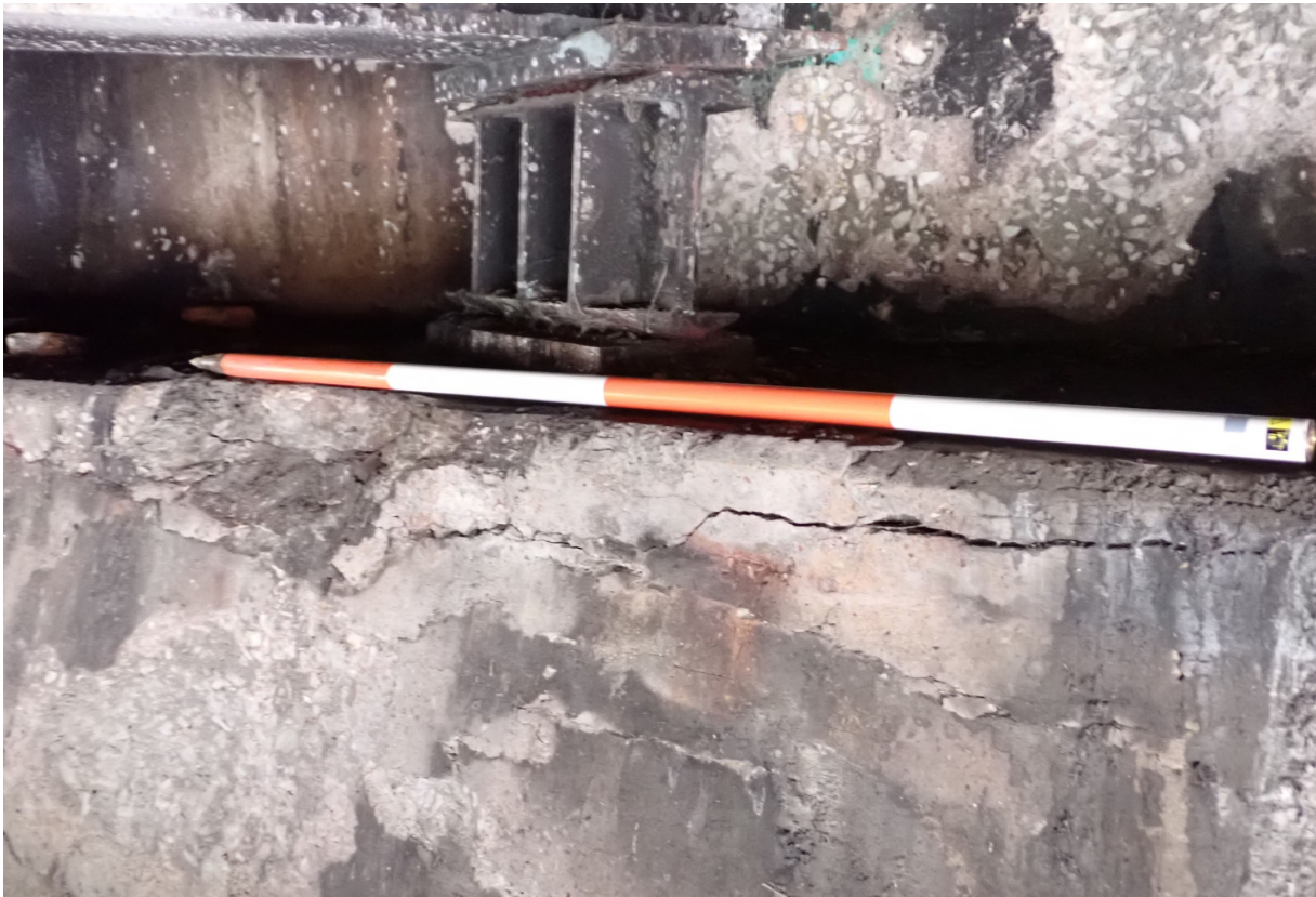
Abutment 4 has wide horizontal cracking plus scaling from fires between Beams 13 and 15 (cap at Beam 14 shown).
