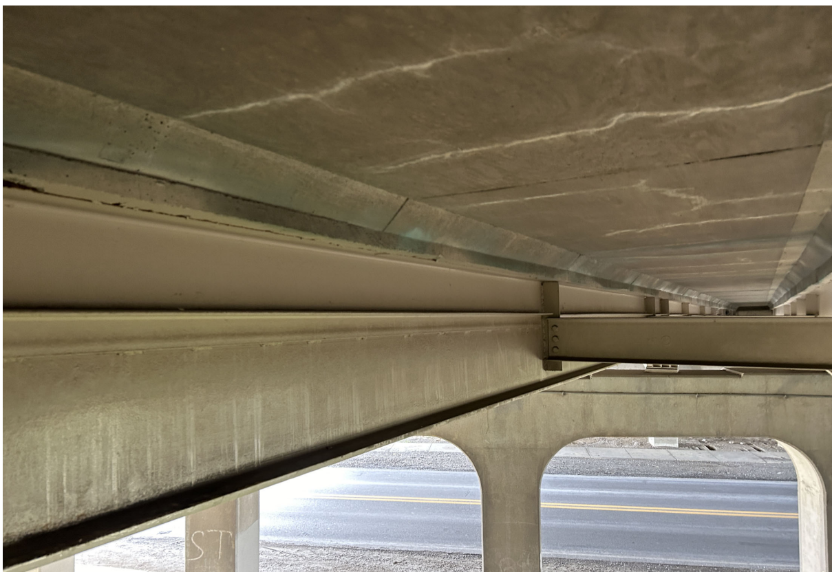
Bridge has potential CIF details (Beam 16 in Span 3 shown).
