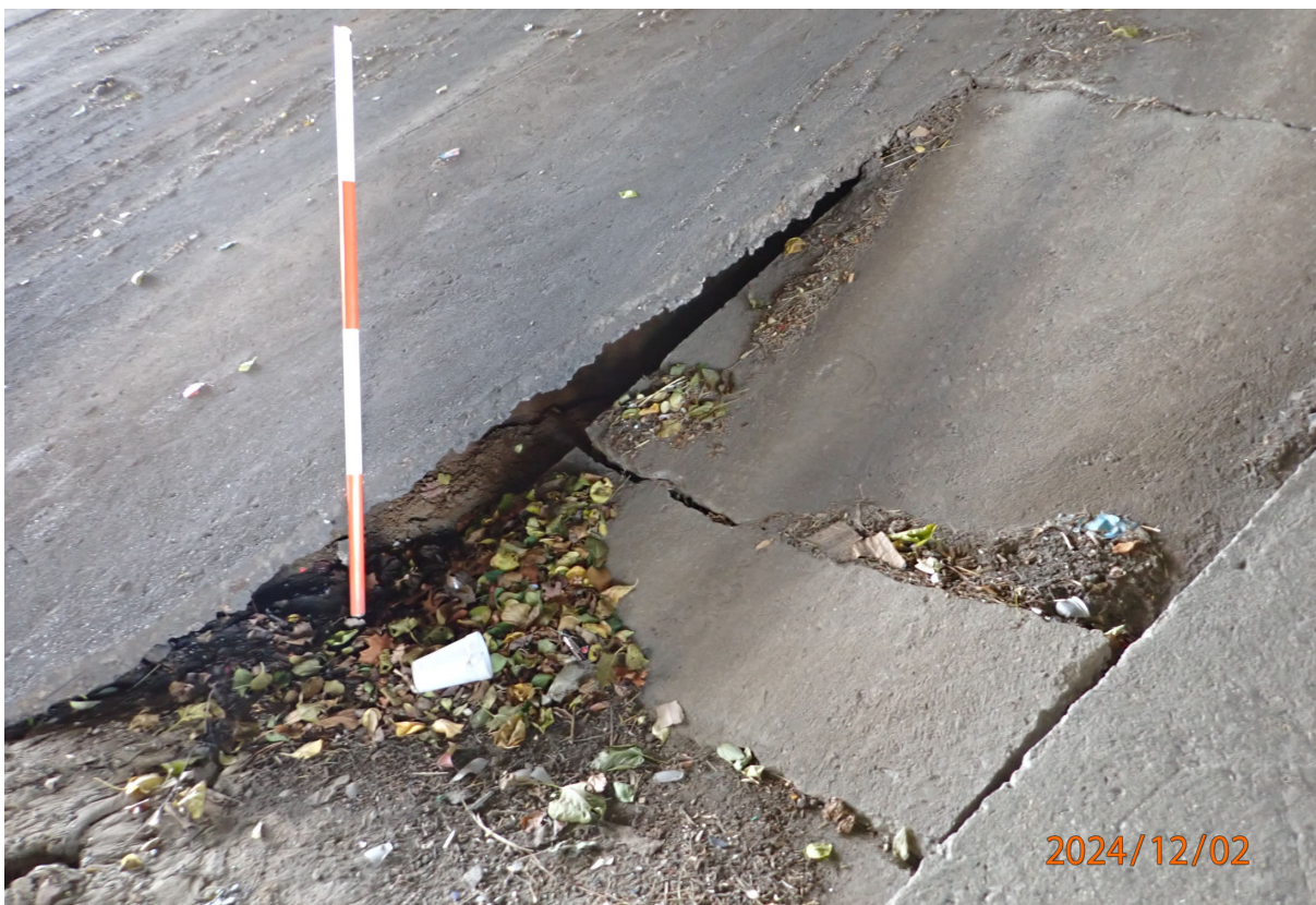
Concrete slope protection has fractured and settled at several locations (Abutment 4 slope shown).
