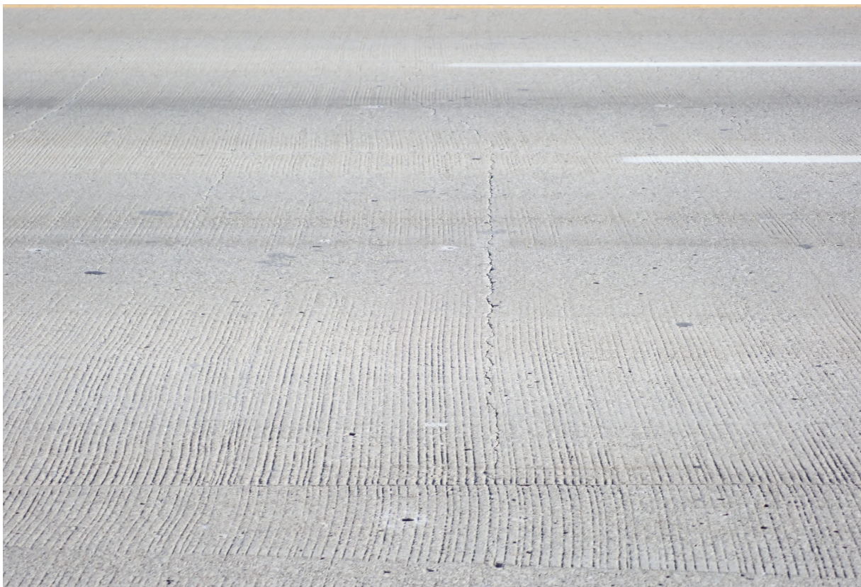
Top of the deck has some wide transverse cracks (SB lanes shown).
