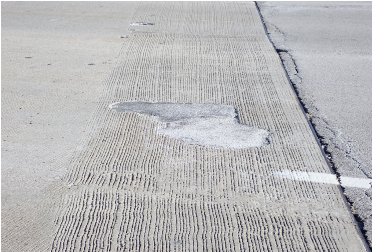
Top of the deck has a 4-foot by 4-foot asphalt patch at the south bridge end in SB Lane 4.
