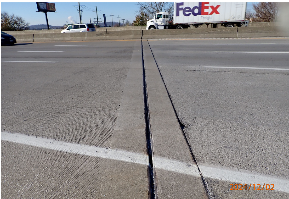
Compression joint seal over Abutment 4 (NB)
