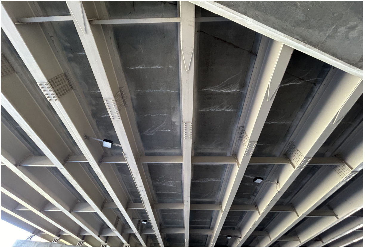
Span 2 soffit Soffit has transverse cracking spaced at less than 3 feet nearly throughout.
