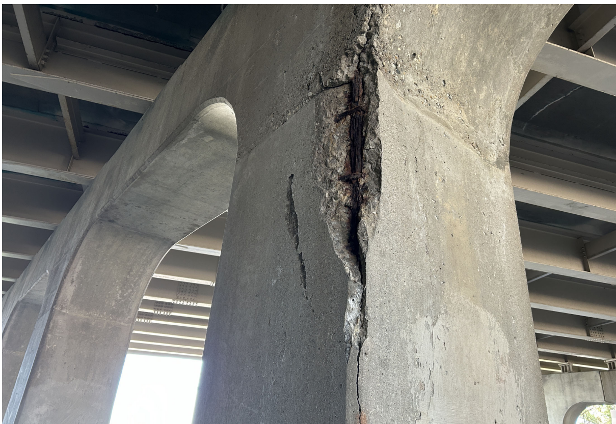
Pier 2-Column 6 has 3' T x 1' W x 3" D spalling with exposed rebar in the south face at the top.
