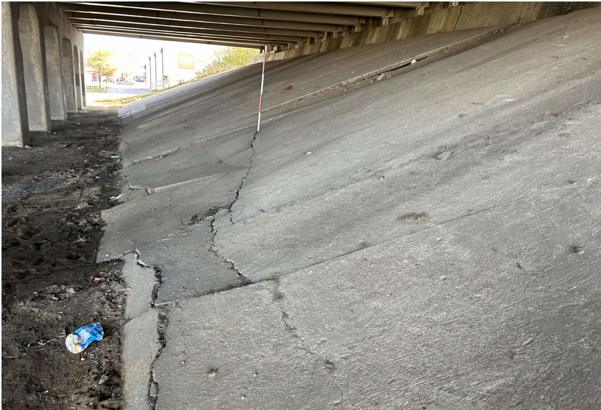
Concrete slope protection has fractured and settled at several locations (looking east along Abutment 1 slope shown).
