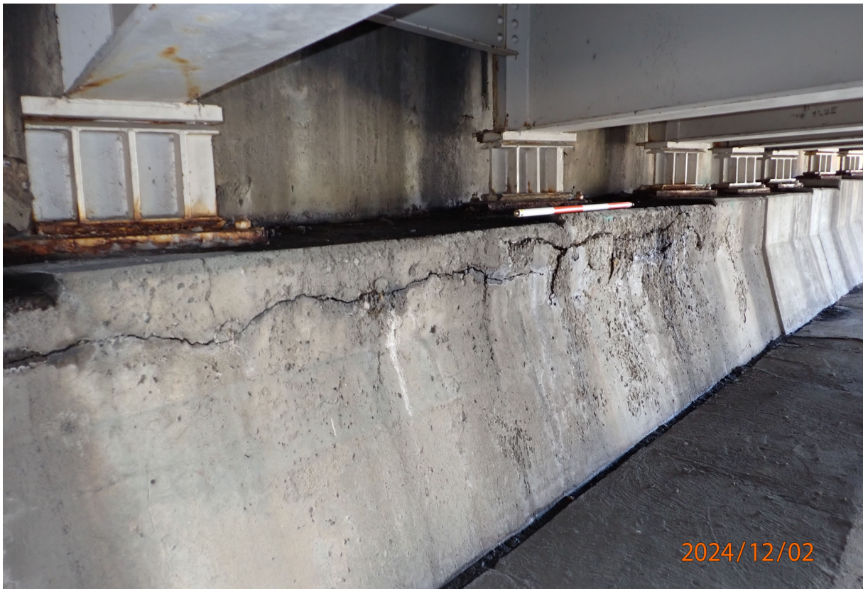
Abutment 1 has 1/4-inch-wide horizontal cracking below Bays 7-11, with some delaminations and scaling.
