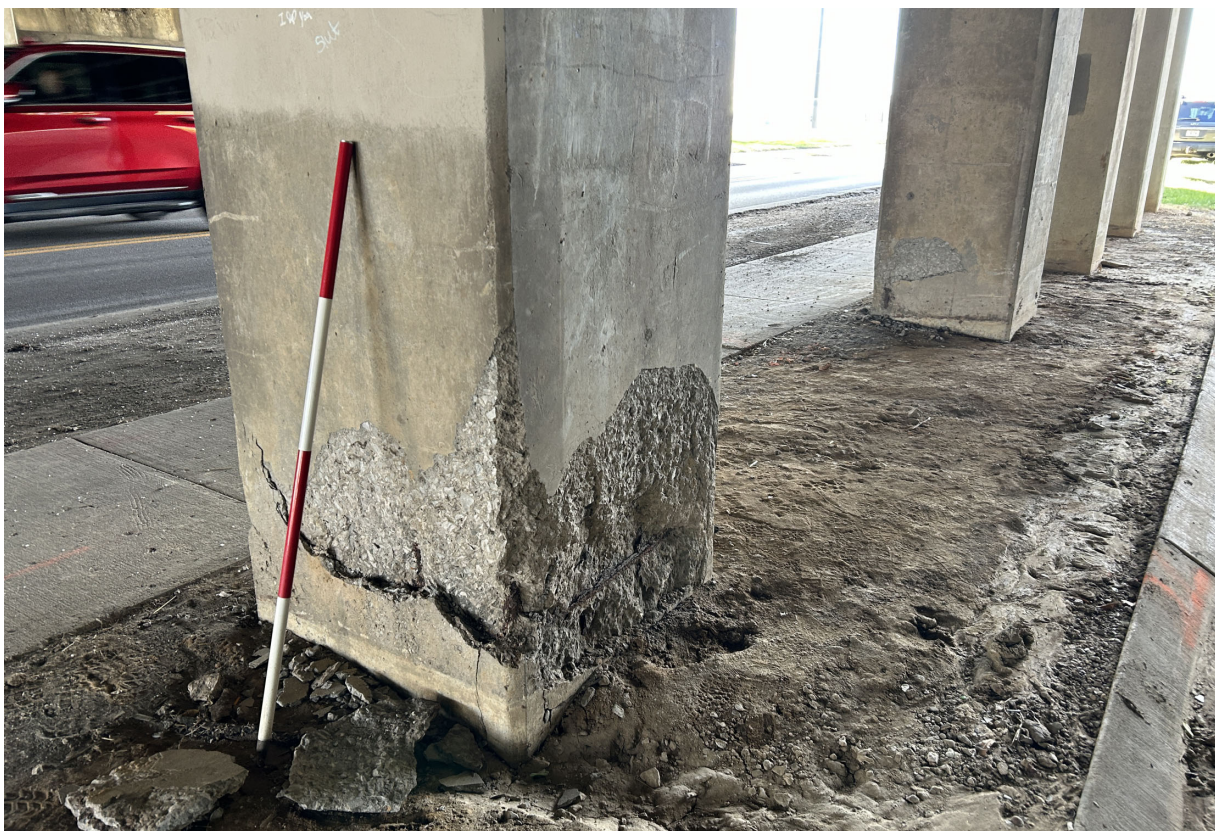
Pier 3-Column 5 has spalling with exposed rebar at the base, roughly 2 feet high.
