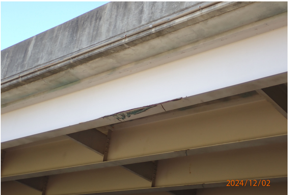
Minor impact damage in Span 2-Beam 1
