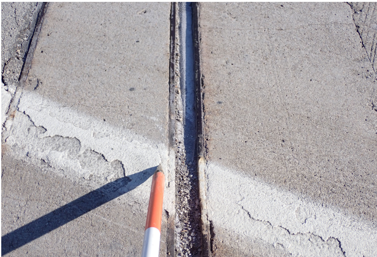
Close up of debris at right SB edge line
