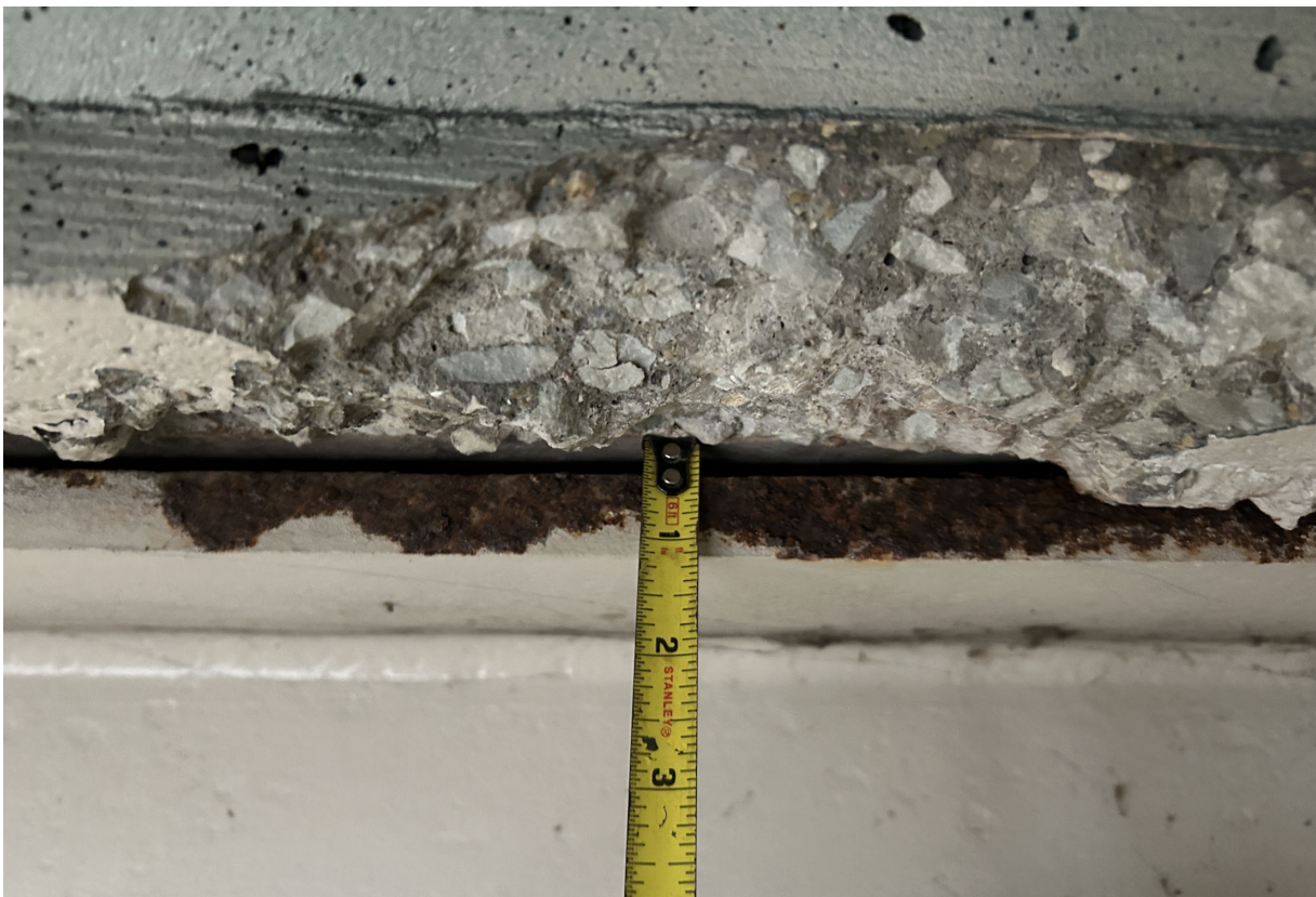
The deck moves independently from the beams at several locations, with gaps up to 3/8" between the deck and top flanges (Beam 16 at Abutment 4 shown).
