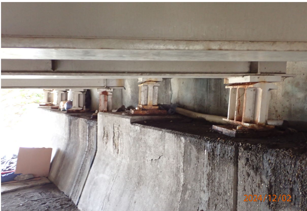
Abutment bearings are expanded at 20° F (tolerable alignment, inconsistent with temperature; Beams 1-6 at Abutment 4 shown).
