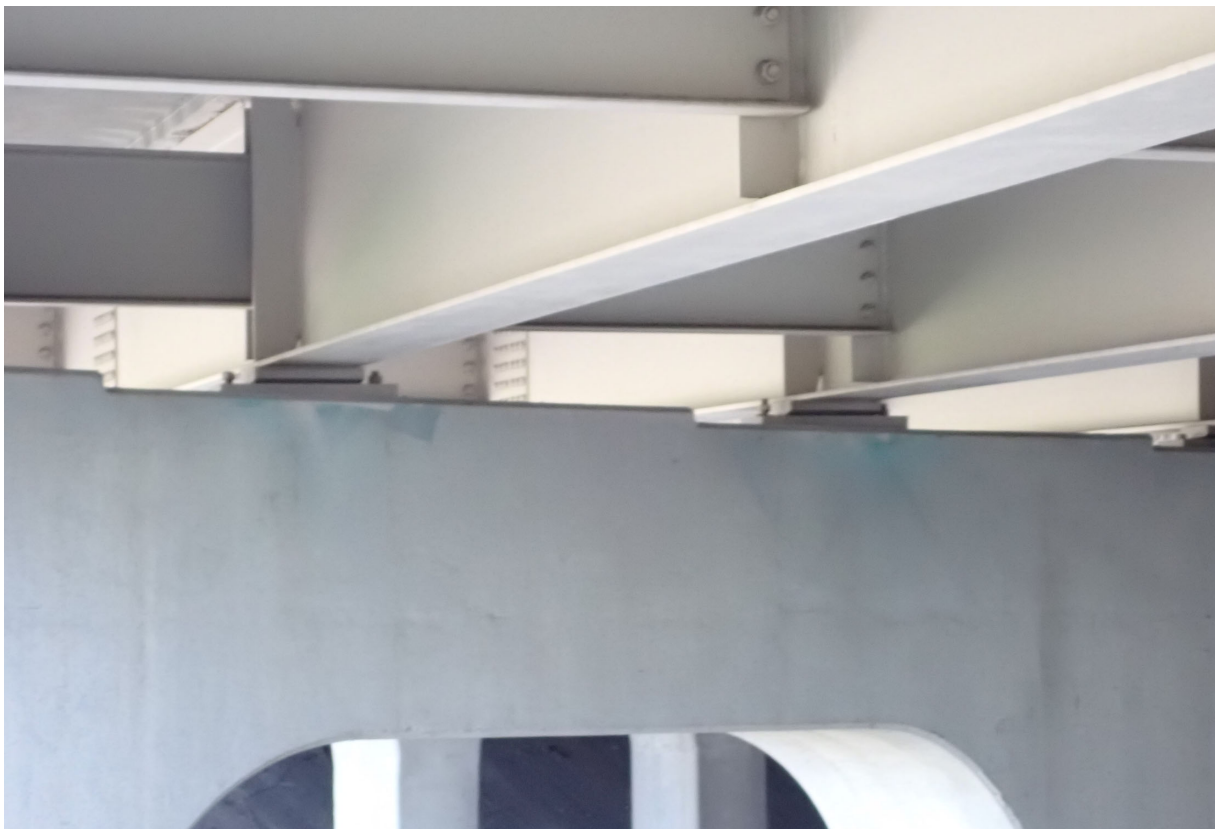
Typical fixed bearings at Pier 2
