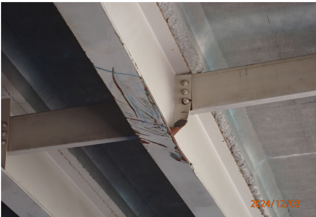
Close up - note haunch spalling and distorted stiffener
