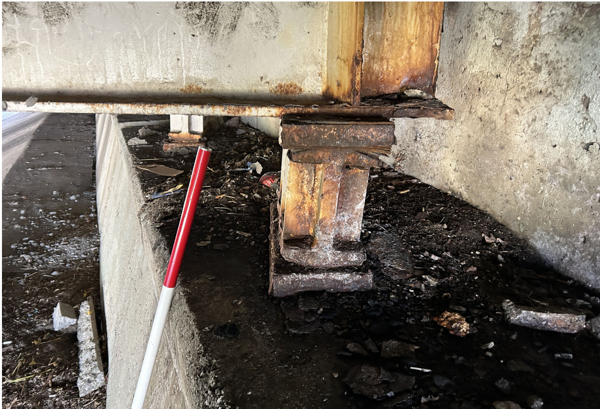
Abutment bearings are expanded at 20° F (tolerable alignment, inconsistent with temperature; Beam 12 at Abutment 1 shown). Note debris on abutment seat.
