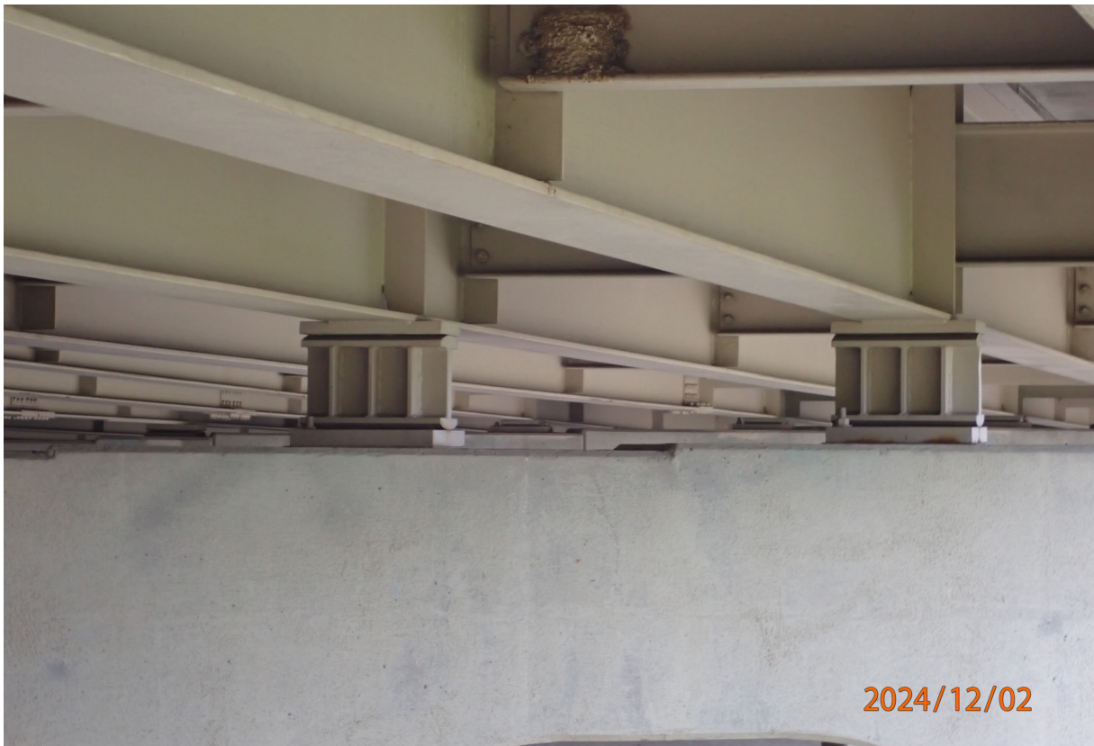
Typical rocker bearings at Pier 3
