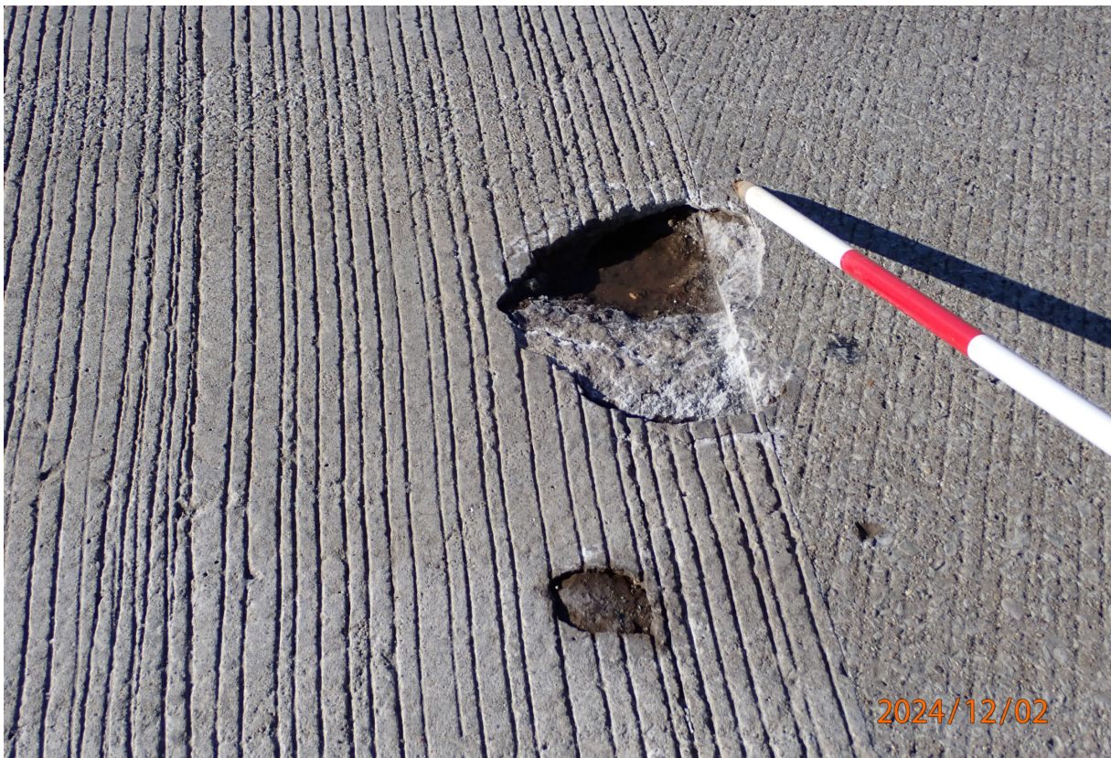
Top of the deck has a 2-foot-diameter by 2-inch-deep spall near the south bridge end in the right NB lane.
