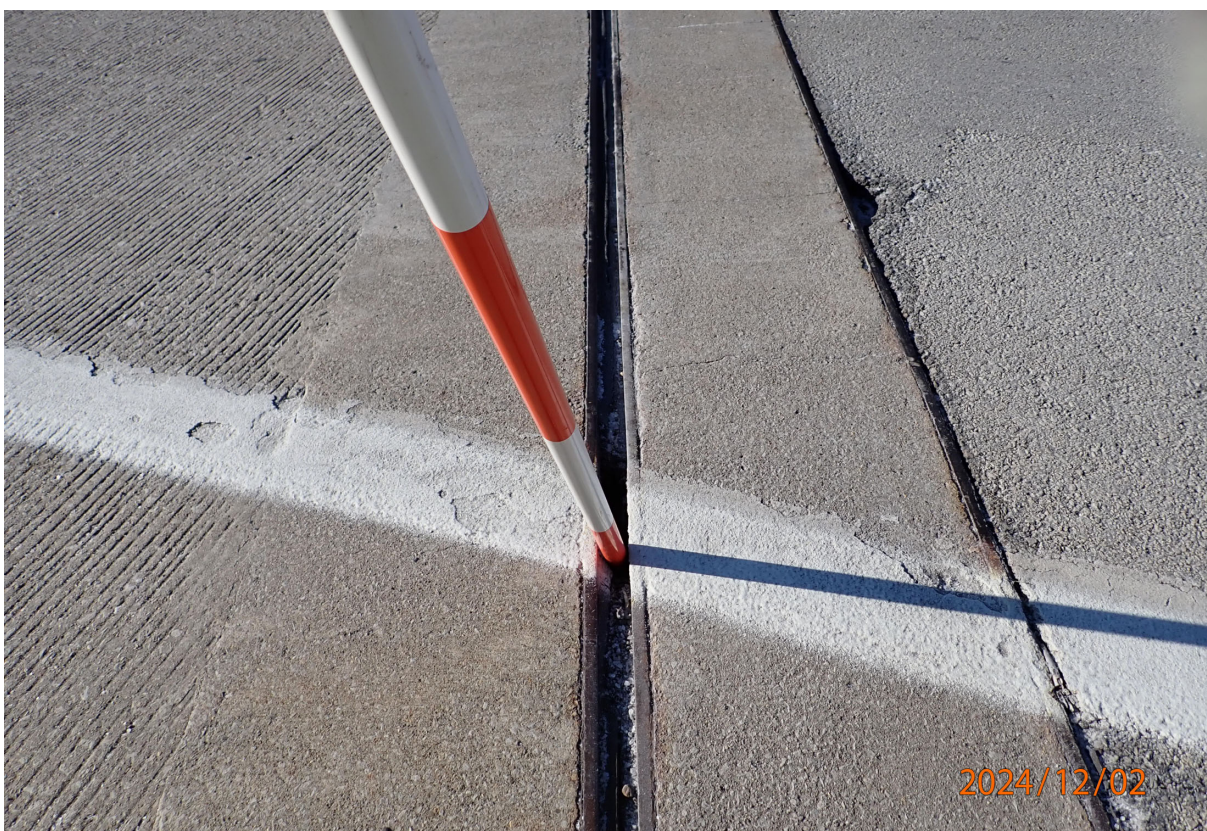
Compression joint seal over Abutment 4 has total loss of adhesion in intermittent areas (right NB edge line shown).
