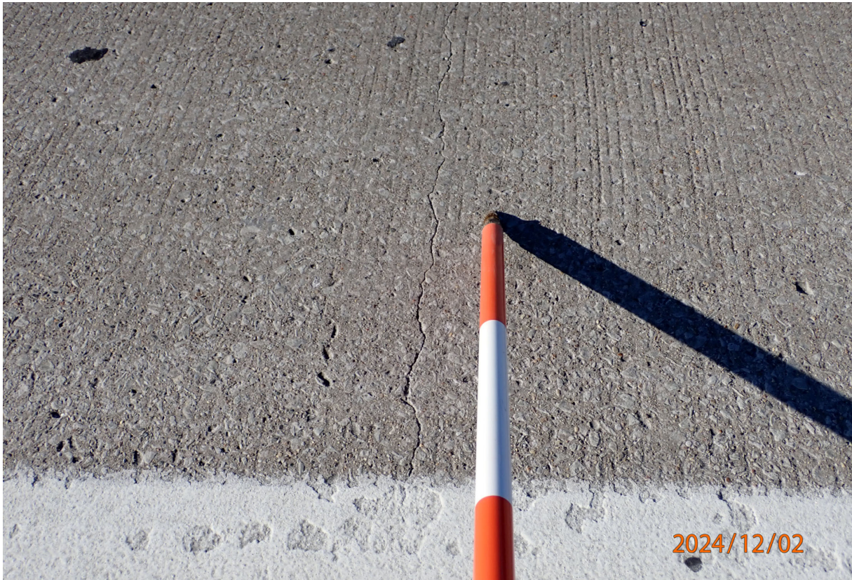
Top of the deck has wearing with exposed coarse aggregate, plus intermittent transverse cracking (NB right lane shown).
