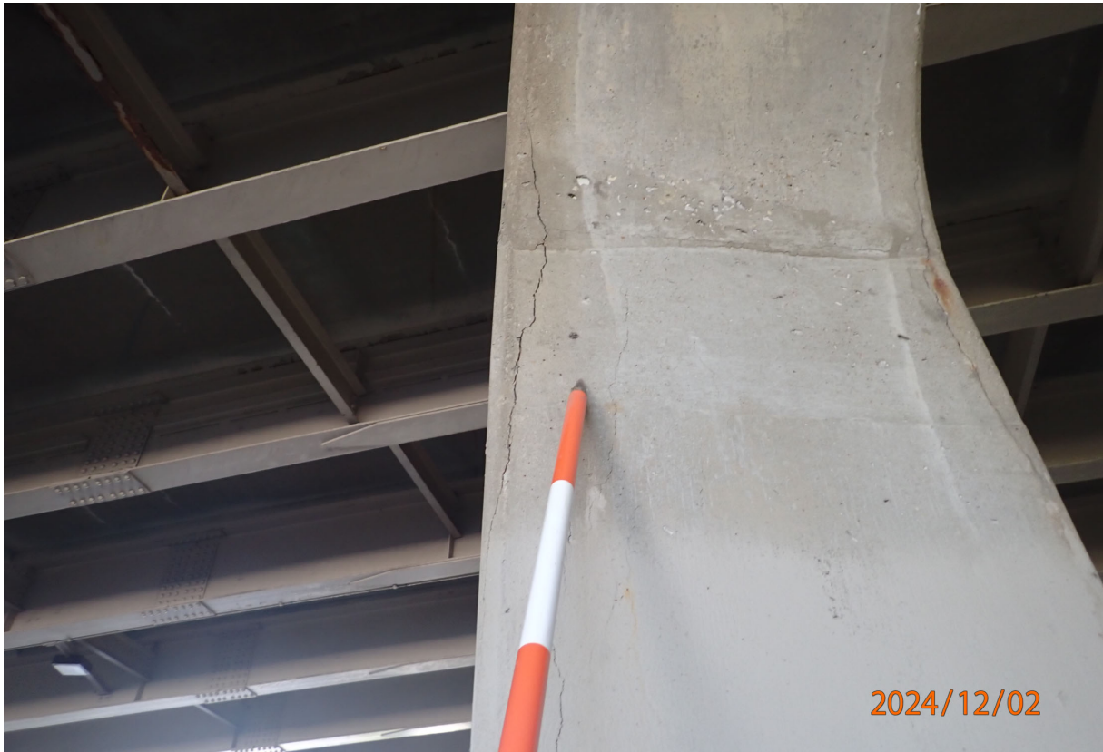
Pier 3-Column 6 has wide vertical cracks in the east face at the top.
