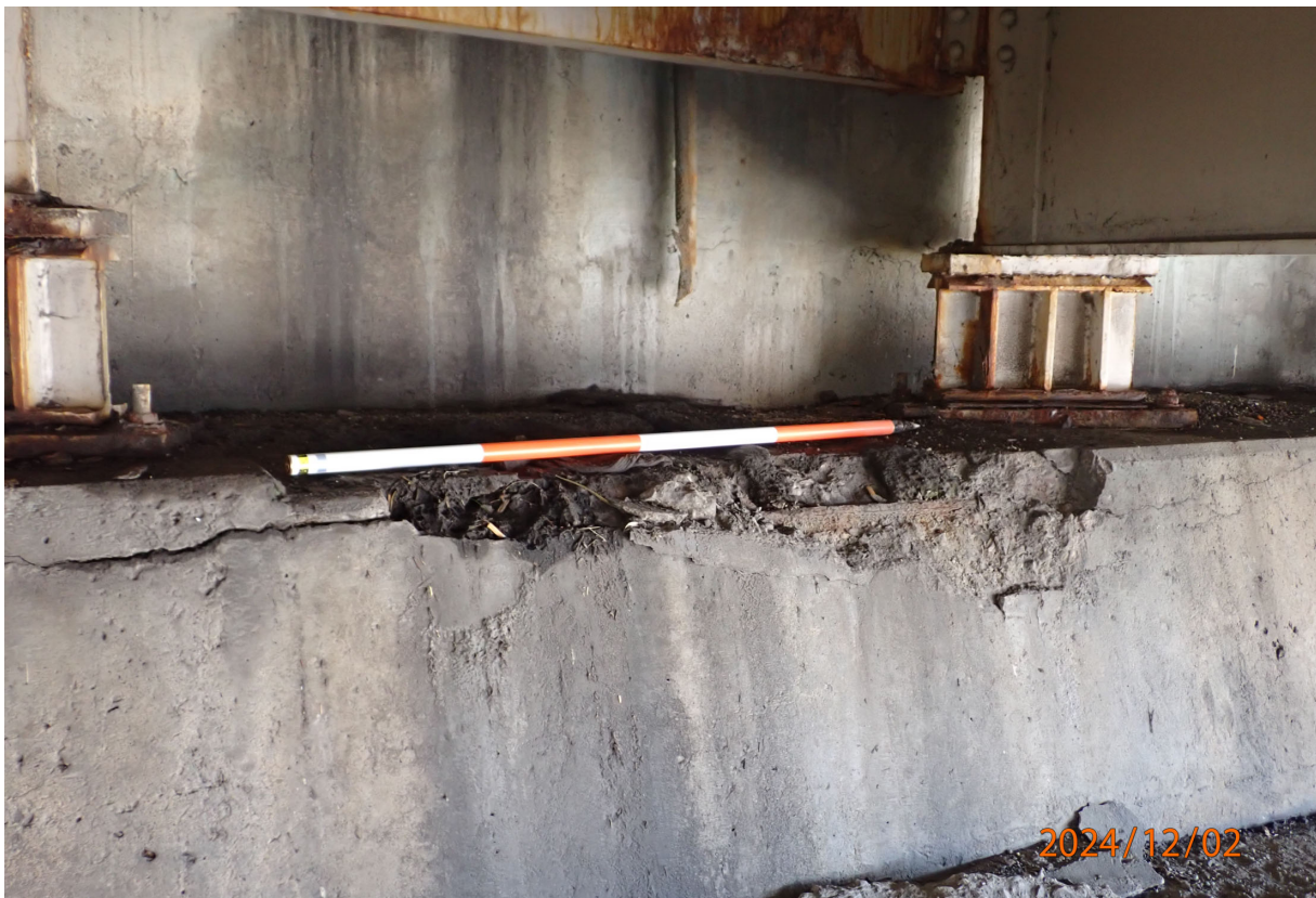
Abutment 4 cap has spalling with exposed rebar below Bay 19, 5' L x 1' T x 3" D.
