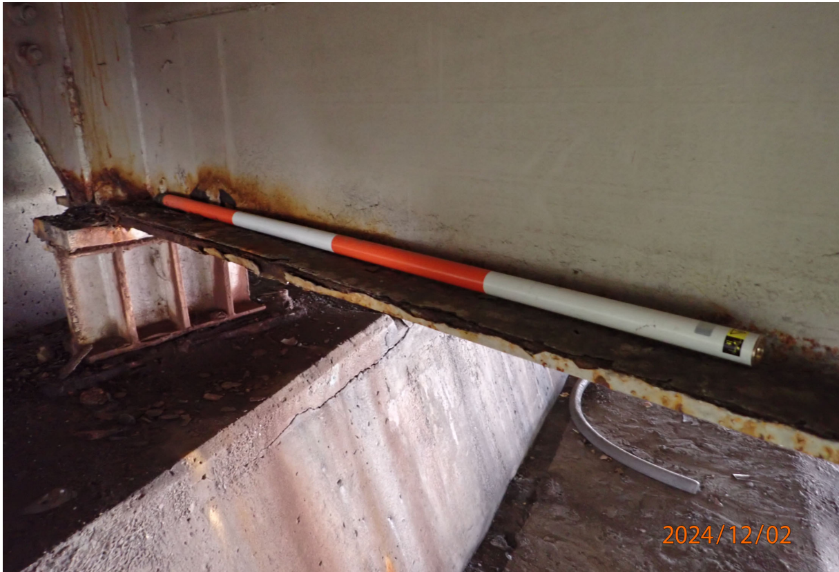
Girders have surface rust scattered throughout, with heavier rust near the beam ends and longitudinal joint (Beam 16 at Abutment 4 shown).
