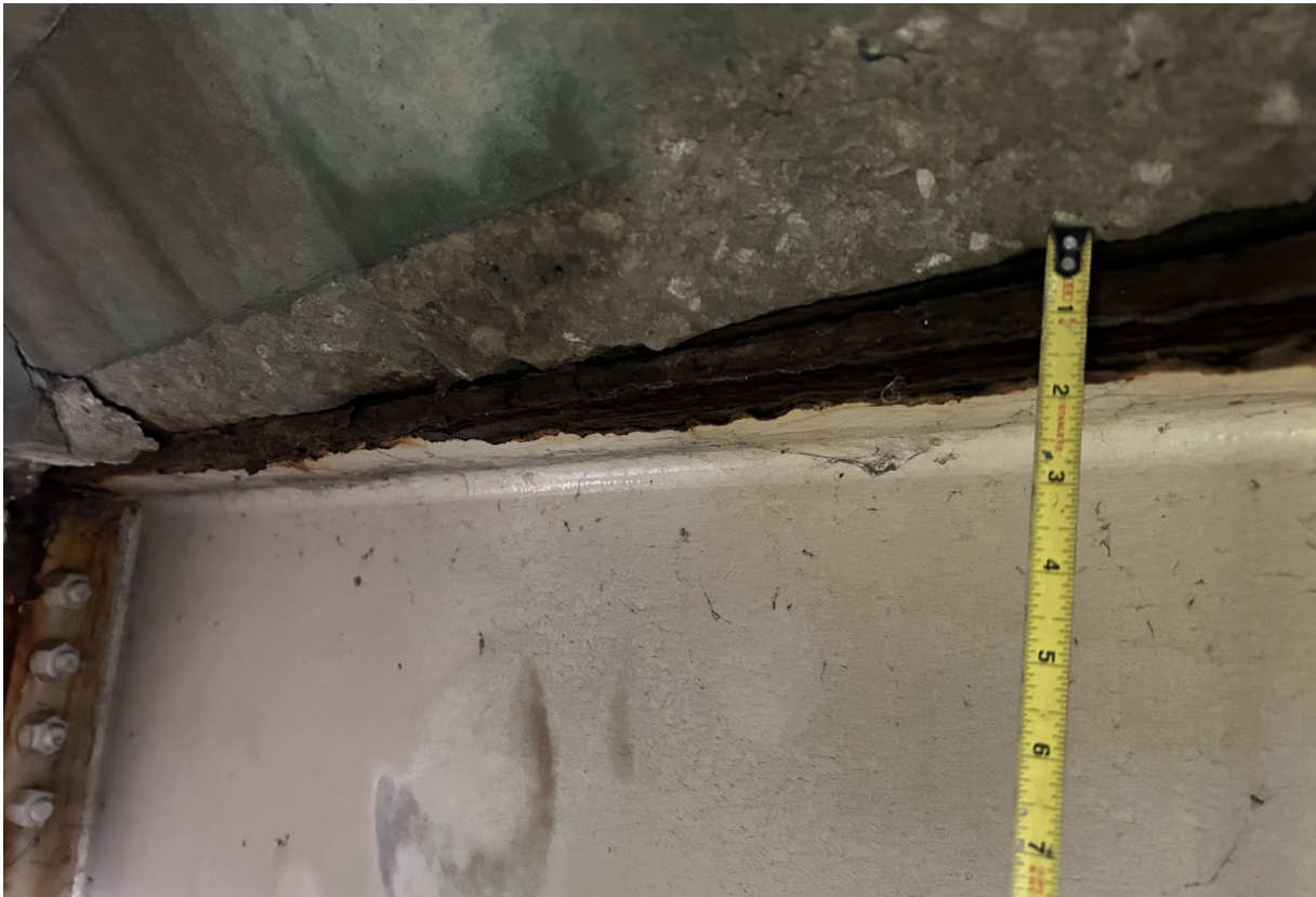
Beam 13 has flaking corrosion on the flanges in Spans 2 and 3 near Pier 3 and Abutment 4 (top flange at Abutment 4 shown).
