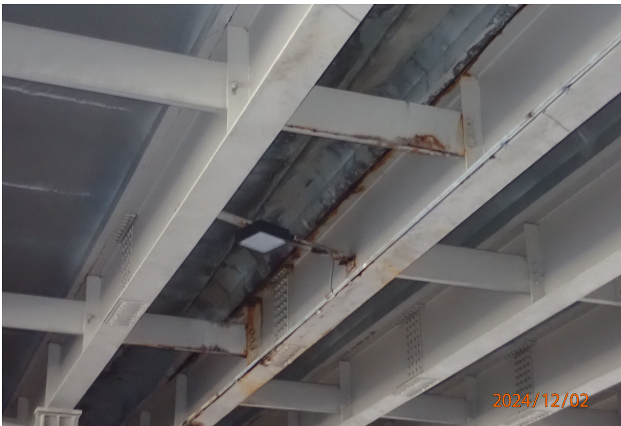
Beam 13 has flaking corrosion on the flanges in Spans 2 and 3 near Pier 3.
