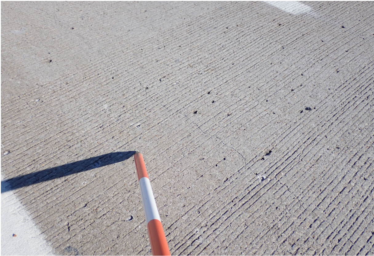
Top of the deck has moderate longitudinal cracking in the flared portion of the SB right lane.
