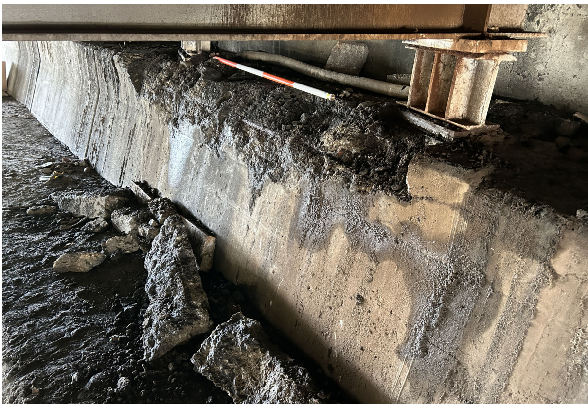
Abutment 4 cap has spalling with exposed rebar below Bay 7, 10' L x 1' T x 6" D; spalling extends to the front edges of the masonry plates for Beams 7 and 8.
