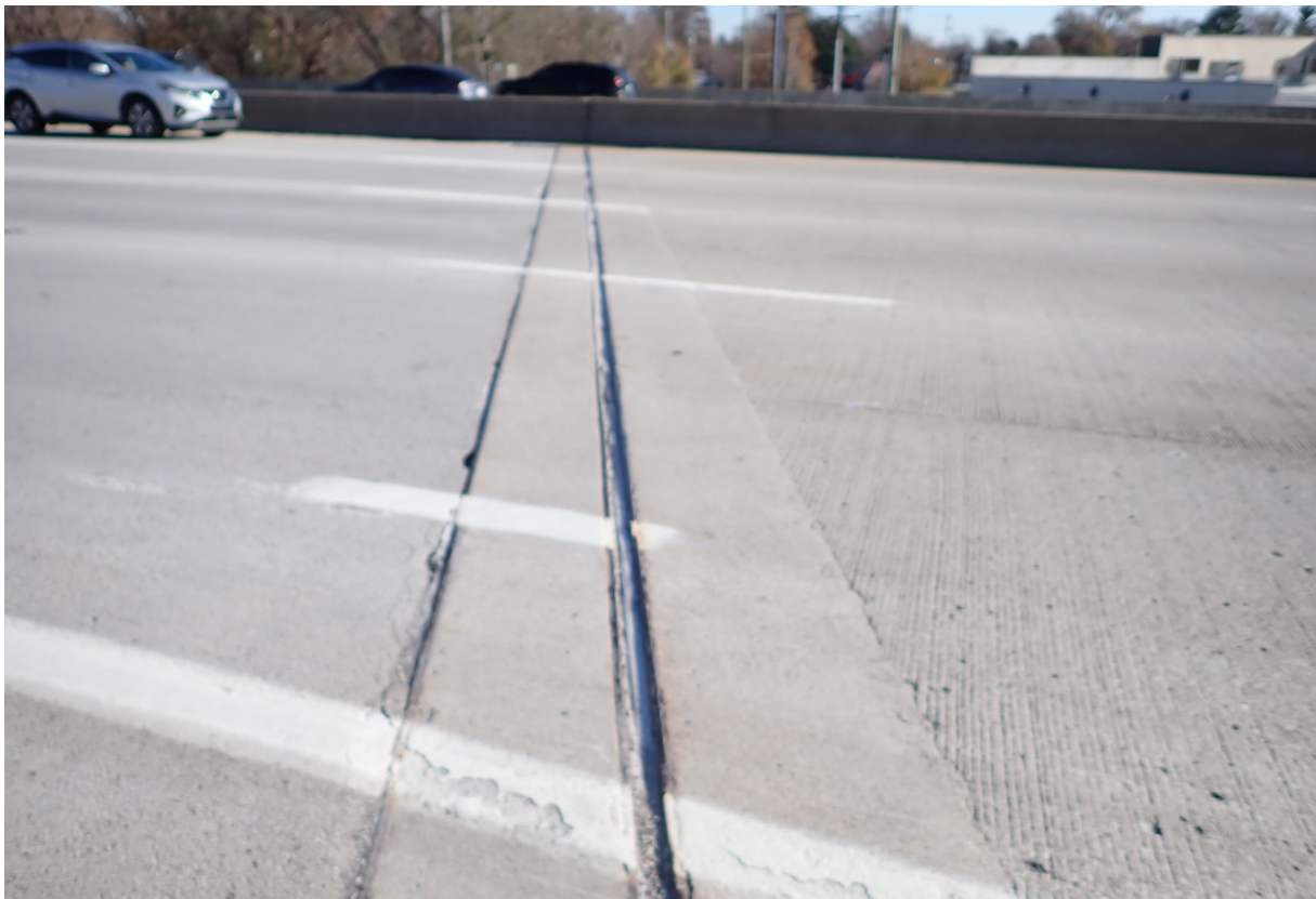
Compression joint seal over Abutment 4 (SB)
