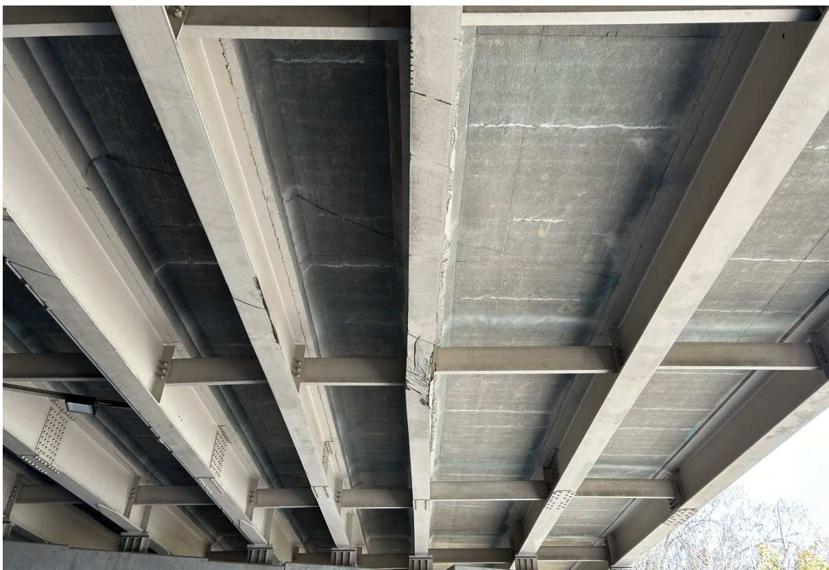
Span 2-Beam 22 has impact damage initially noted during 09/11/18 inspection; out-of-plane distortion is worst at the midspan diaphragm, but appears to affect the full length between field splices (33 feet CS4).
