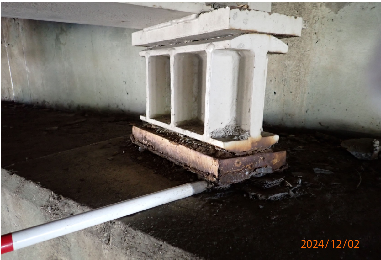
Several abutment bearings have gaps between the rocker and plates and/or masonry plate and abutment seat due to pack rust (Beam 15 at Abutment 1 shown).
