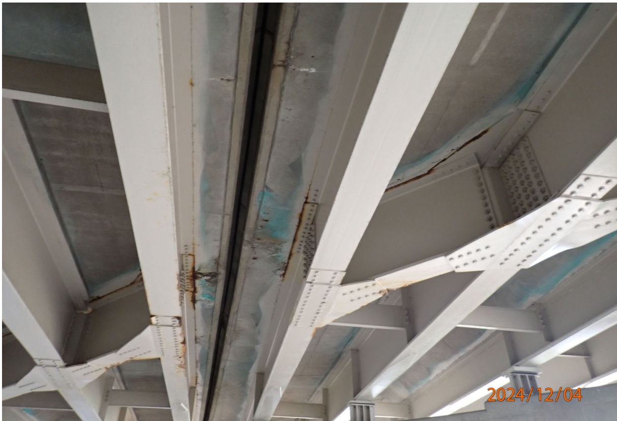
Beams and diaphragms have flaking corrosion scattered throughout the top flanges, especially near the longitudinal joints (Span 4 shown).
