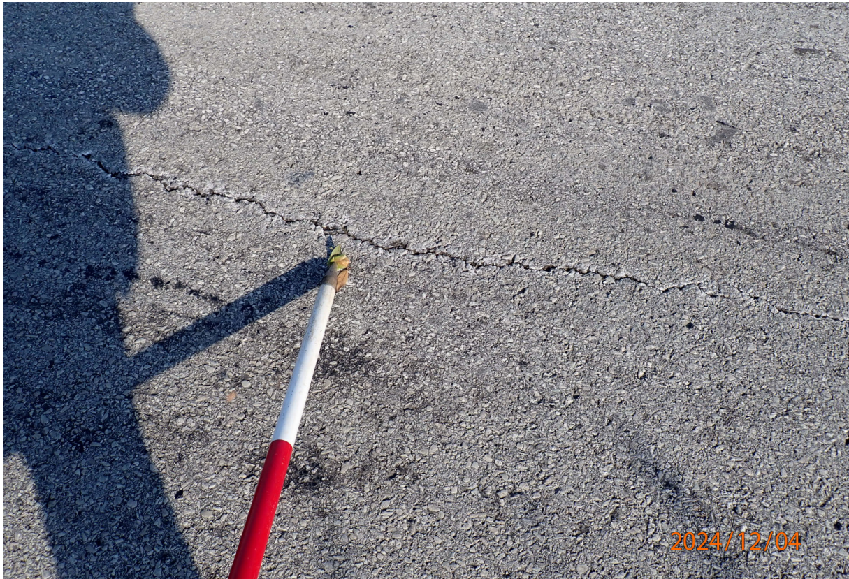
Overlay has minor wearing throughout, and intermittent longitudinal cracking in the right SB lane in Spans 1 and 2.
