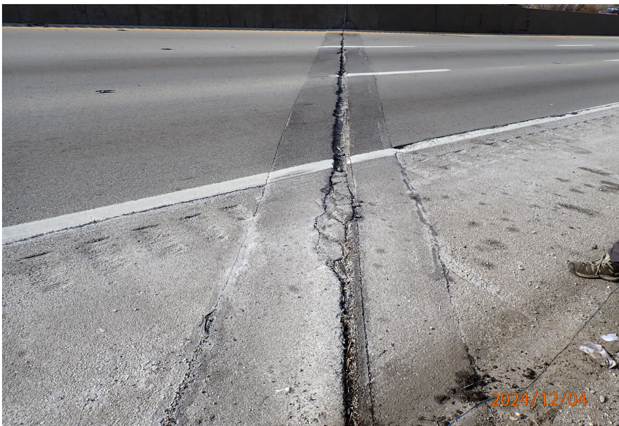
Asphalt plug joint over Abutment 5 (NB)
