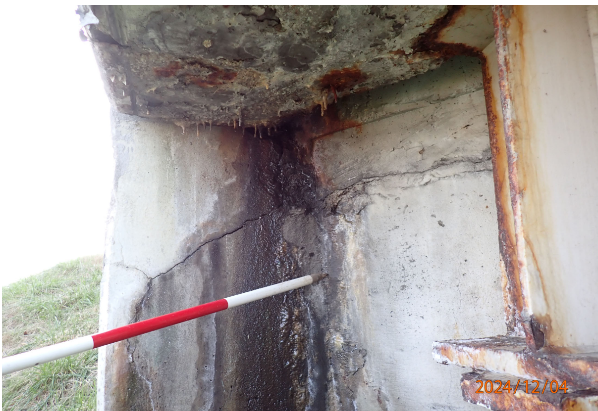
Abutment 1 backwall has 1/4" wide diagonal cracking at both ends (east end shown).
