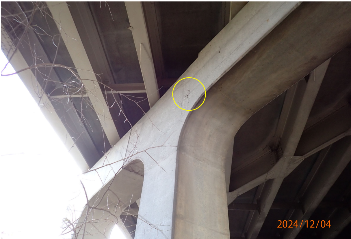
Pier caps have scattered moderate cracks, delaminations, and small spalls (north face of Pier 3 shown).
