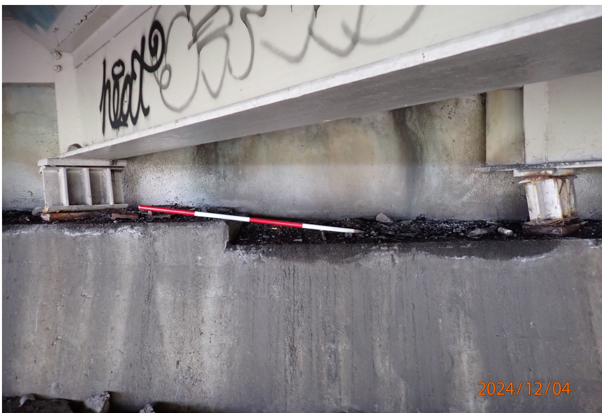
Abutment bearings are expanded at 40° F (tolerable alignment, inconsistent with temperature; typical Abutment 5 NB beams shown). Note debris and moisture on seat.
