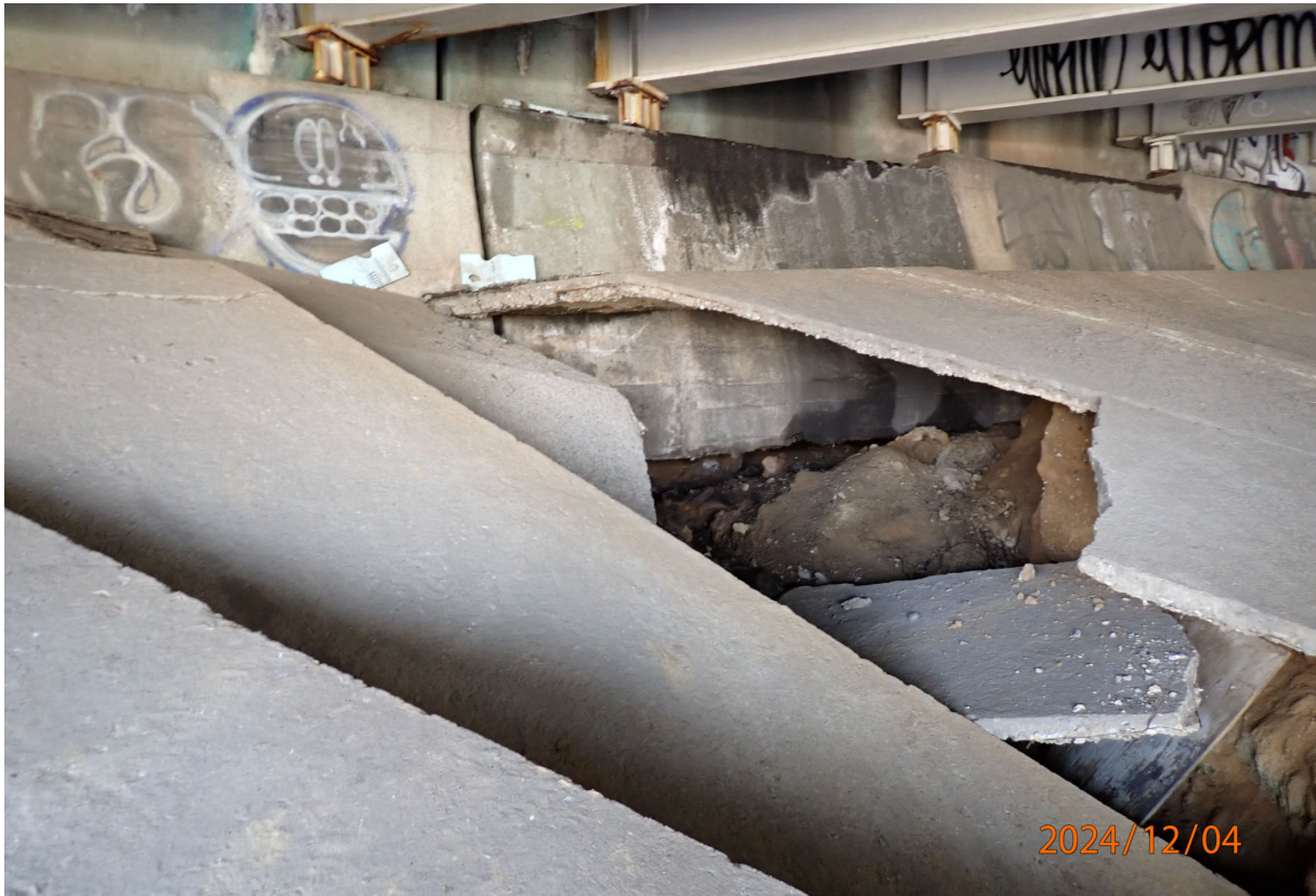
At the failed sections of concrete slope, the Abutment 1 cap is undermined 22' L x 6' D x 1' T with at least three exposed piles.
