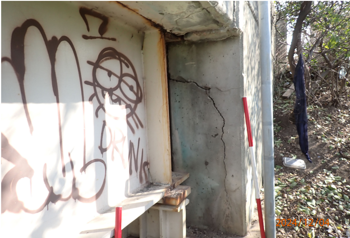
Abutment 1 backwall has 1/4" wide diagonal cracking at both ends (west end shown).
