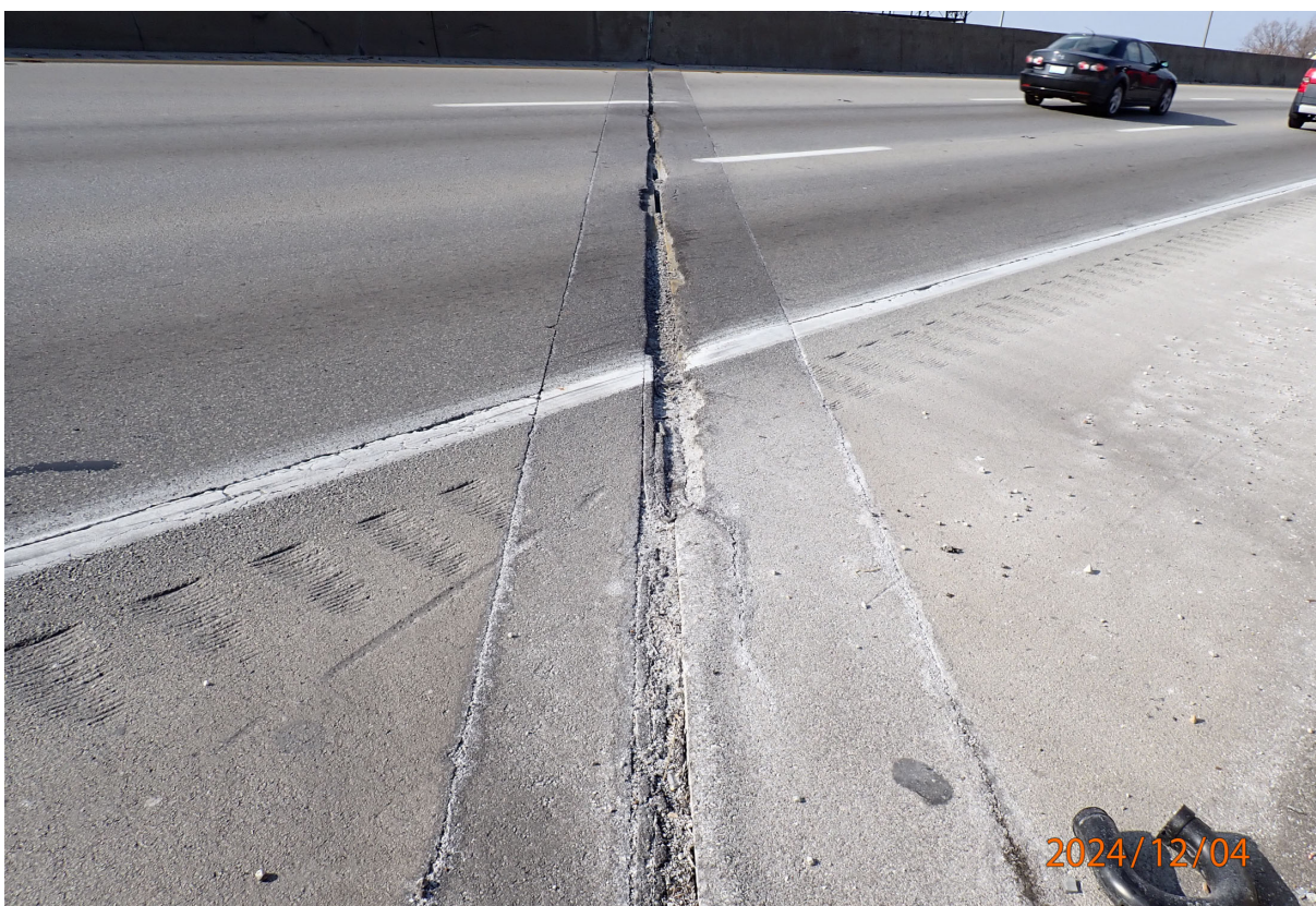
Asphalt plug joint over Abutment 1 (NB)
