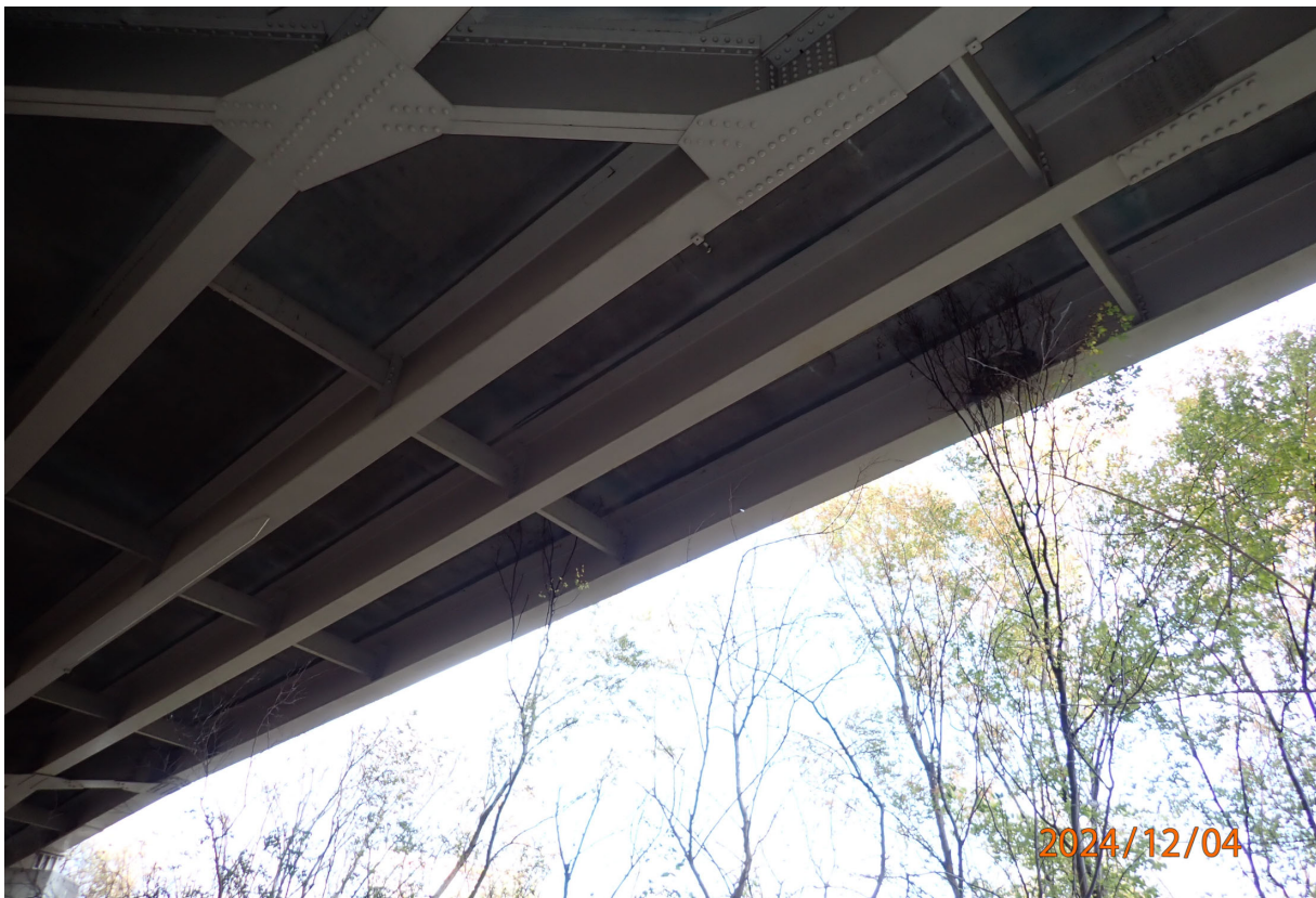
Trees are growing against the superstructure in a few areas (east side of Span 3 shown).
