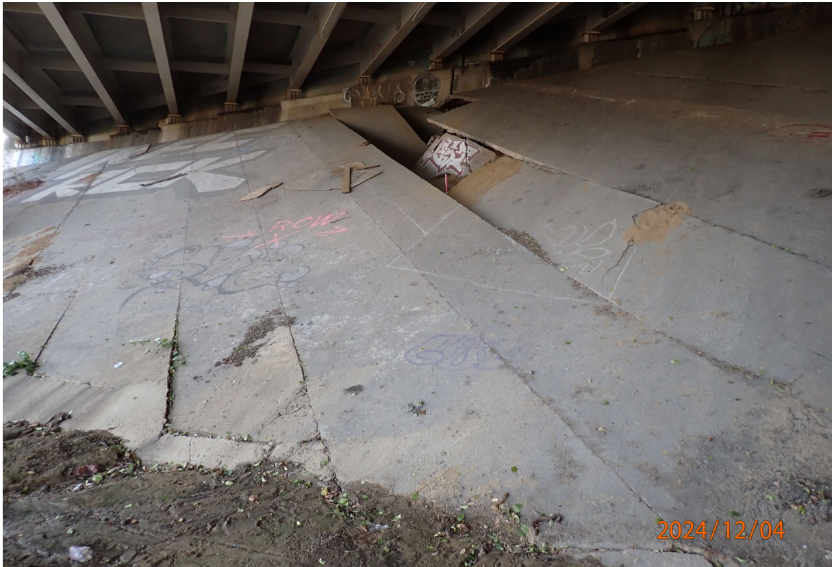
Abutment 1 concrete slope has two fractured panels between Beams 15 and 17; the broken sections have fallen into the 5' deep void in the underlying embankment.
