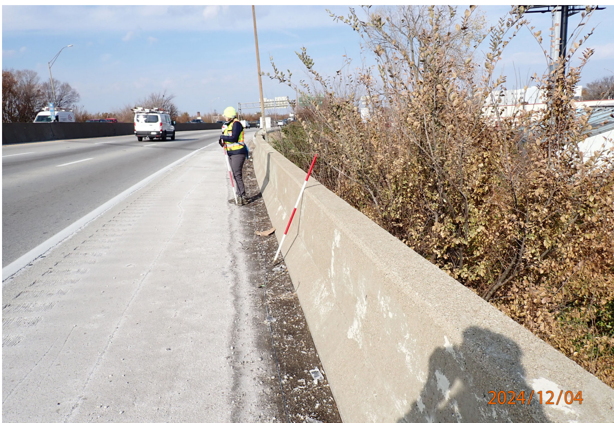
Dirt and debris are piling in the gutter lines. Vegetation is beginning to overhang the bridge railings (east side shown).
