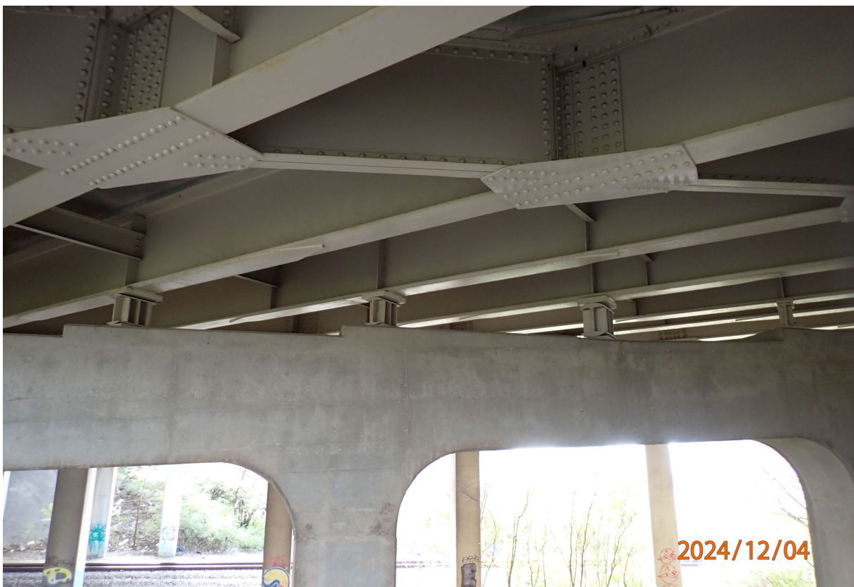
Typical rocker bearings at Pier 4
