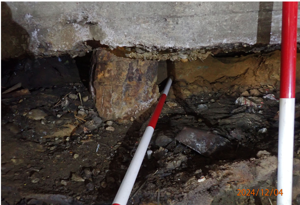
One of the exposed piles has flaking corrosion with section loss.
