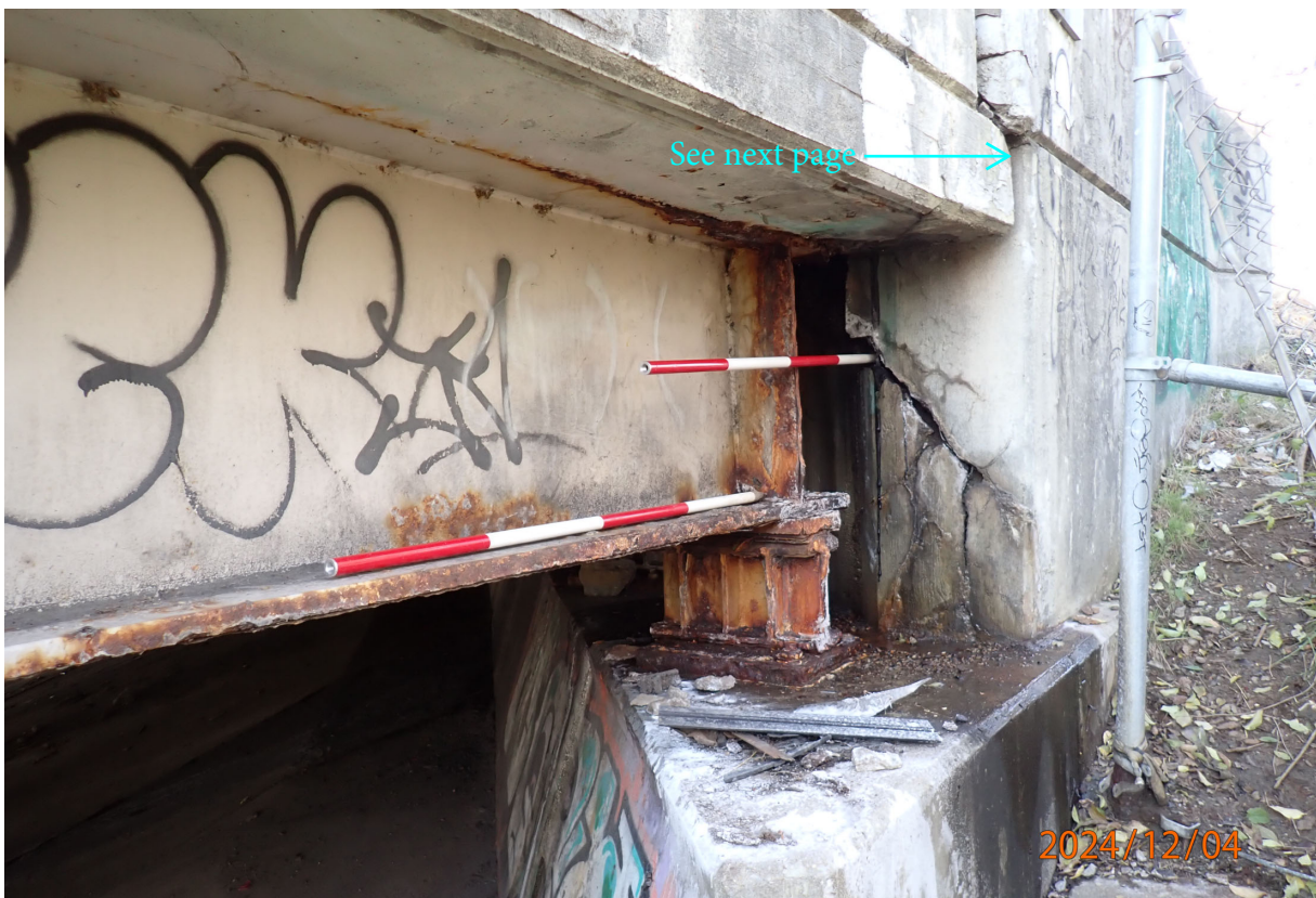
Abutment 5 backwall has a 1" wide diagonal crack/fracture at the east end with map cracking. The northeast wing is tilting out by 1.5" as measured at the top of the deck.
