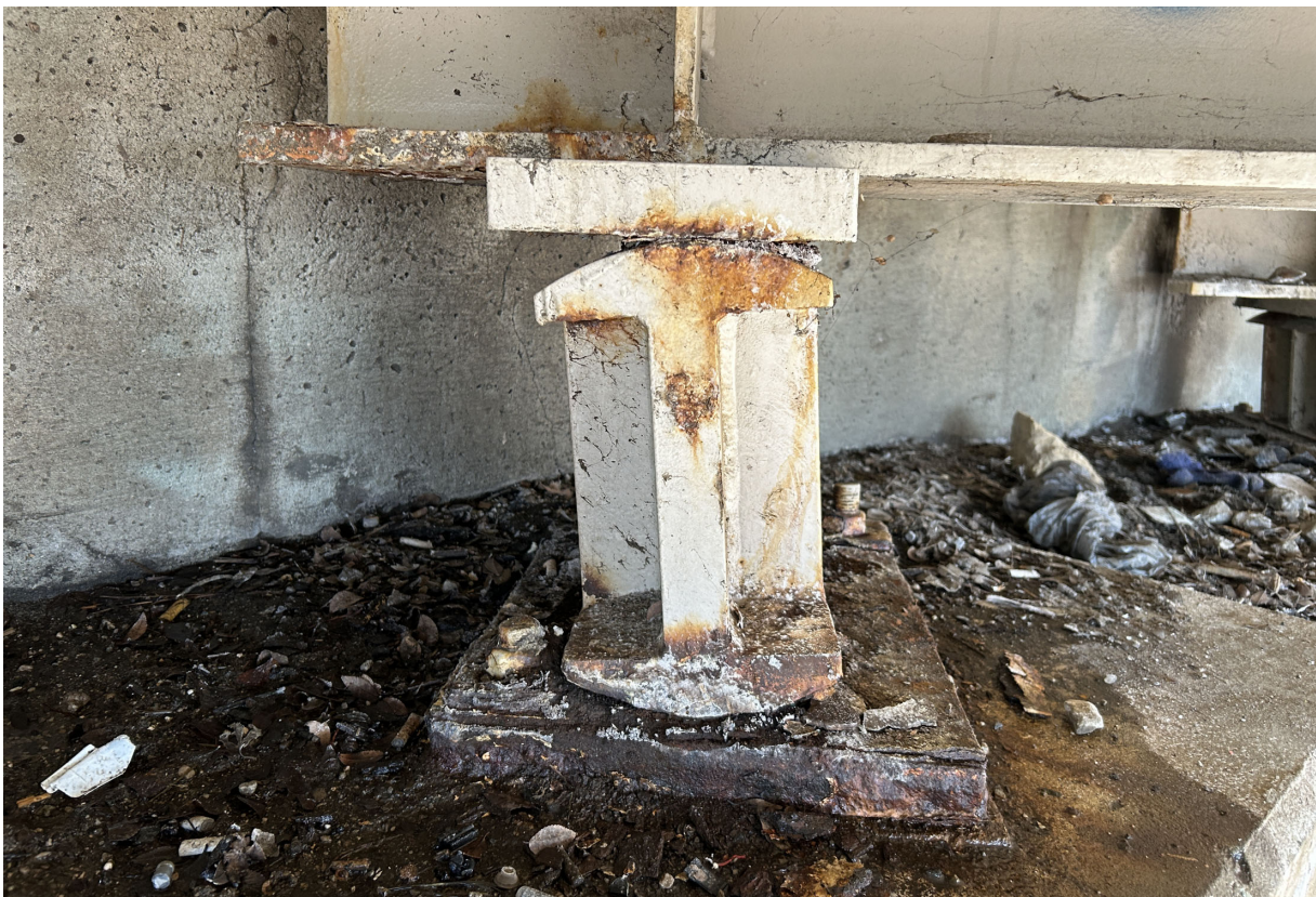
Typical rocker bearing expanded at 40° F (Girder 3 at Abutment 5 shown)
