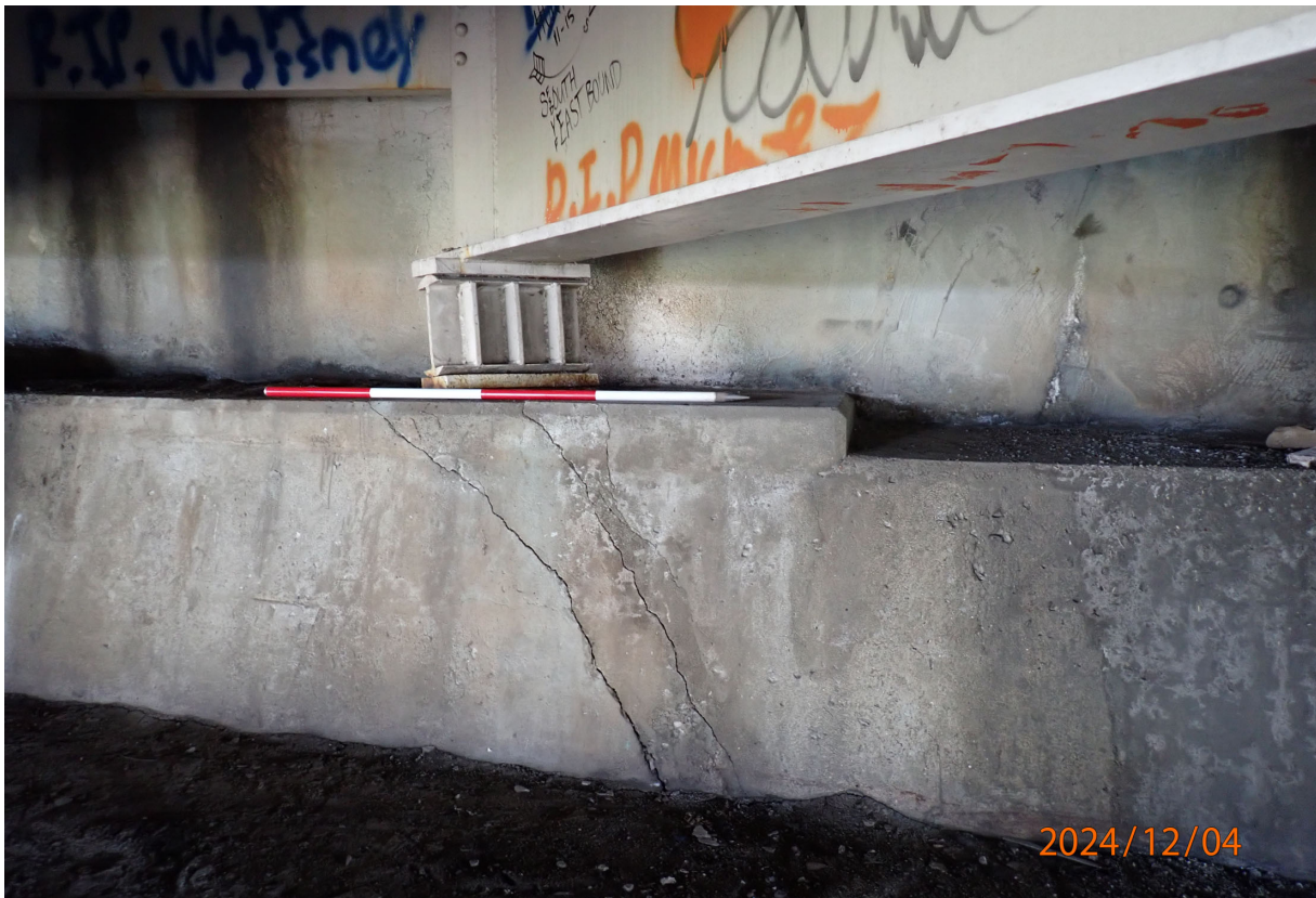
Abutment 5 cap has two wide diagonal cracks below Beam 16.
