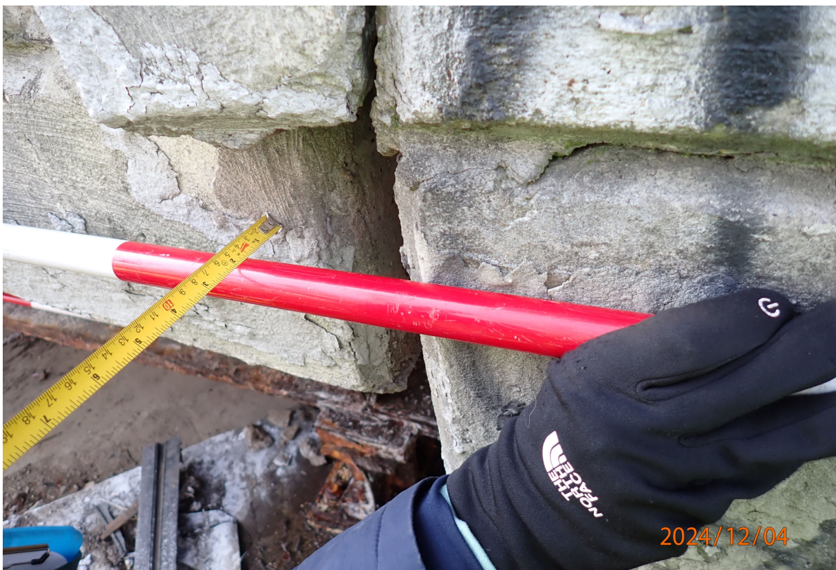
The northeast wing is tilting out by 1.5" as measured at the top of the deck (close up).
