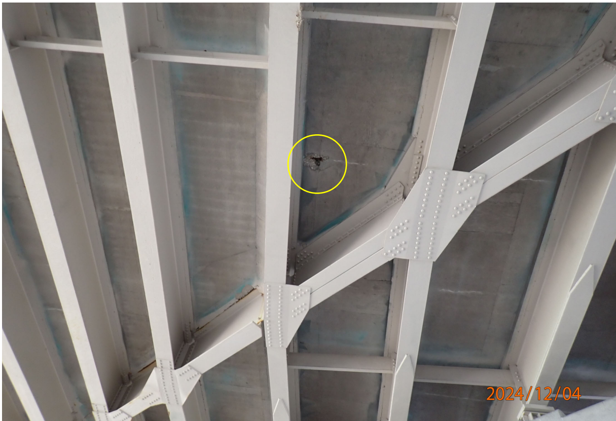
Soffit has a few scattered spalls with exposed rebar (Span 3-Bay 13 shown).
