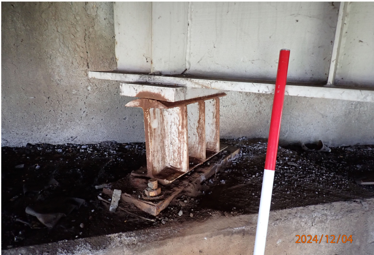
At Abutment 5-Beams 7 and 8, the sole plates are not in contact with the rocker bearings and can be moved by hand, except under live load (Beam 8 shown). Note fretting rust.
