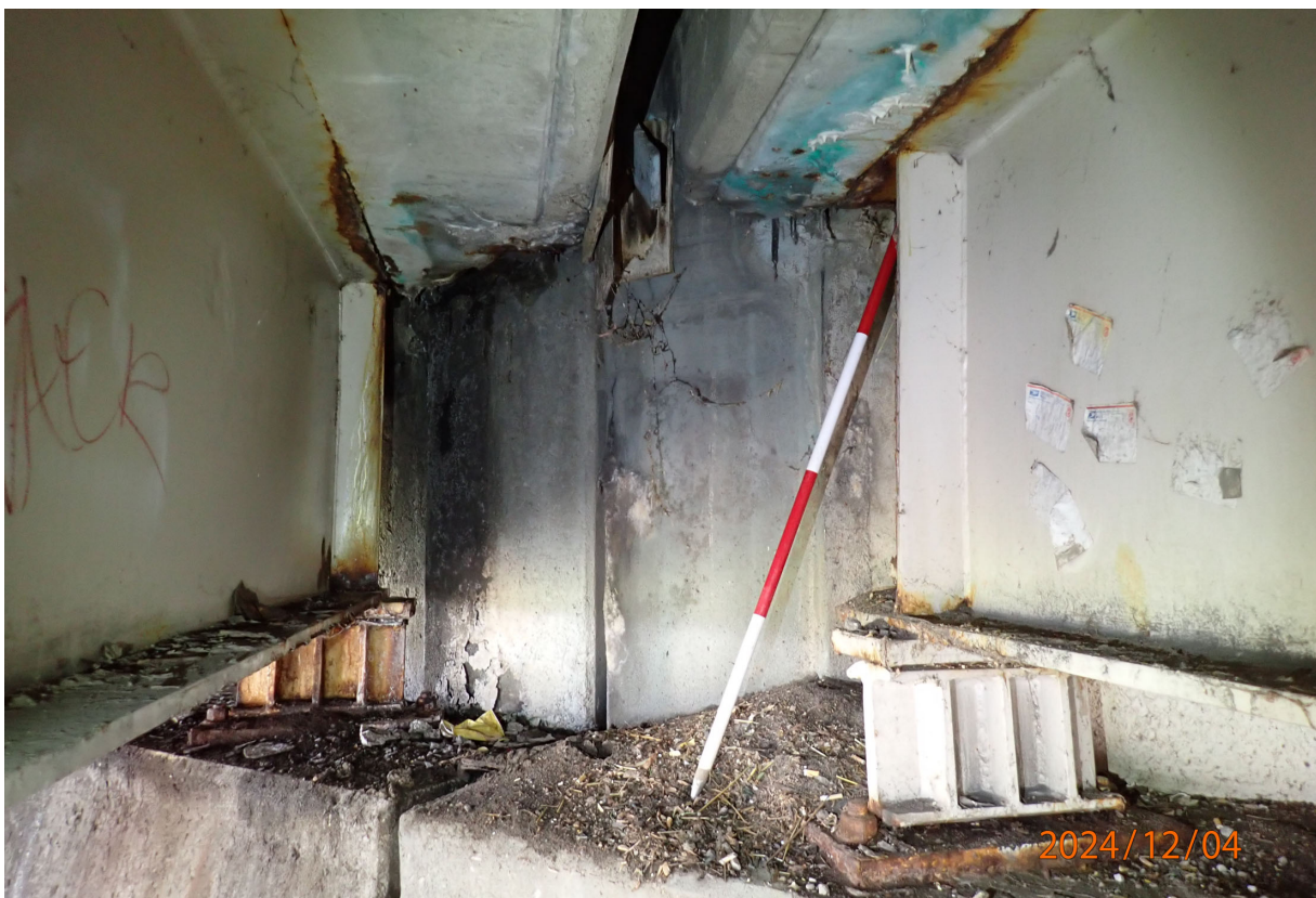
Soffit and backwalls have spalls at the longitudinal joint (Abutment 5 shown, see next photo).
