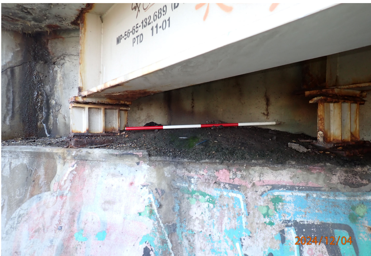
There is up to 1 foot of debris piled on the abutment seats (east end of Abutment 1 shown).
