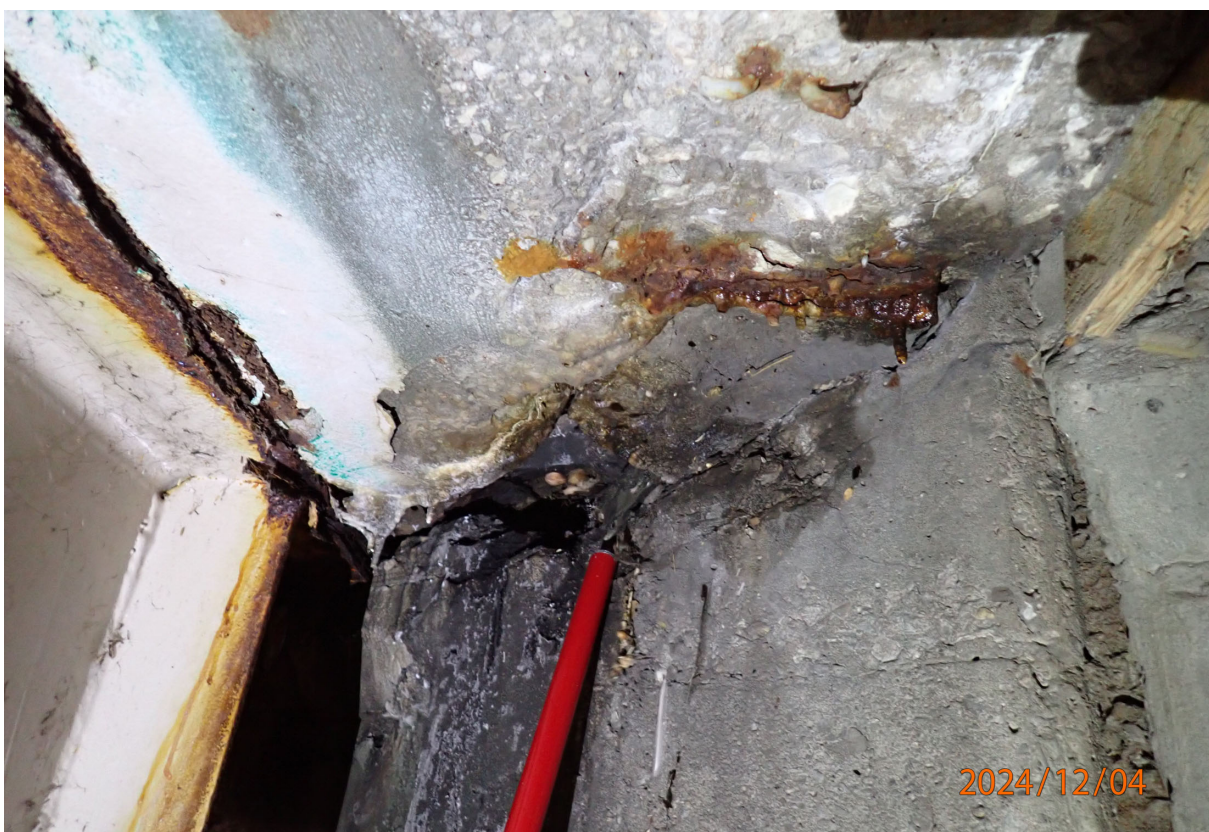
Spalling in Abutment 5 backwall and soffit at longitudinal joint
