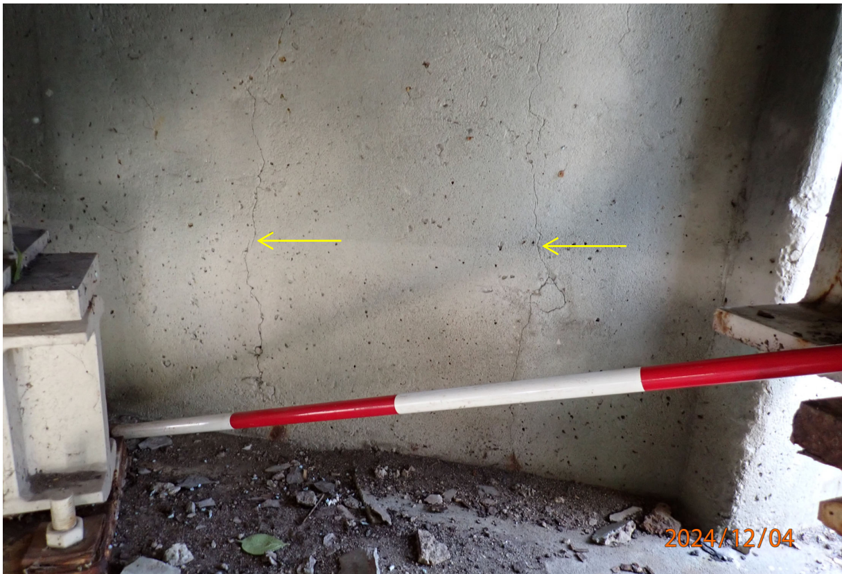
The backwalls have vertical cracks spaced at less than 3 feet in some areas (west end of Abutment 1 shown).
