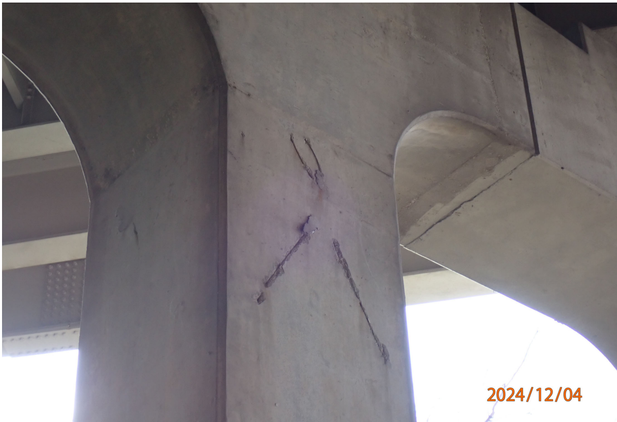
Pier 2-Columns 2 and 4 and Pier 4-Column 4 have shallow spalls with exposed tie wire (Pier 2-Column 2 shown).
