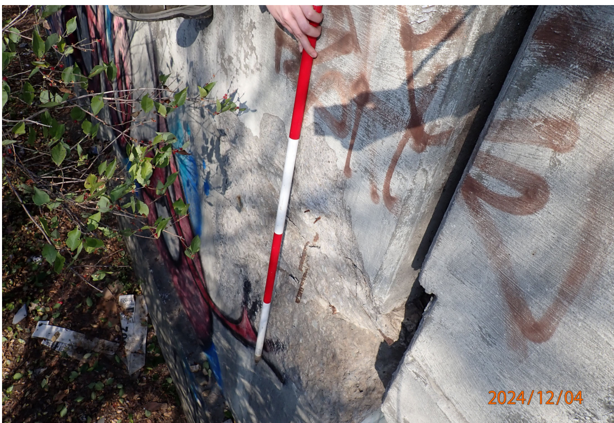
Northwest wingwall has a 3-foot-diameter spall with exposed rebar.
