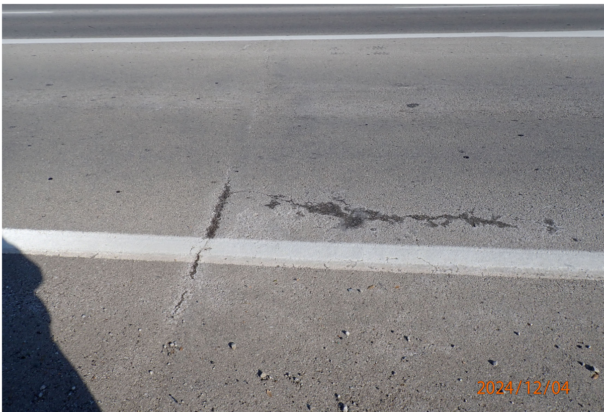
Overlay has transverse cracking in the right SB lane north of Pier 2 in Span 2.
