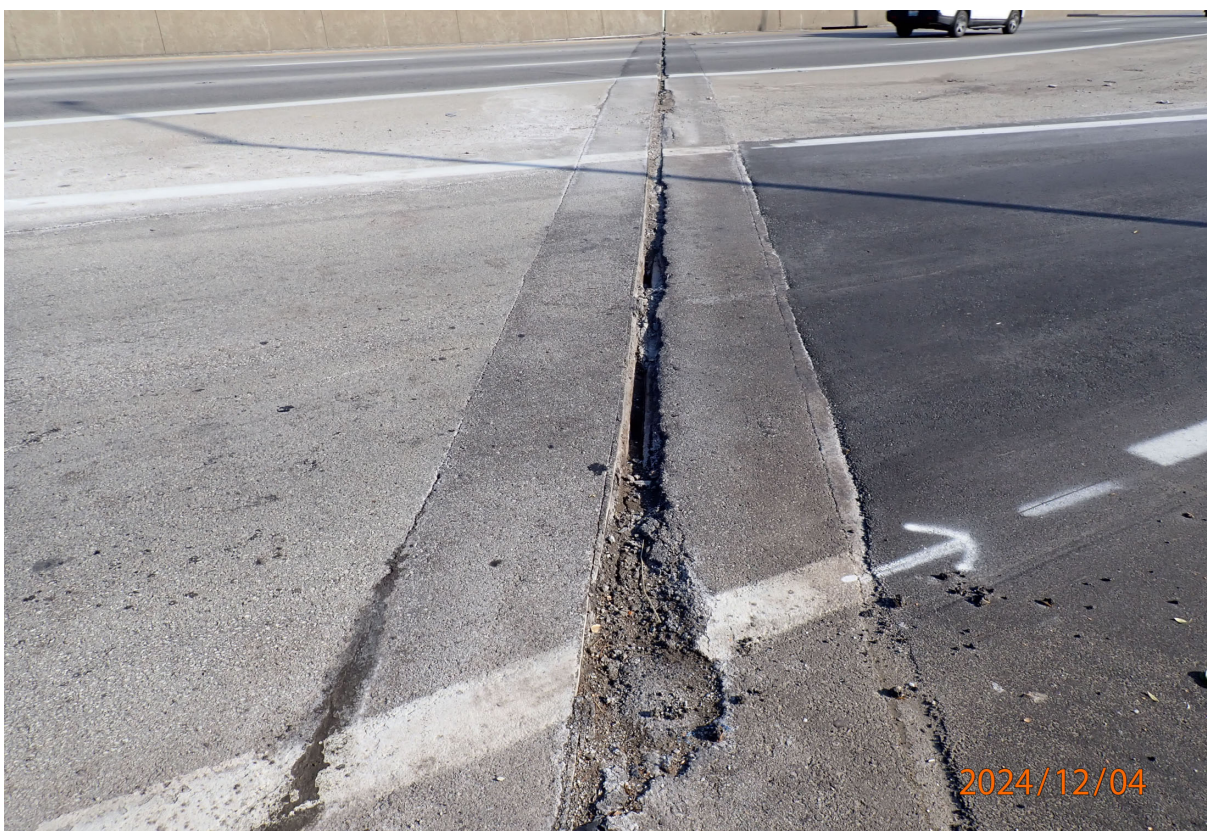
Asphalt plug joint over Abutment 1 (SB)
