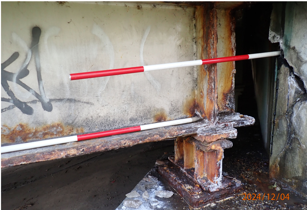
Some beam ends have flaking corrosion on the flanges (Beam 19 at Abutment 5 shown).
