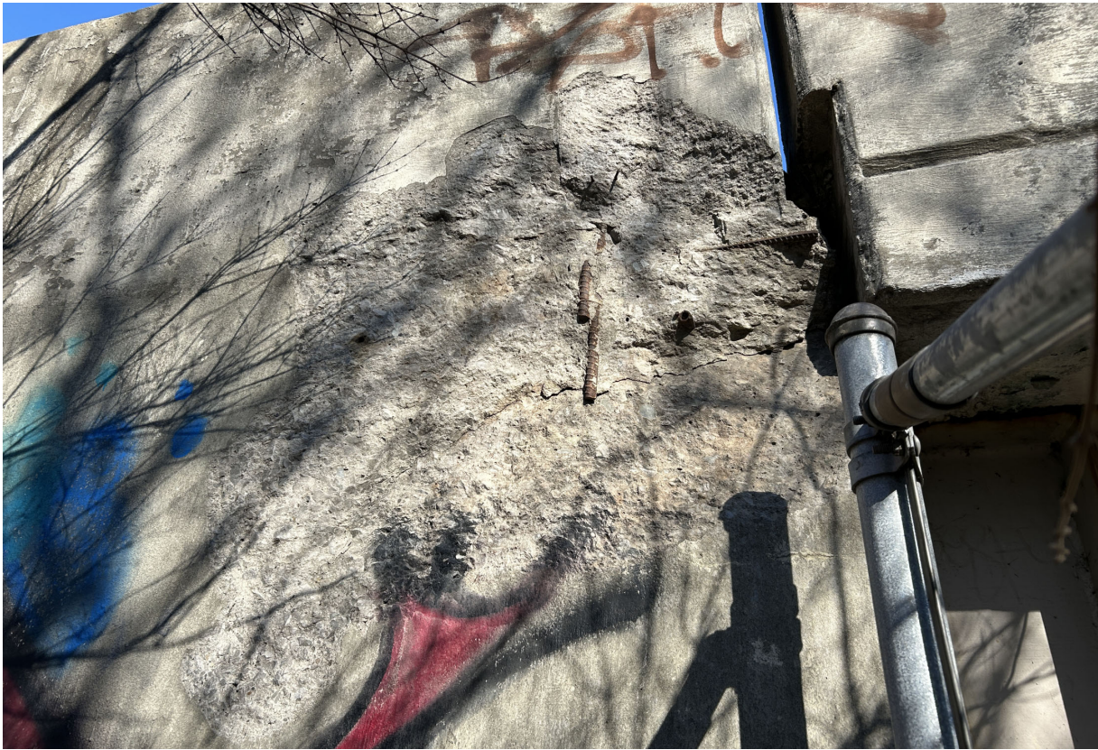
3' diameter by 8" deep spall with exposed rebar in northwest wingwall
