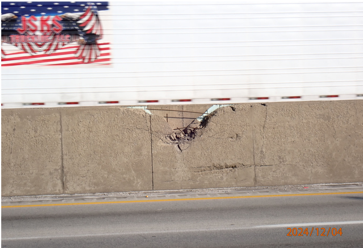
The SB median barrier has a 6' L x full depth spall with exposed rebar in Span 3.
