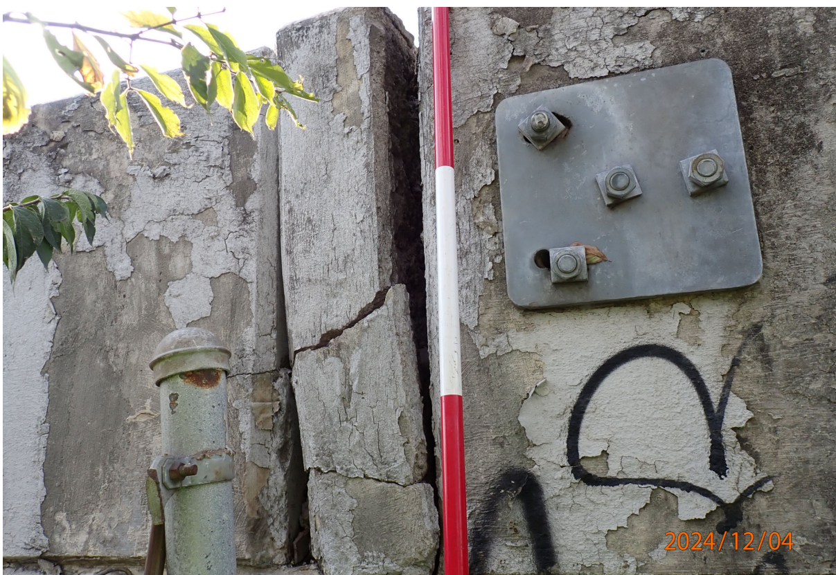
The section of the east railing above the Abutment 4 expansion plate is fractured (exterior face shown).
