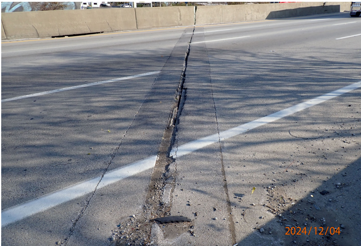
Asphalt plug joint over Abutment 5 (SB)
