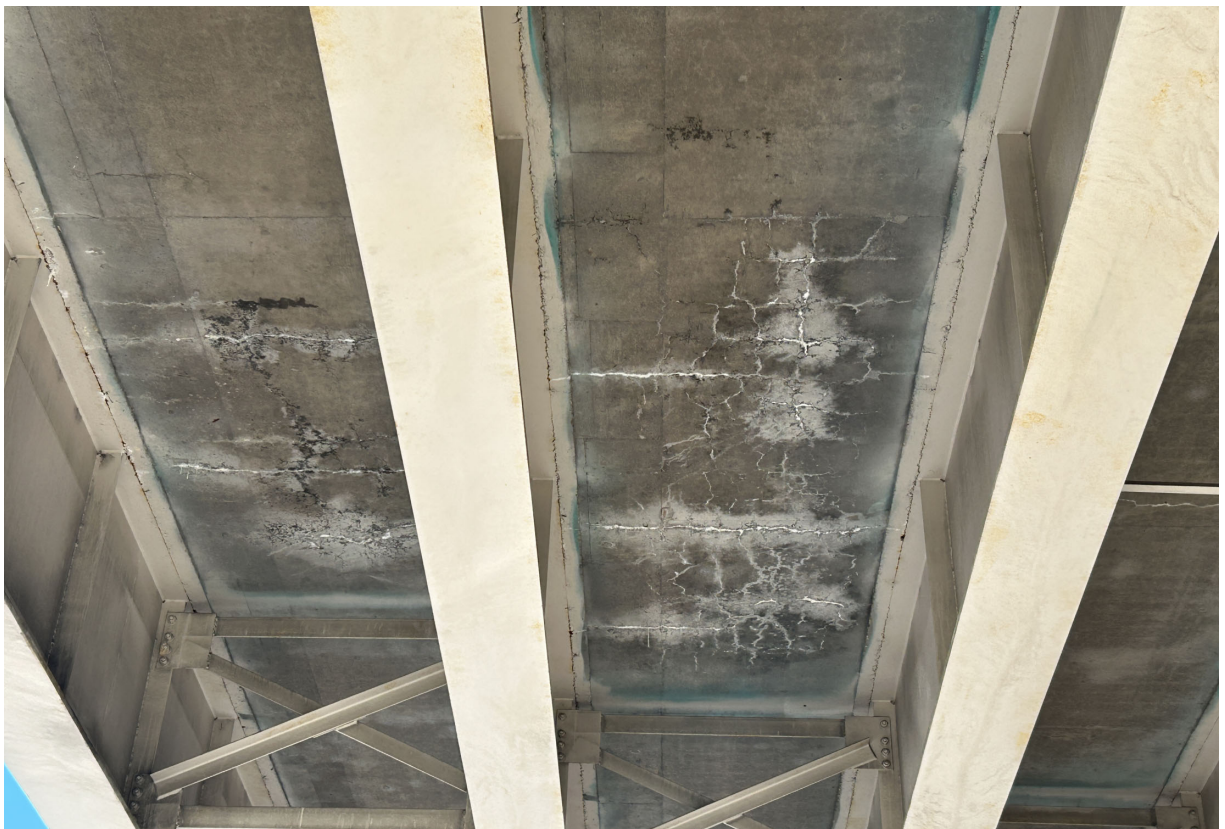
Soffit has areas of full depth deterioration in Bays 4, 6 and 7. Bays 6 and 7 shown.
