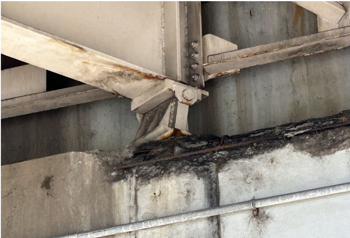
Abutment 2 has 8 feet of spalling with exposed rebar below Beam 6.
