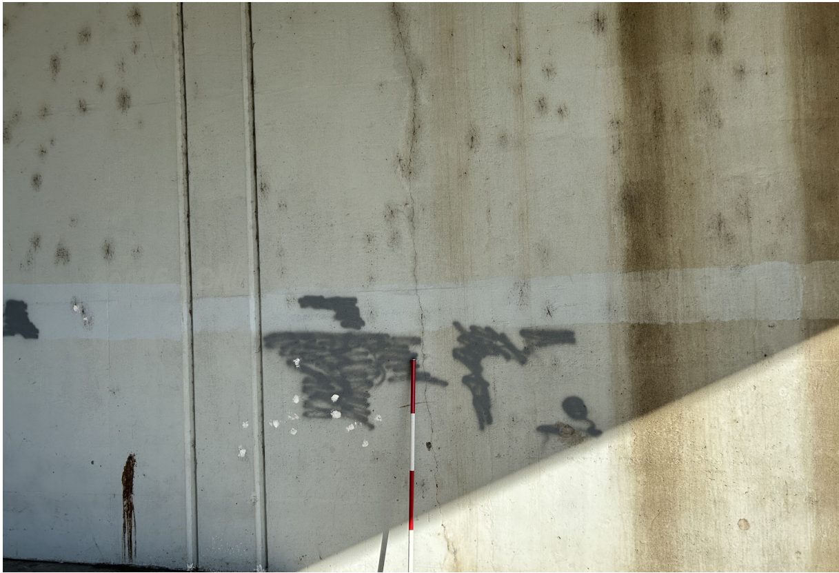
Abutment 2 vertical crack.
