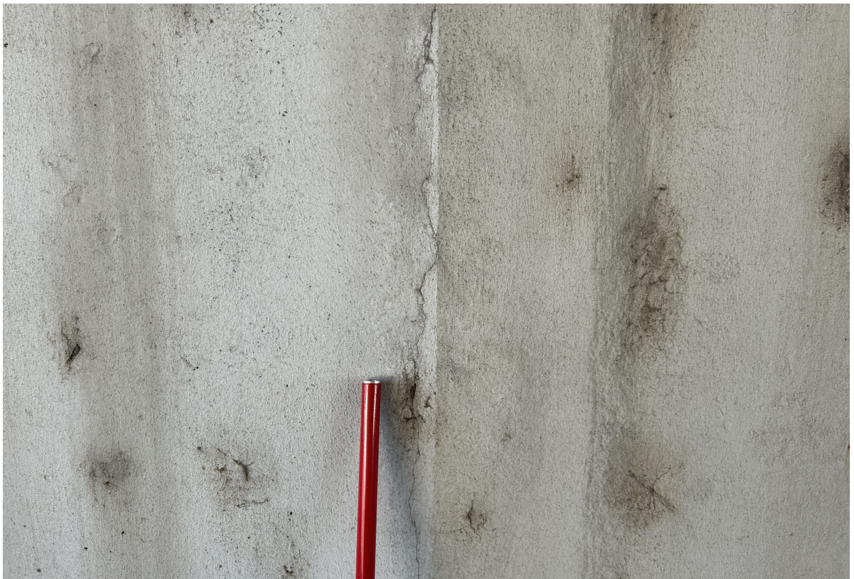
Abutment 1 vertical crack.
