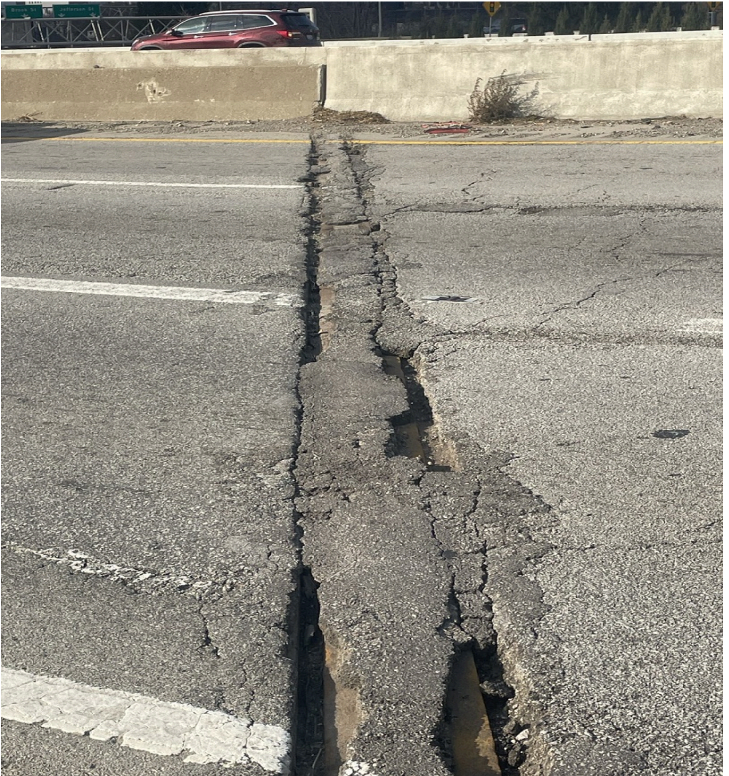
Pourable joint seal over Abutment 2.
