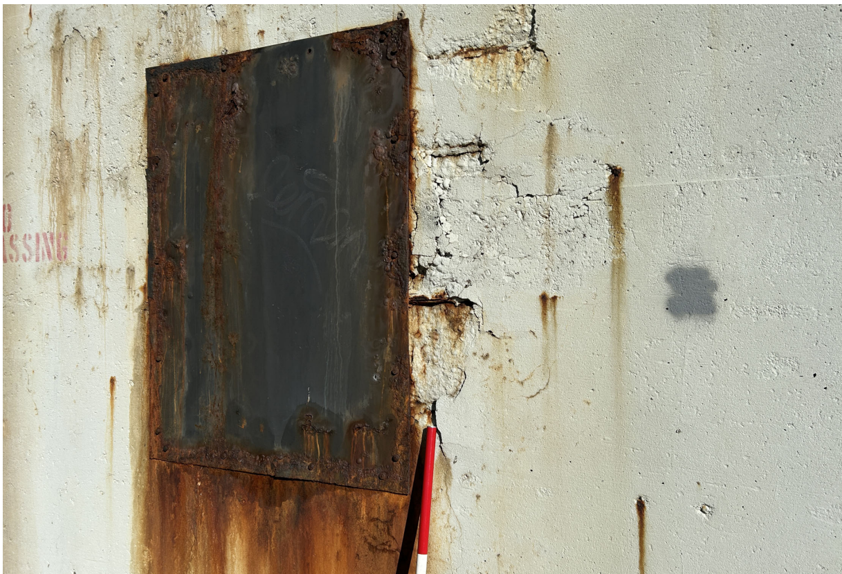
Abutment 2 has spalls with exposed rebar and rust staining around utility box at the east end.
