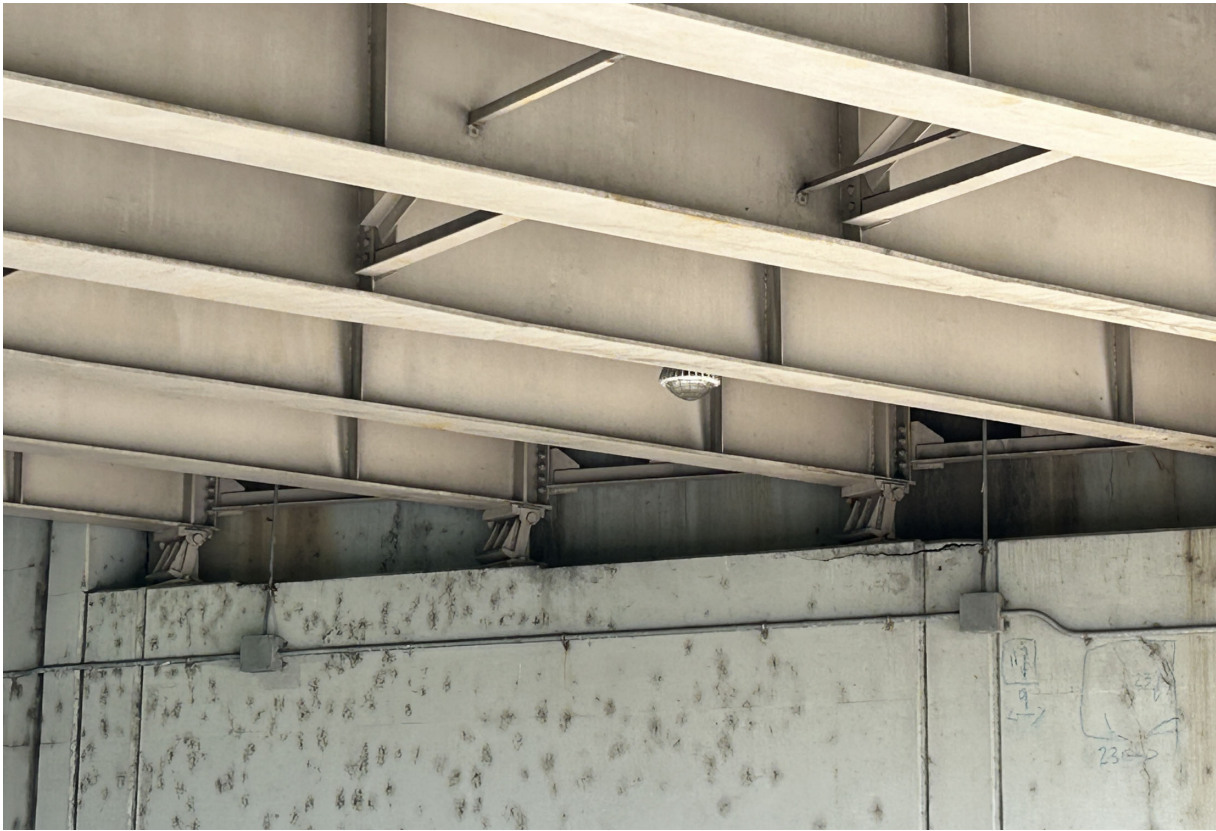
Rocker bearings at Abutment 2 are expanded.
