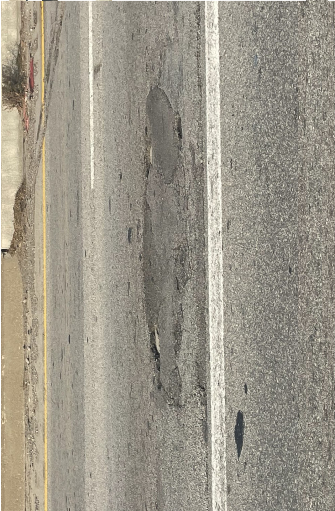
Deck overlay has several cracks and spalls. Center lane near the north bridge end has asphalt patching and spalling exposing the bridge deck.
