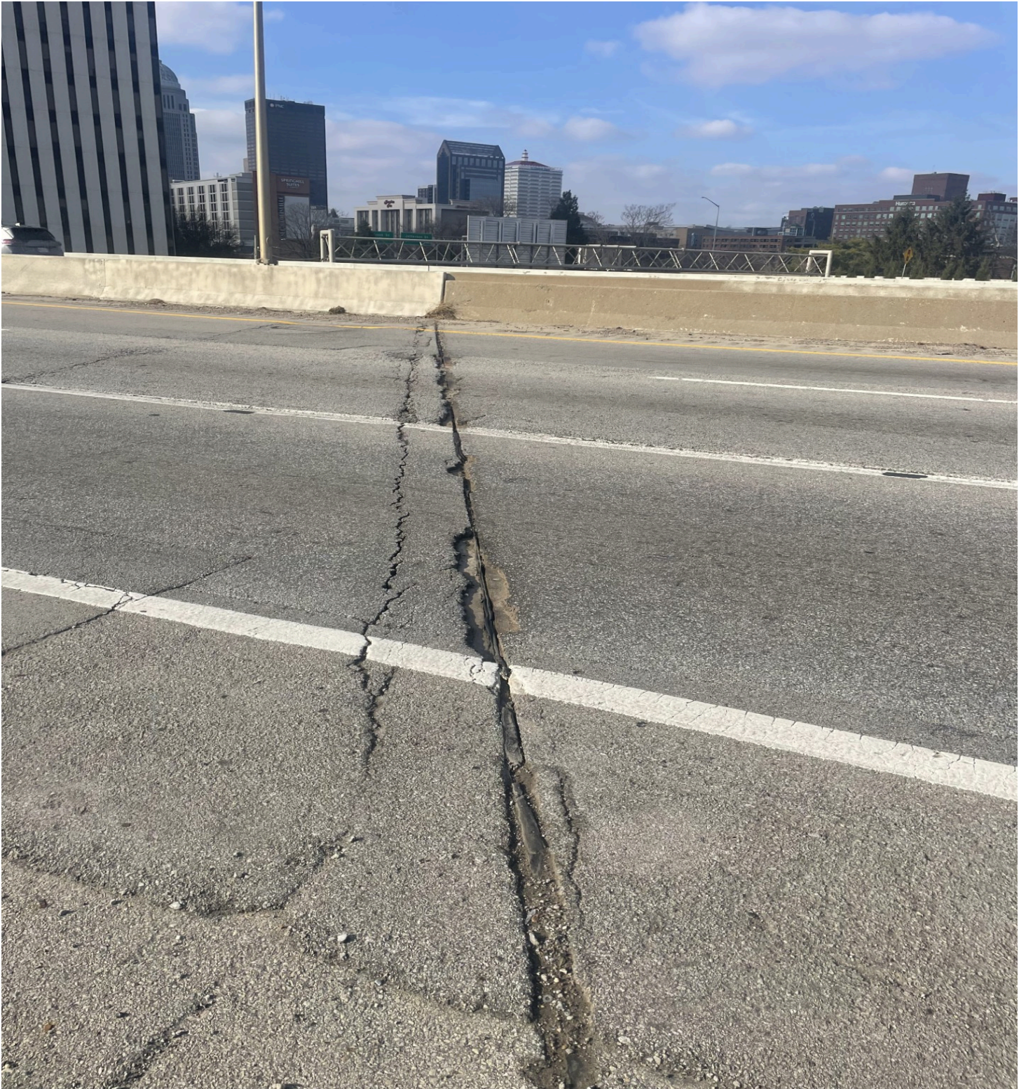
Pourable joint seal over Abutment 1.
