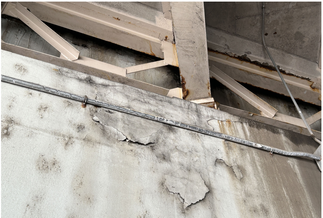
Abutment 1 delamination below Beam 2.
