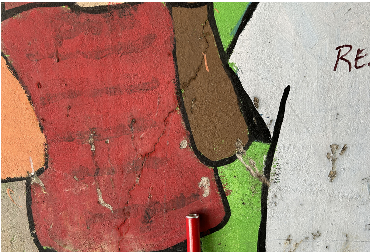
Abutments have moderate to wide full height vertical cracks.
