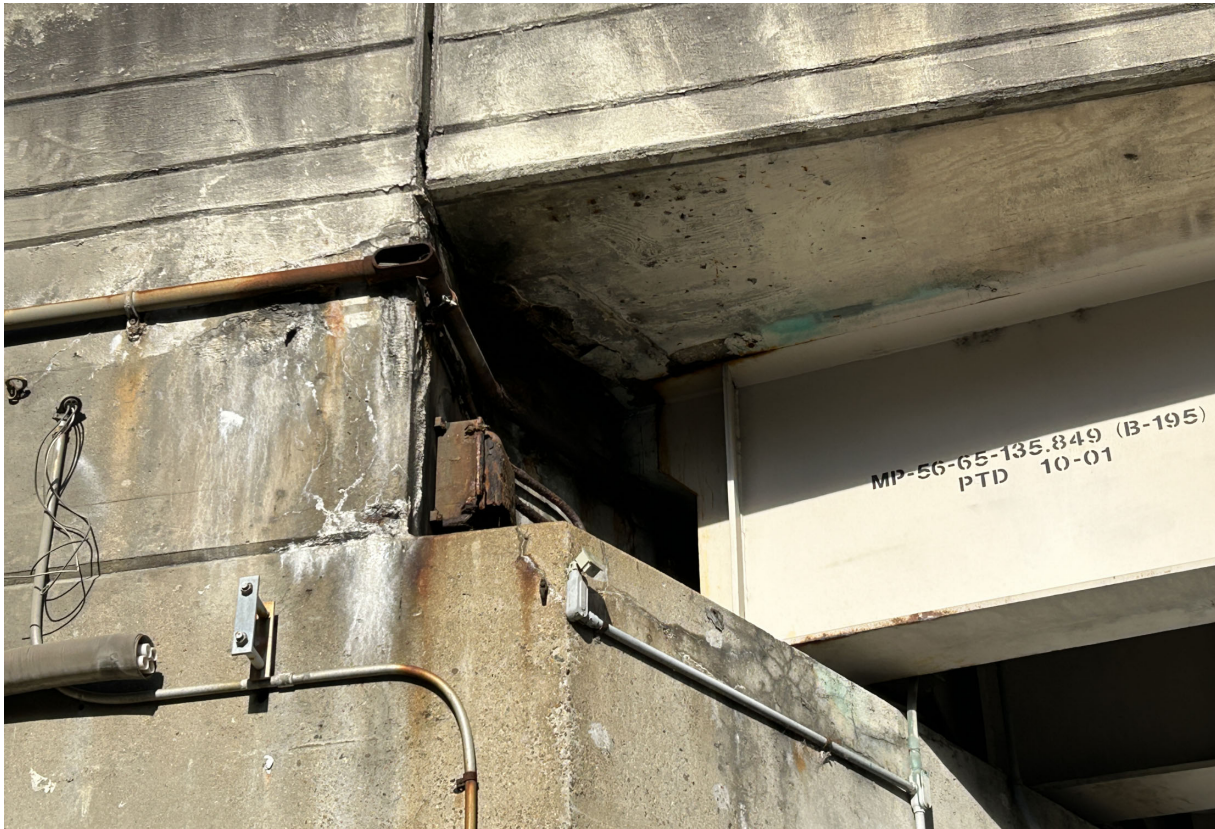
East end of Abutment 1 has cracking and efflorescence below Beam 10 and in the backwall.
