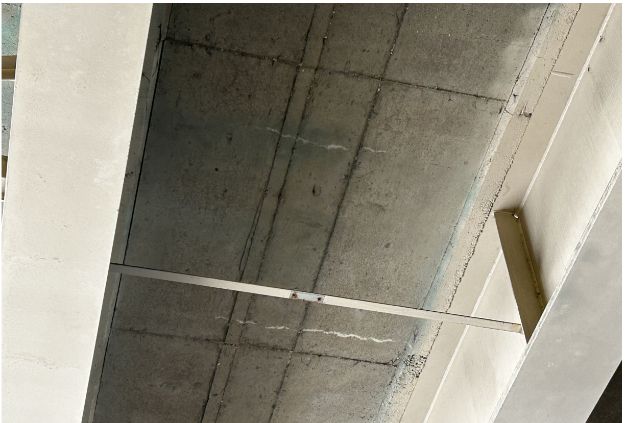
Soffit has some transverse cracks with efflorescence, mainly in Bays 7-9.
