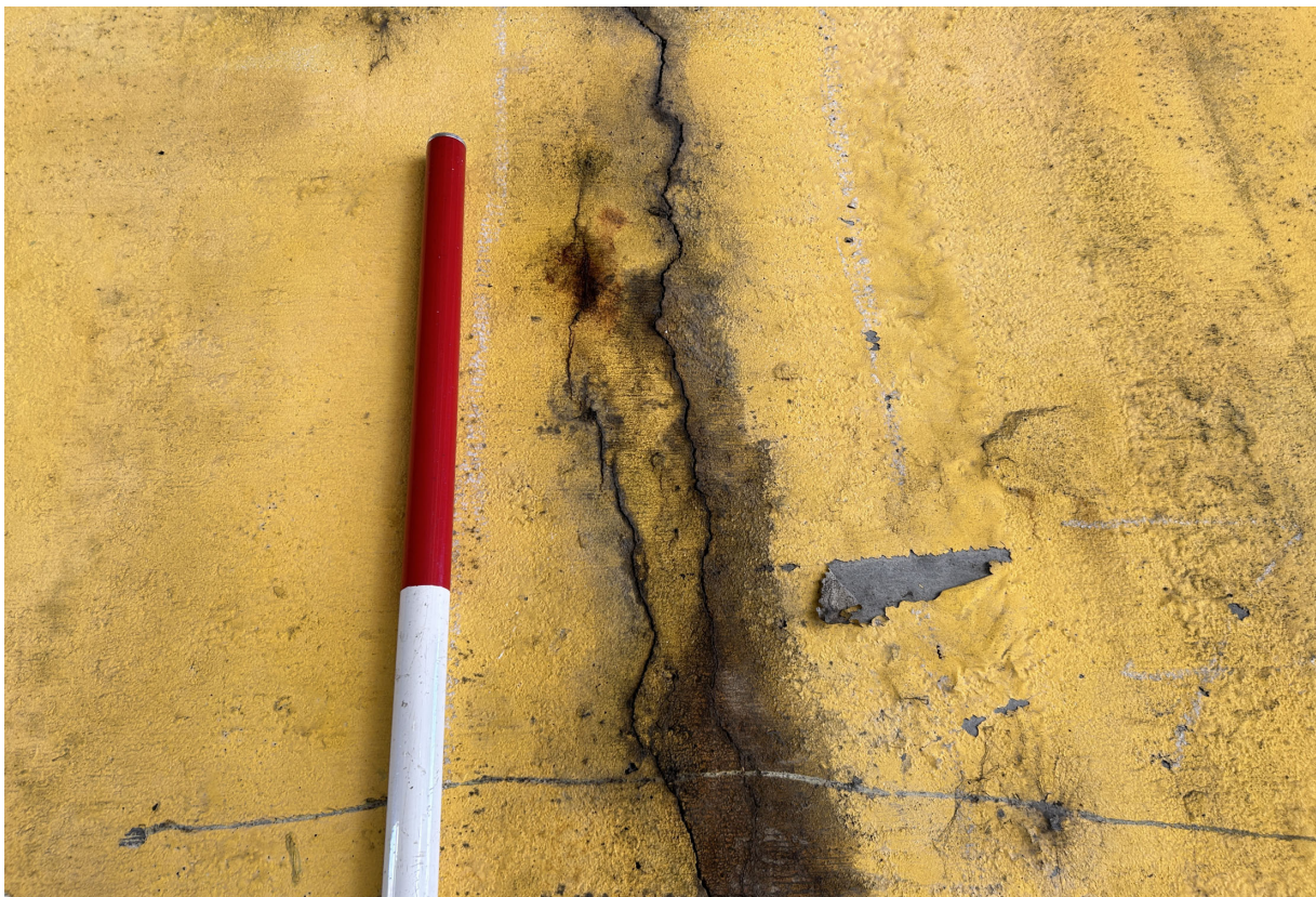
Abutment 2 full height wide vertical crack.
