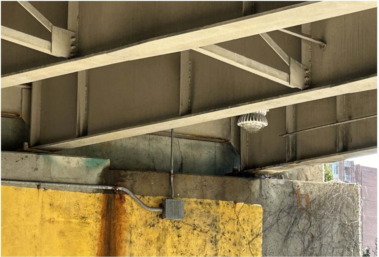
Bearings 9 and 10 at Abutment 2 have pack rust between the bearing and masonry plate.
