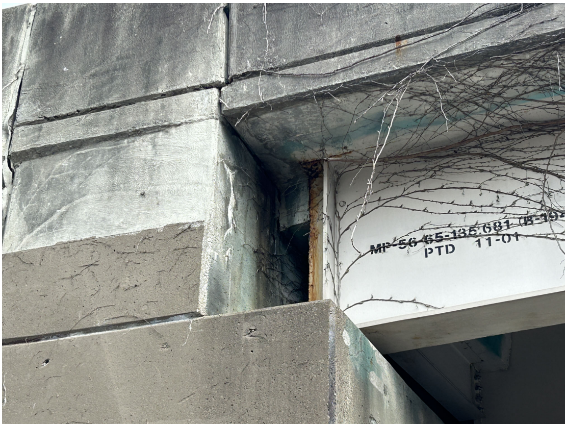
Abutment 2 backwall has cracking with efflorescence at the ends. West end shown.
