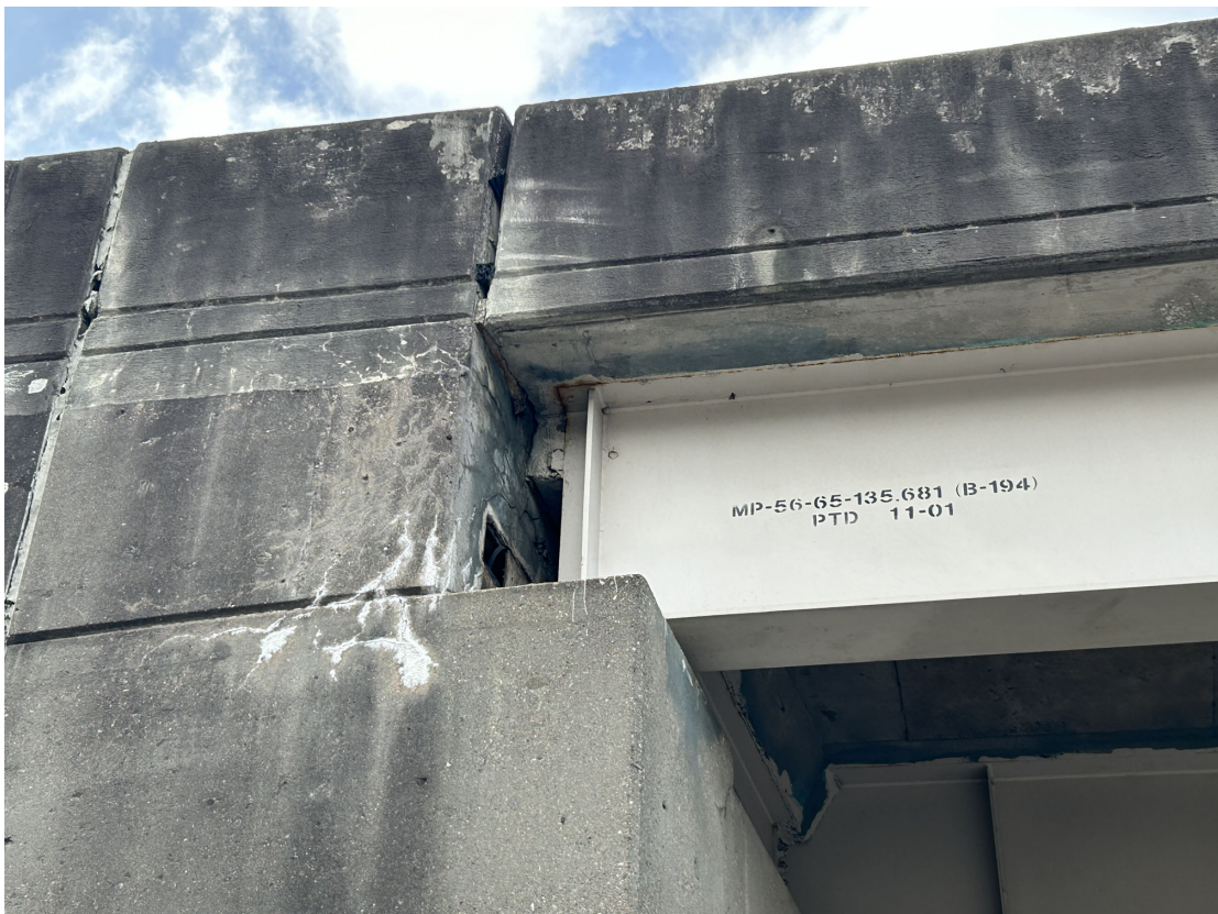
SE wingwall also has dense pattern cracking near the top.
