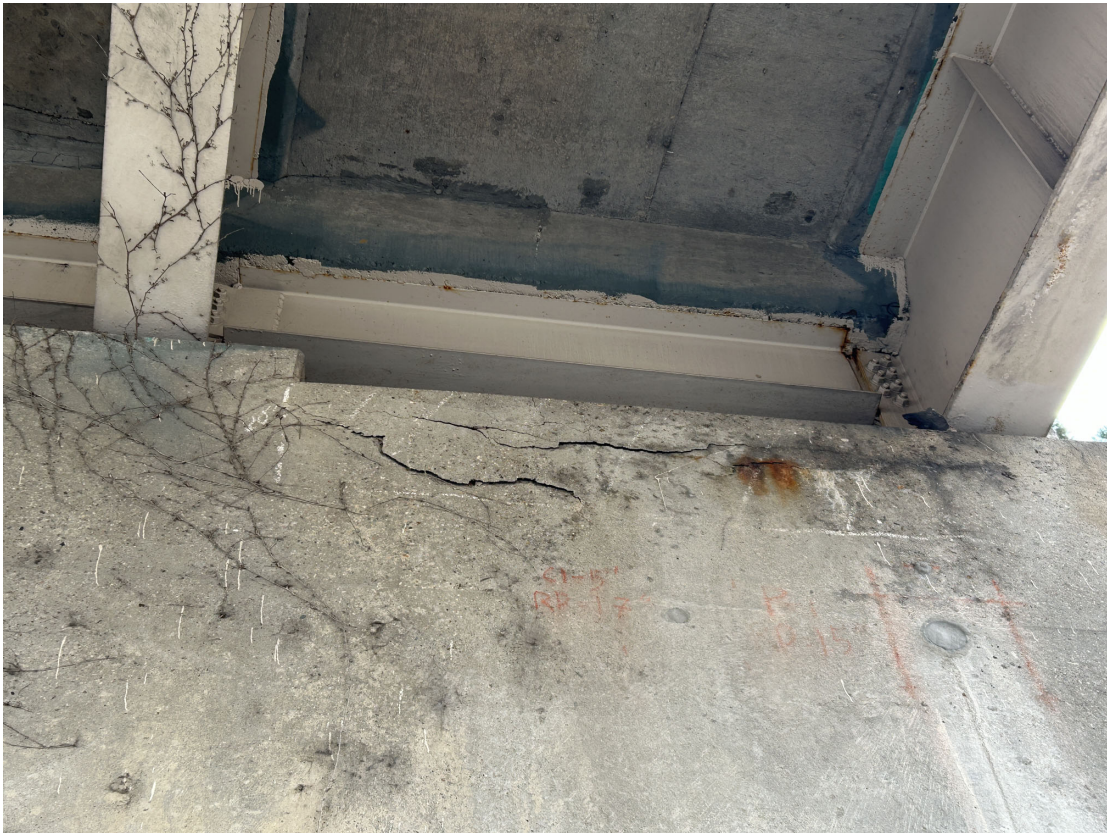
Abutment 1 has wide horizontal cracking with some rust staining near the top of the seat under Bay 1.
