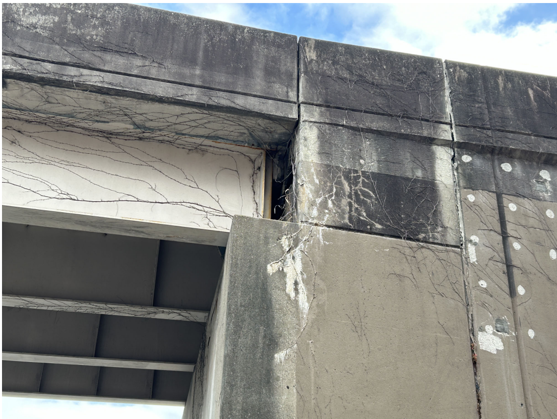
SW wingwall has dense pattern cracking with efflorescence near the top.
