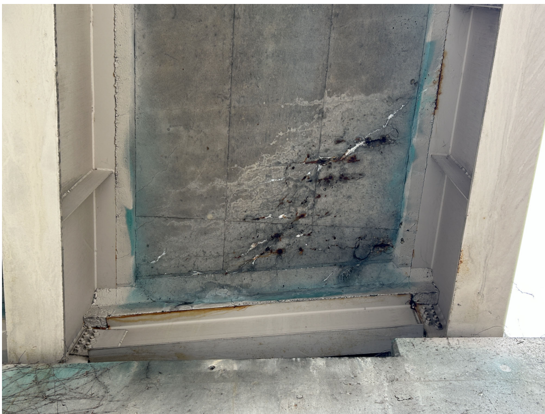
Soffit has an area of full depth deterioration in Bay 3 at Abutment 2.
