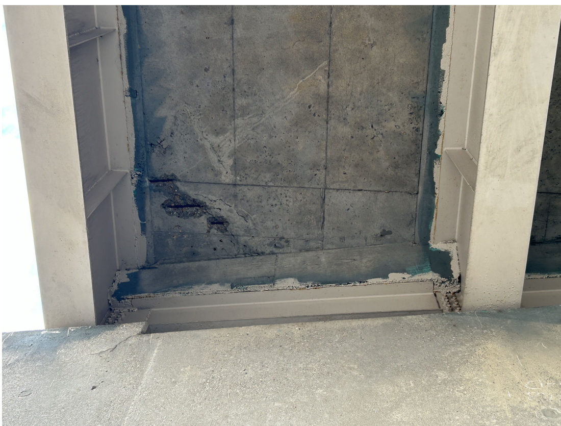
Deck soffit has an area of spalling with exposed rebar in Bay 3 at Abutment 1.
