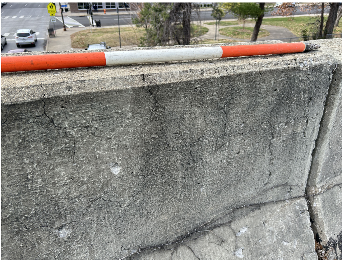
West rail has cracking throughout the length.
