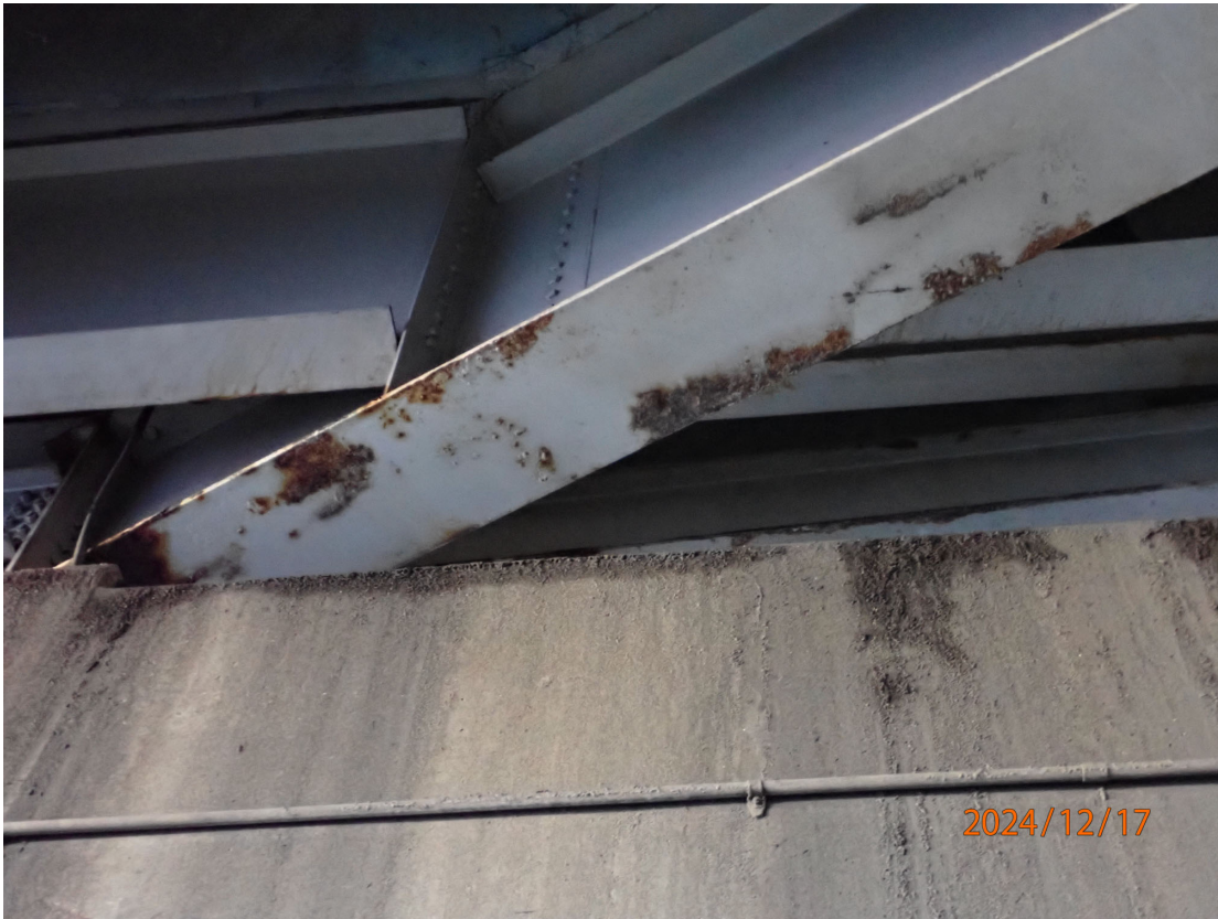
Girder ends typically have corrosion near the substructure units. Example Span 1-Pier 2-Girder 9.
