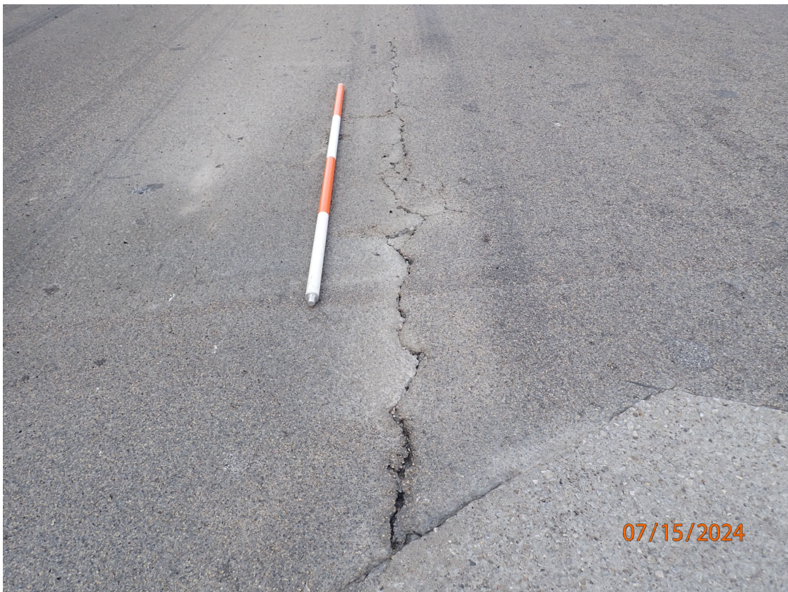
SB Lanes: Wide Crack from Concrete Patch (typical; closer view)
