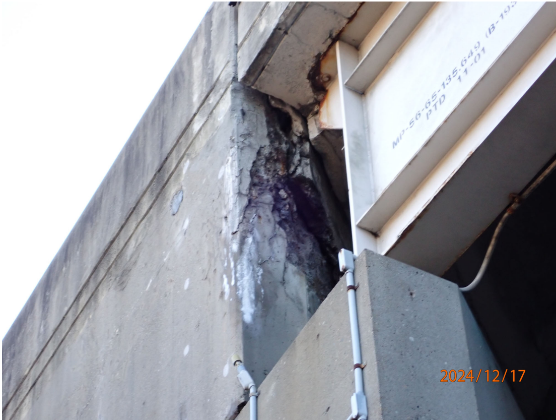
Abutment 6 back wall has dense pattern cracking and deep spalling at the west end.
