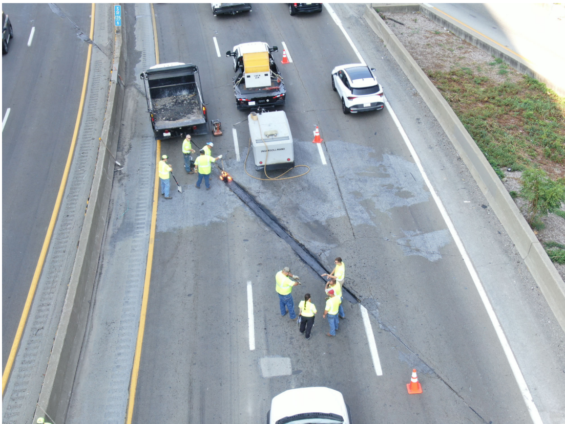
SB Lanes: Pourable Joint over Abutment 1 (drone view)
