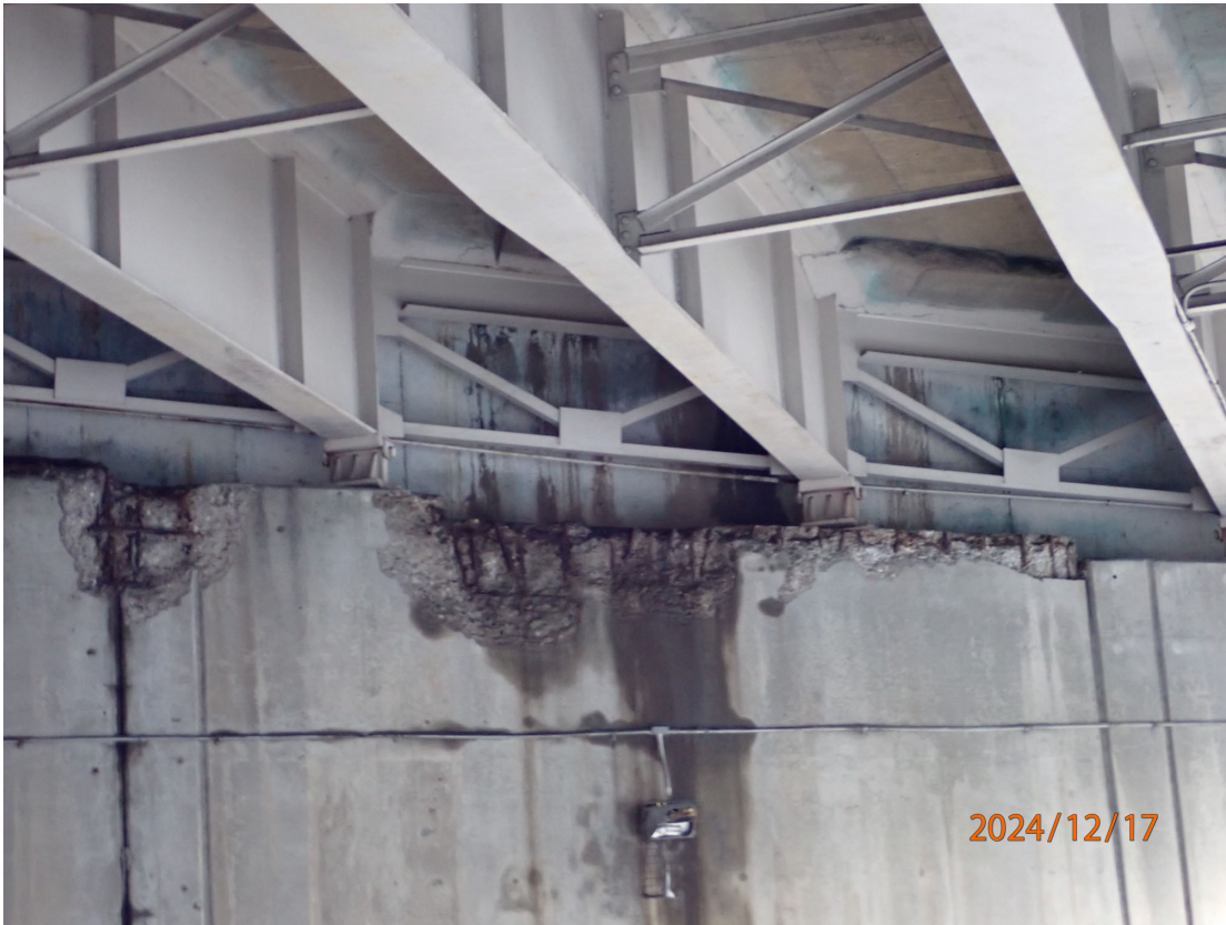
Abutment 6 has large, deep spalls with exposed rebar along the top of the beam seat. Example below Bays 9-11.
