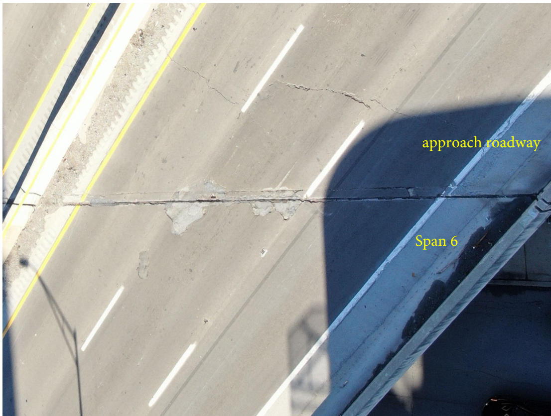
Joint over Abutment 6 NB Note patches along the joint extending into Span 6 in the center lane.
