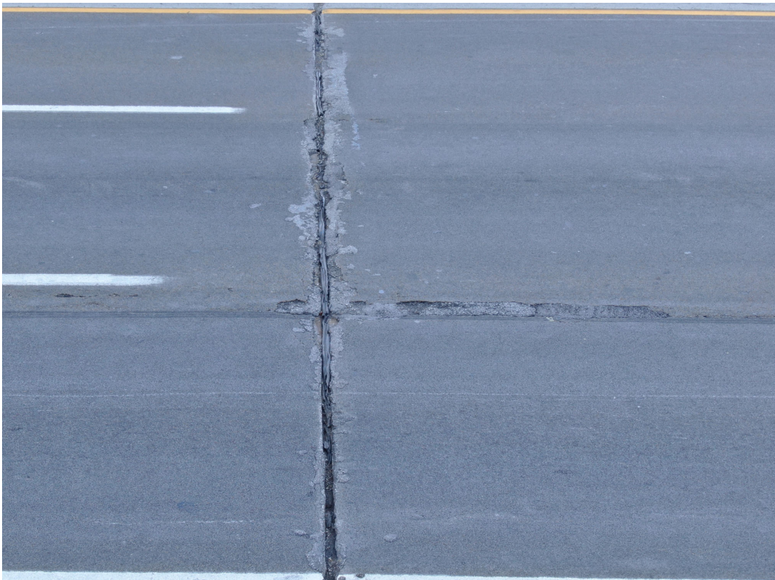
Close-up of joint over Pier 4 with original deteriorated joint seal visible.
