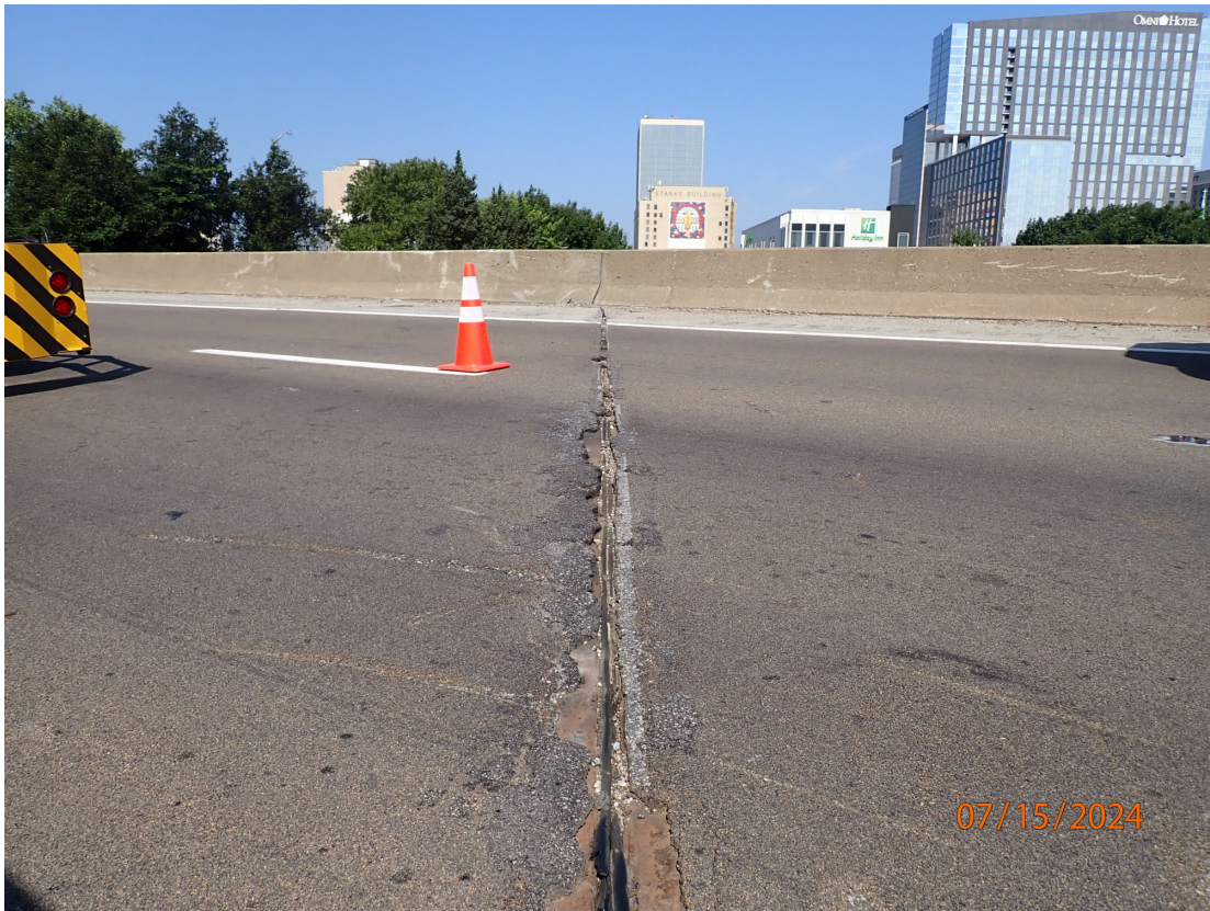
SB Lanes: Pourable Joint over Pier 5
