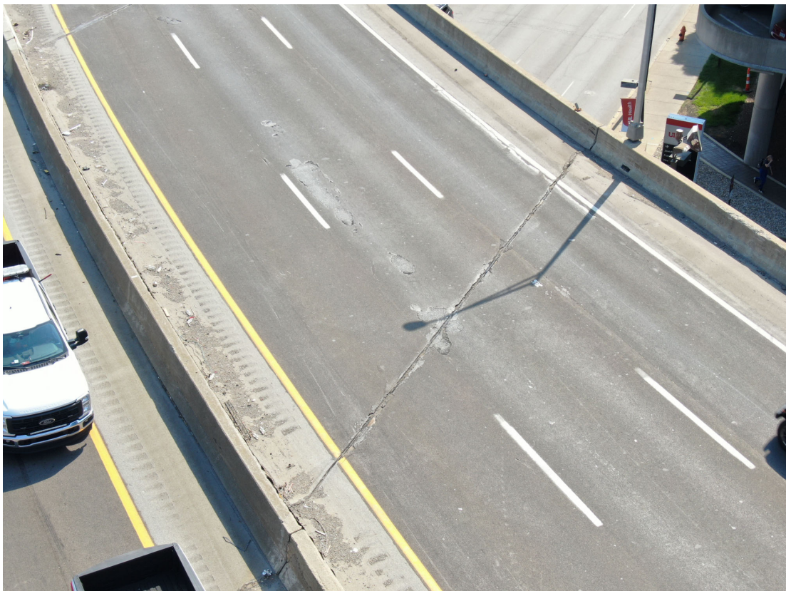
NB Lanes: Asphalt Patches in Span 6 (drone view)
