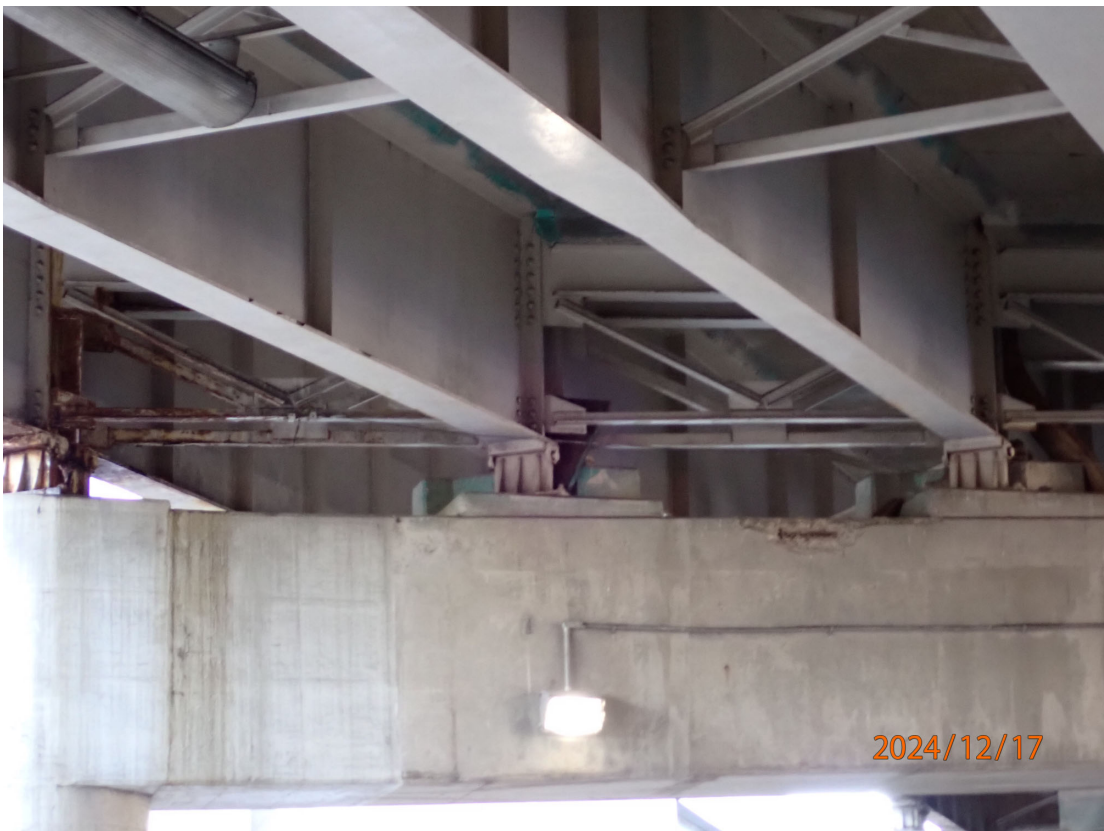
Pier 5 typical bearings
