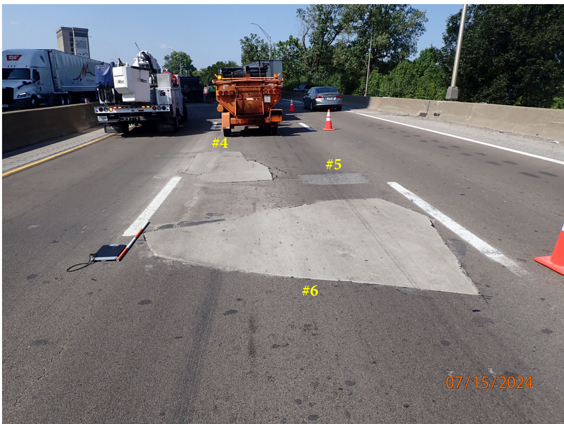
SB Lanes: Concrete Patches #4-6 in Span 1 (closer to P2 joint)
