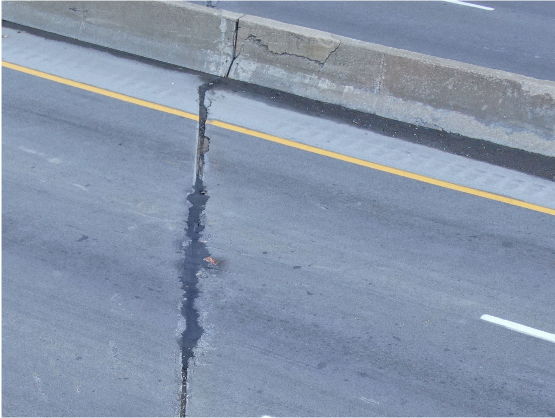
Joint over Pier 5 SB has generally failed. There is asphalt patching in the center and left lanes. Also not patch in median railing.
