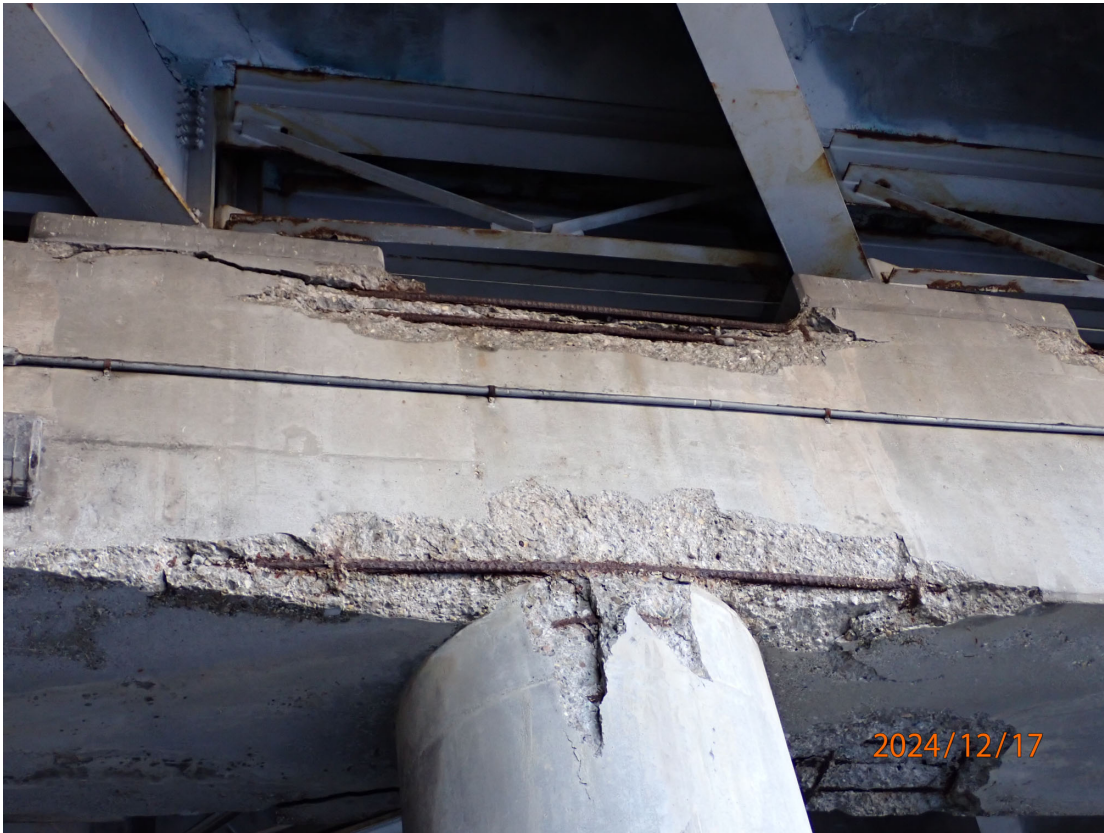
Close-up of deep spalling in the Pier 5 cap north face at Column 2 as well as spalling in the column.
