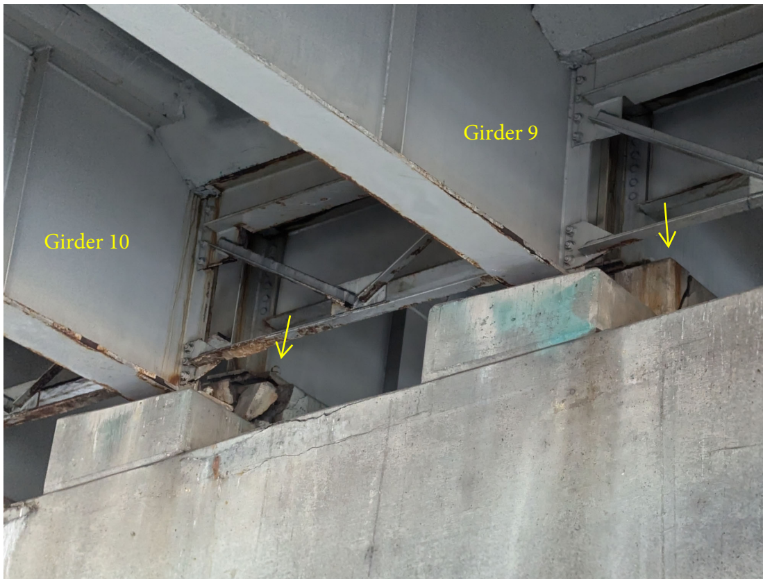
Pier 3 north face at Girders 9 and 10. Pedestal for girder 9-Span 2 has a wide crack, and pedestal for Girder 10-Span 2 has a deep spall, potentially causing loss of bearing area.
