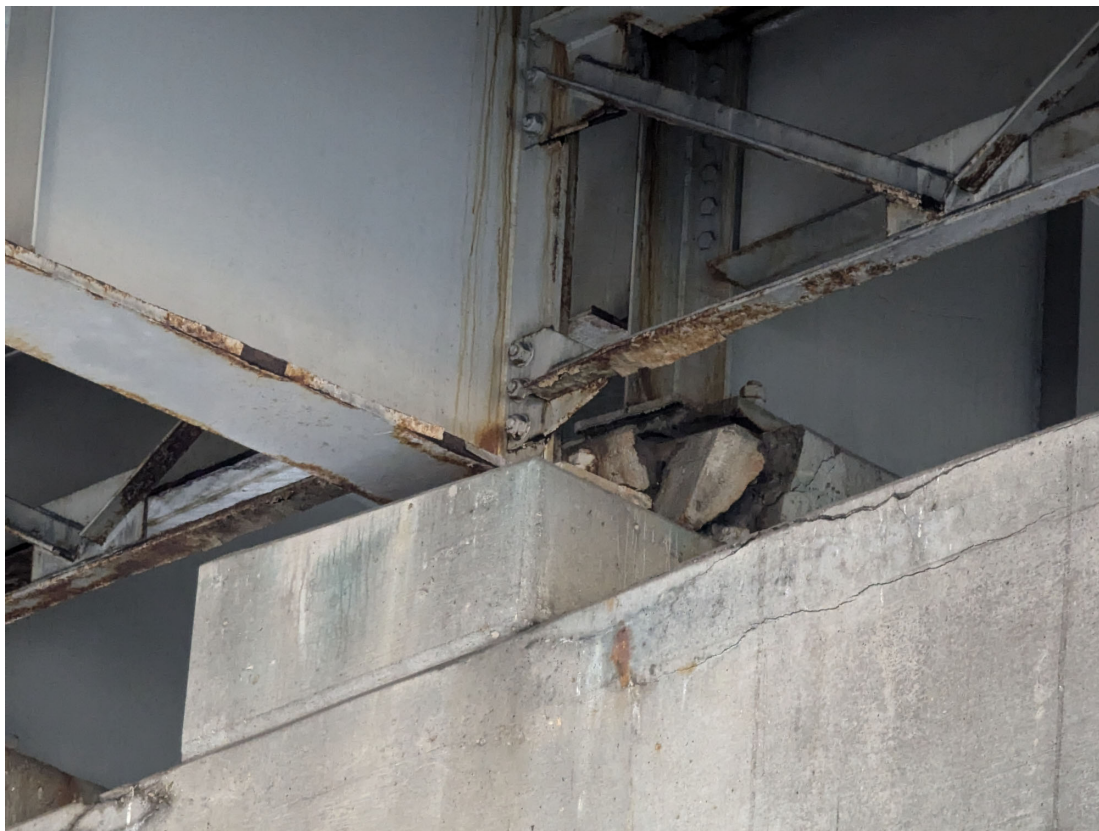
Closer view of pedestal for Pier 3-Girder 10-Span 2 spalling, plus wide cracking in the north face of Pier 3 cap.
