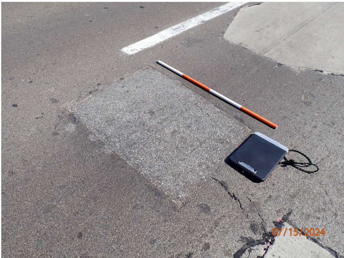
SB Lanes: Concrete Patch #5 = 3'L x 4'W = 12 SF
