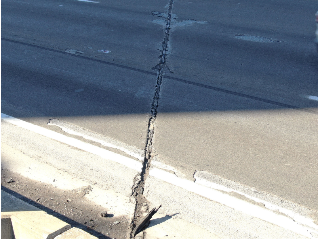
Joint over Pier 5 NB has failed and original torn joint material is exposed.
