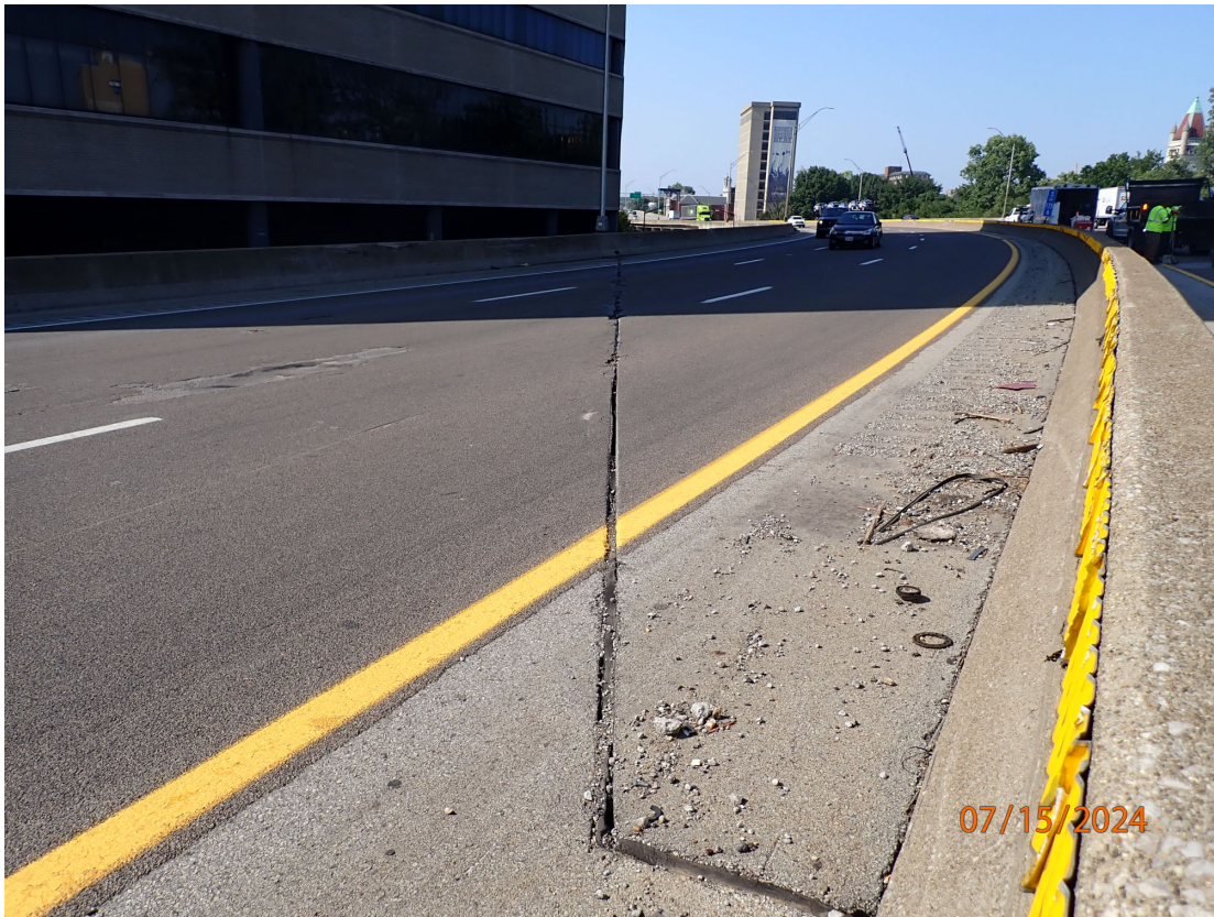
NB Lanes: Pourable Joint over Pier 2
