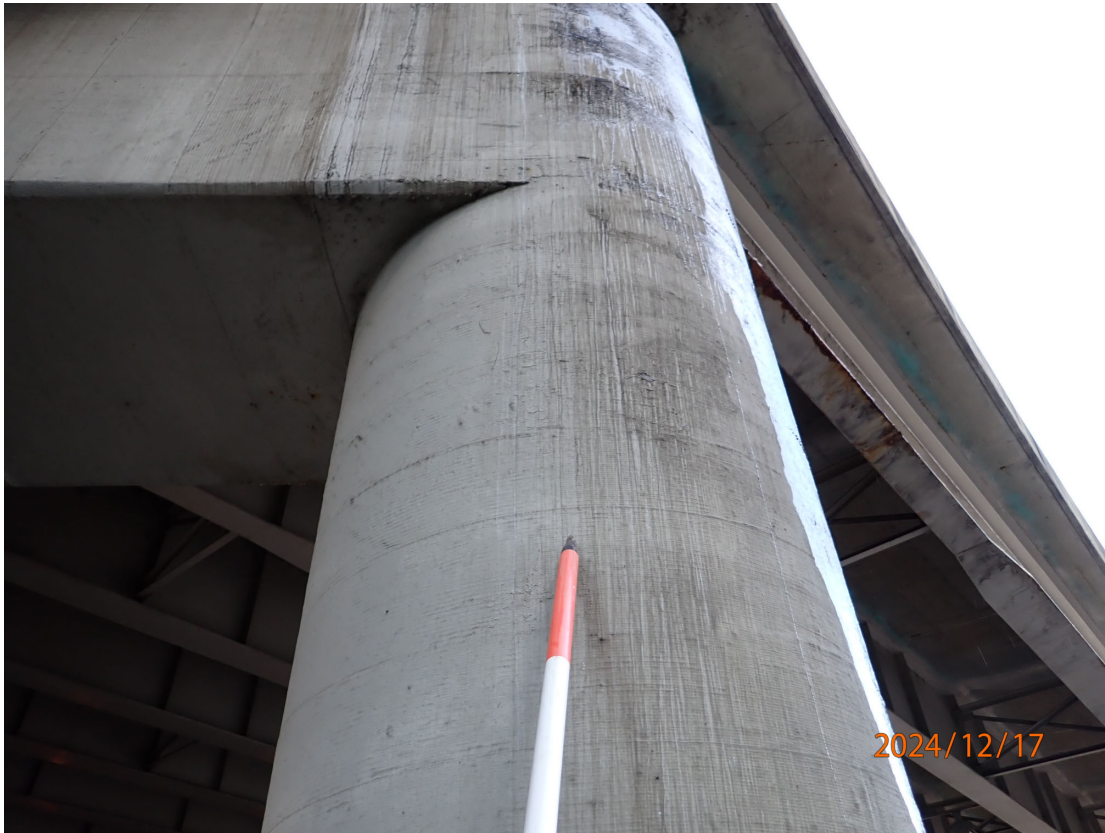
Pier 5-Column 6 and the east end of Pier 5 cap have CFRP repair from 2009. Repairs are in good condition.
