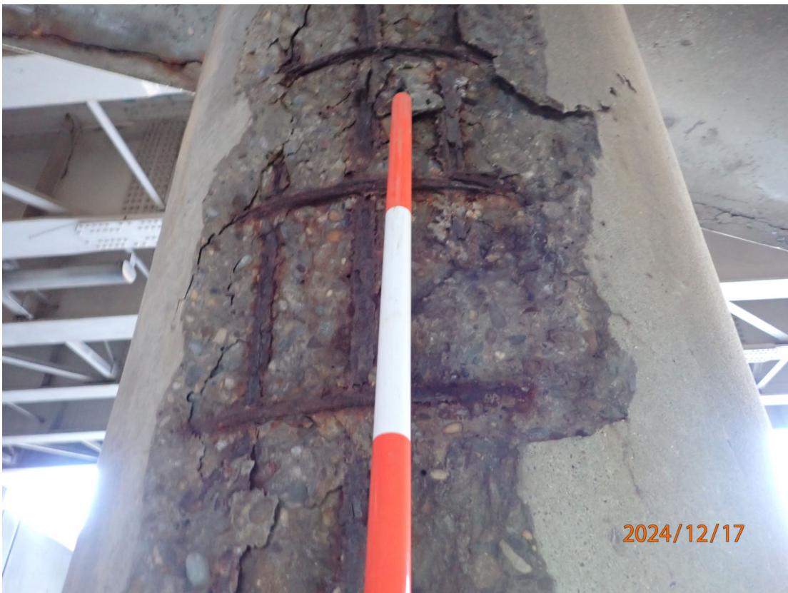
Close-up of Pier 2-Column5 spall with exposed rebar having section loss.
