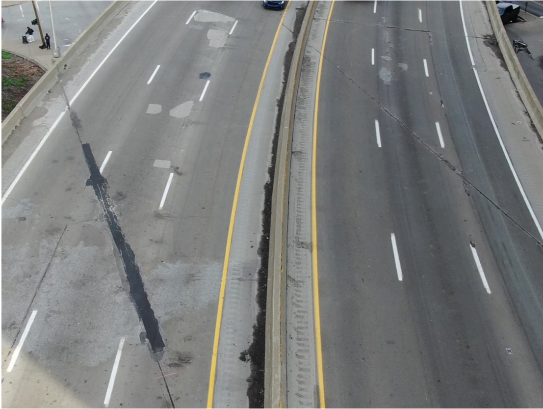
Abutment 1 SB joint plus Span 1. SB Span 1 deck and overlay has several full depth concrete patches. SB joint has been patched numerous times with asphalt and is cracking in the center lane.
