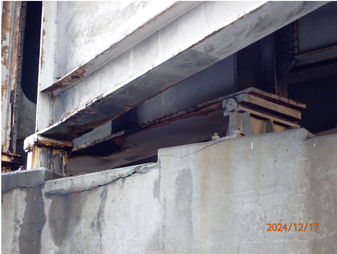
Wide cracking in the east end of Pier 2 north face, plus typical Pier 2 bearings.
