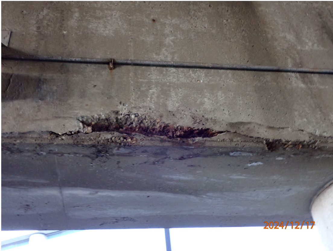
Another example of cracking and spalling in the Pier 2 cap between Columns 9 and 10.
