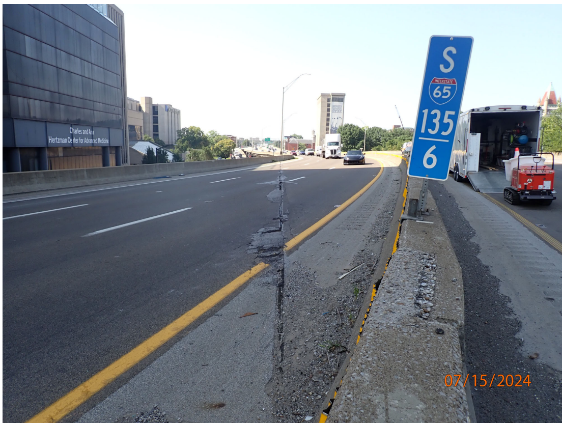
NB Lanes: Pourable Joint over Abutment 1
