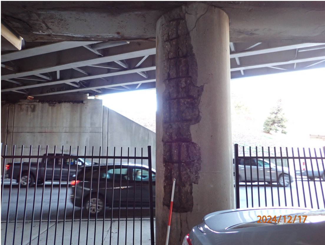
Pier 2-Column 5 has a large spall with exposed rebar, roughly 10 feet tall by 2 feet wide by 2.5 inches deep, on the north side.
