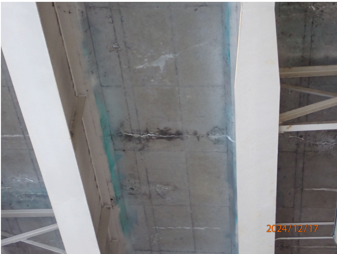
Example of transverse cracking in the deck soffit in Span 6.
