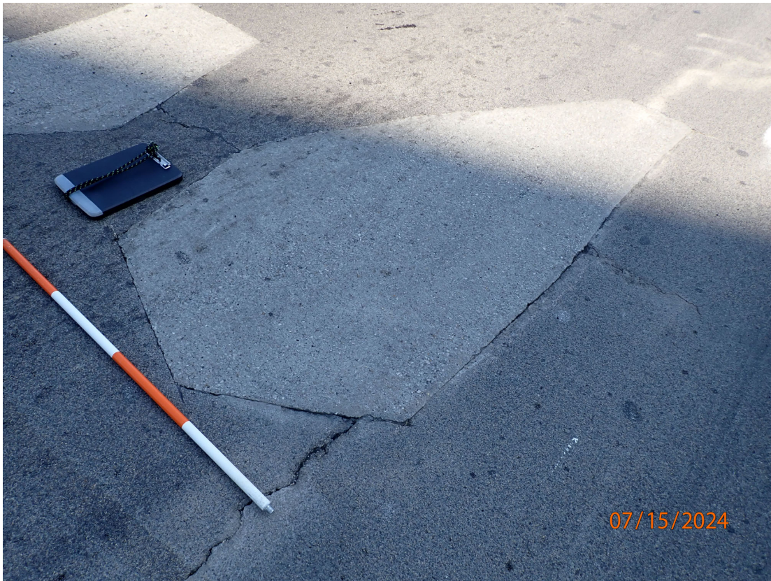
SB Lanes: Concrete Patch #3 = 8'L x 4'W = 32 SF
