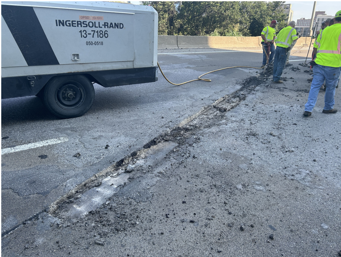
SB Lanes: Pourable Joint over Abutment 1 (before repair)
