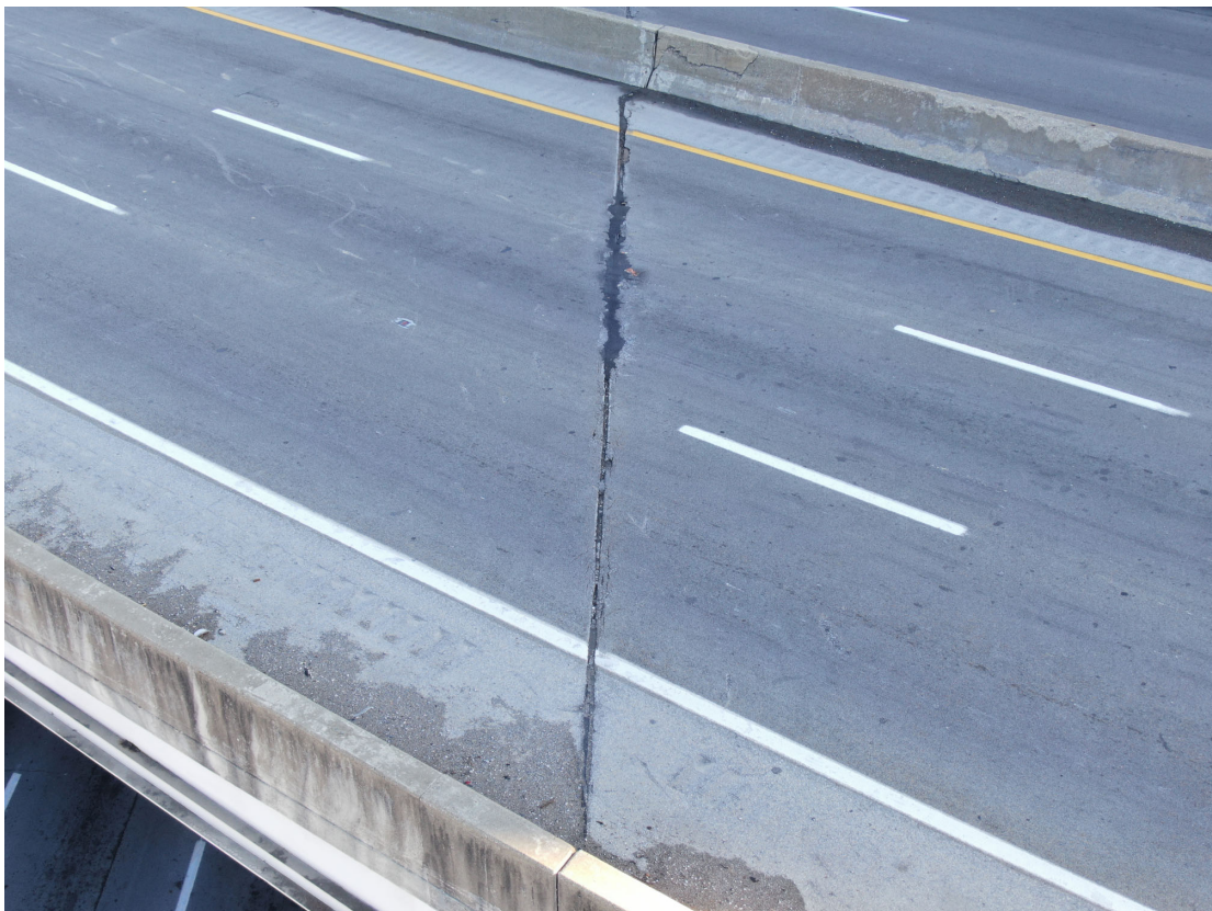
Joint over Pier 5 SB.
