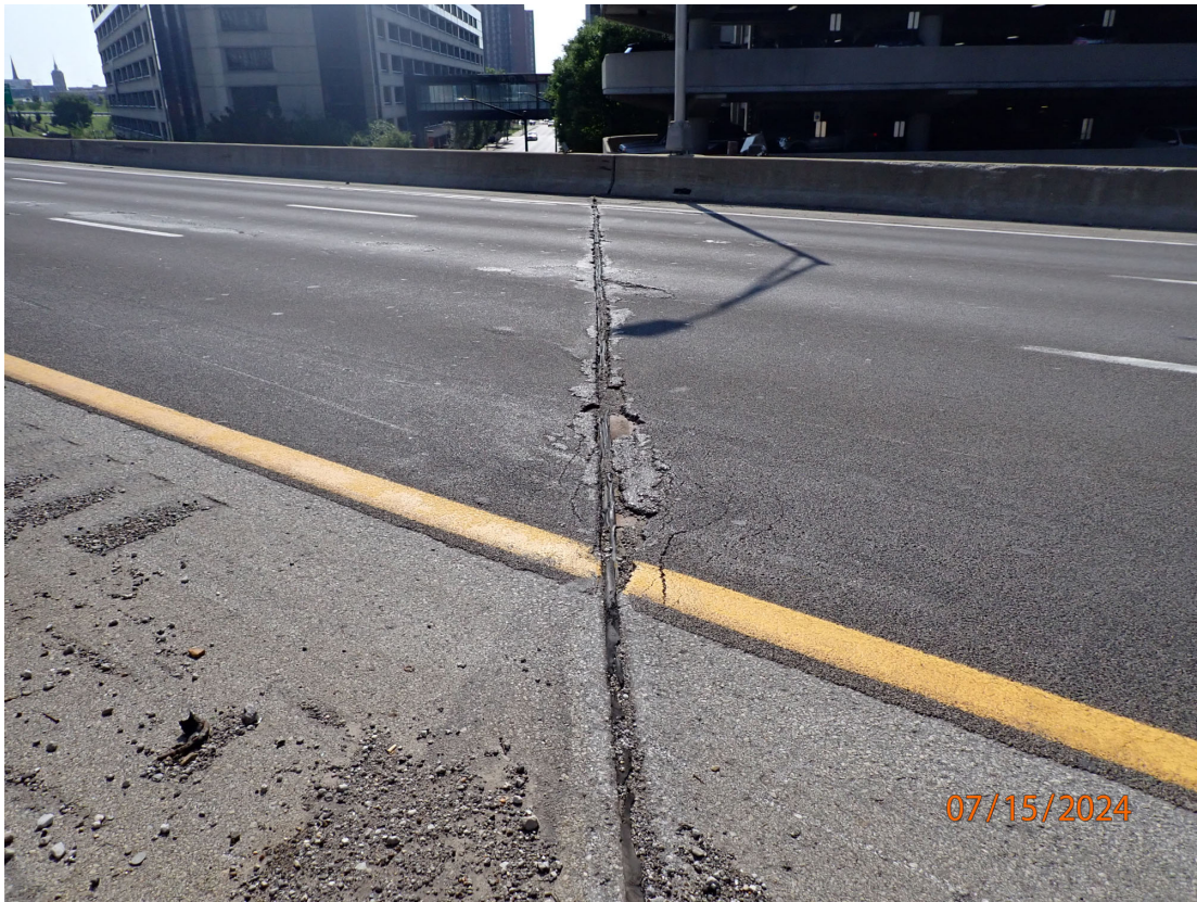
NB Lanes: Pourable Joint over Pier 5
