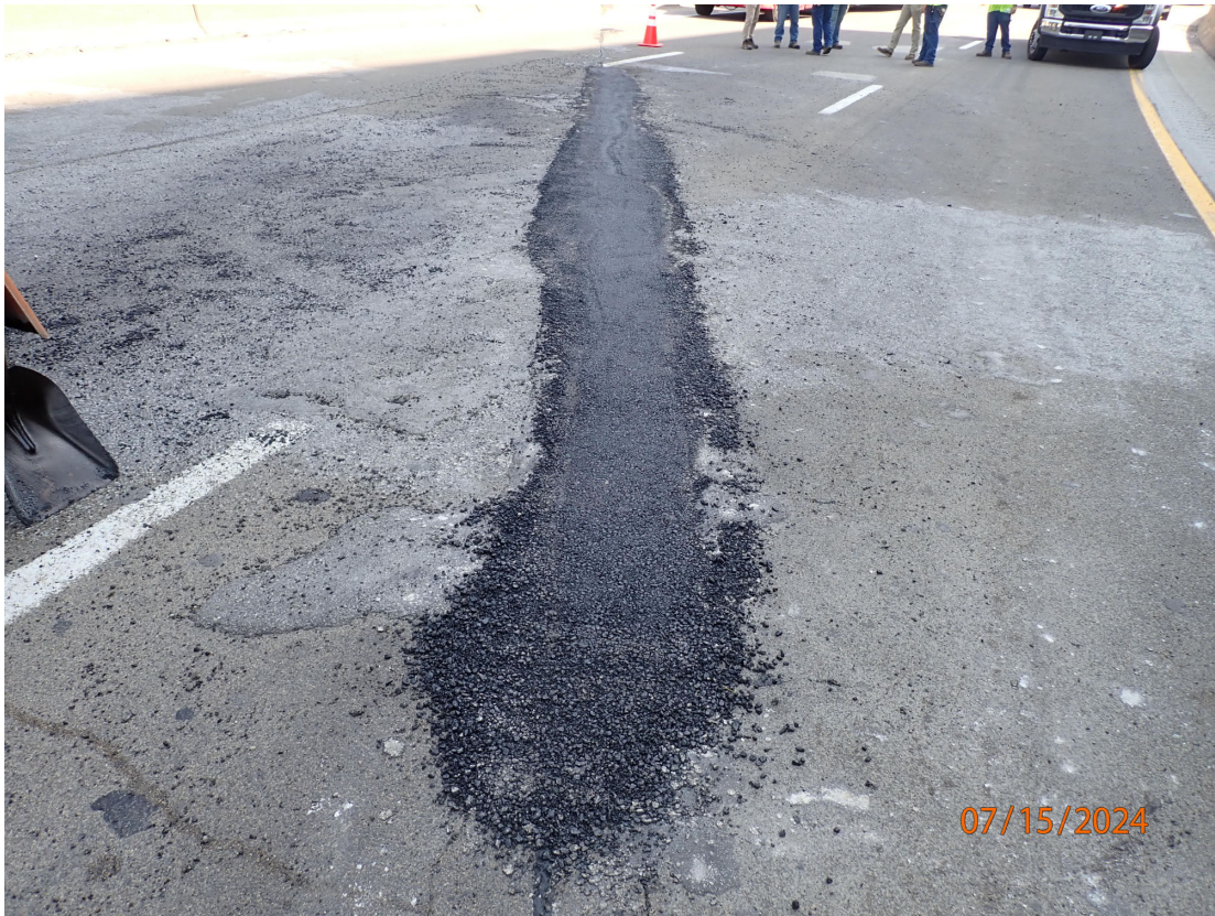
SB Lanes: Pourable Joint over Abutment 1 (after repair; looking west)
