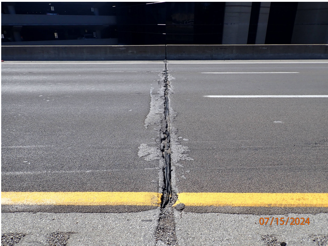
NB Lanes: Pourable Joint over Pier 4
