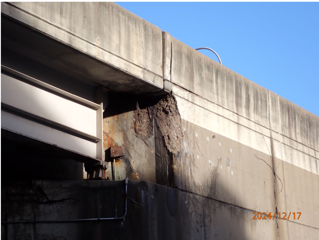
East end of Abutment 6 back wall has closely spaced diagonal cracking with rust staining plus a large spall with exposed rebar.
