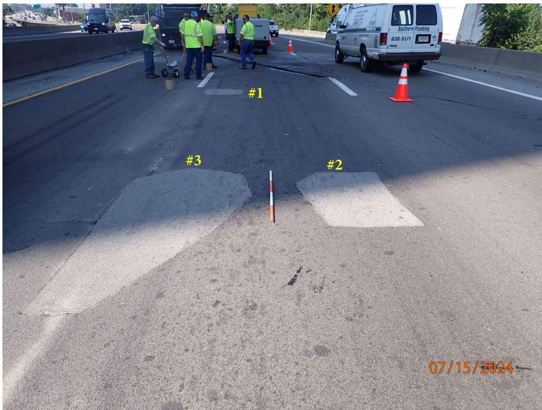
SB Lanes: Concrete Patches #1-3 in Span 1 (closer to A1 joint)
