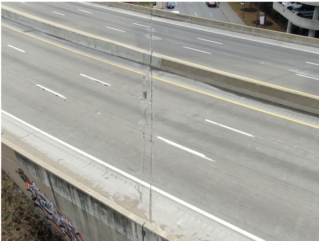
Joint over Abutment 6.
