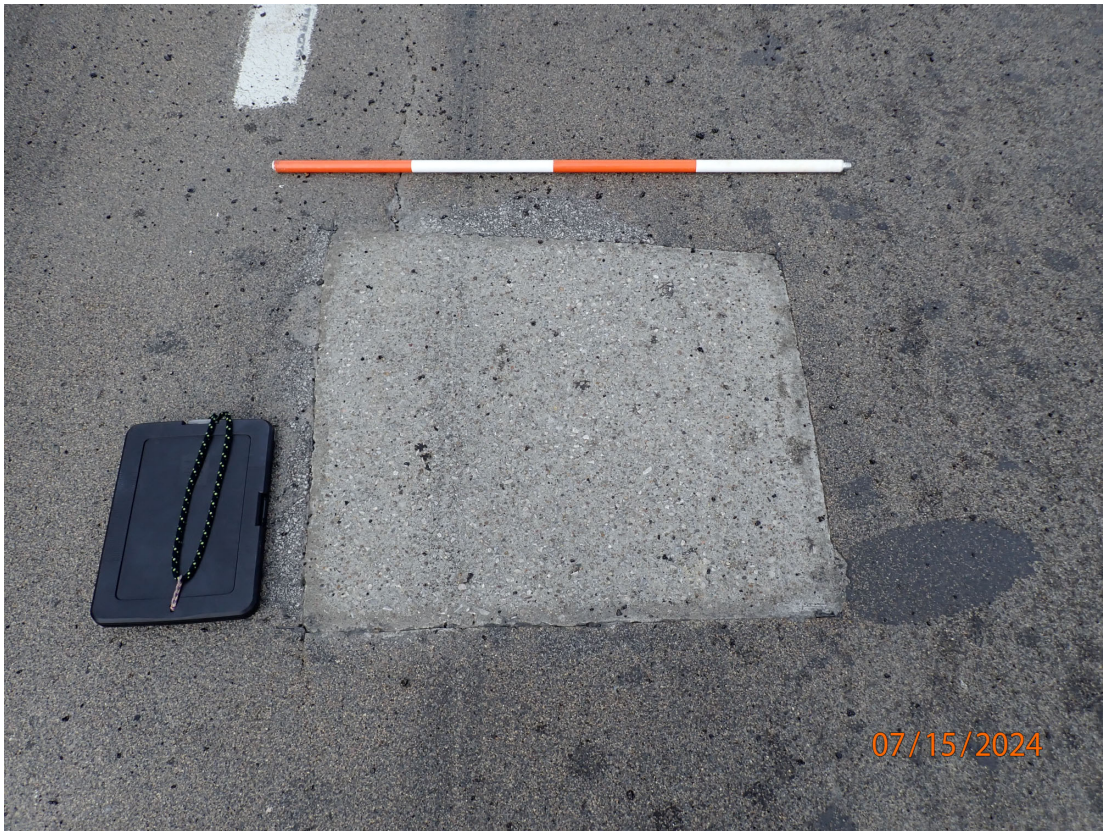
SB Lanes: Concrete Patch #1 = 3'L x 3'W = 9 SF
