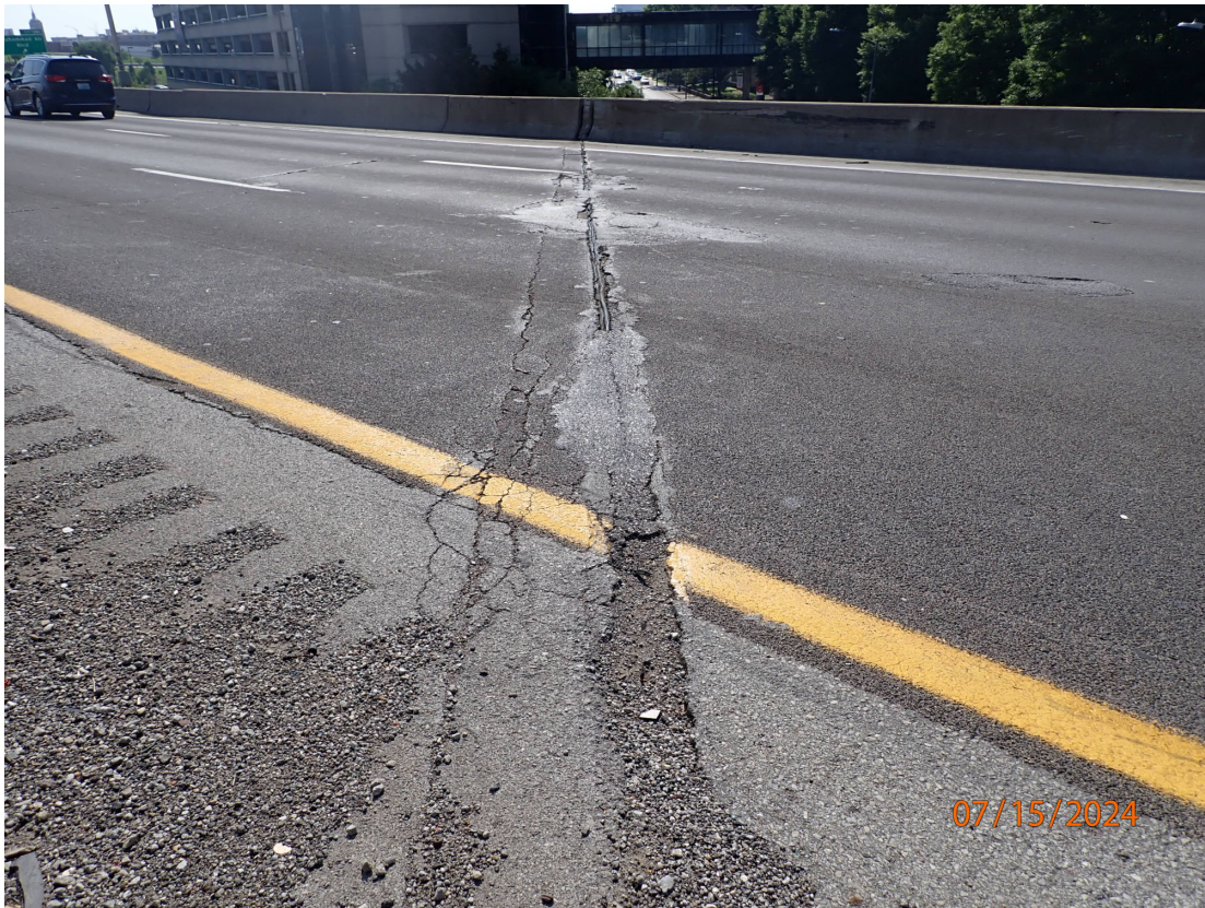
NB Lanes: Pourable Joint over Abutment 6
