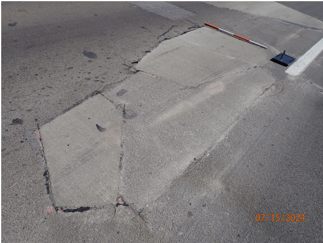
SB Lanes: Concrete Patch #4 = 12'L x 5'W = 60 SF
