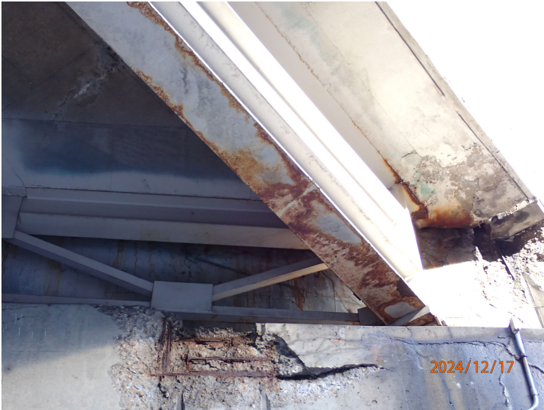
Spall with exposed rebar in Abutment 6 at Girder 14, plus corrosion along the bottom flange of Girder 14.
