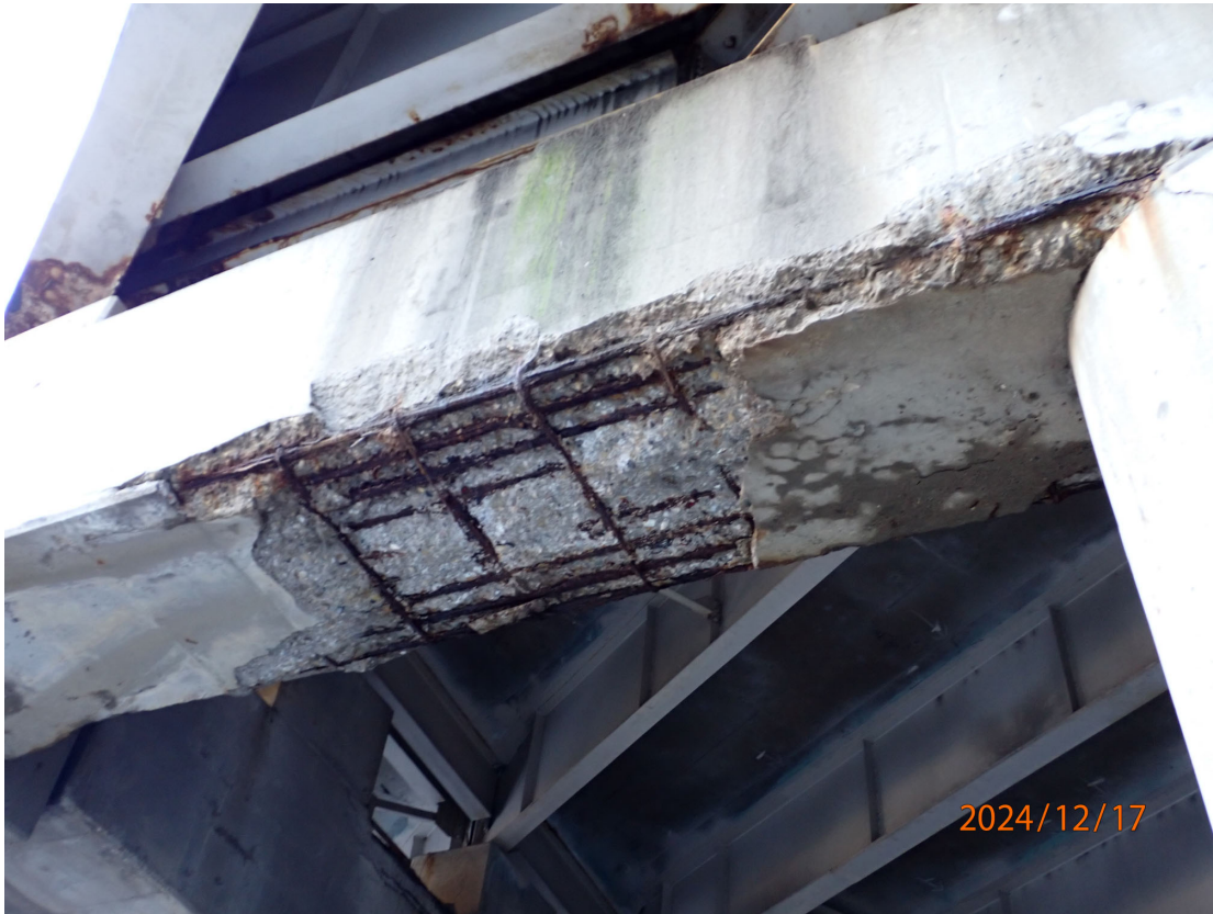
Pier 2 cap has wide cracking and/or large spalls with exposed rebar for much of the length. Largest spall on the bottom face between Columns 1 and 2 shown.
