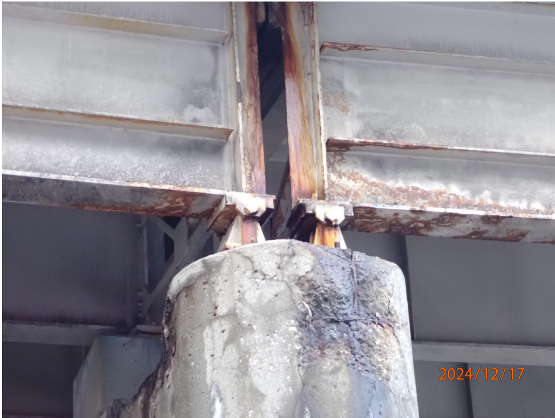
Girder 14 over Pier 4 has heavier corrosion along the girders and the bearings.
