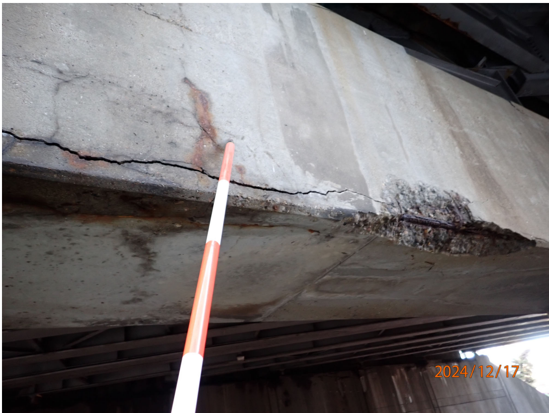
Wide horizontal cracking and spalling along the bottom north face in Pier 2 cap between Columns 10 and 11.
