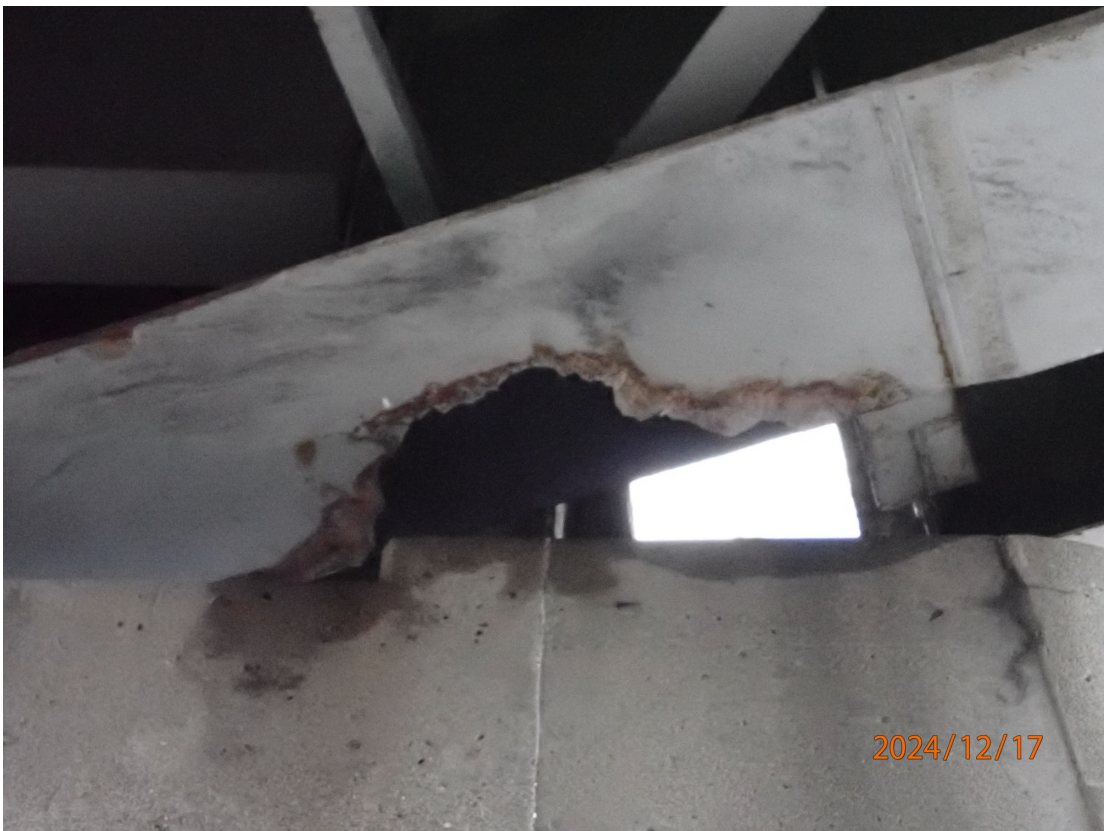
Another example of corrosion and peeling paint in Span 1-Pier 2-Girder 14.
