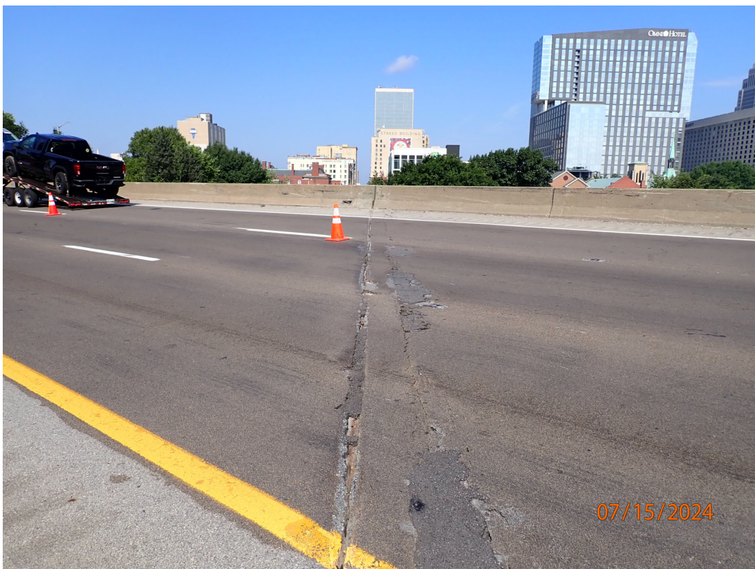
SB Lanes: Pourable Joint over Abutment 6
