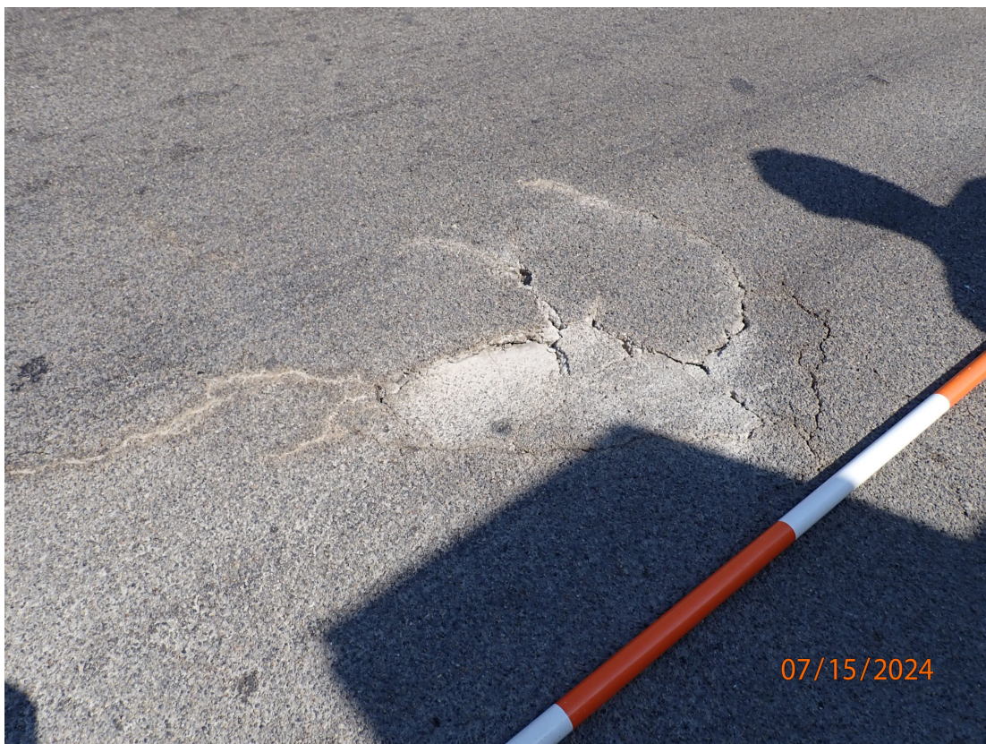
SB Lanes: Deck Spall in Span 1
