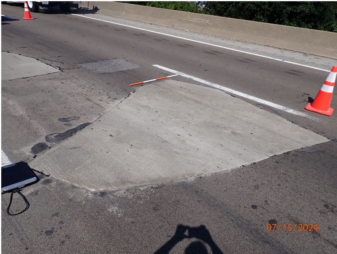
SB Lanes: Concrete Patch #6 = 9'L x 11'W = 99 SF
