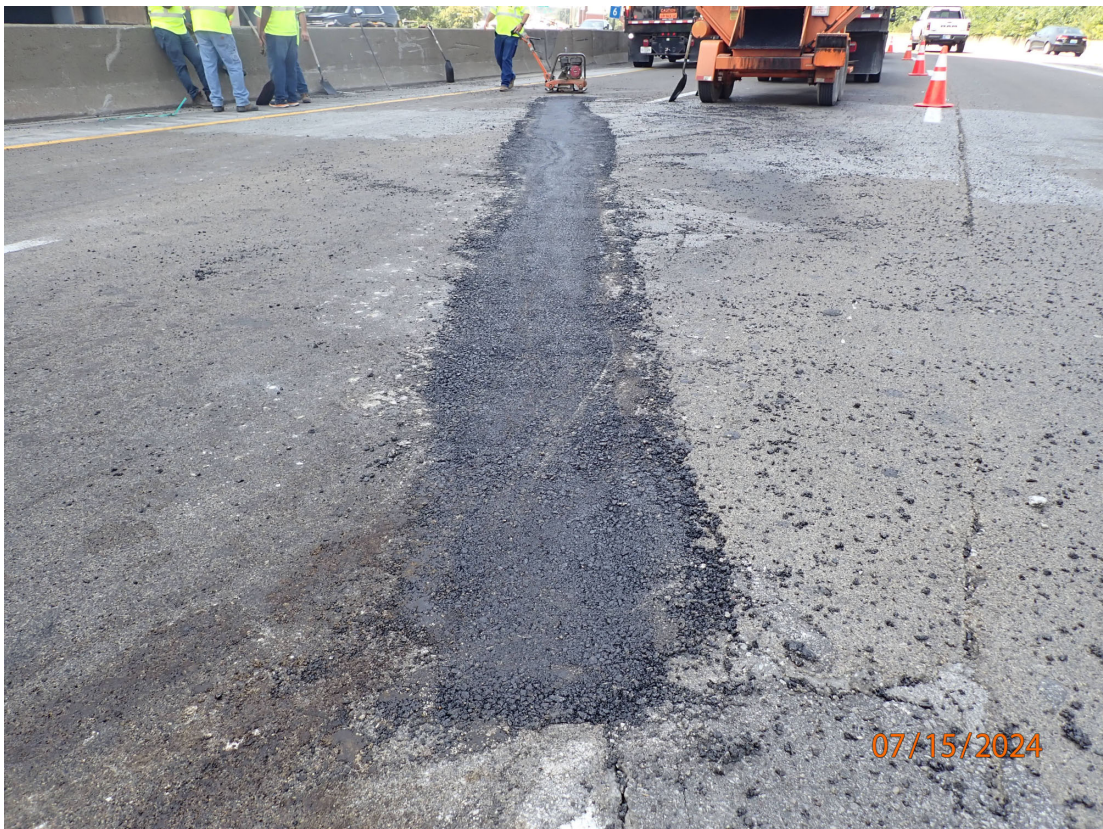
SB Lanes: Pourable Joint over Abutment 1 (after repair; looking east)
