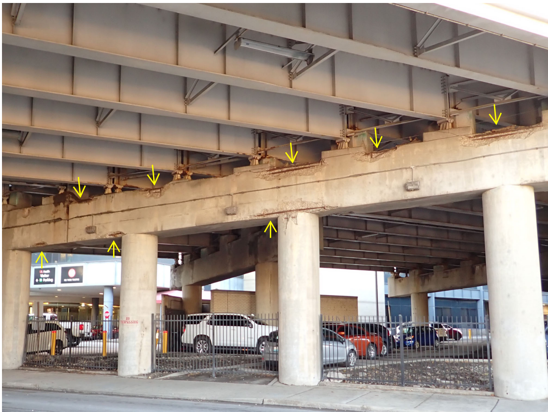
Numerous spalls with exposed rebar in Pier 5 north face between Columns 1 and 4.
