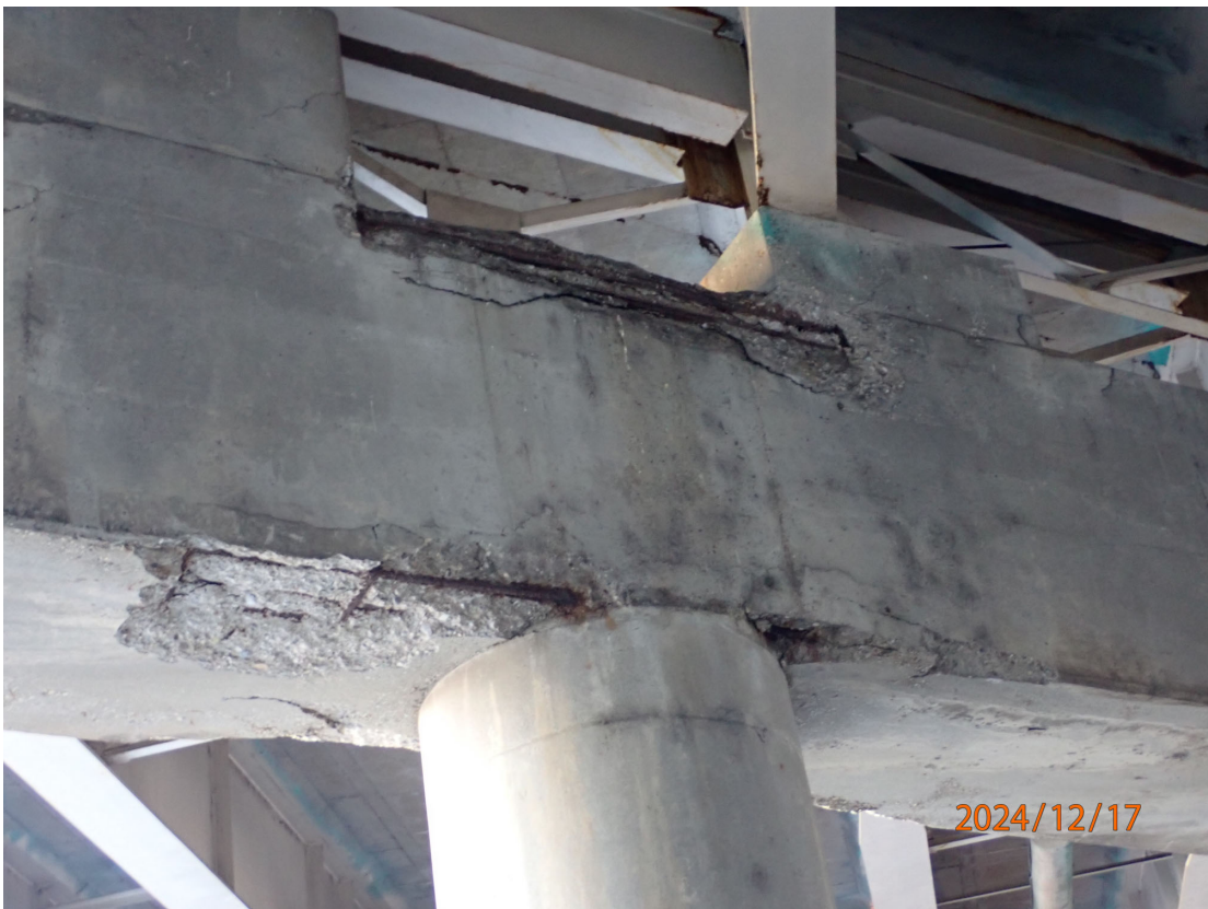
Pier 5 south face at Column 2 with spalling and exposed rebar.
