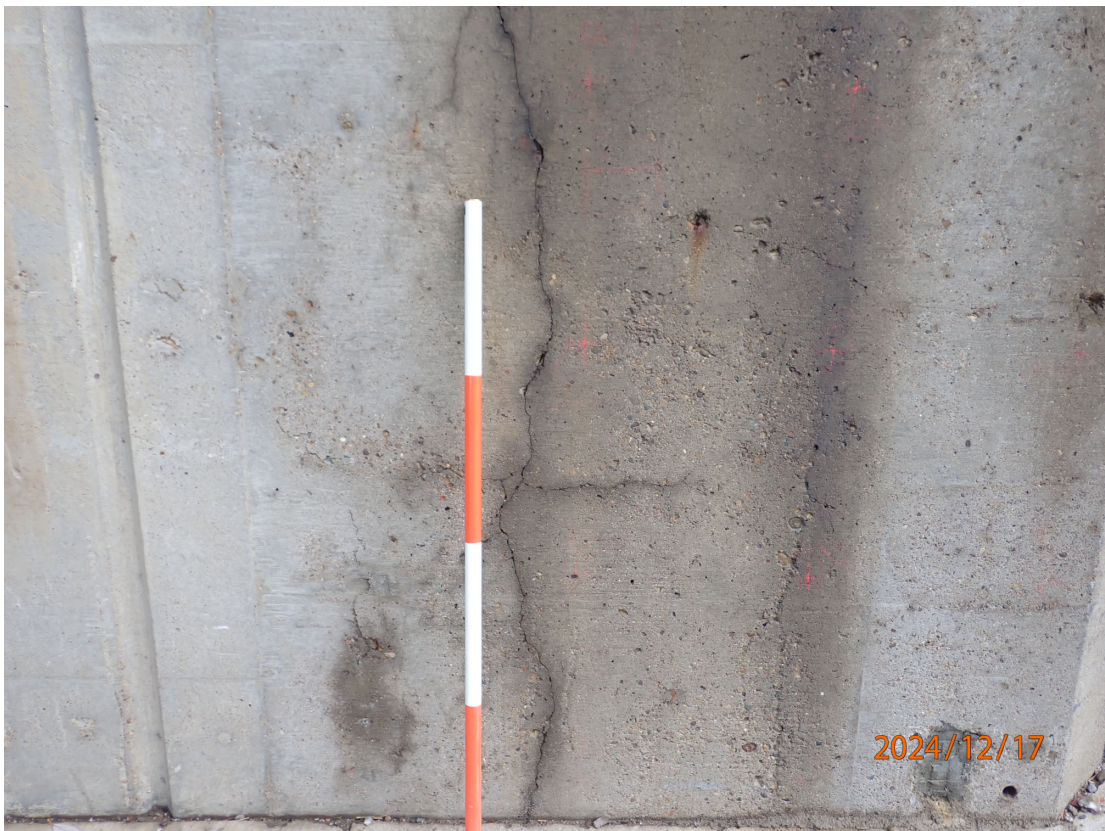
Abutment 6 has a few full height vertical cracks.
