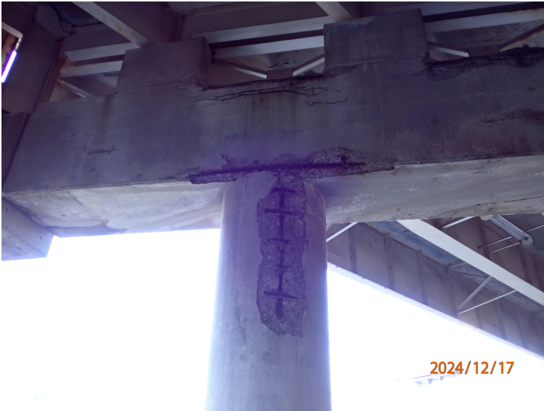
Pier 5 has wide cracking plus spalls with exposed rebar in the cap and several columns. Pier 5 south face at Column 1 shown.
