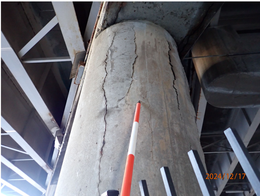
Several columns at Piers 2 and 5 have wide cracks and/or spalls with exposed rebar. Pier 2-Column 5 south face shown with closely spaced wide cracks.
