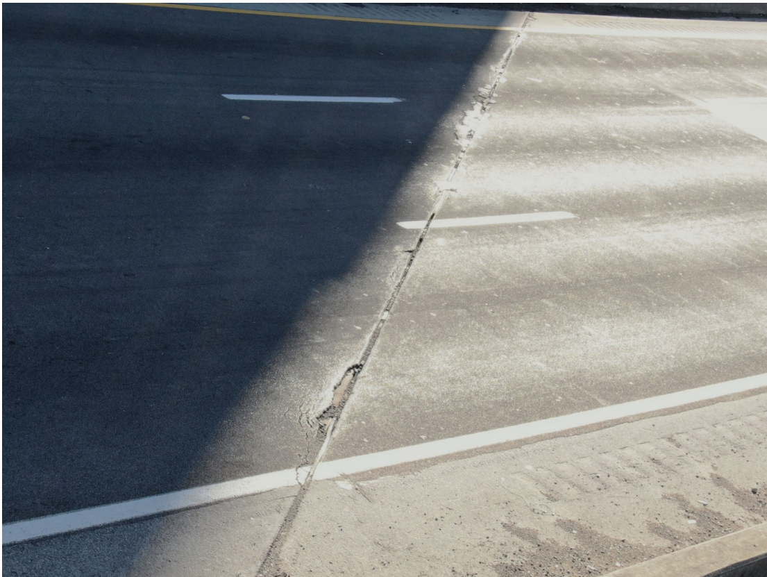
Close-up of joint over Pier 2 SB.
