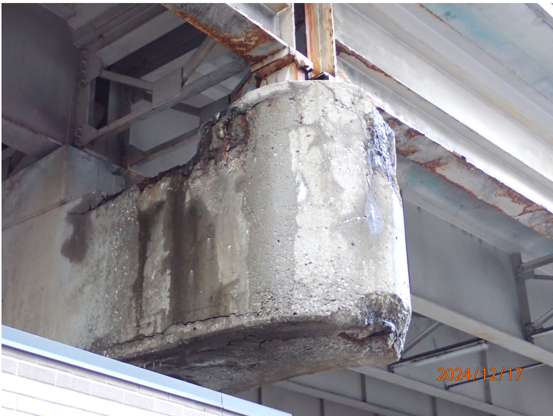
East end of Pier 4 has spalling with exposed rebar and wide cracking. South face shown.
