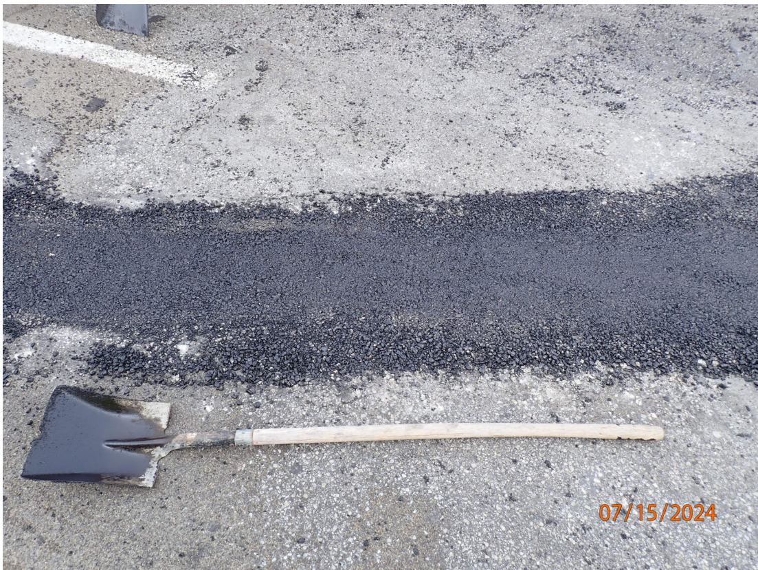
SB Lanes: Pourable Joint over Abutment 1 (after repair; closer view)
