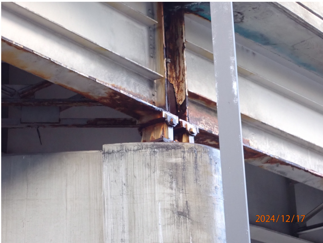
Girder 14 at Pier 5 as well as the bearings have heavy corrosion with section loss.
