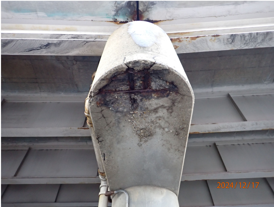
Spalling on the bottom face of Pier. 3 cap at the east end
