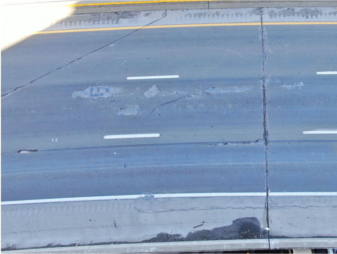
Span 2 and joint over Pier 3 Rosphalt overlay in Span 2 has several asphalt patches in the center NB lane. There is also spalling along the lane line between the center and right lanes.
