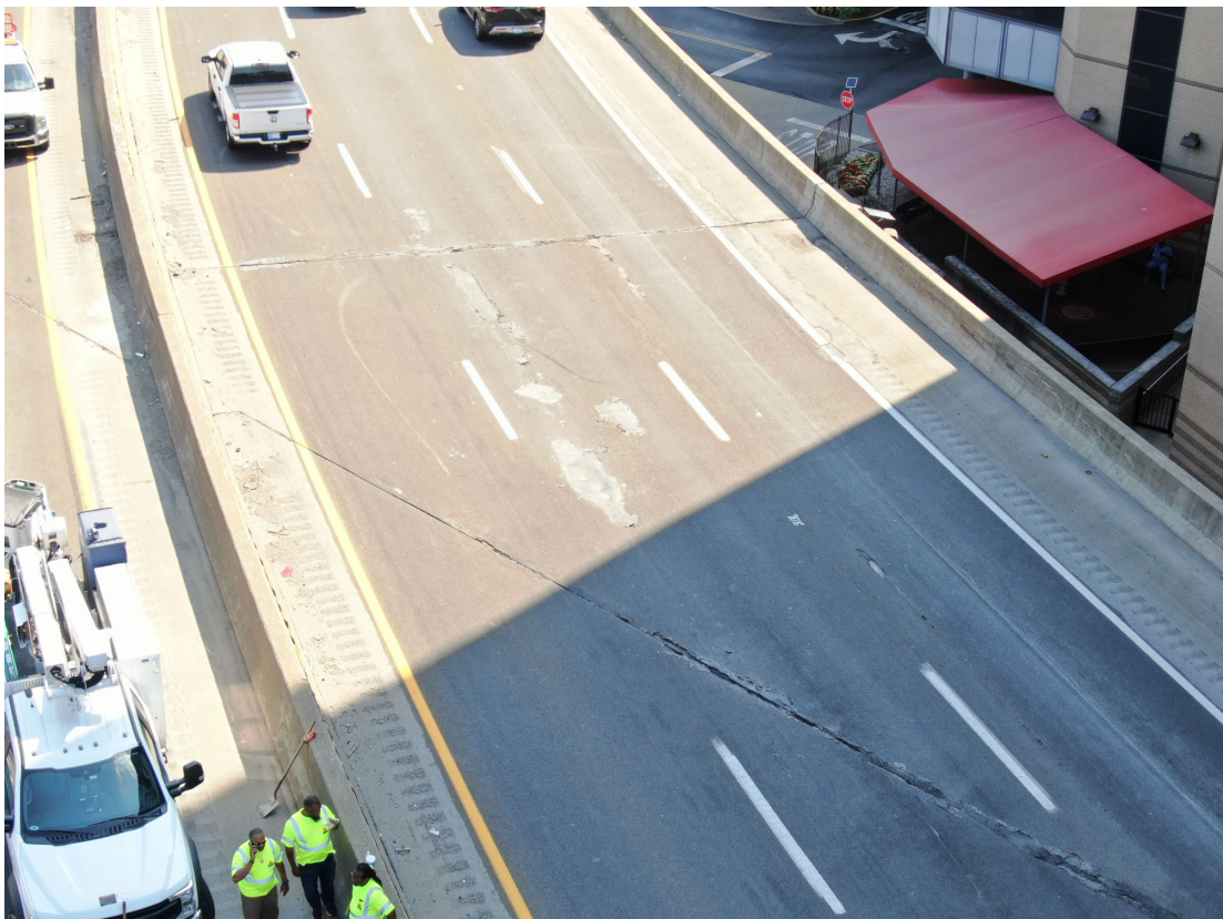
NB Lanes: Asphalt Patches in Span 2 (drone view)
