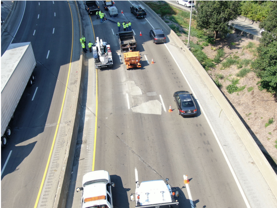
SB Lanes: Concrete Patches in Span 1 (drone view)
