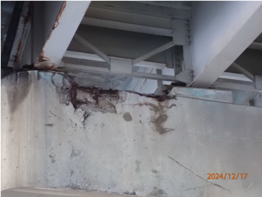
Pier 4 cap has spalls with exposed rebar. Example in the south face under Bay 8 shown.
