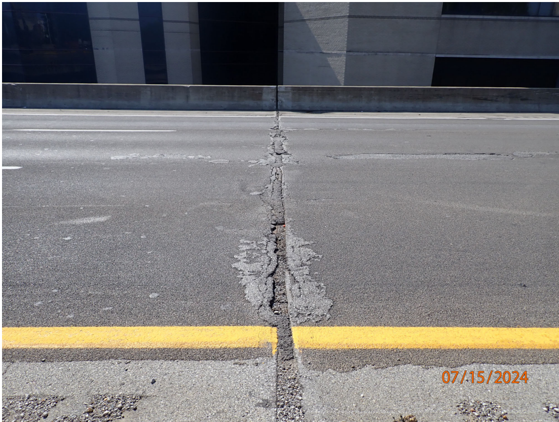
NB Lanes: Pourable Joint over Pier 3
