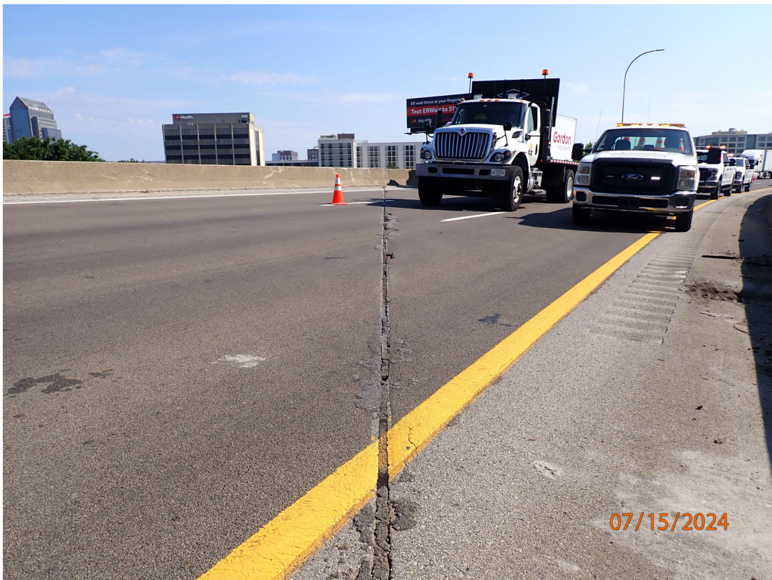
SB Lanes: Pourable Joint over Pier 2
