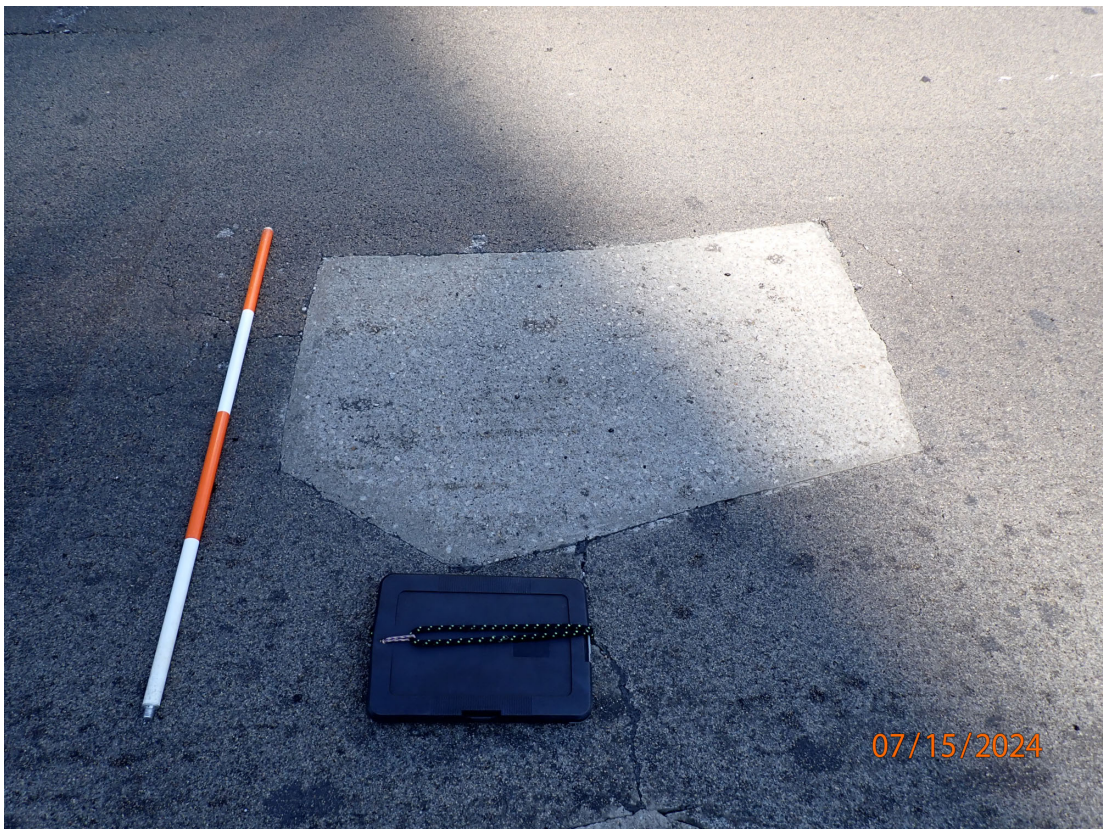
SB Lanes: Concrete Patch #2 = 4'L x 3'W = 12 SF
