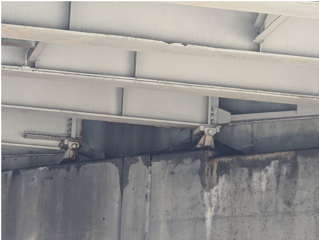
Abutment 6 Girders 7 and 8. Bearings have surface corrosion and are all slightly expanded, inconsistent with temperature. Girder 8 bearing is also partially buried in asphalt, restricting movement.
