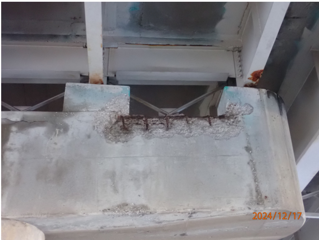
Spalling in the north face of Pier 4 cap under Bay 8.
