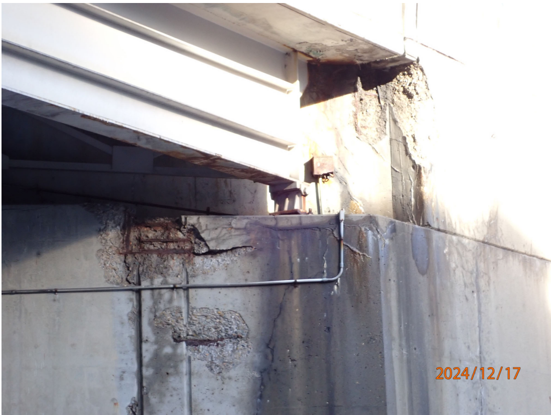
East end of Abutment 6 with cracking, spalling, and exposed rebar.
