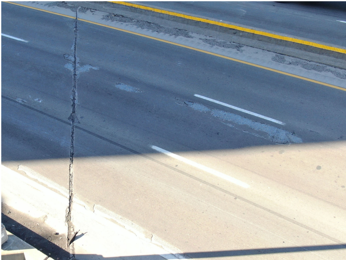
Close-up of failing joint over Pier 5 NB plus overlay patching in Span 6 NB.
