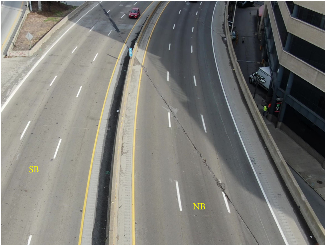
Joint over Abutment 1
