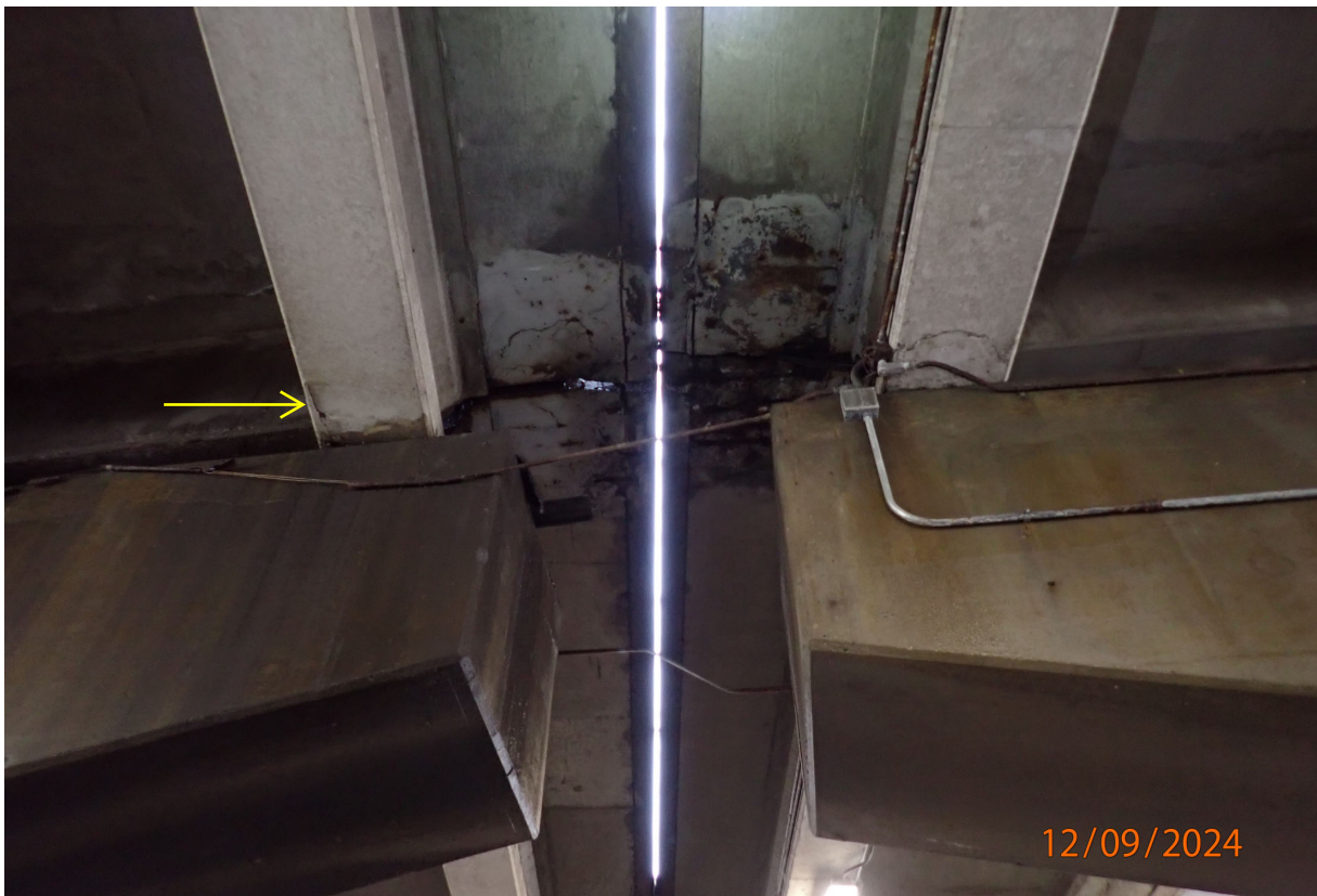
S3-B8 at P3 has a wide longitudinal crack. Note delamination in Beam 9 and deterioration of soffit below longitudinal joint.
