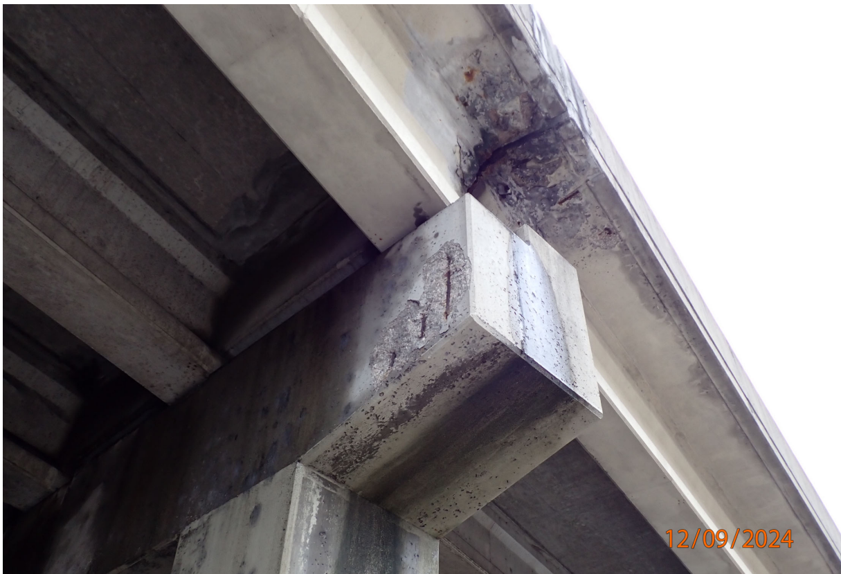
Delamination in S8-B1 top flange, and staining on overhang and pier
