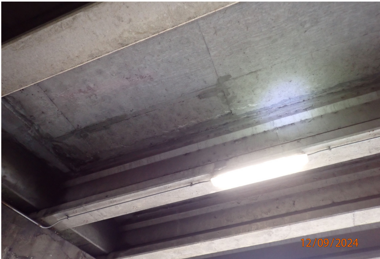
S4-Bay 3 soffit has 14 feet of longitudinal cracking with light efflorescence.
