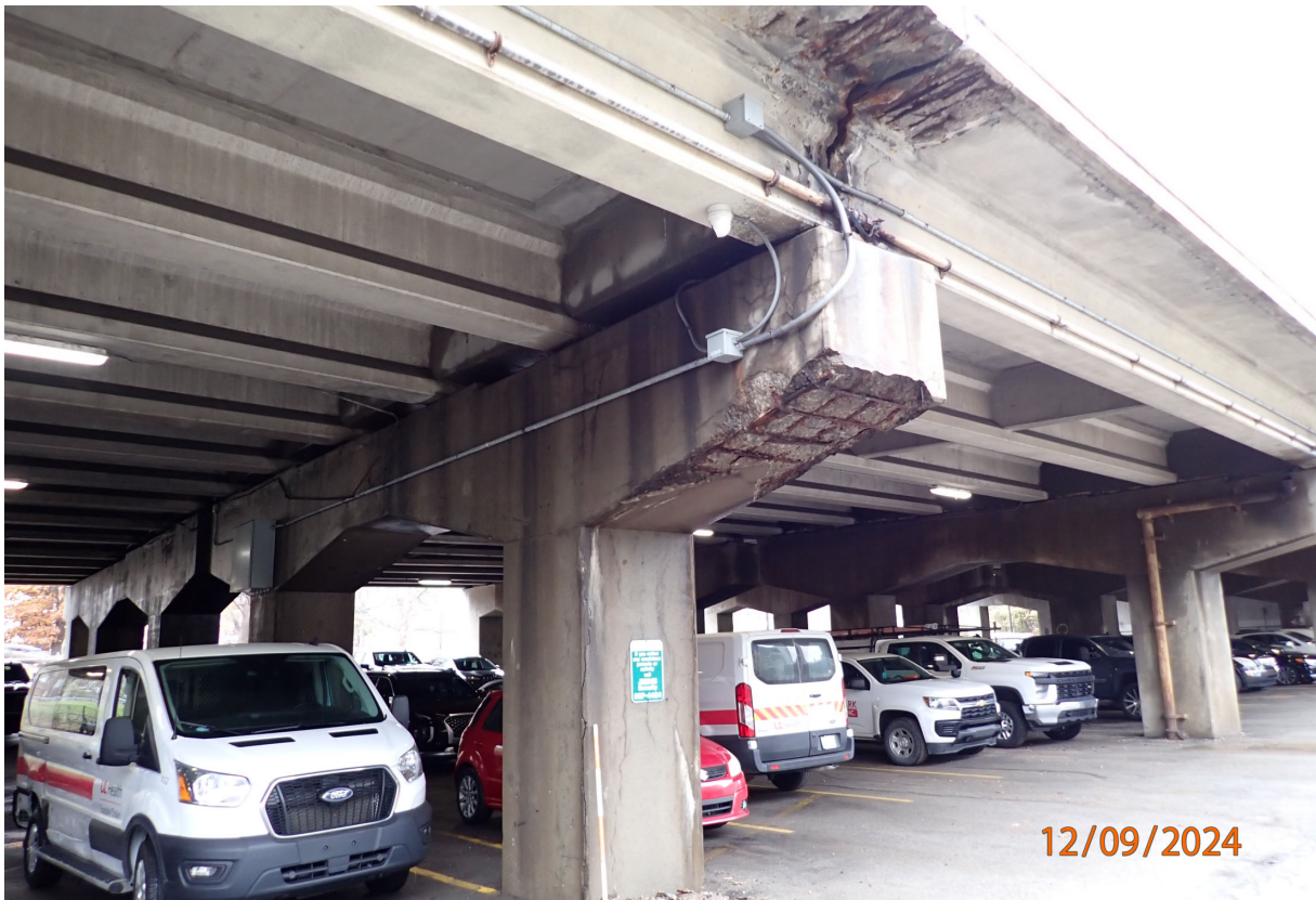
P3 and P7 caps have spalling up to 4 inches deep with fully exposed rebar in the bottom face at the east end (P3 shown).
