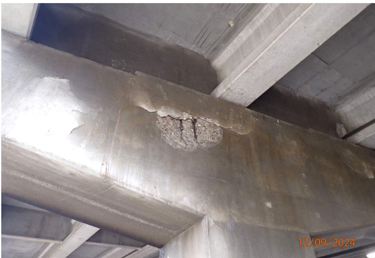
Pier caps have moderate to wide cracking, delaminated areas, and spalling with exposed rebar (P1 shown).
