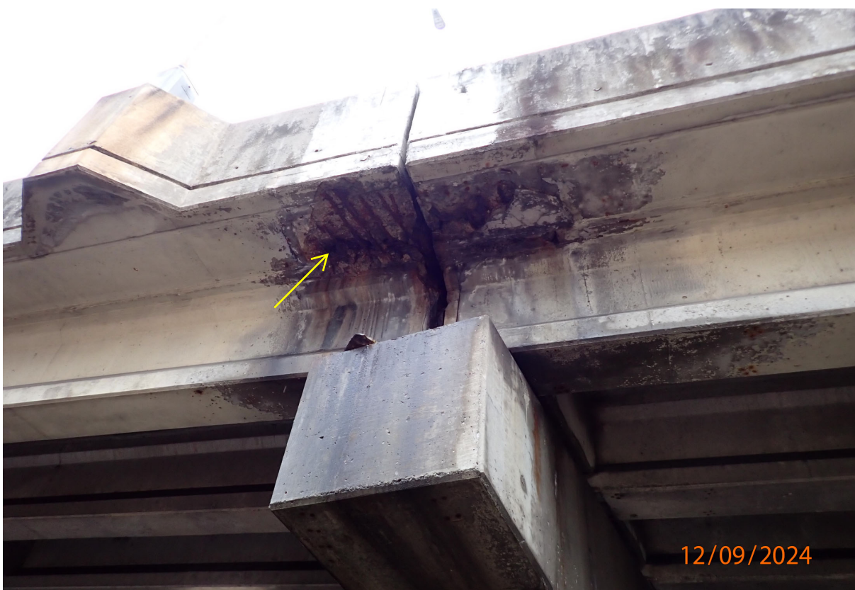
South face of P3 Note staining along the full length of the pier.
