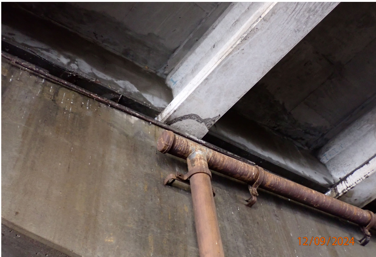
S7-B7 at P7 has a spall with three exposed prestressed strands (difficult to see due to spalled concrete sitting on cap).
