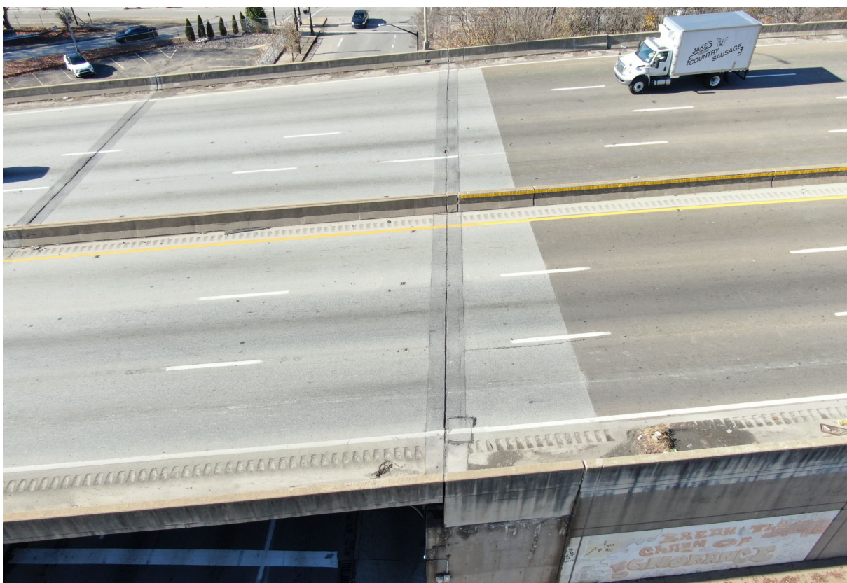
Asphalt plug joint over north abutment
