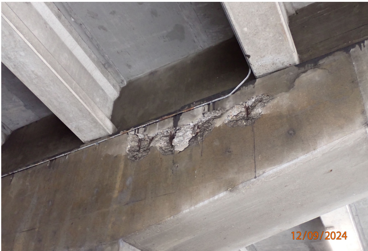
Pier caps have moderate to wide cracking, delaminated areas, and spalling with exposed rebar (north face of P6 between B3 and B4 shown).
