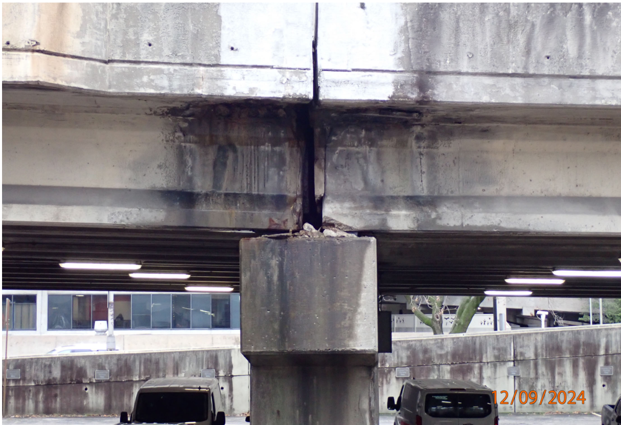
S3-B1 has a deep end spall with at least one exposed prestressed strand at P3W. Note staining on beams and pier.
