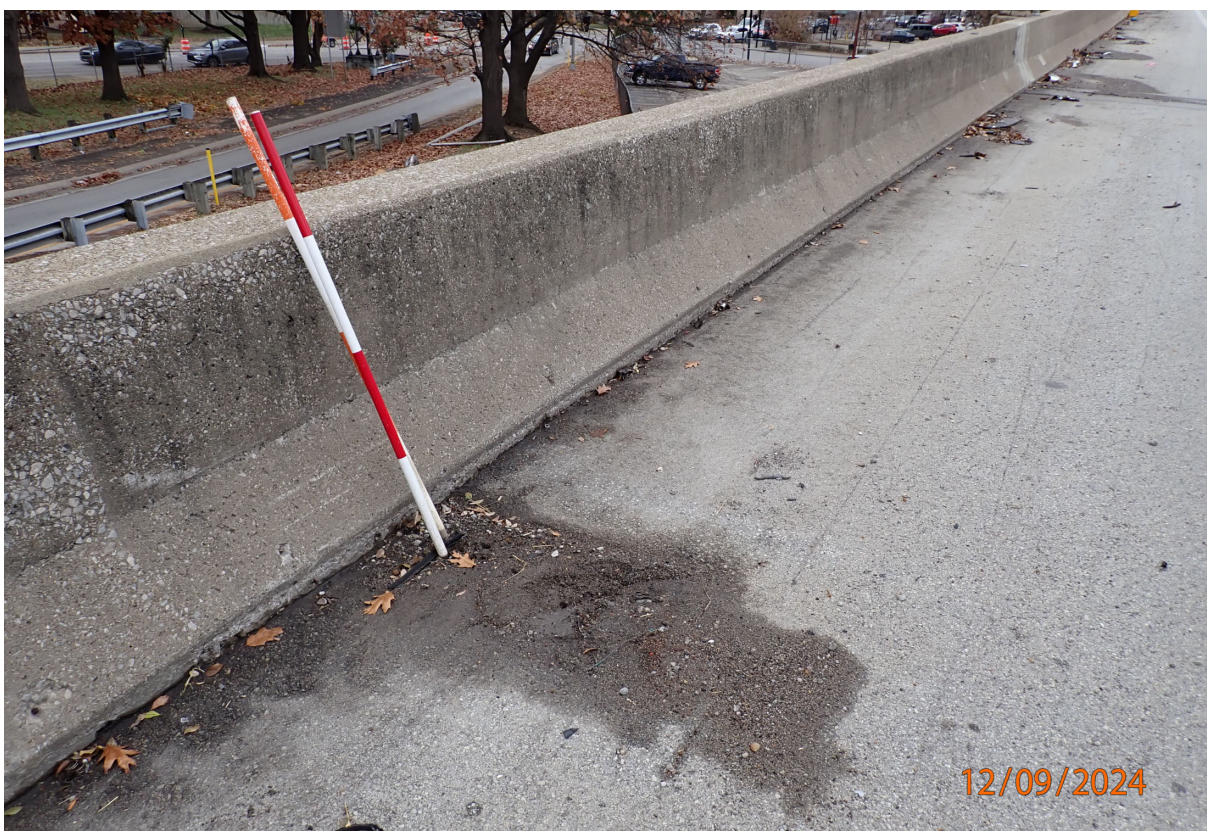
Deck drains are clogged (SB shoulder near south bridge end shown).
