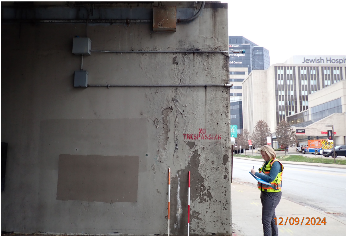
The north abutment has full height vertical cracks, some with efflorescence.
