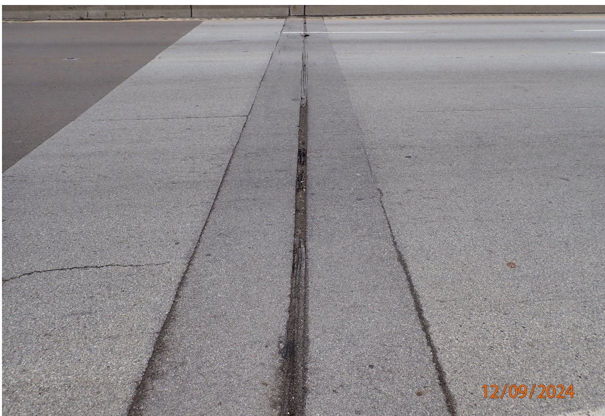
Asphalt plug joint over the north abutment (SB)
