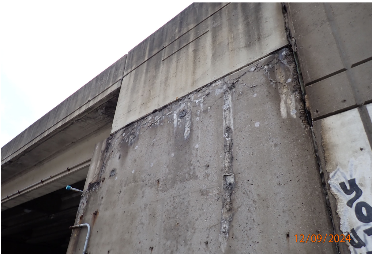
The northeast wingwall has heavy pattern cracking with efflorescence along the top for the full length, plus some spalling along the end joint.
