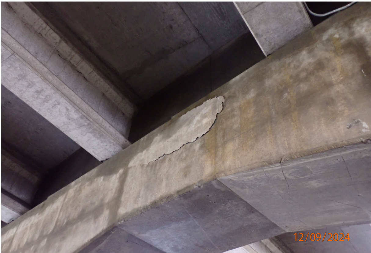
Pier caps have several delaminated areas (south face of P102 shown).
