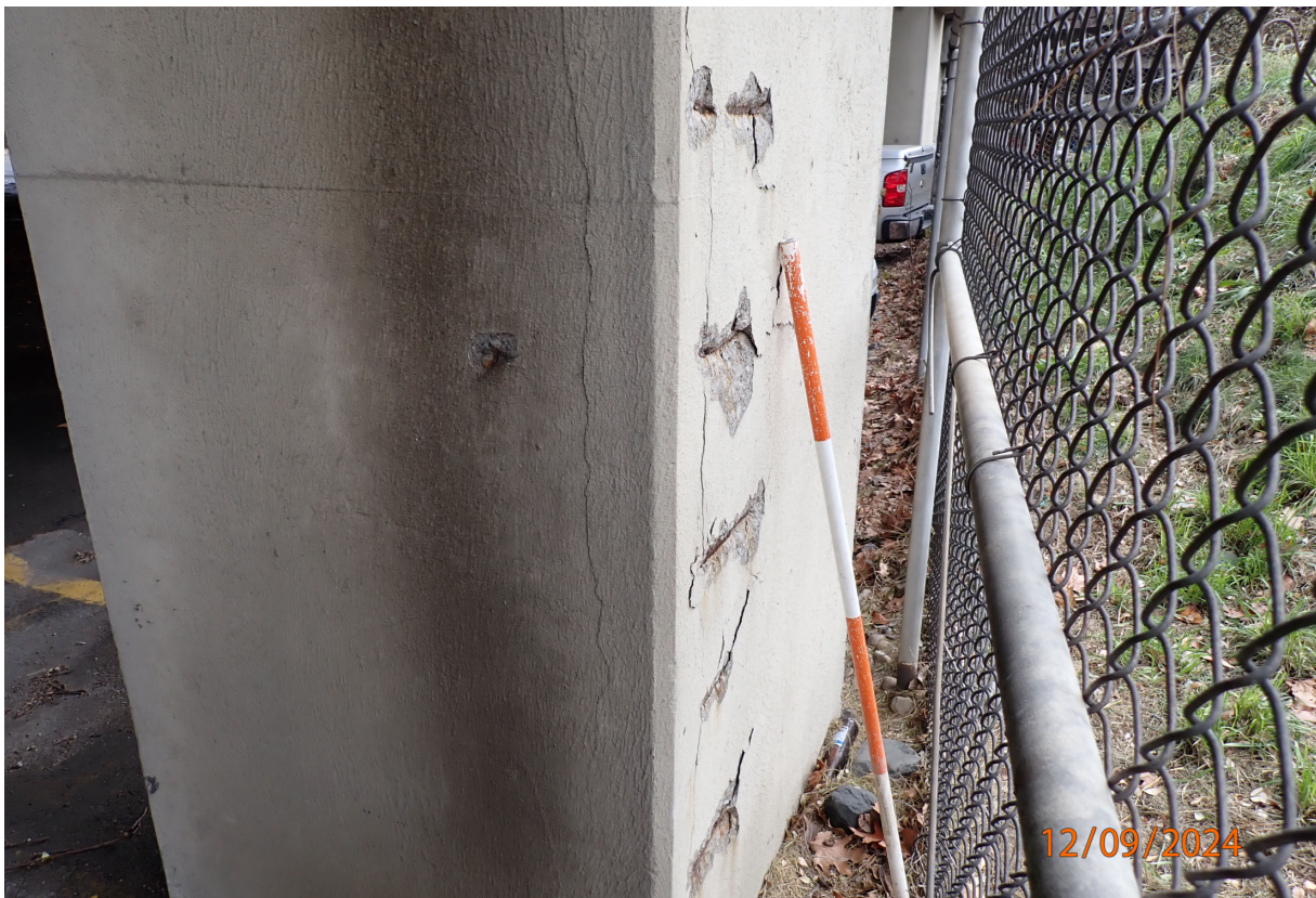
P2-C1 has several 1 SF spalls with exposed rebar in the west face.
