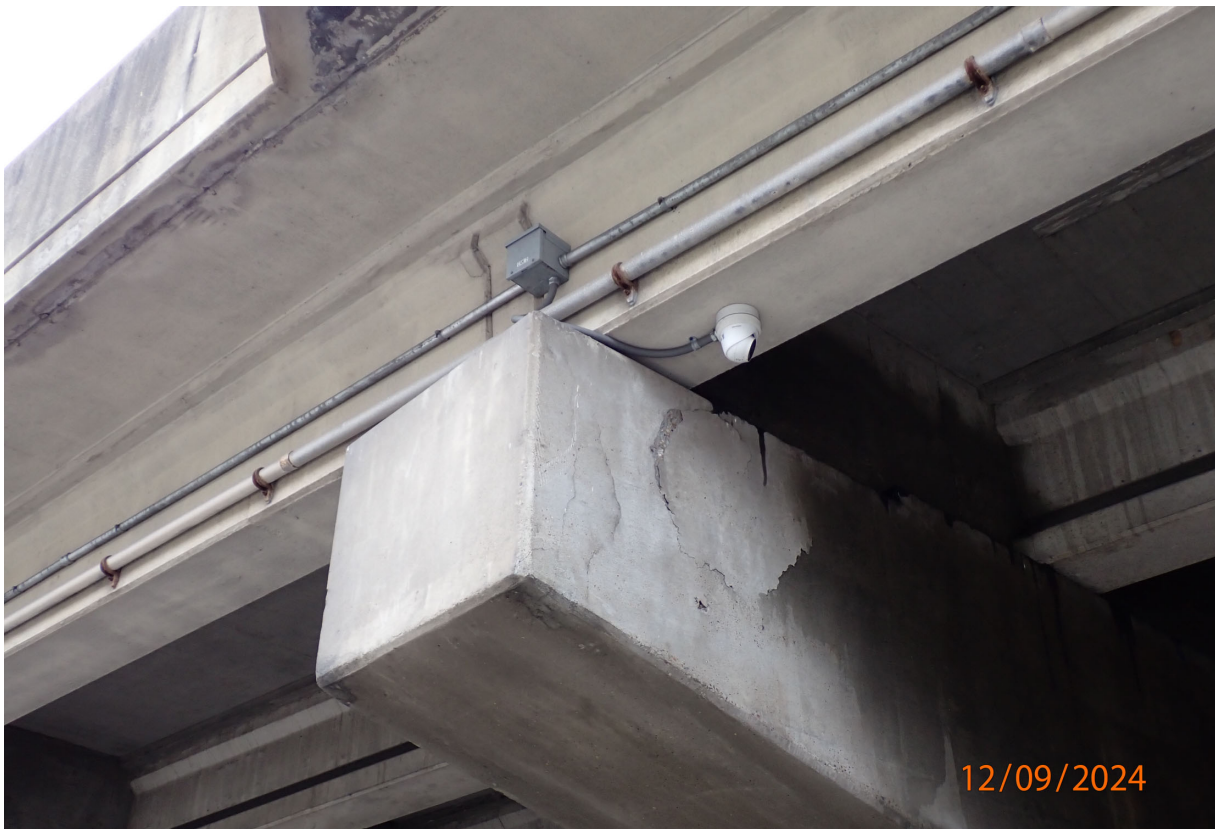
Pier caps have moderate to wide cracking, delaminated areas, and spalling with exposed rebar (north face of P5 shown).
