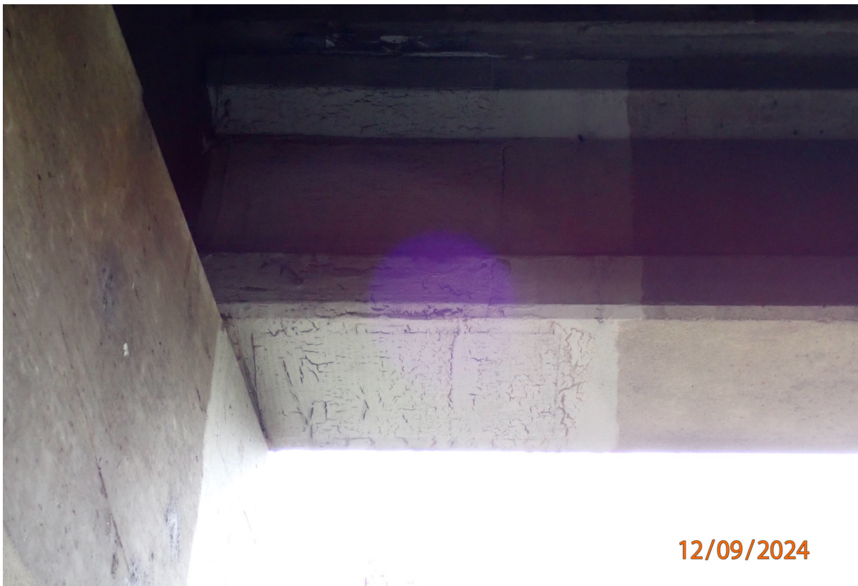
CFRP patch on S2-B1 at P1 has insignificant shrinkage cracking.
