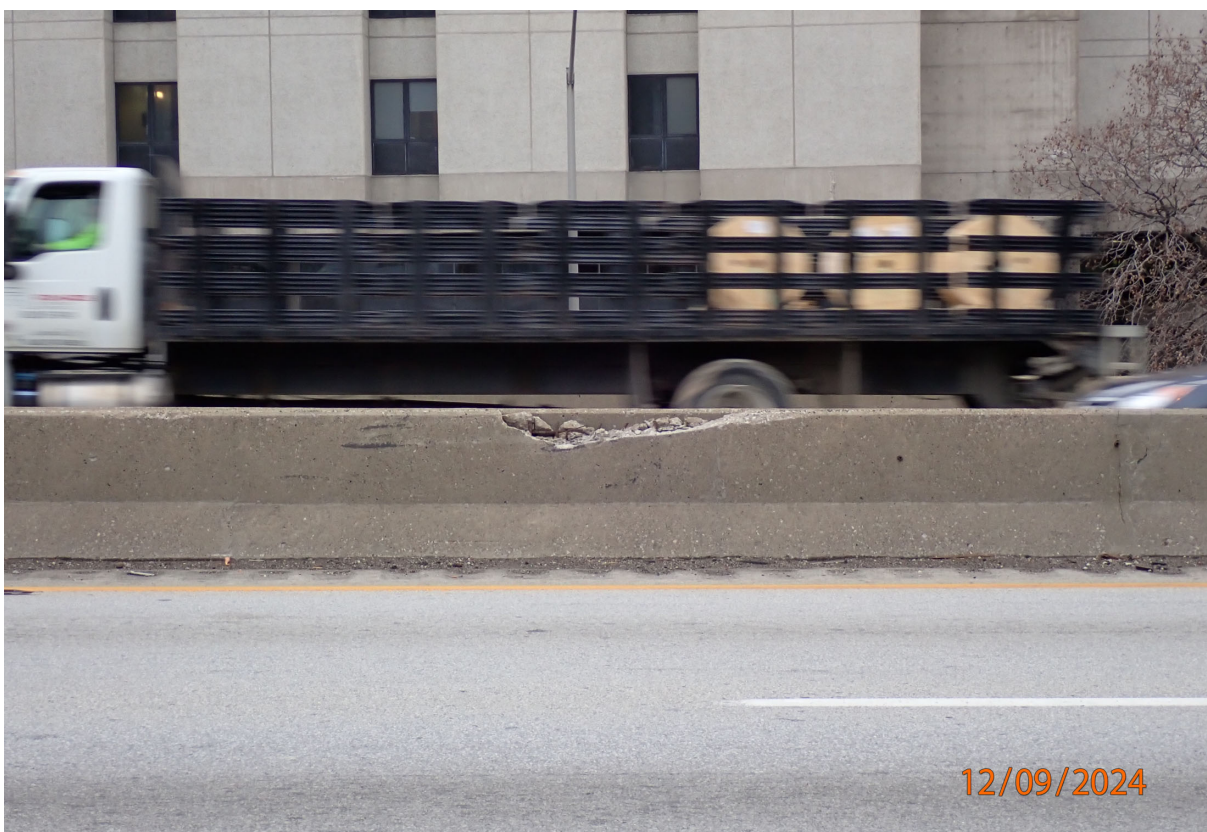
The SB median barrier has a 6-foot-long full depth spall with exposed rebar just north of Pier 3W joint.
