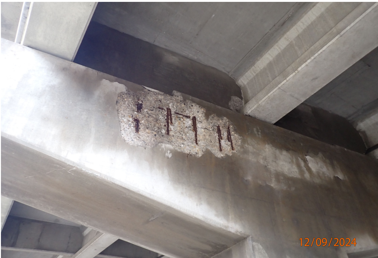
Pier caps have moderate to wide cracking, delaminated areas, and spalling with exposed rebar (north face of P2E shown).
