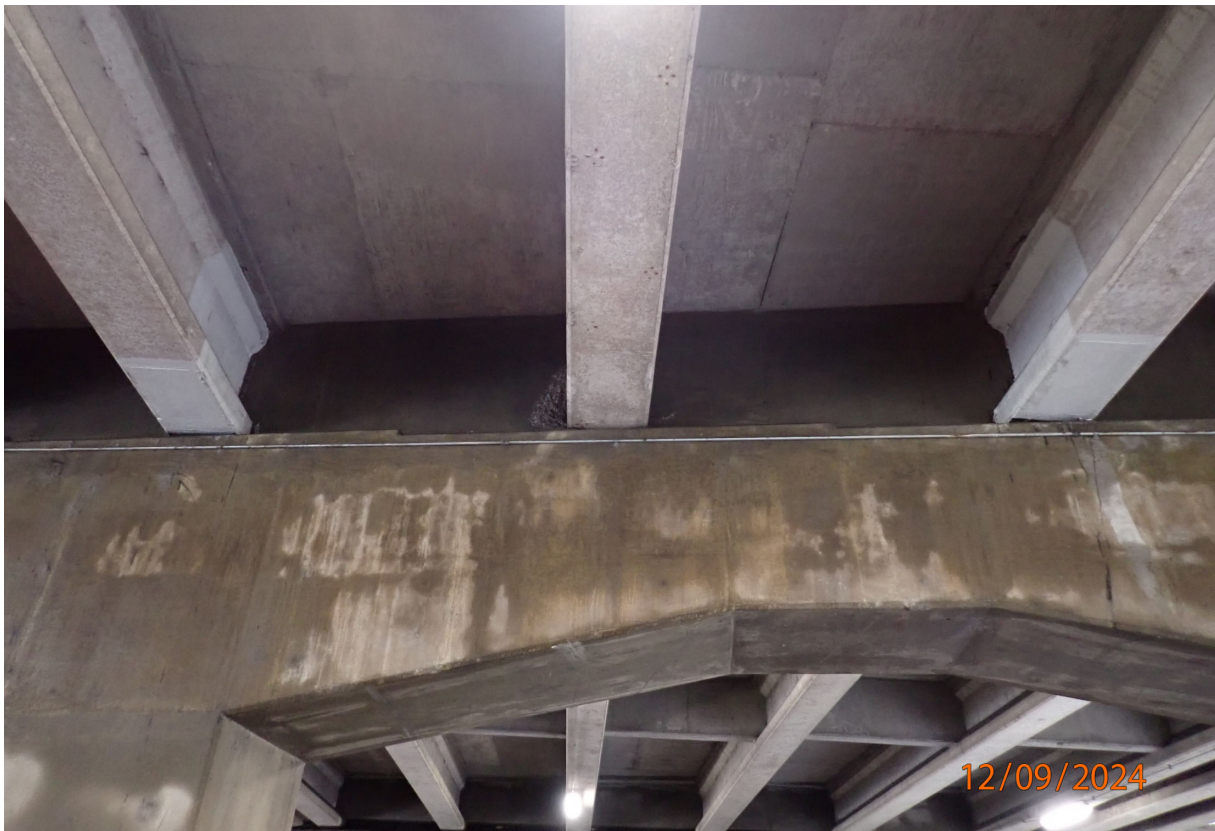
Some beam ends have CFRP patches (S1-B5 and B7 at P102 shown).
