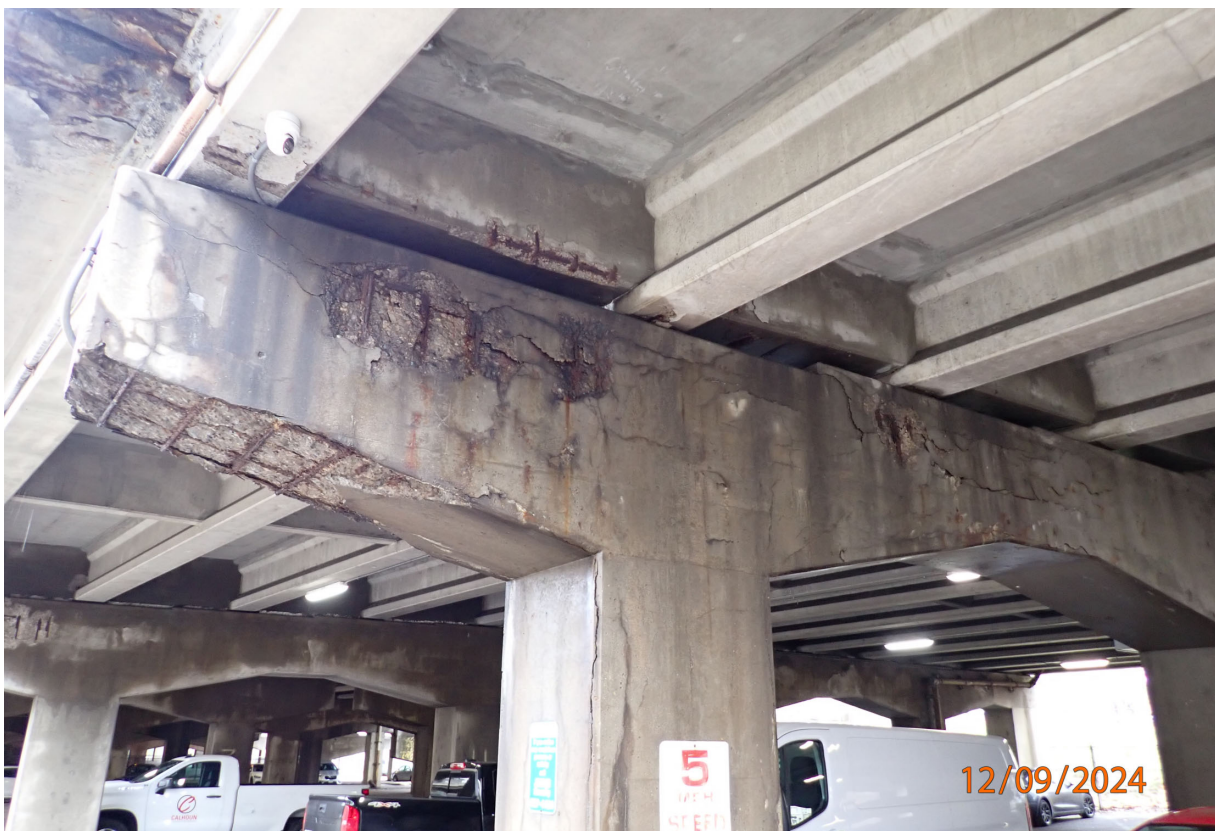
Additional view of east end of P3, north face. Note diaphragm spall with exposed rebar.
