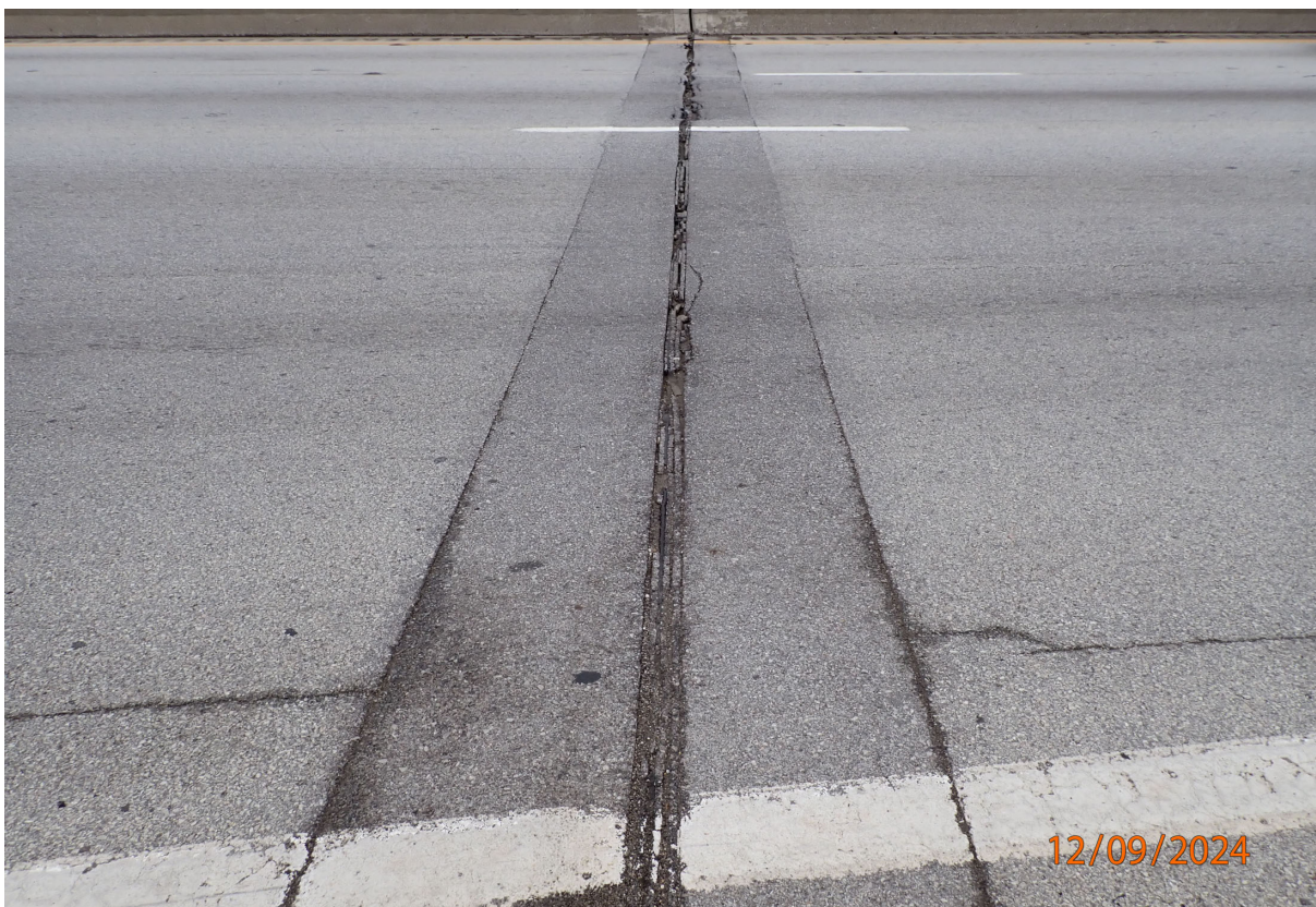
Asphalt plug joint over Pier 7W
