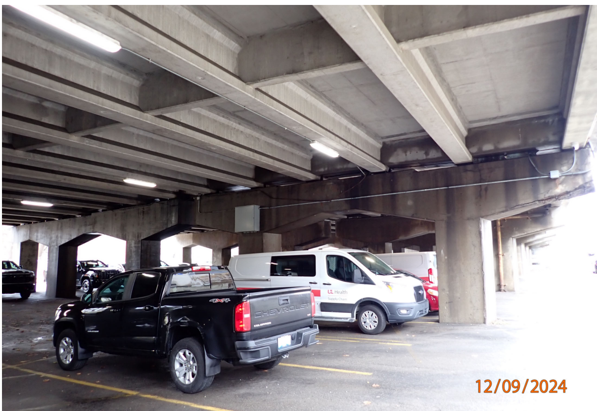
South face of P3 Note staining along the full length of the pier.
