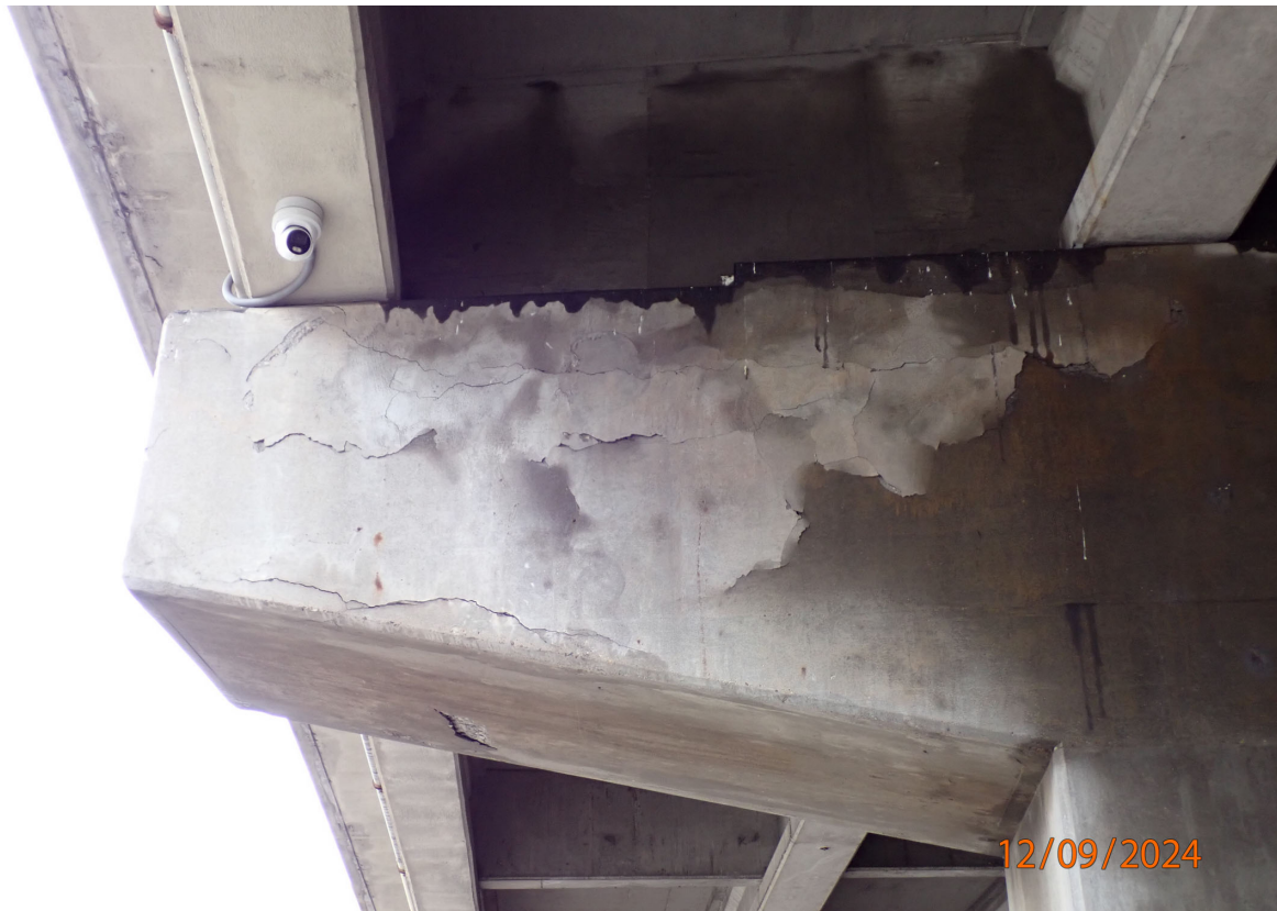
Large delaminated area with map cracking on the north face of P6 at the east end
