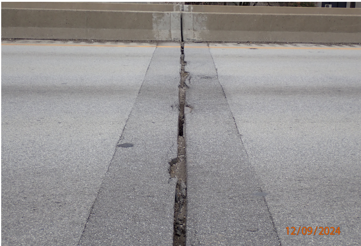
Asphalt plug joints have failed in the traffic lanes, with some spalling and rutting (close up).
