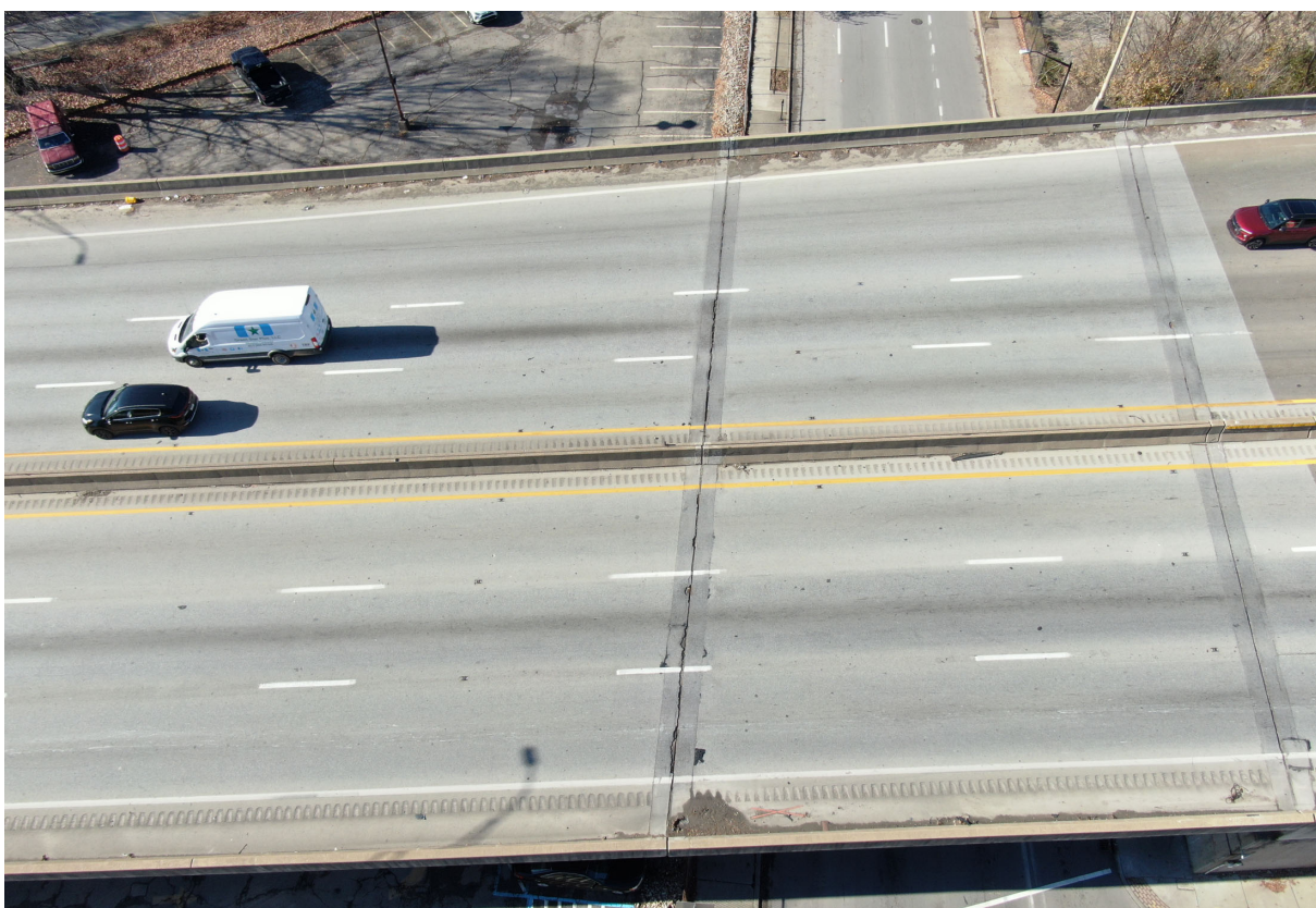
Asphalt plug joint over Pier 7
