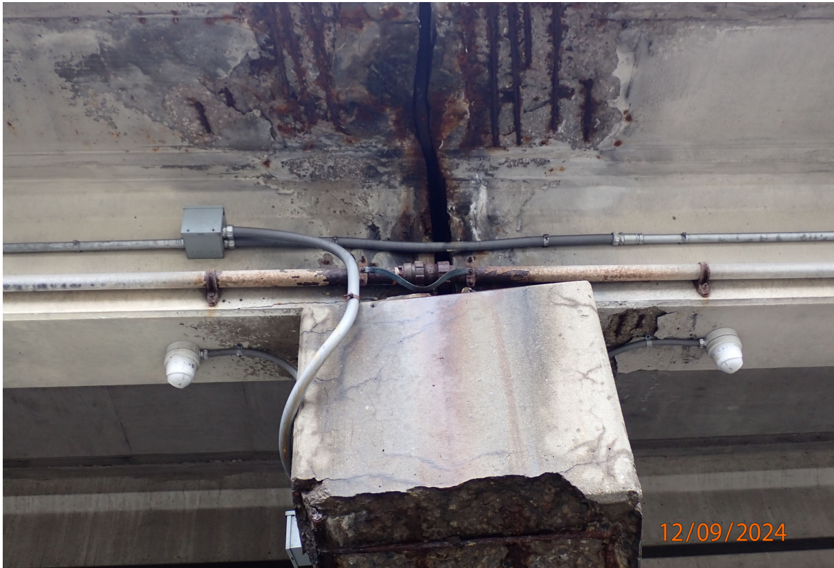
At P3, B14 has wide cracking and spalling, roughly 3 feet long at both beam ends. Note typical overhang spalling below joint.
