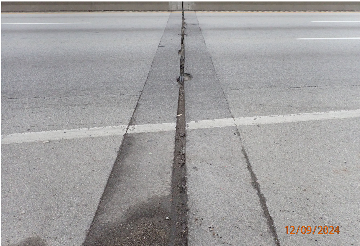
Asphalt plug joint over Pier 3W
