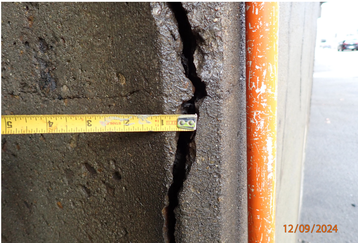
Column cracking is up to 1/2 inch wide (P3-C5 shown).
