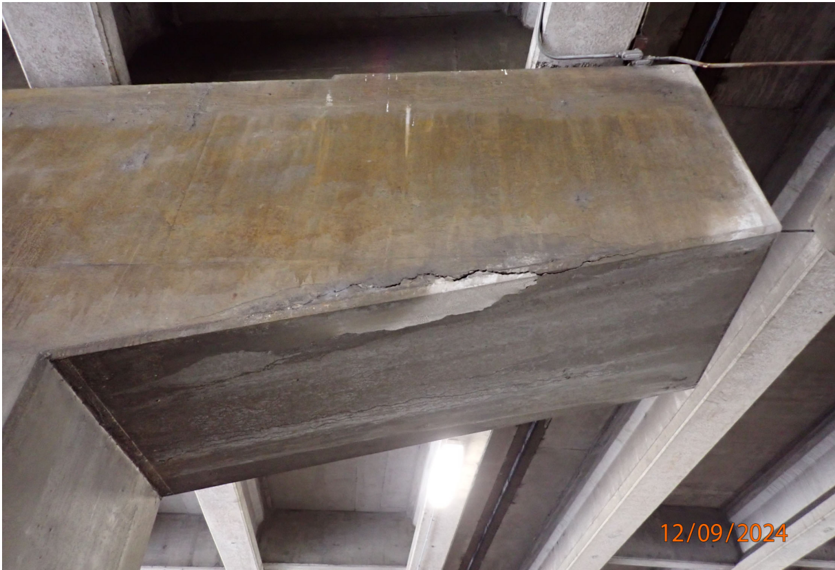
Pier caps have moderate to wide cracking, delaminated areas, and spalling with exposed rebar (south face of P2W shown).
