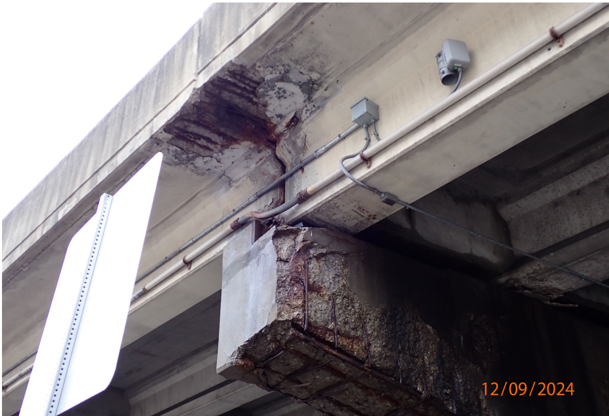
P7 cap spalling is encroaching on S8-B14 bearing area. B14 has a spall with one exposed strand.
