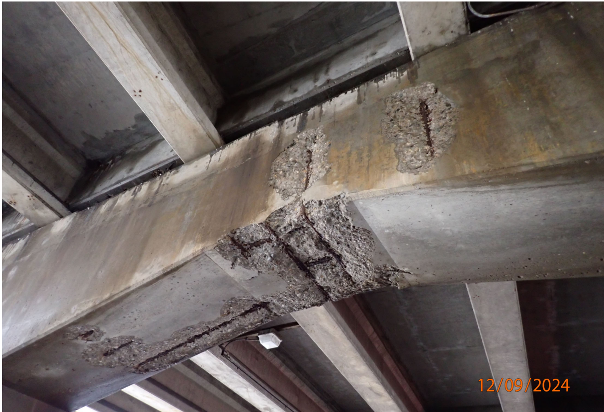
Deterioration is widespread on P3 and P7 (between C1 and C2 shown) below the joints.
