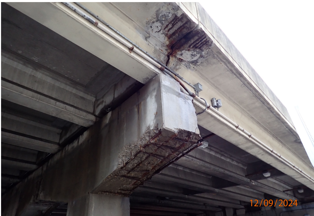
P3 and P7 caps have spalling up to 4 inches deep with fully exposed rebar in the bottom face at the east end (P7 shown). Note typical overhang spall at joint.
