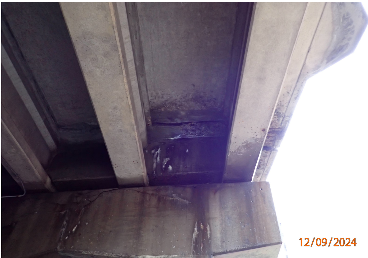
Soffit has a 10 SF area of full depth deterioration in S4-Bay 1 at P3W.
