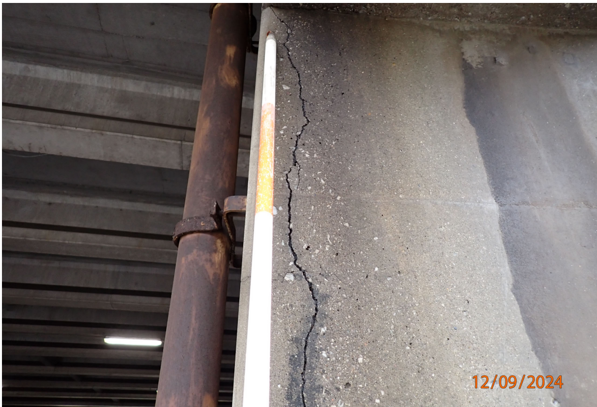
Some columns have wide vertical cracks (P102-C5 shown).
