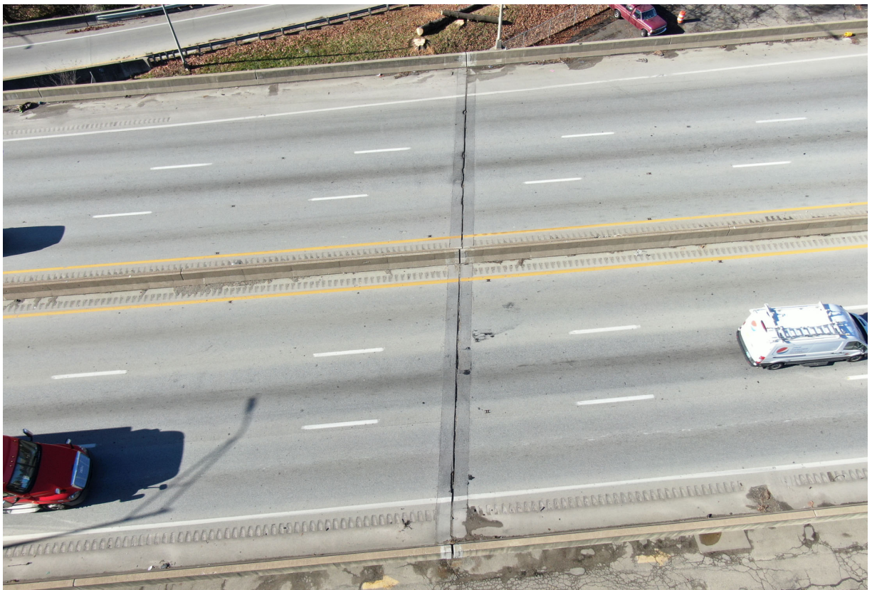
Asphalt plug joint over Pier 3
