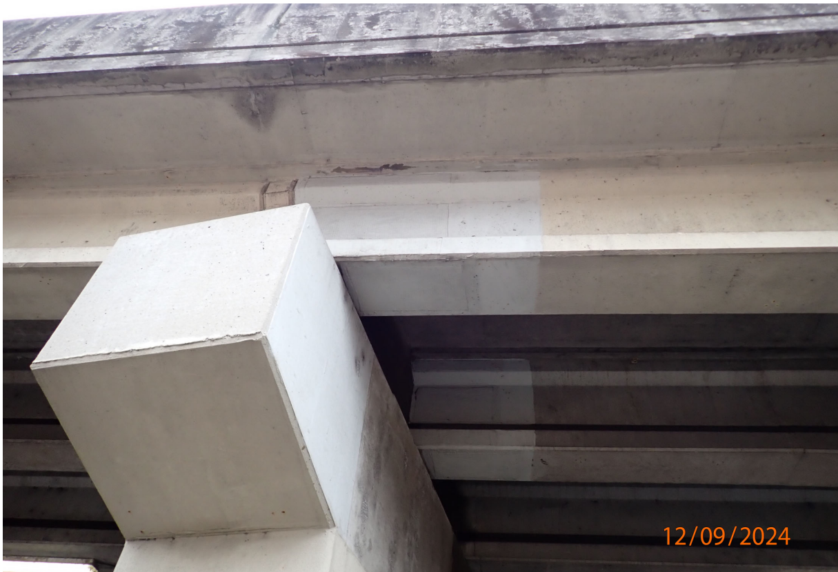
Some beam ends have CFRP patches (S4-B1 and B2 at P4 shown).
