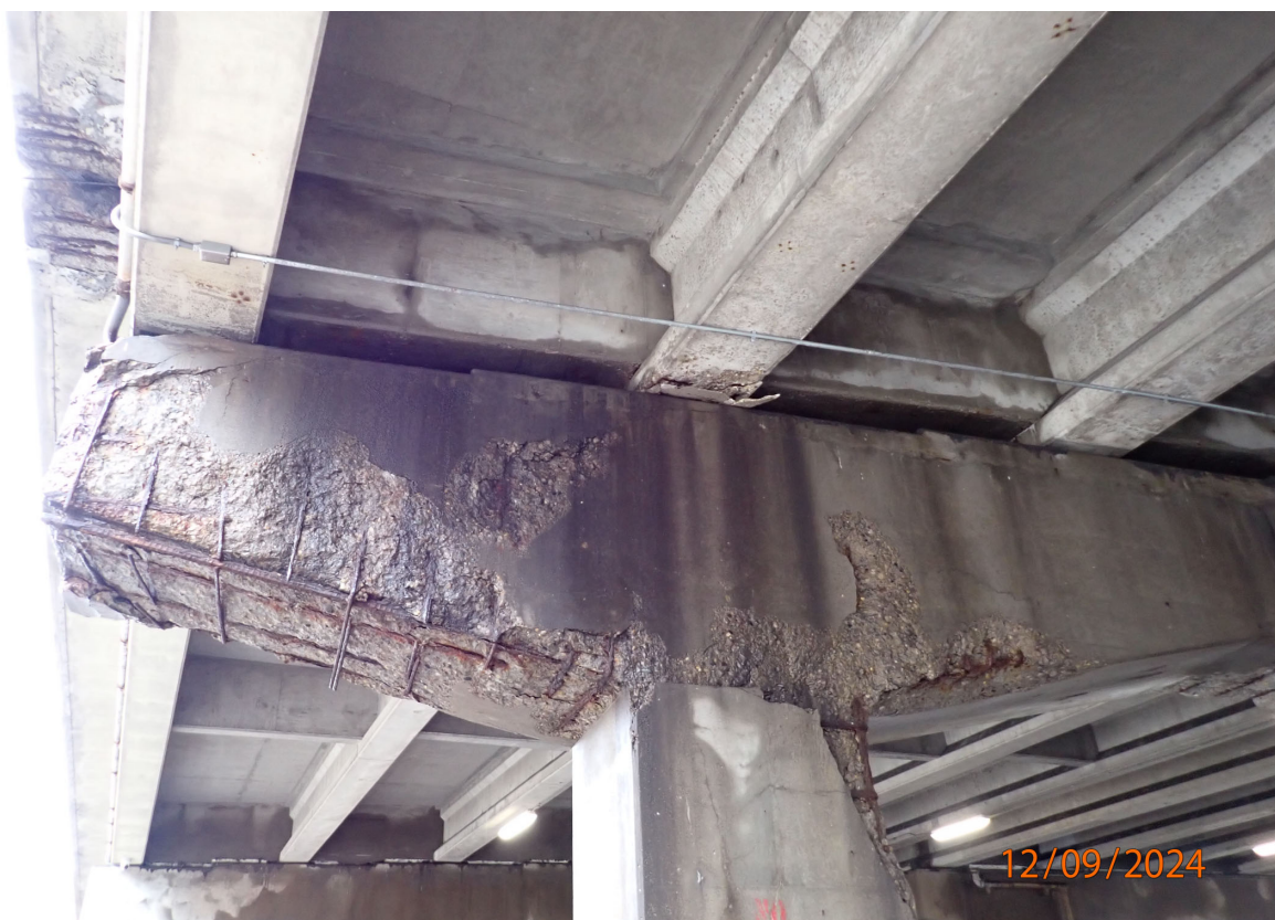
Deterioration is widespread on P3 and P7 (east end shown) below the joints. Note spall in B13 bottom flange.
