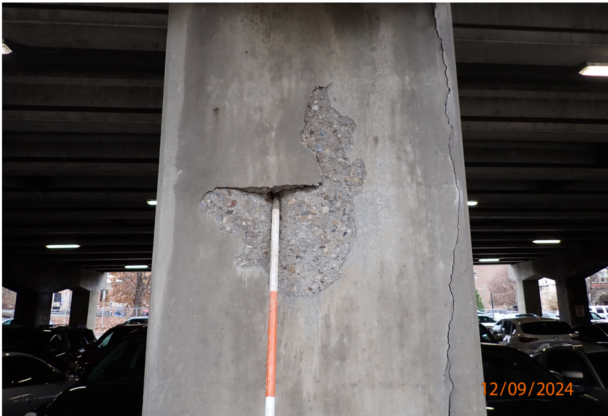
P5-C5 has a 2 SF spall and wide vertical cracking.
