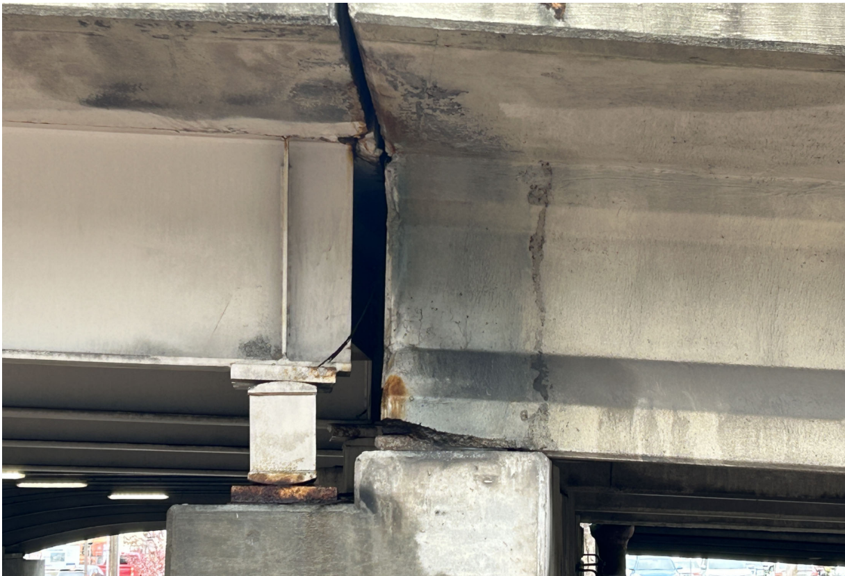
Ramp A: Pier A-4 typical bearings.
