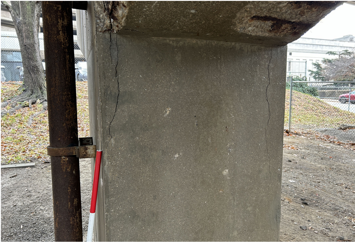
Ramp A: Pier A-4 column wide vertical cracks.
