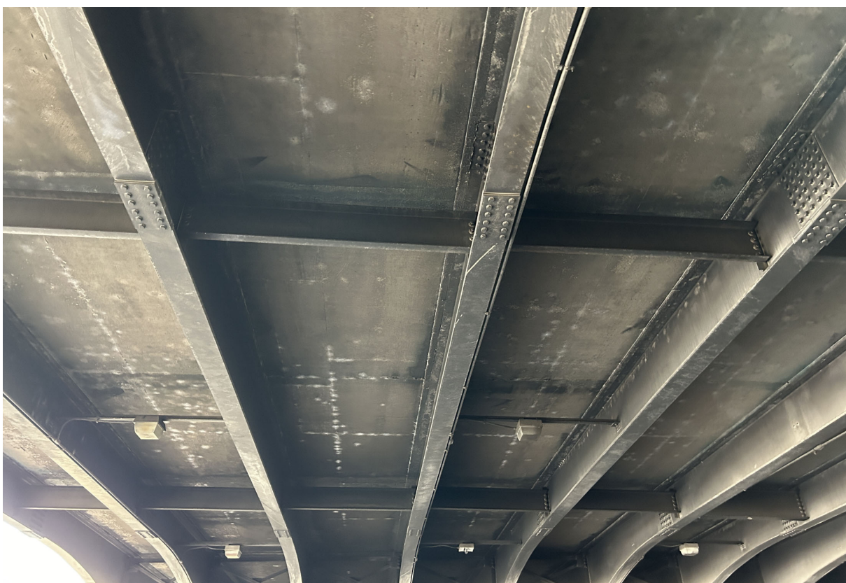
Span 123 is covered in soot from fires under the bridge.
