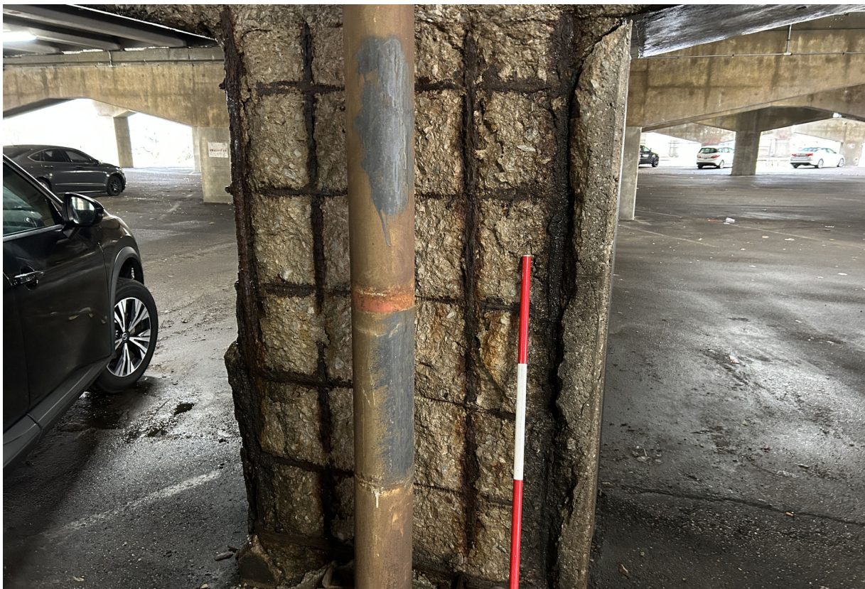
Pier 109E-Column 1 has spalling with exposed rebar throughout the south face.
