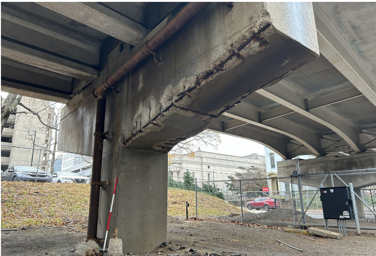
Ramp A: Pier A-4 has large spalls with exposed rebar on the west end of the cap.
