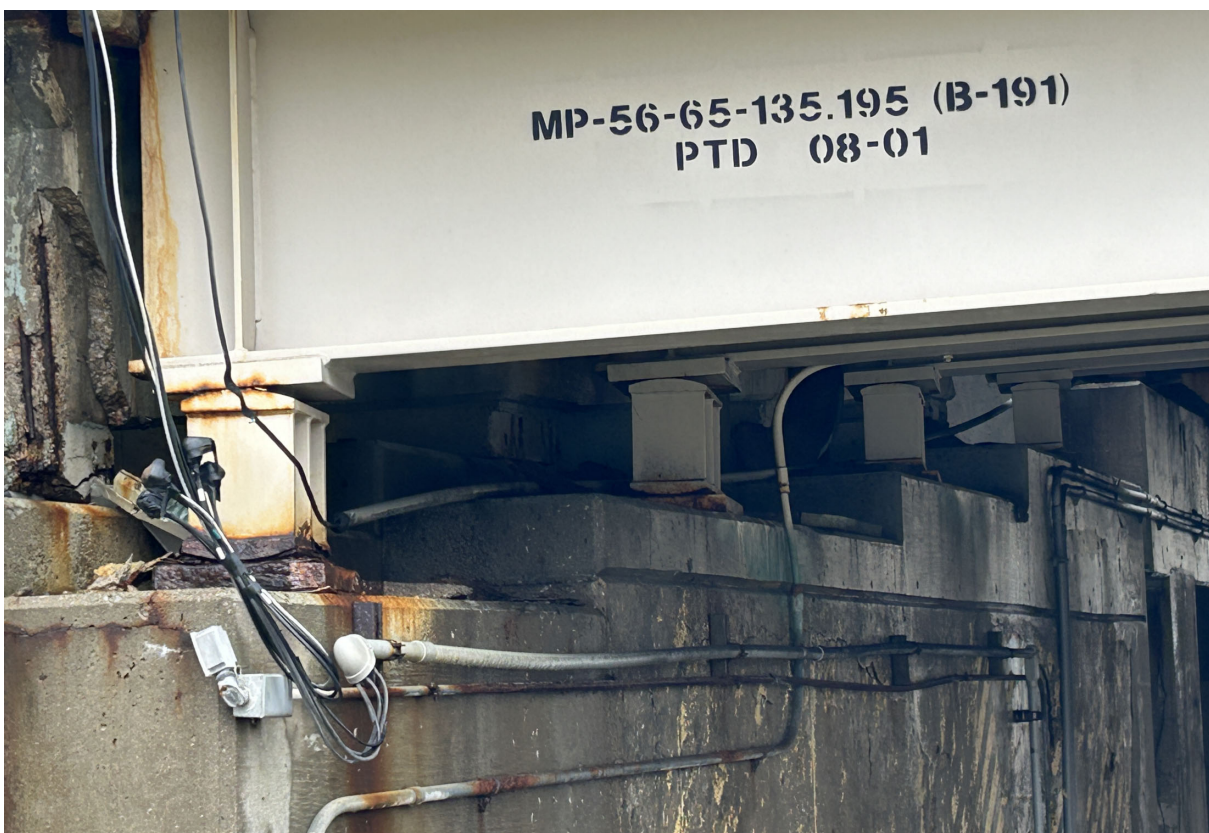
Ramp B: Pier B-2 typical rocker bearing in Span 104 with corrosion on the lower part of the bearing and the masonry plate.
