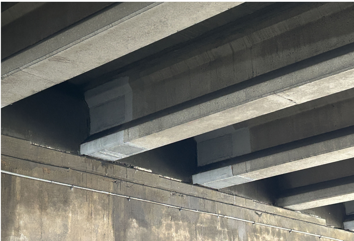
Several PCI beam ends in Spans 107 through 112 have sound CFRP patches, most in the SB portion. Span 107 at Pier 107W shown.
