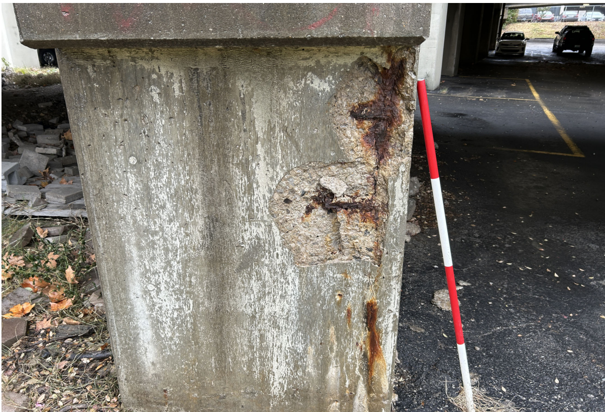
Ramp B: Pier B-1 Column 1 has large spalls with exposed rebar.
