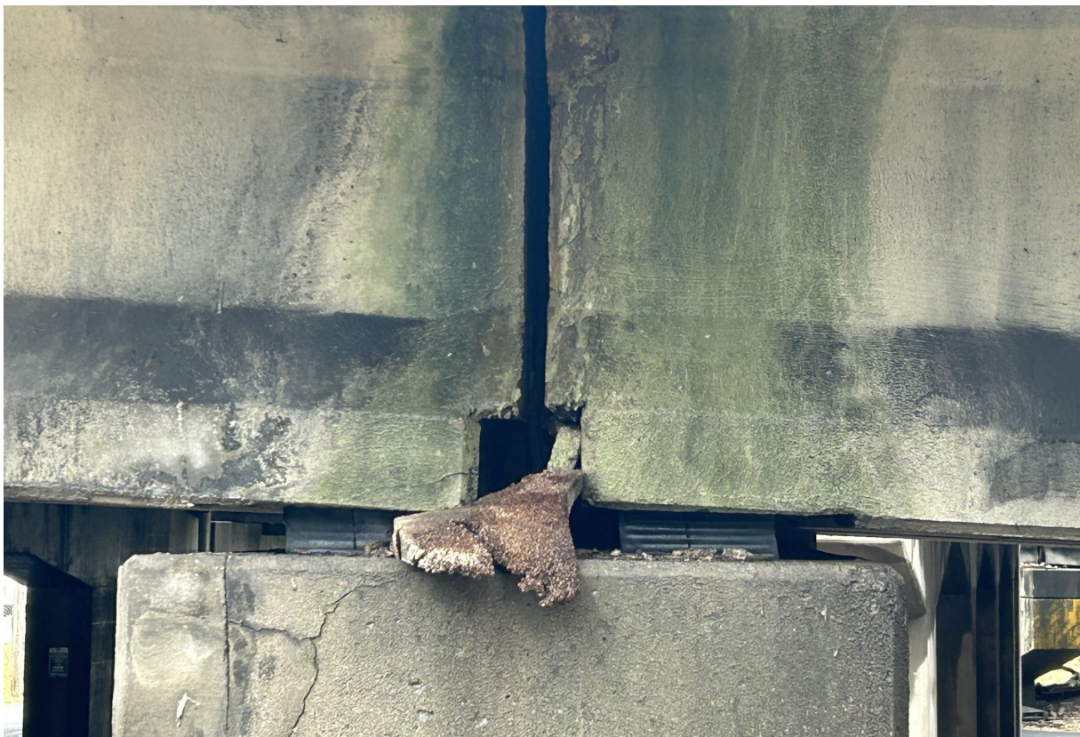
Typical Pier A-5 bearing pads.
