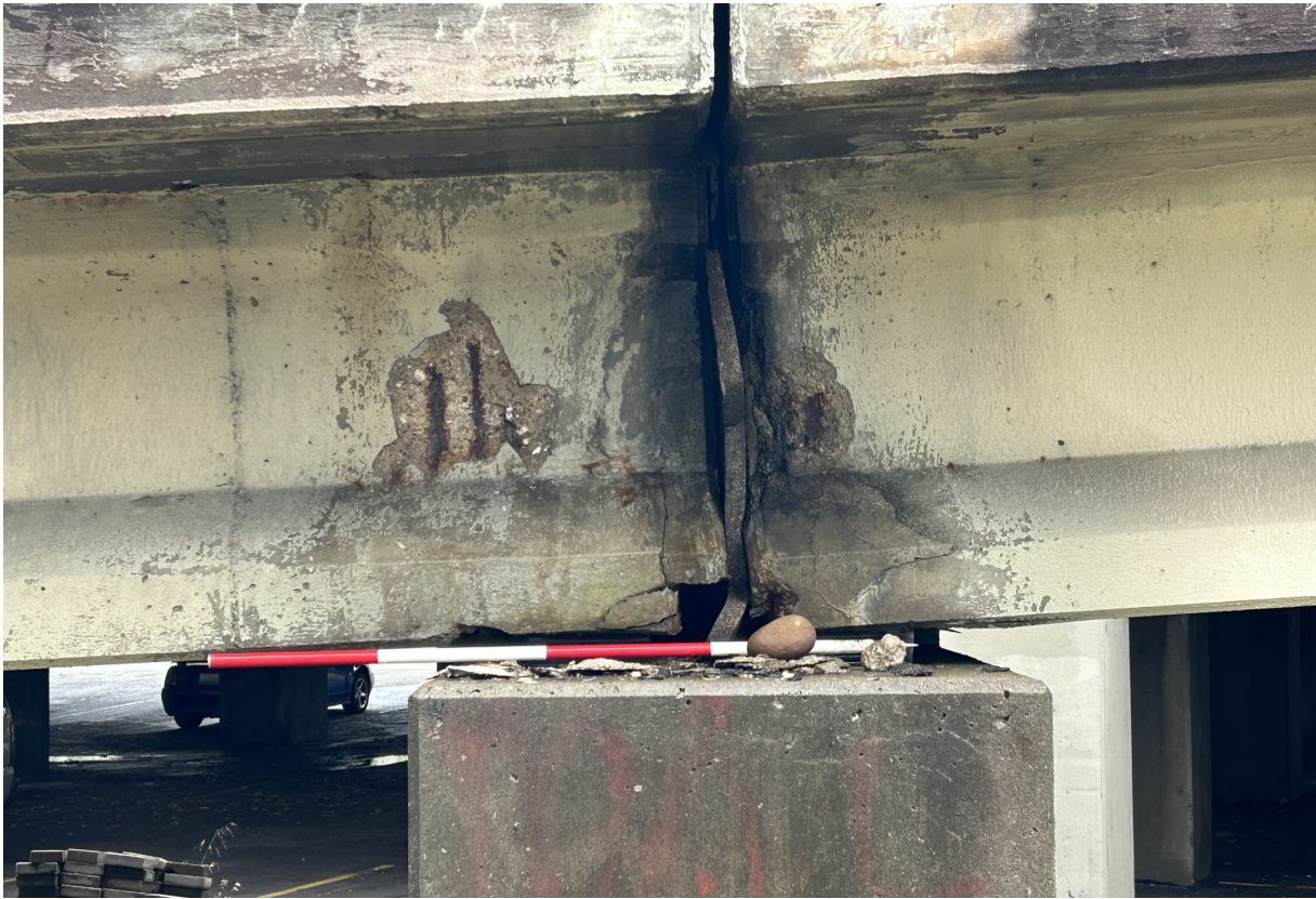
Ramp B Beam 4 at Pier B-1 wide cracking and spalls with exposed rebar.
