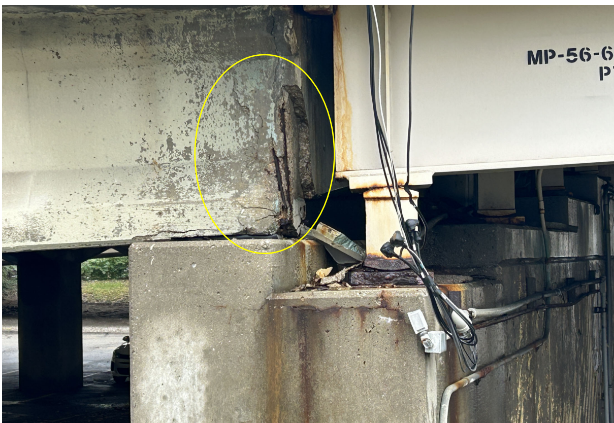
Ramp B: Beam 1 at Pier B-2 spalling with exposed rebar.
