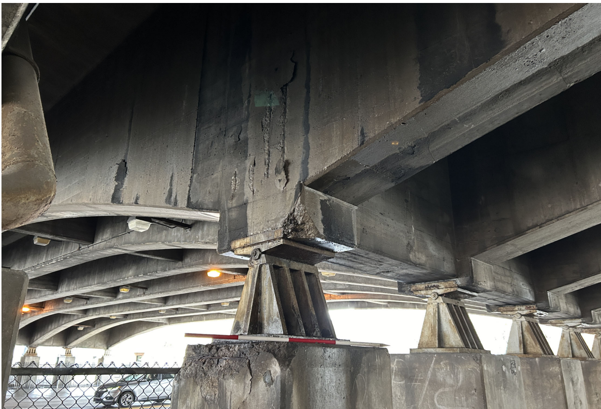
Pier 113 Column 7 has a large corner spall with exposed rebar.
