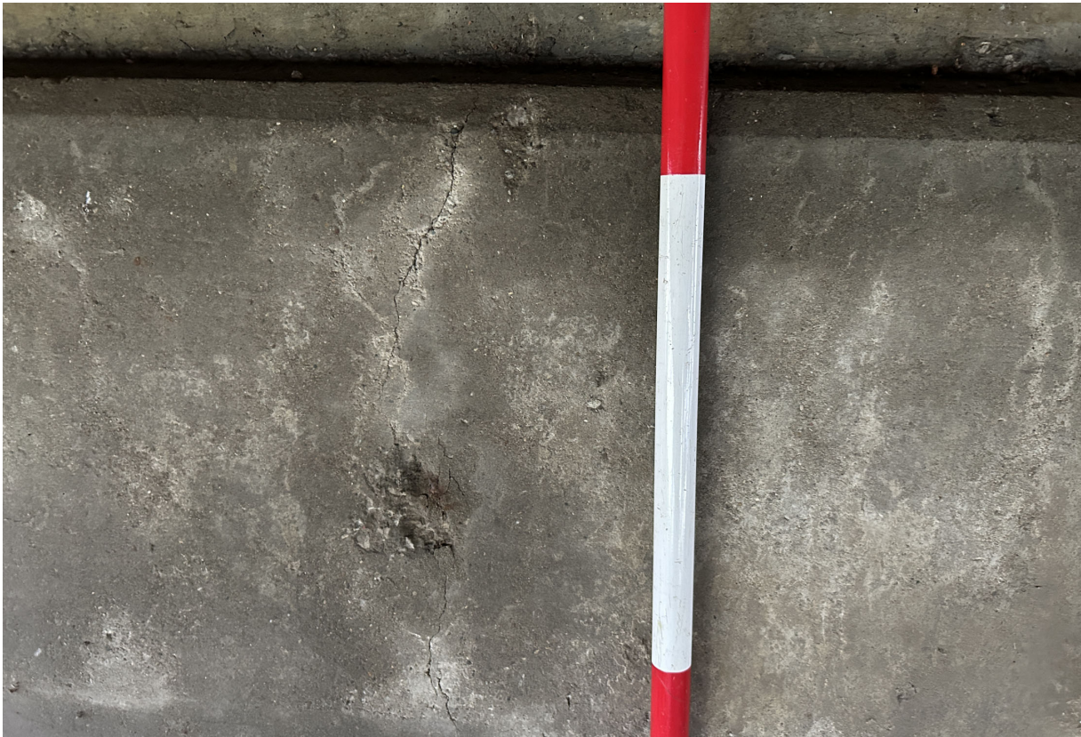
Abutment B has a few vertical cracks and small delaminations.
