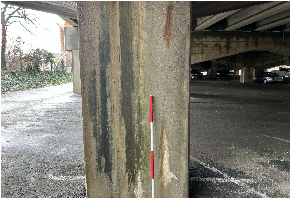
Pier A-1/Column 1 cracking with efflorescence and rust staining.
