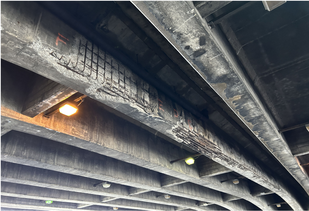
Beam 8 in Span 114 over Broadway has large spalls with exposed rebar for 72 linear feet.
