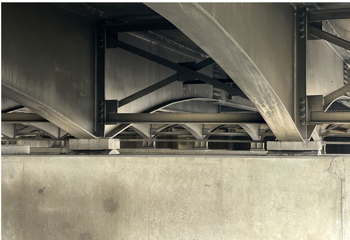
Typical Pier 123 bearings.
