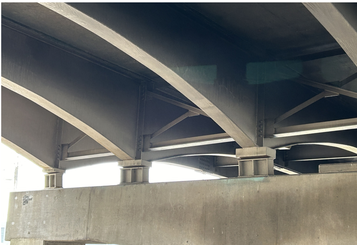
Typical Pier 122 bearings.
