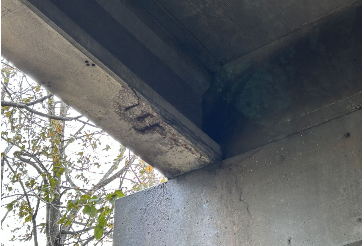
Large spall and wide longitudinal cracking on the bottom face of Beam 16 in Span 119 at Pier 119E.
