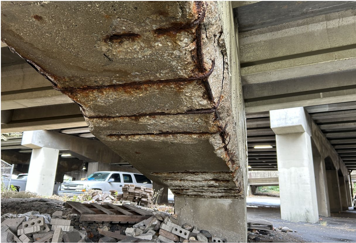
Ramp B: Bottom face of Pier B-1 cap has large spalls with exposed rebar.
