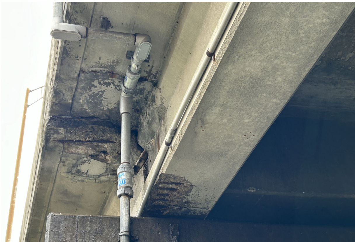
Beam 1 at Pier 109W in Span 110 has a large spall with exposed rebar in the bottom face. West overhang also has large spalling at the pier joint.
