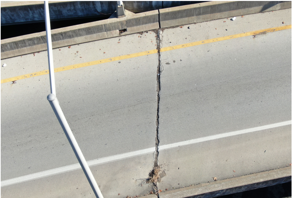
Joint over Pier B-2.
