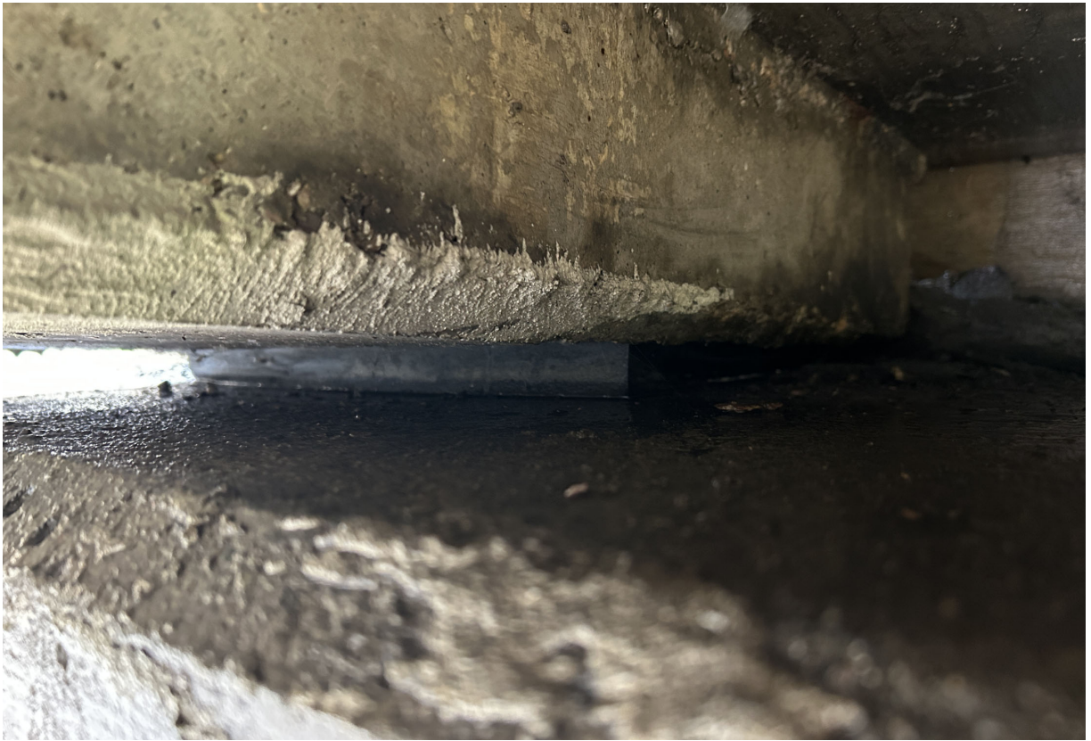
Ramp A: Typical Abutment A bearing pad.
