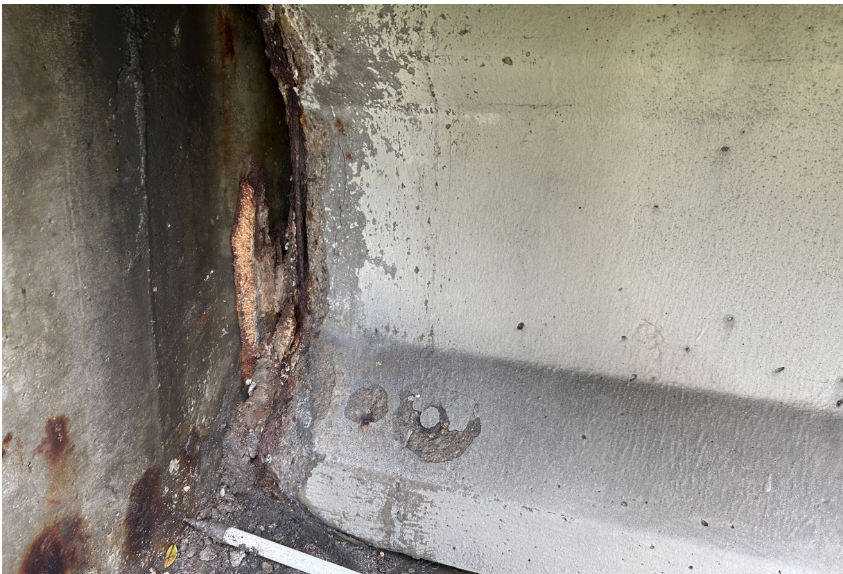
Ramp B Beam 1 has cracking and spalling with exposed rebar at the end.
