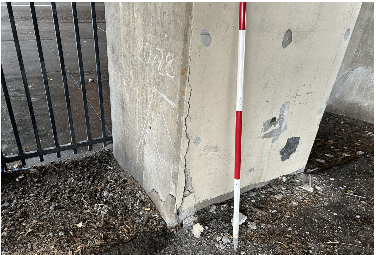
Wide vertical cracking on Column 4 at Pier 114.
