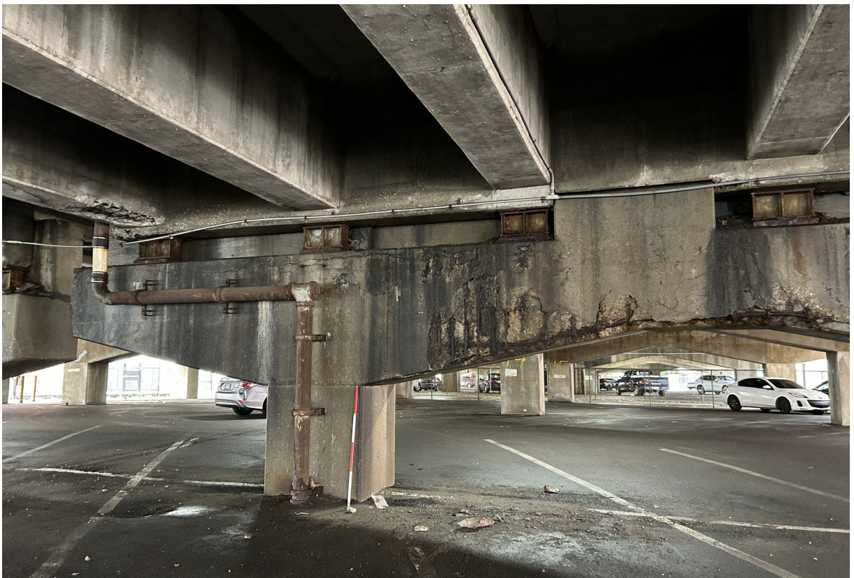
Pier 112E south face large spalls with exposed rebar and wide horizontal cracking.
