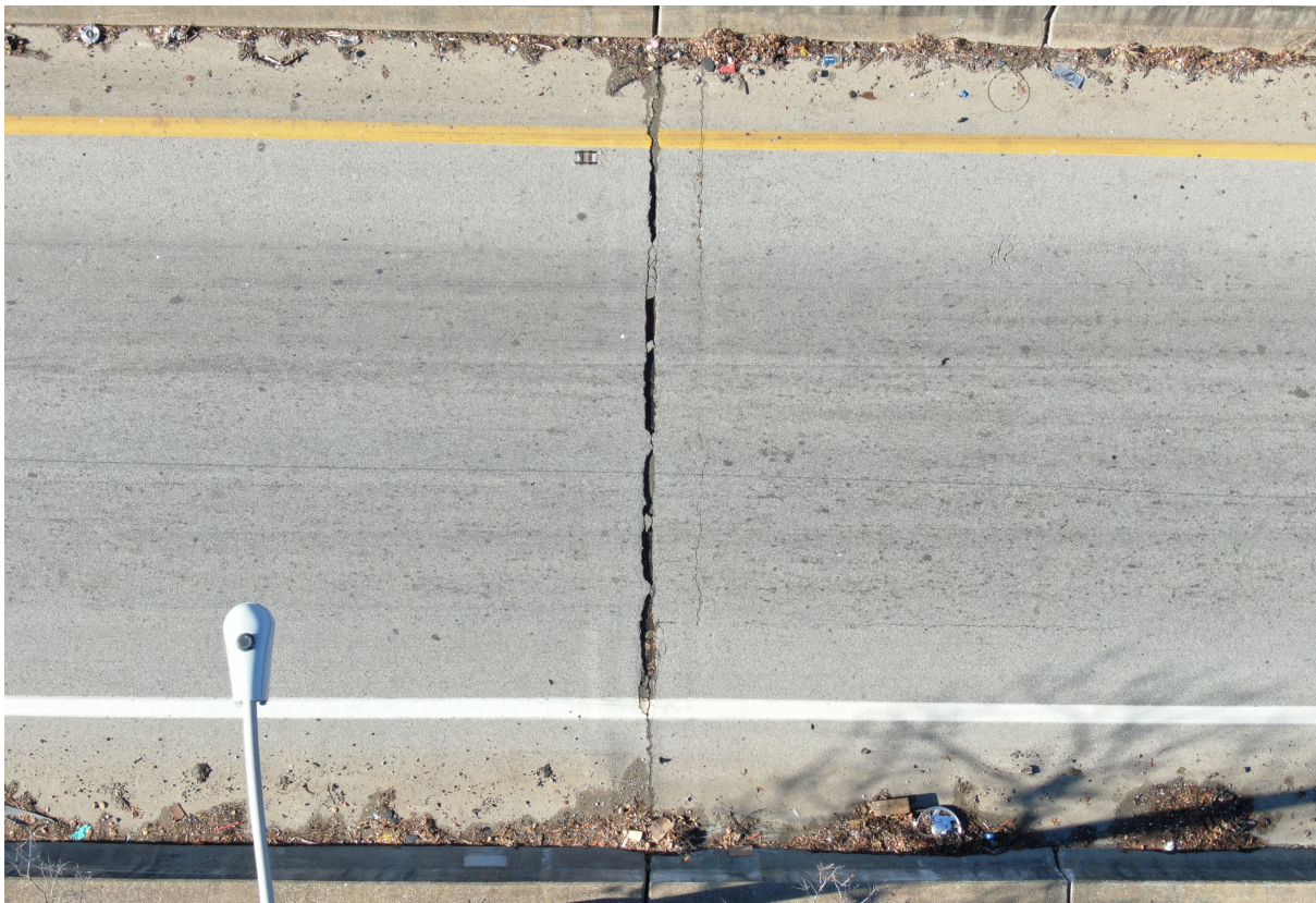
Joint over Abutment A.
