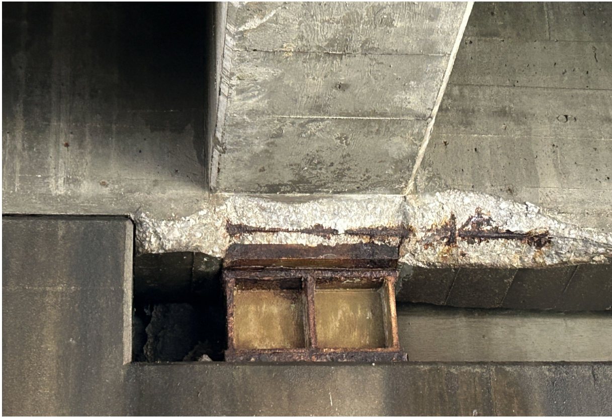
Typical Pier 115 bearing. Note spalling in diaphragm.
