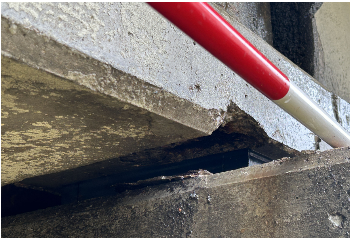
Ramp B: Pier B-1 typical bearing pad.
