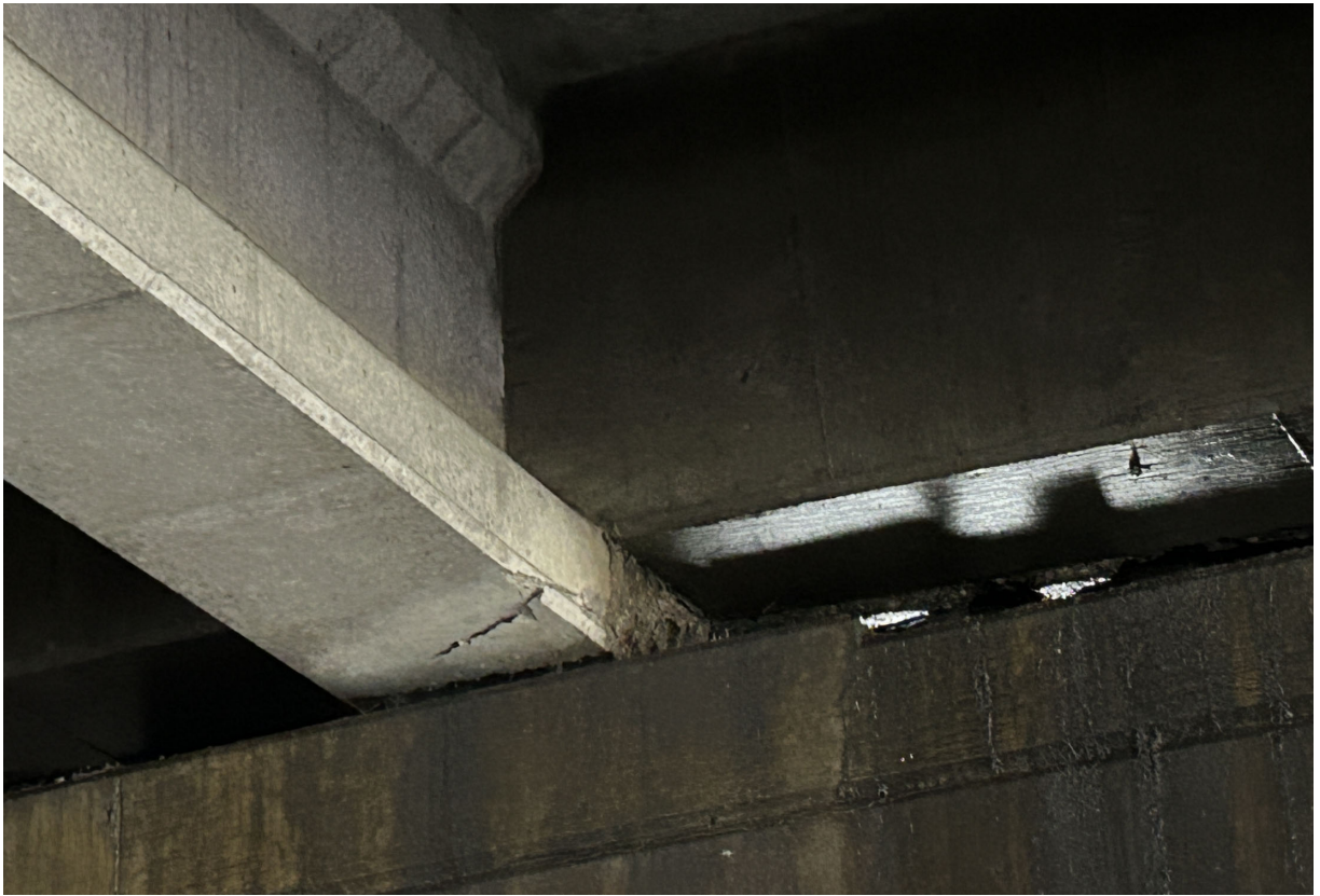
Beam 9 at Pier 109W has a wide crack in the bottom face in Span 109.
