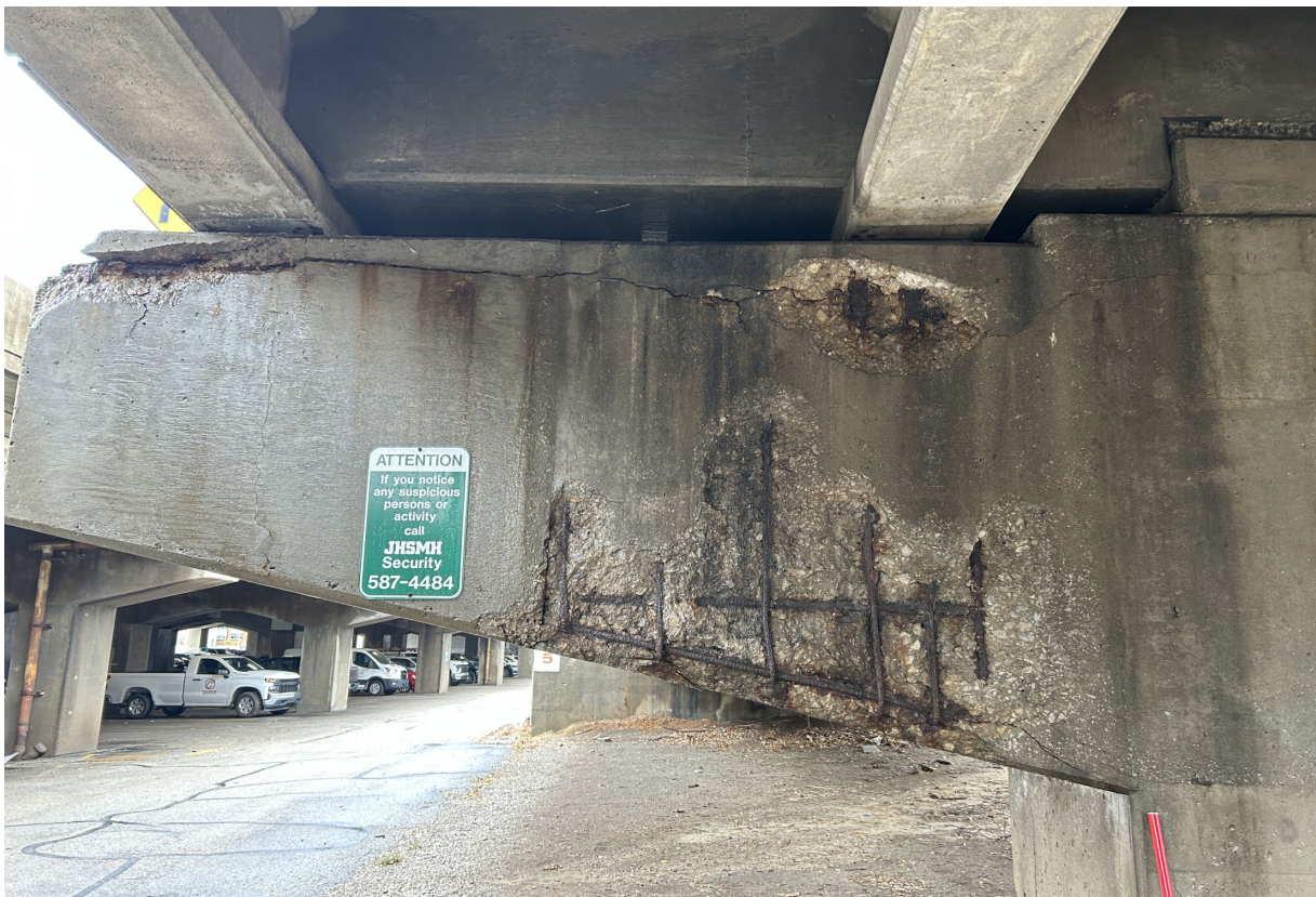
South face of Pier A-5 has large spalls with exposed rebar and wide horizontal cracking.
