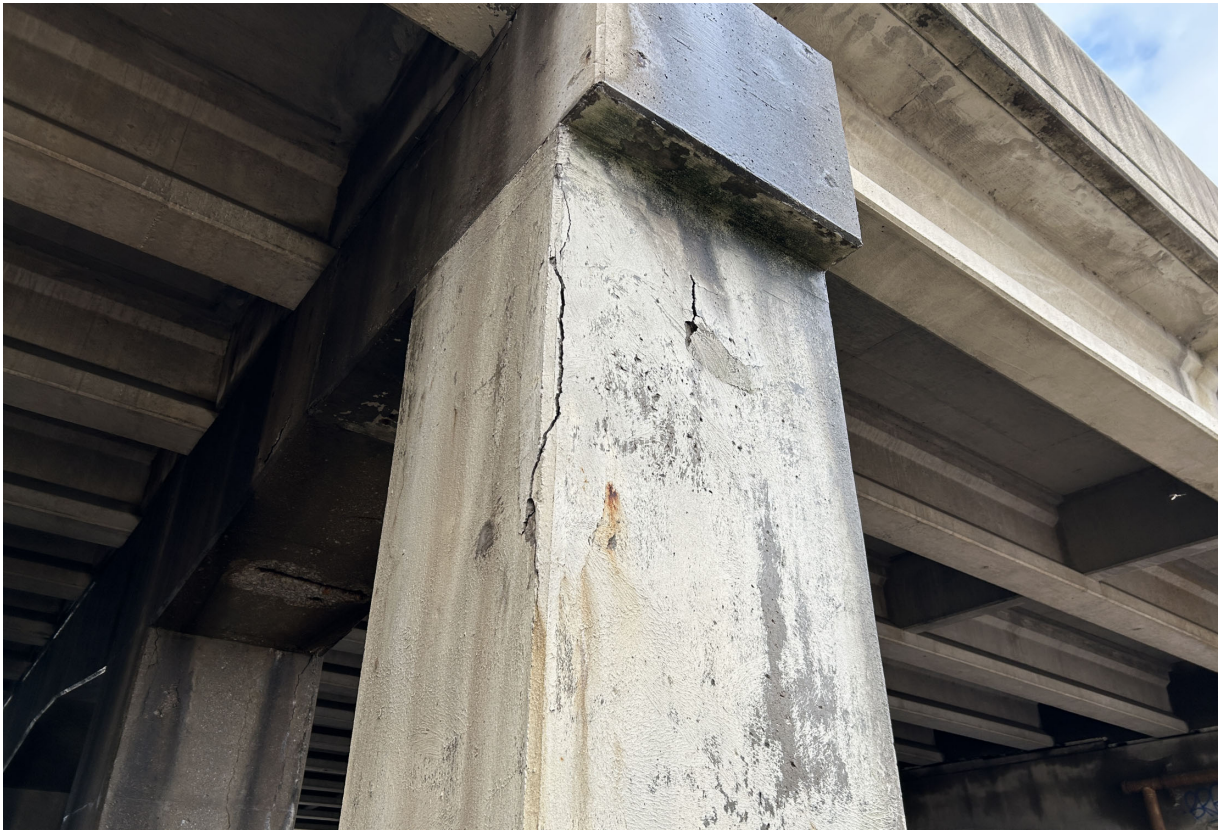
Wide vertical cracking on Column 6 at Pier 118E.
