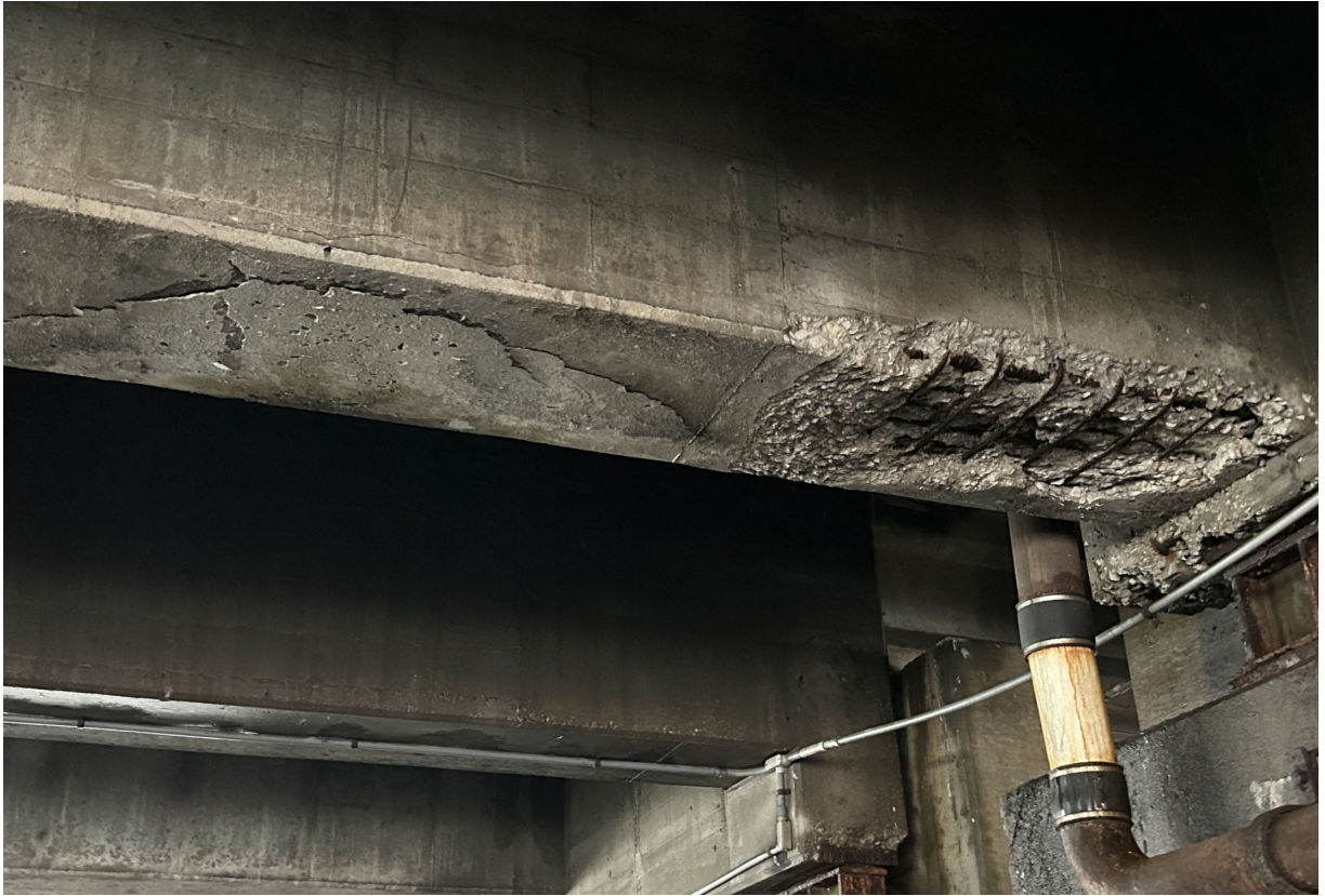
Beam 8 in Span 113 near Pier 112E has wide cracking and a large spall with exposed rebar.
