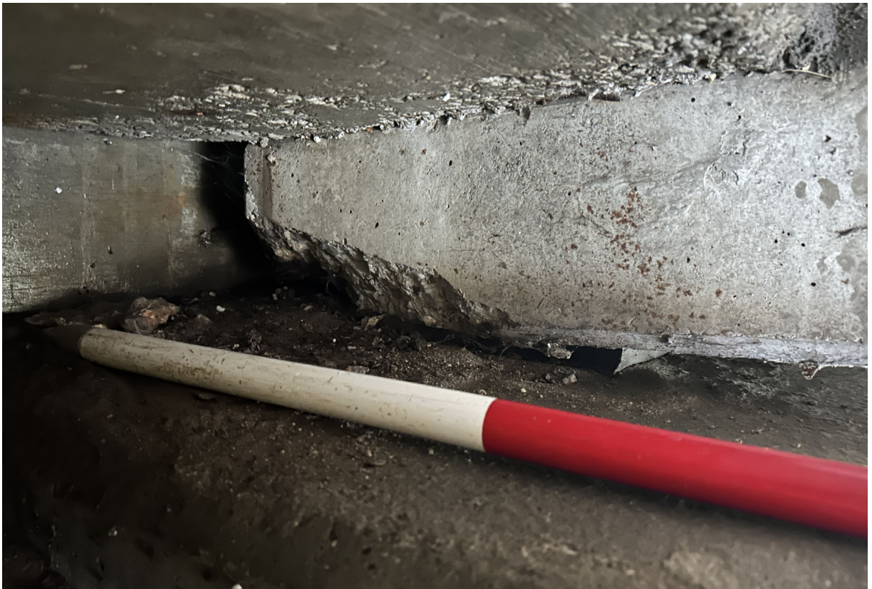
Beams 3 and 4 at Abutment A have end spalls with exposed strands. Beam 3 shown.
