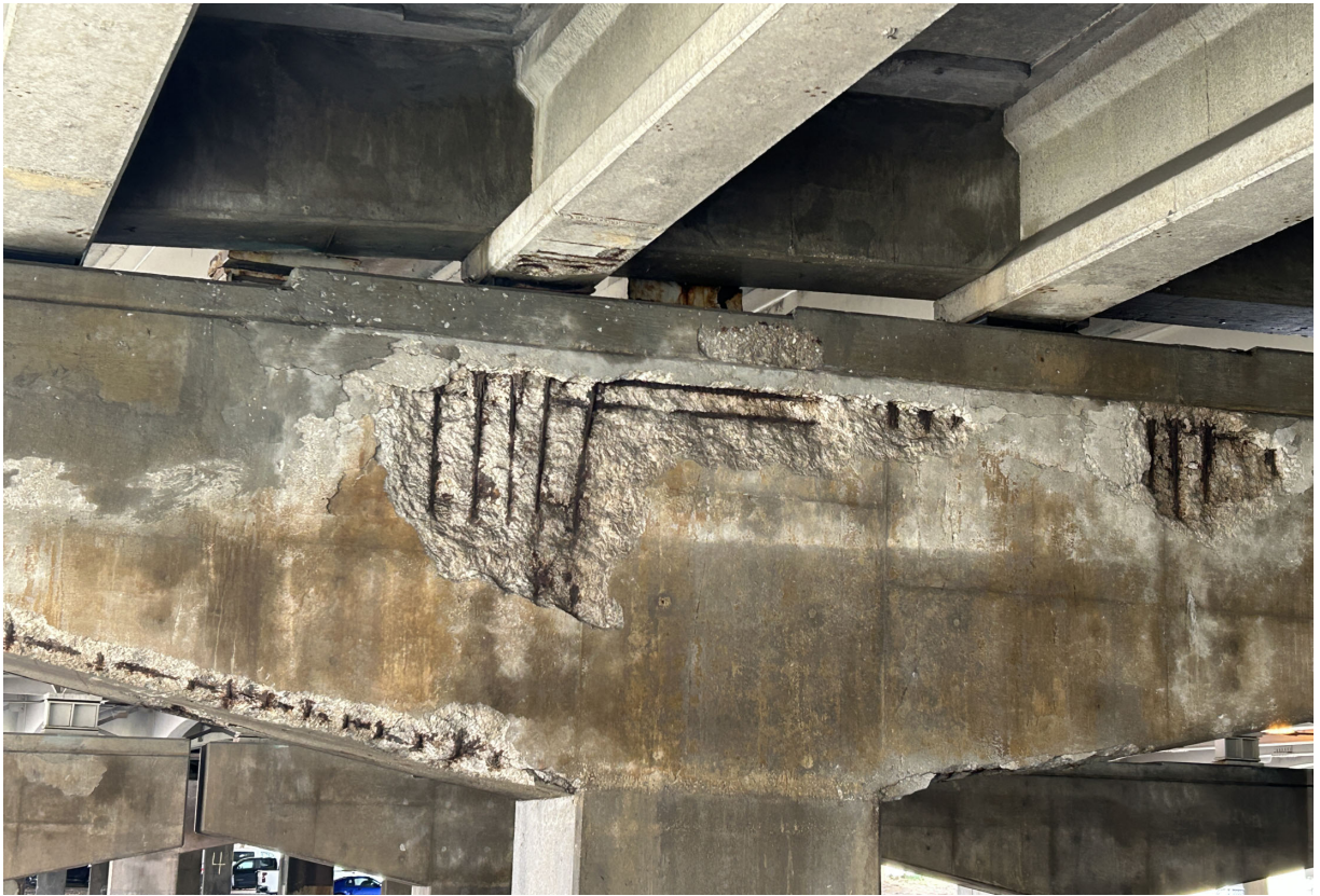
Pier 106W south face large spalls with exposed rebar.
