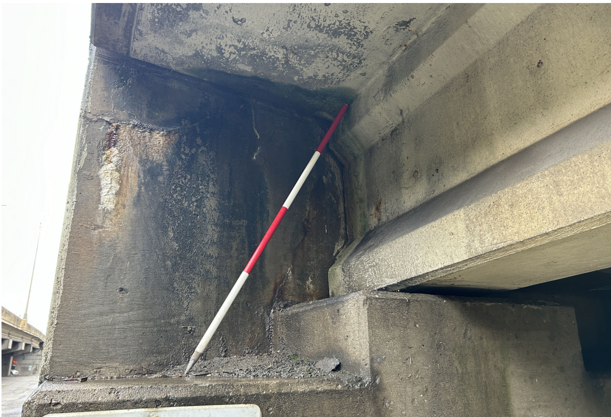
Ramp A: Backwall of Abutment A has cracking with efflorescence and rust staining at the west end.
