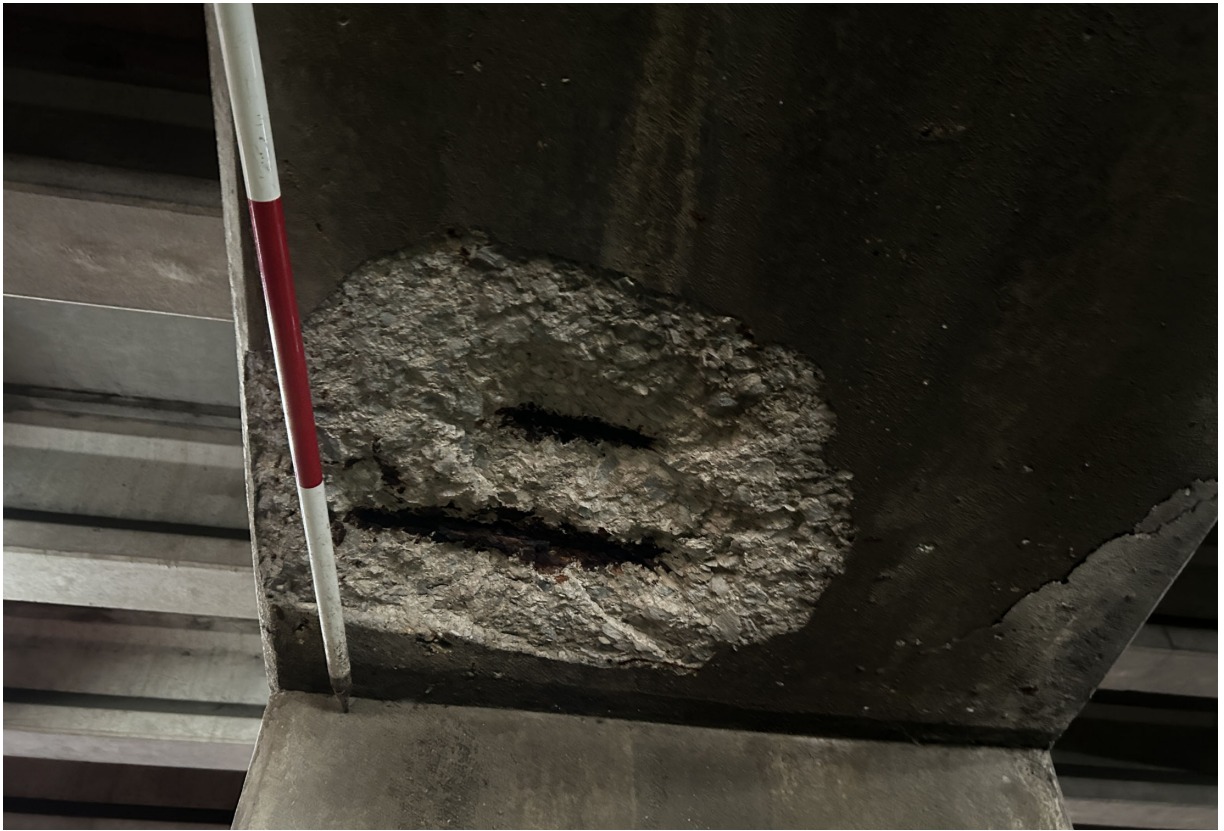
Pier 111E cap has a large spall with rebar in the bottom face.
