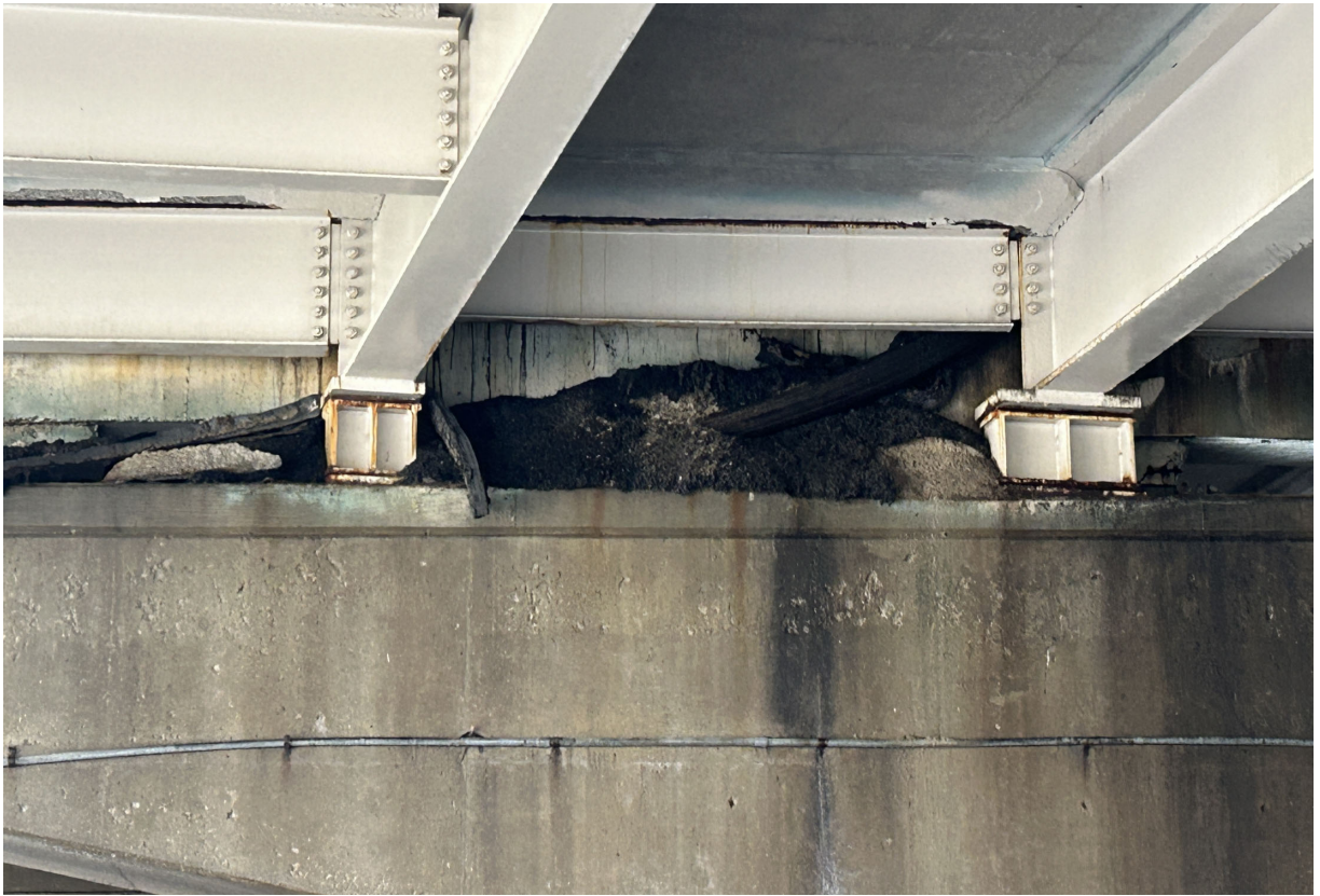
Pier 106E north face bearings partially covered with asphalt.
