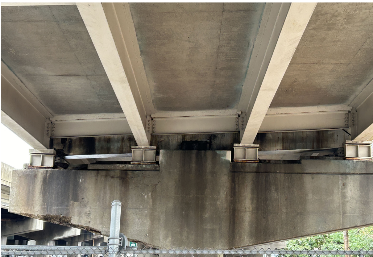
Pier A-4 Span 104 bearings.
