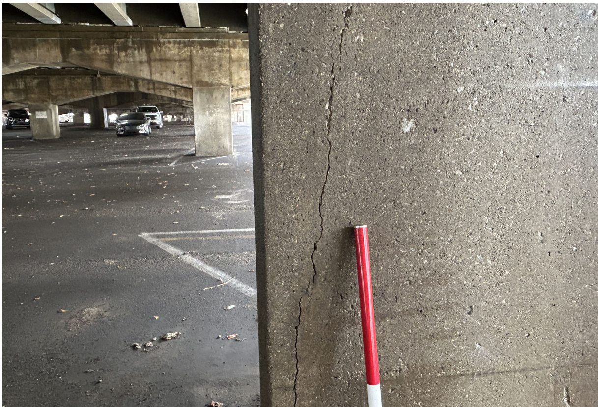
Pier 106W Column 2 wide vertical crack.
