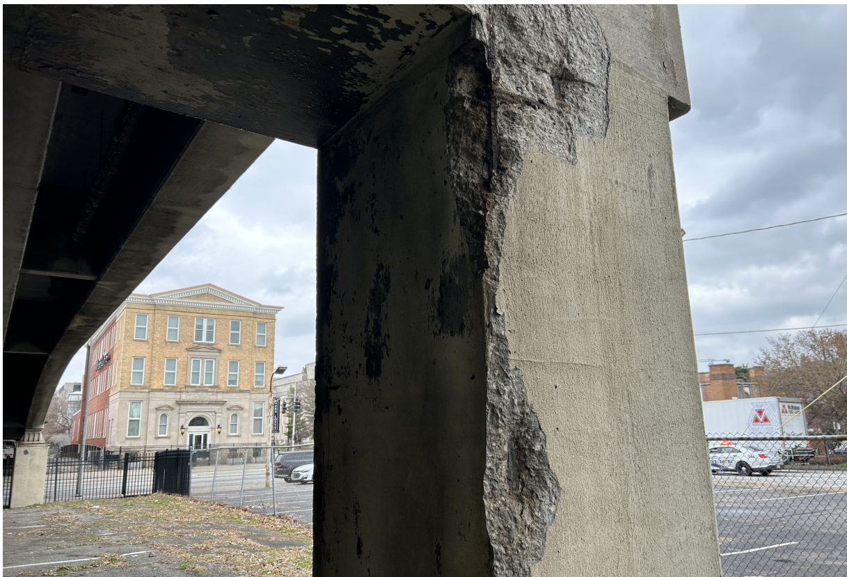
Spalling with exposed rebar in Pier 115E Column 3.
