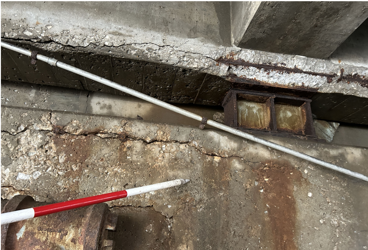
Pier 112W south face wide horizontal crack.
