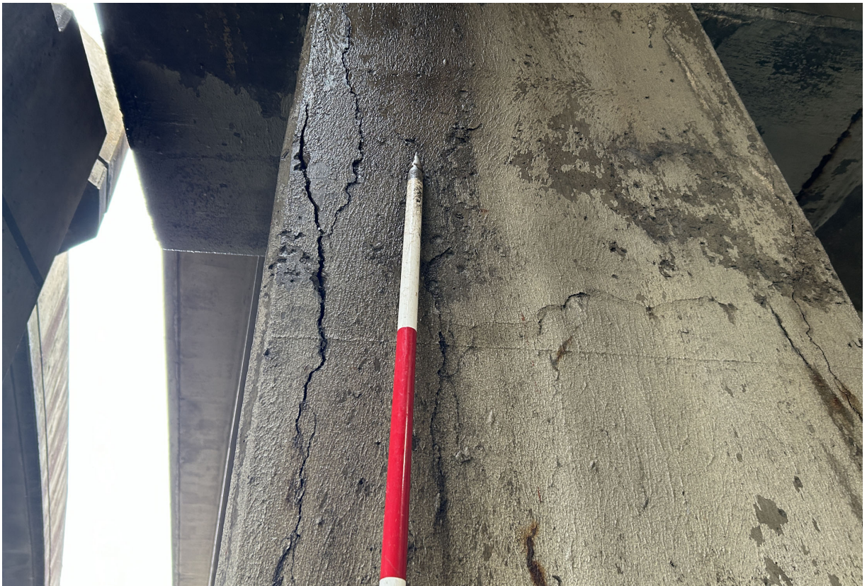
Pier 103W wide vertical cracking on Column 1.
