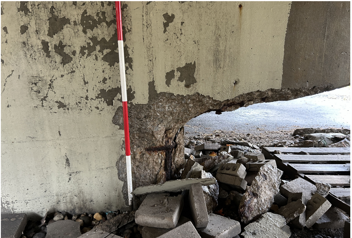
Ramp B: Pier B-1 Column 2 has deep spalls with exposed rebar.
