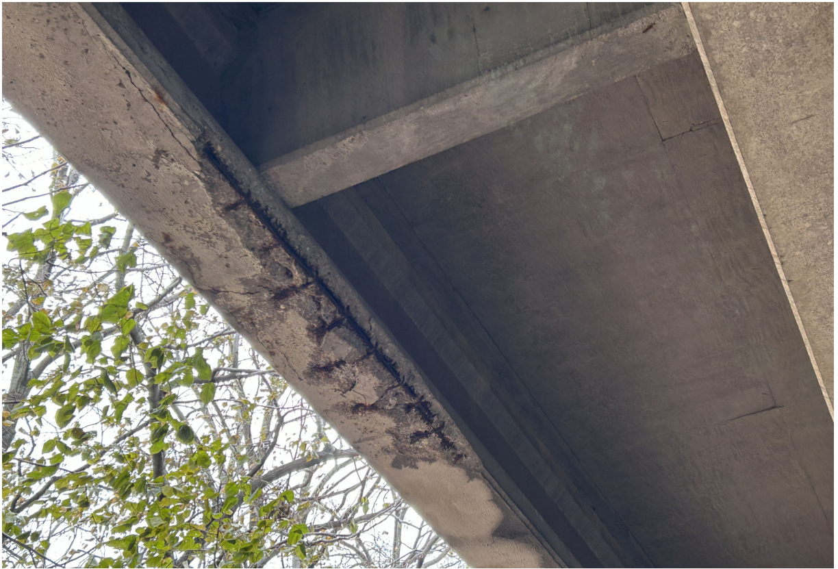
Beam 16 bottom flange in Span 120 has cracking and a large spall with exposed rebar mid-span.
