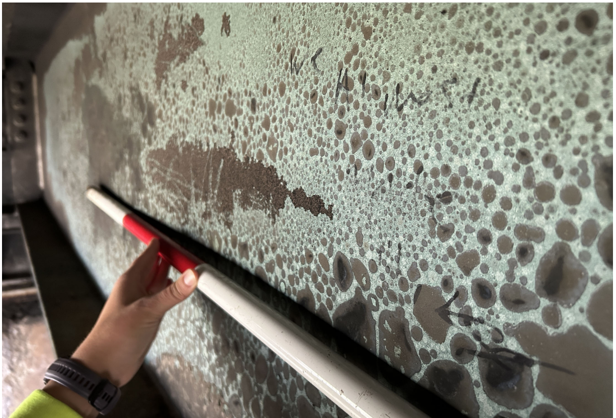
Close up of peeling paint on Beam 13 at Abutment C.
