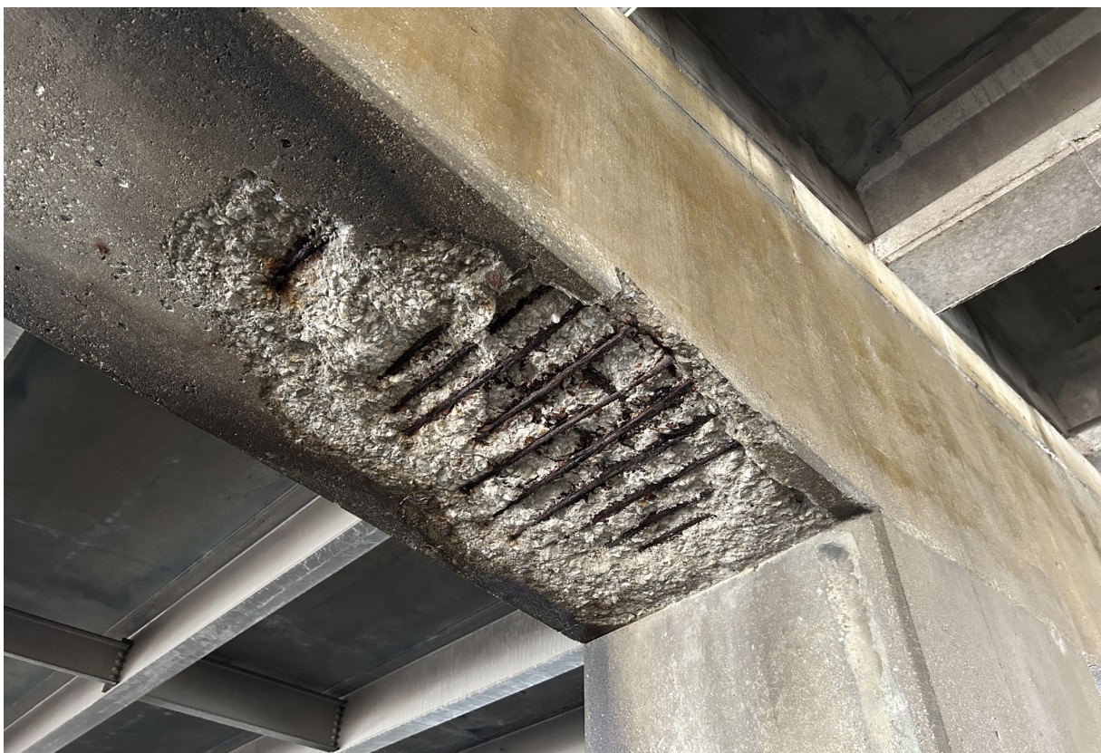
Bottom face of Pier 121E cap has a large spall with exposed rebar.
