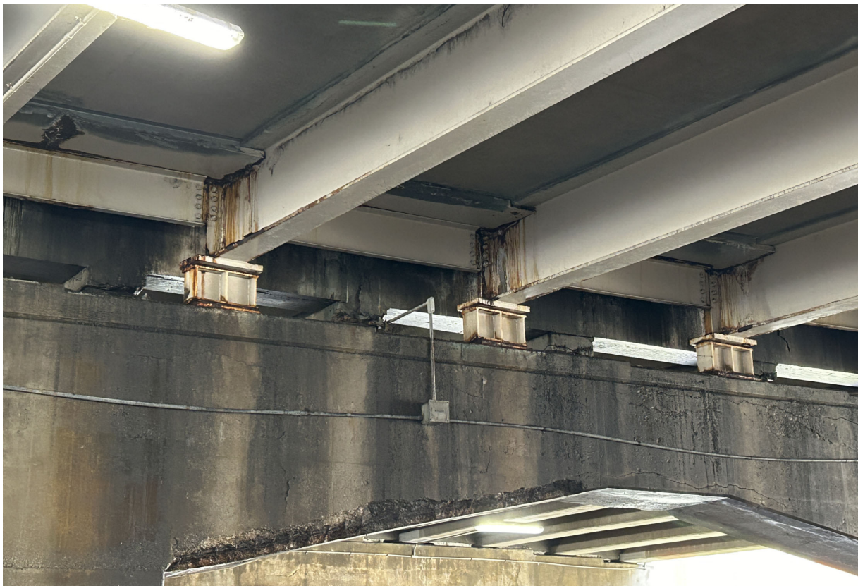
Typical Pier 106W north face bearings.
