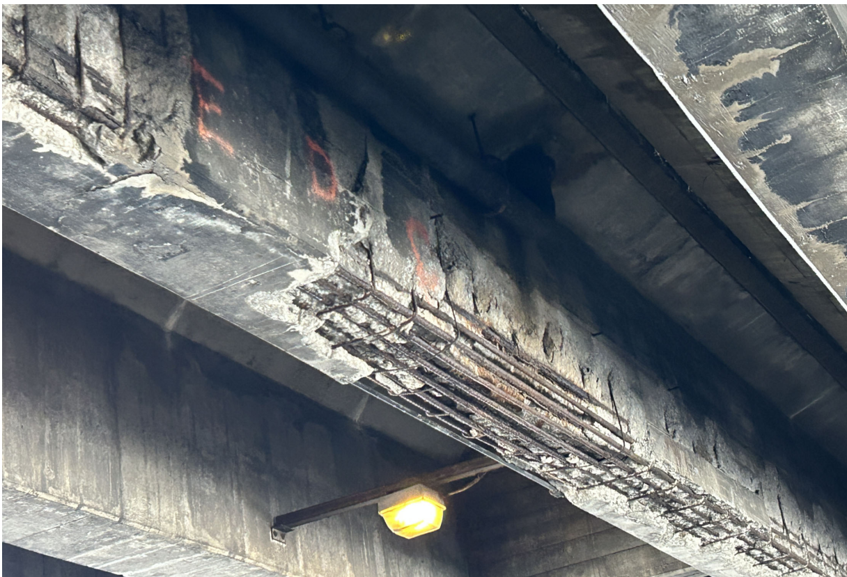
Spalling in Beam 8 is worst near midspan exposing 3 layers of rebar with section loss.
