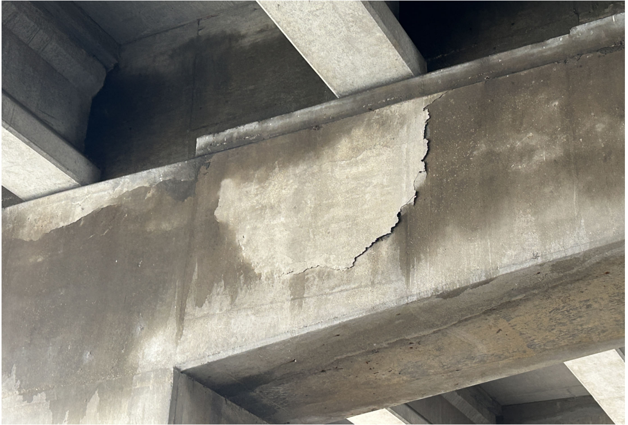
Pier 117E cap has a large delamination on the north face.
