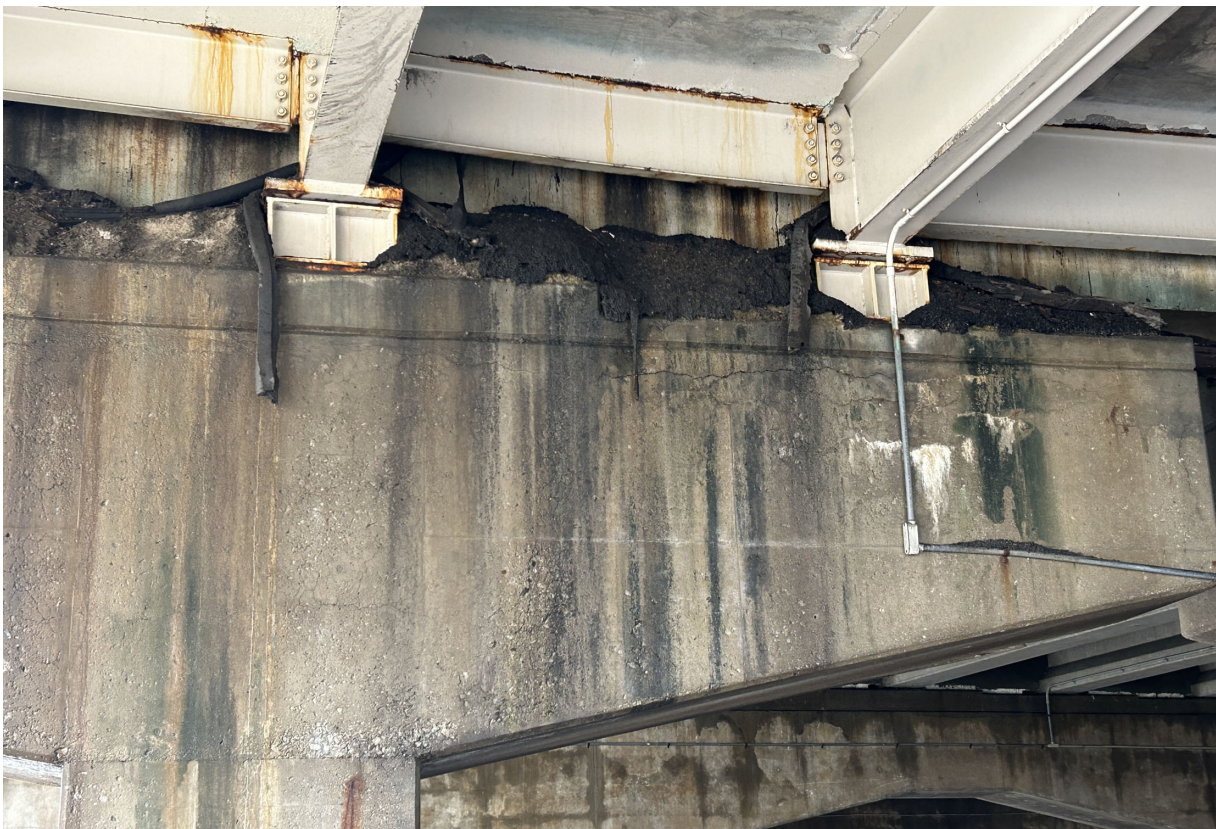
Several rocker bearings at Pier A-1 are partially buried in asphalt.
