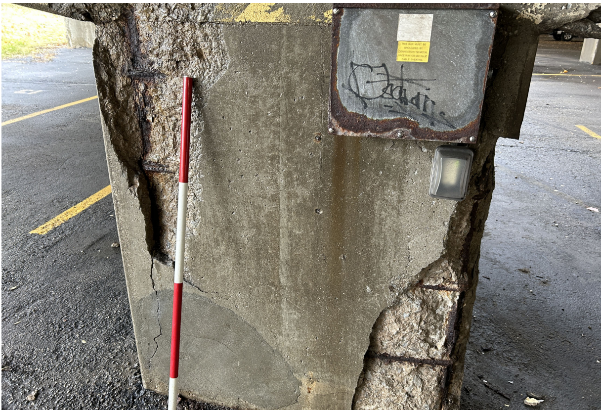
Ramp B: Pier B-2 Column 2 has deep spalls with exposed rebar.
