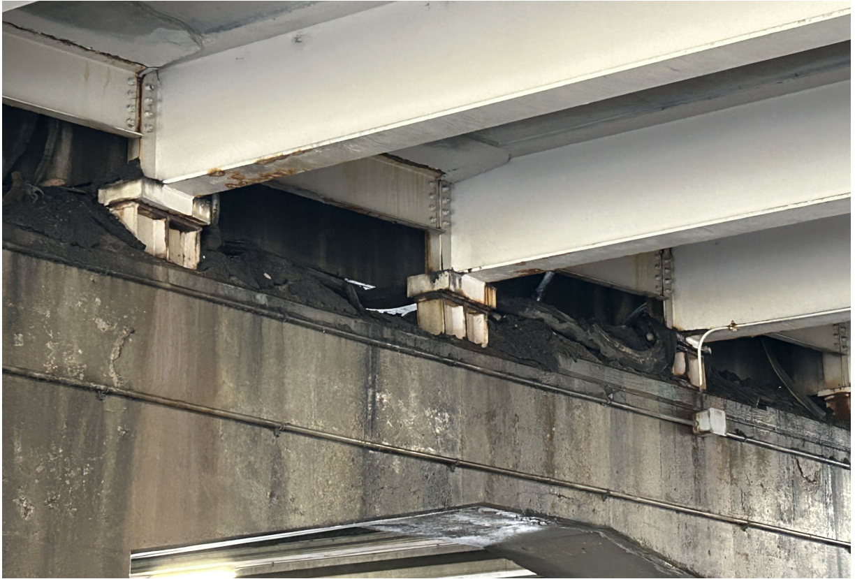
Several rocker bearings at Pier 103W and 103E are partially buried in asphalt.
