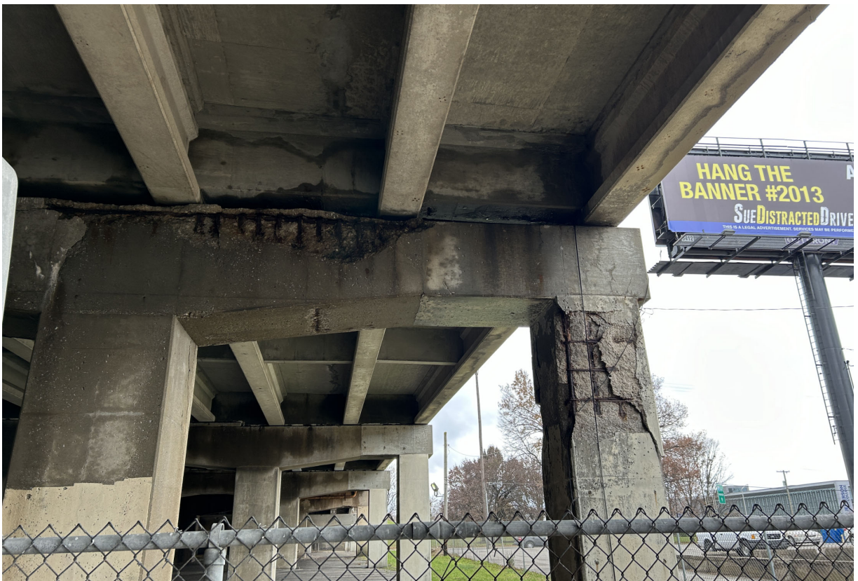
Large spalling in Pier 118W north face and Column 1.
