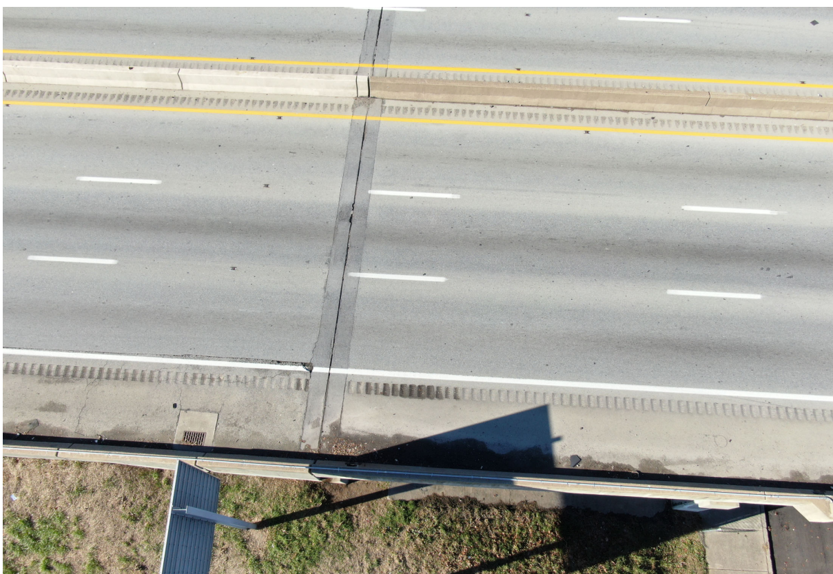
Joint over Abutment C.
