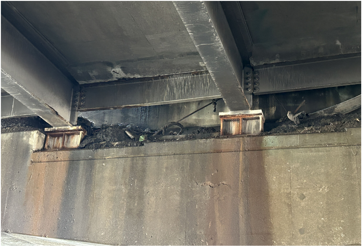
Typical Pier 121 bearings partially covered with debris.
