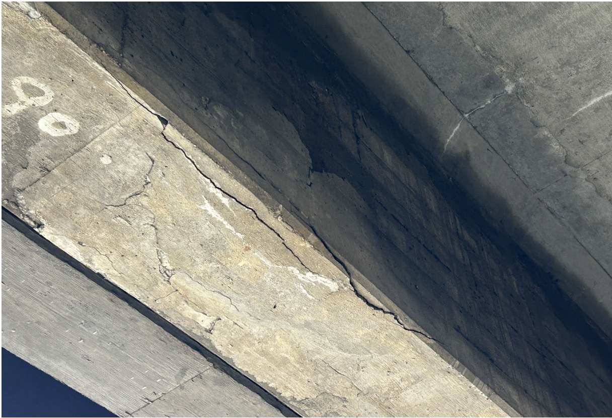
Beam13 in Span 115 has wide longitudinal cracking in the bottom flange.
