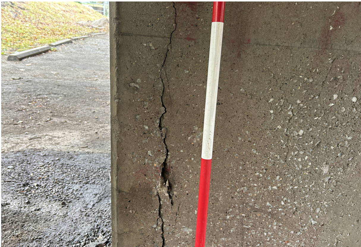
Ramp A: Wide vertical cracking in Pier A-5 column.
