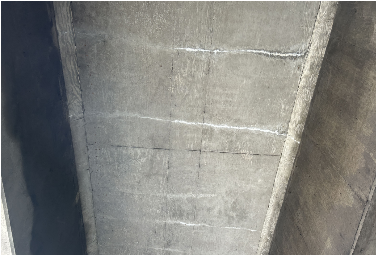
Span 113 soffit has a few intermittent transverse cracks with efflorescence.
