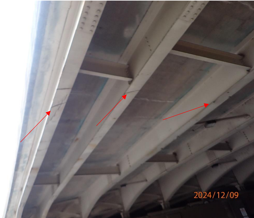
Span 2 Beams 1, 2, and 3 bottom flanges are scraped due to vehicular impact
