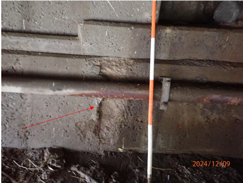
Spalling in Abutment 4 below Bay 3
