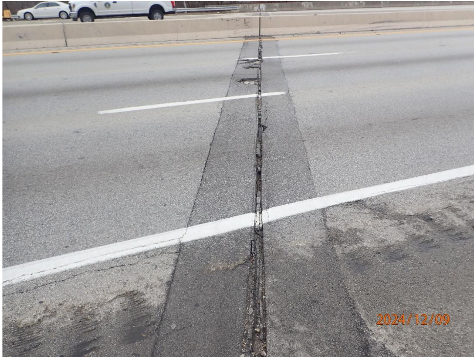
Joint over Abutment 4, SB lanes
