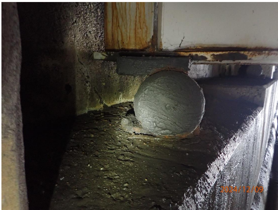
Many roller bearings are misaligned, movement is inconsistent with temperatures conditions (Beam 10 at Abutment 4 pictured)
