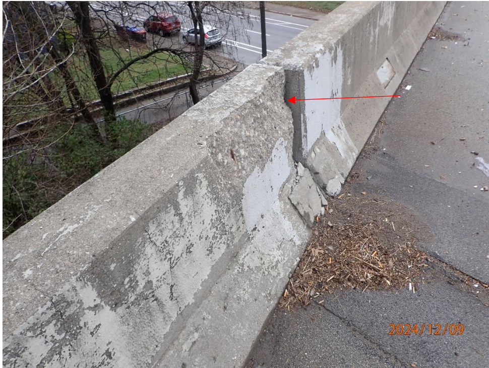
The approach concrete rail at the NE corner along the exit ramp has impact damage
