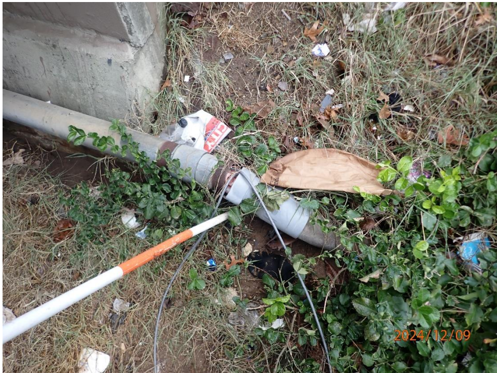
There is metal conduit attached to the full-length of Abutment 4 that has flaking corrosion and is broken at the east end
