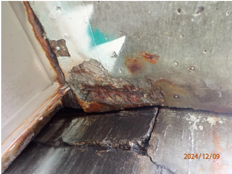
spalling with exposed rebar at Abutment 1 in the west overhang
