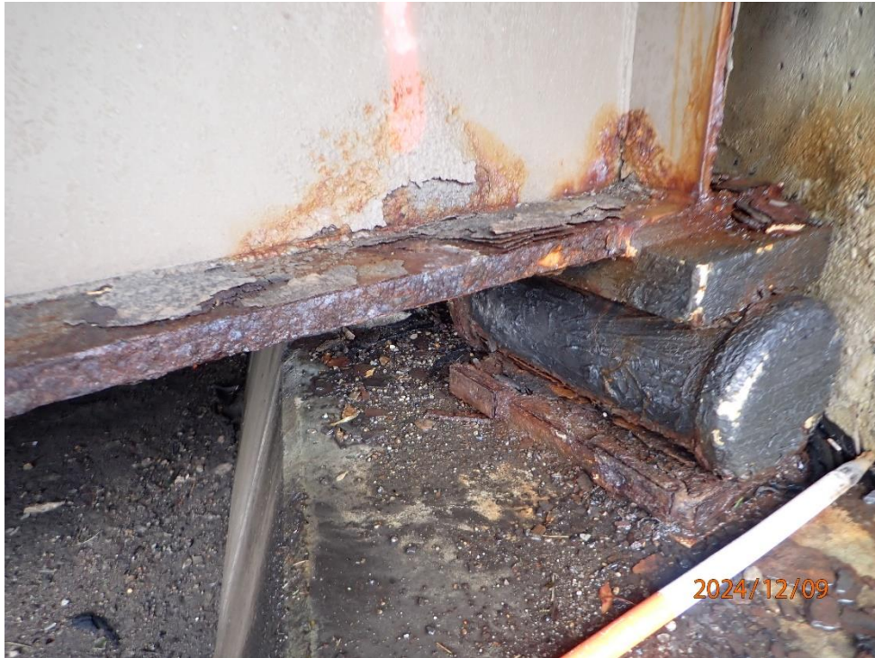
Flaking corrosion with very minor section loss on the bottom flange of Beam 1 at Abutment 1. Note flaking corrosion in the masonry plate.
