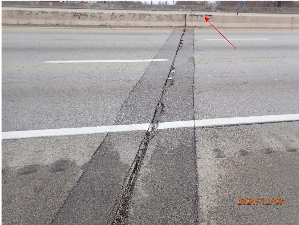
Joint over Abutment 1, SB lanes. There is a 3'L spall with exposed rebar along the top of the approach median at Abutment 1.
