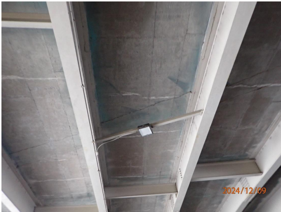
Soffit has transverse cracks with efflorescence
