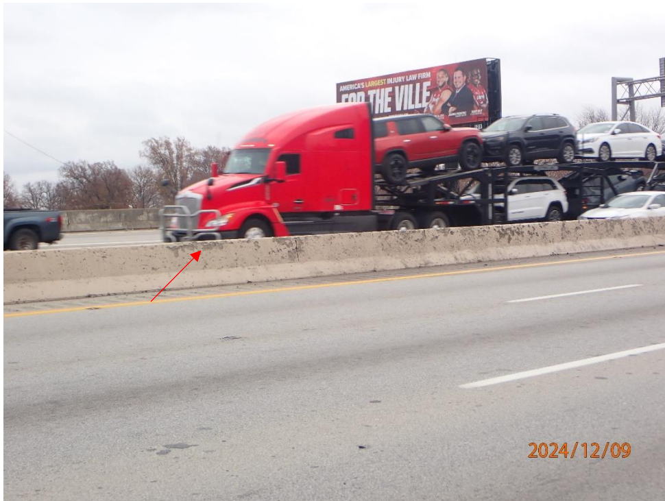
SB median barrier has moderate to heavy scaling for the south half of the bridge length
