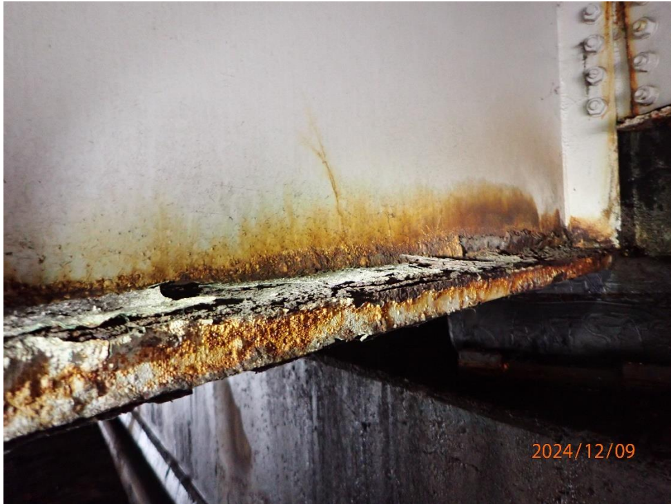
Beam 11 at Abutment 4 has flaking corrosion with very minor section loss on the bottom flange
