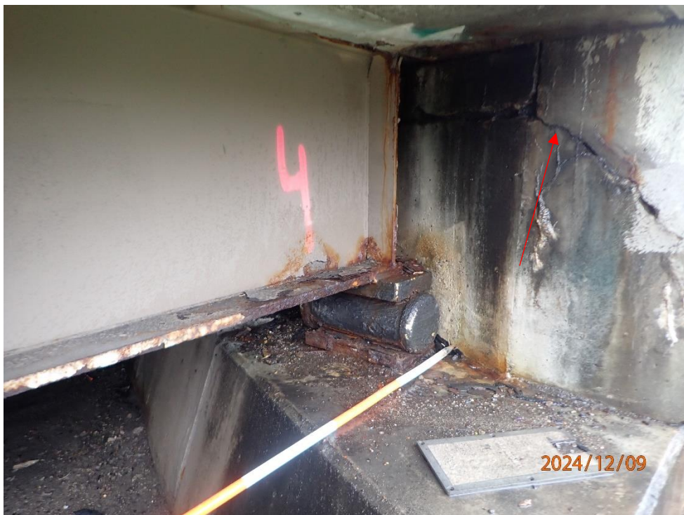
Abutment 1 backwall has wide diagonal cracking with rust staining at the west end
