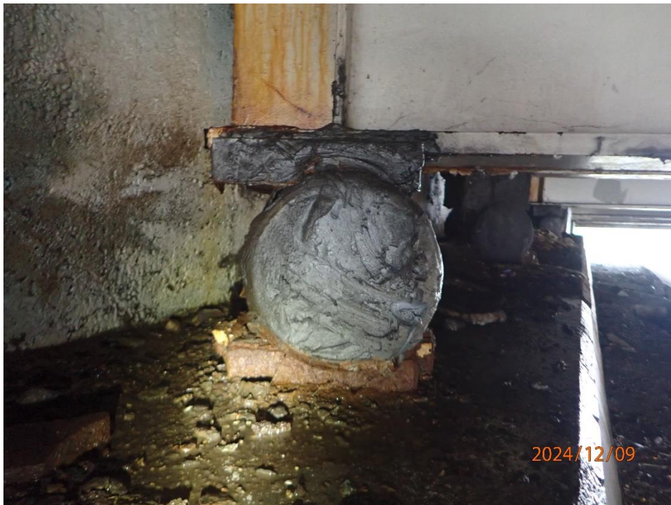
Many roller bearings are misaligned, movement is inconsistent with temperatures conditions (Beam 8 at Abutment 1 pictured)
