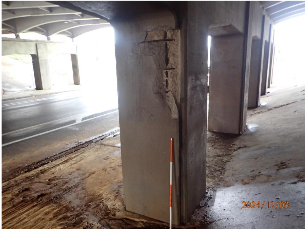
Pier 2 Column 5 has a 3.5-foot tall by 2-foot wide by 2-inch deep spall with exposed rebar in the west face
