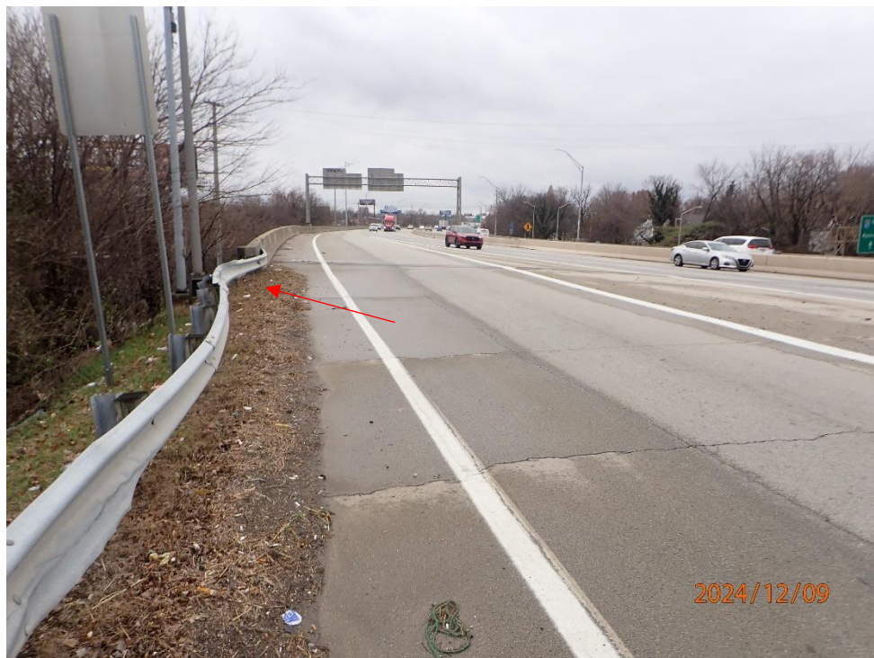
Looking south along I-65 NB. The approaching guardrail at the NE corner along the exit ramp has impact damage.
