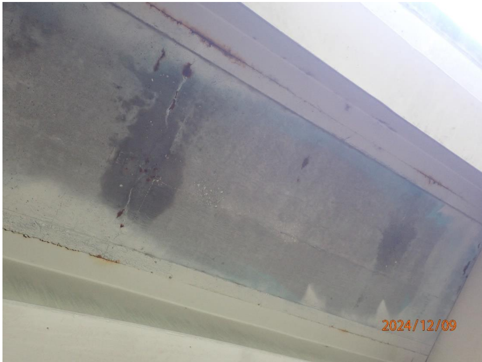
There are local areas of full depth deterioration along the longitudinal joint and Bay 1 in all three spans (Span 1 Bay 1 pictured)
