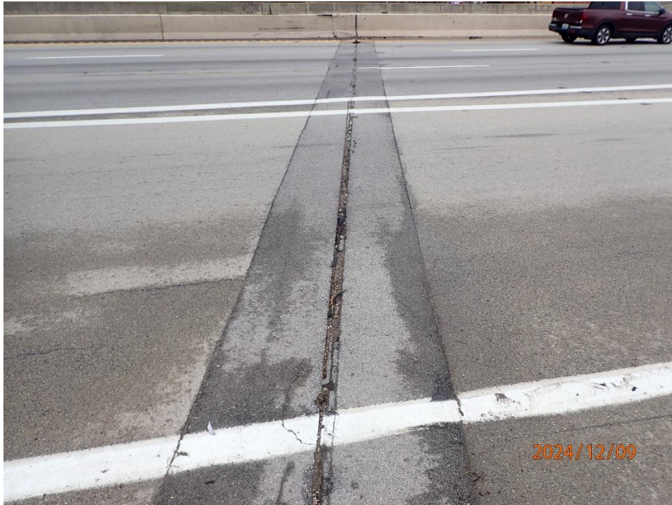
Joint over Abutment 1, NB lanes
