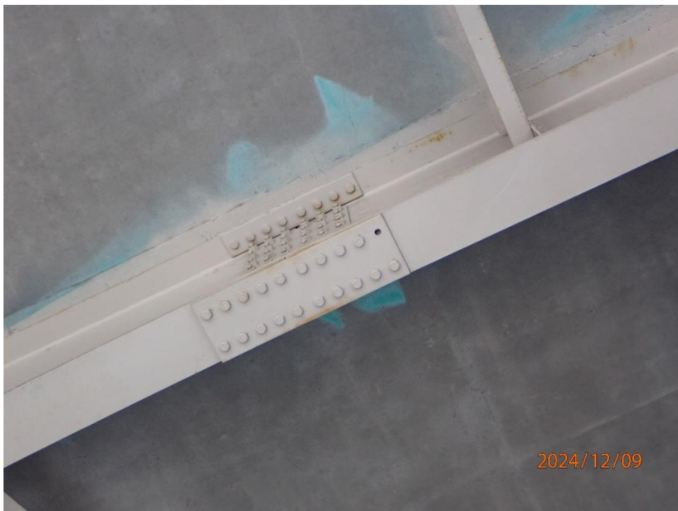
Span 2 Beam 15 splice plate near Pier 2 has one missing bolt
