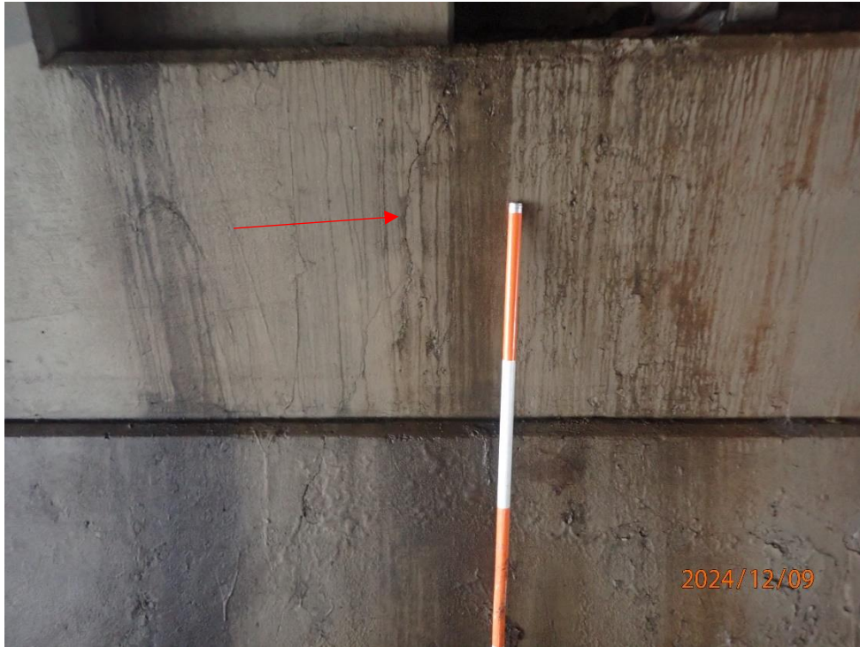
Typical vertical cracking in abutments
