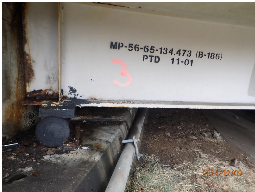
Paint stamp on Beam 1 at Abutment 4
