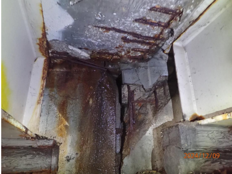
Soffit has spalling with exposed rebar at Abutment 1 at the longitudinal joint
