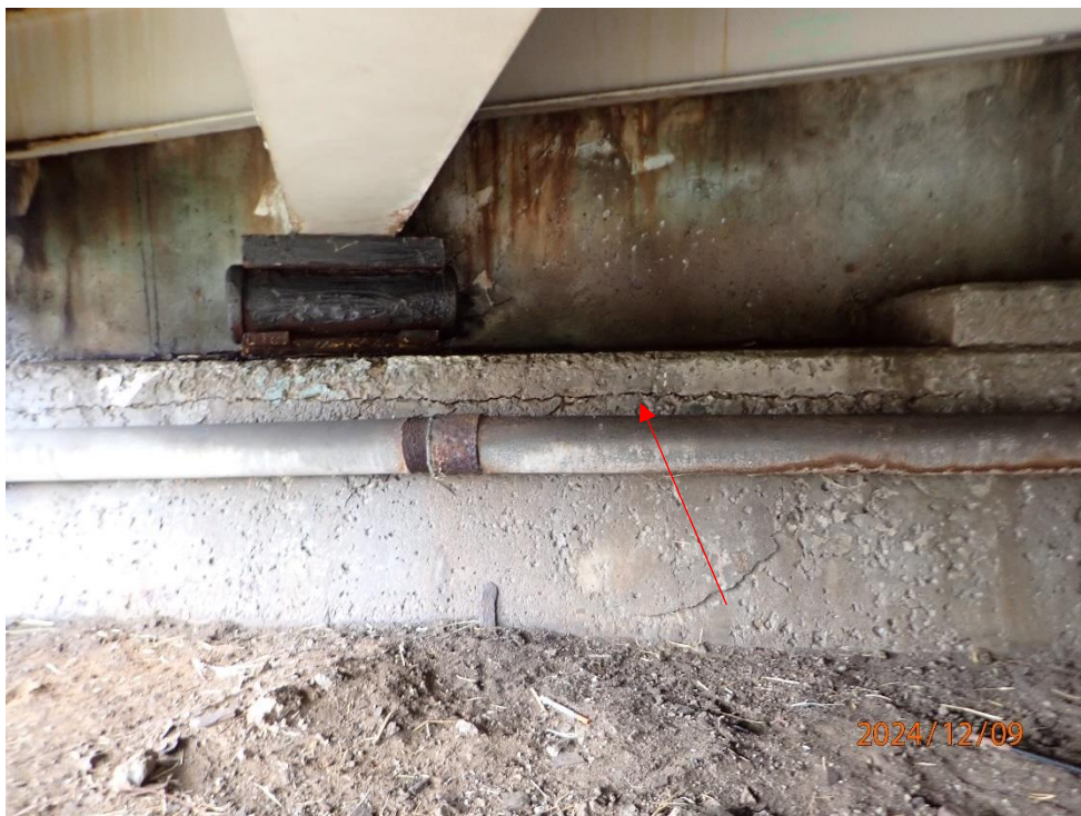
Abutment 4 has 14 feet of wide horizontal cracking at the west end
