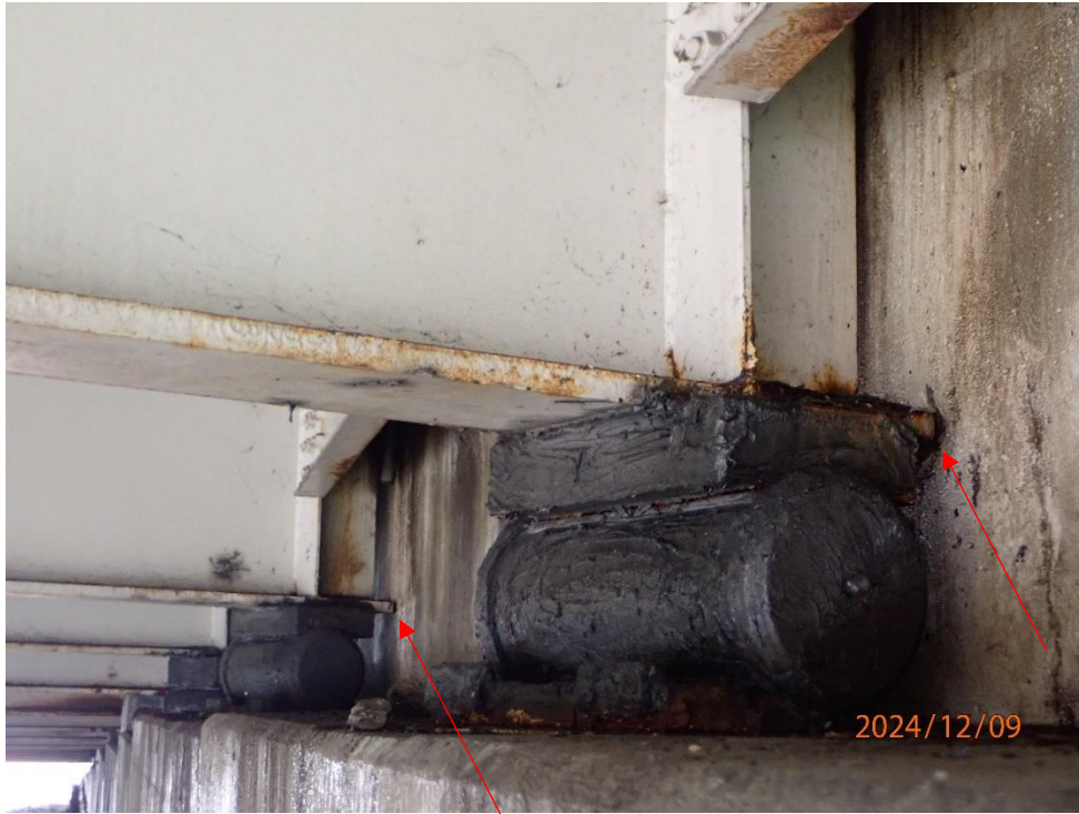
The northeast corner of Beams 13 through 15 bottom flanges are in bearing against the Abutment 4 backwall
