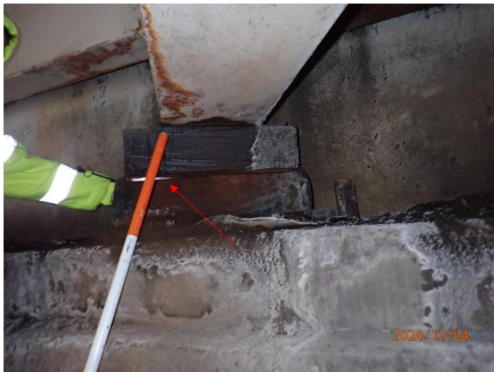
Beam 5 sole plate not in contact with the roller and moves vertically under live load at Abutment 1 (note light visible between sole plate and roller)
