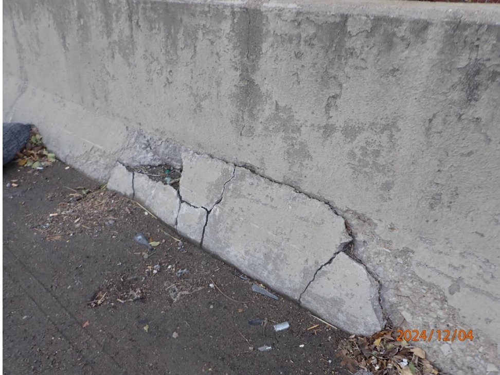
The west SB rail has an area of wide delamination cracking and spalling in Span 1.
