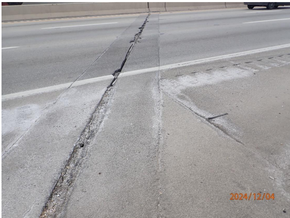
Joint over Abutment 4, NB lanes
