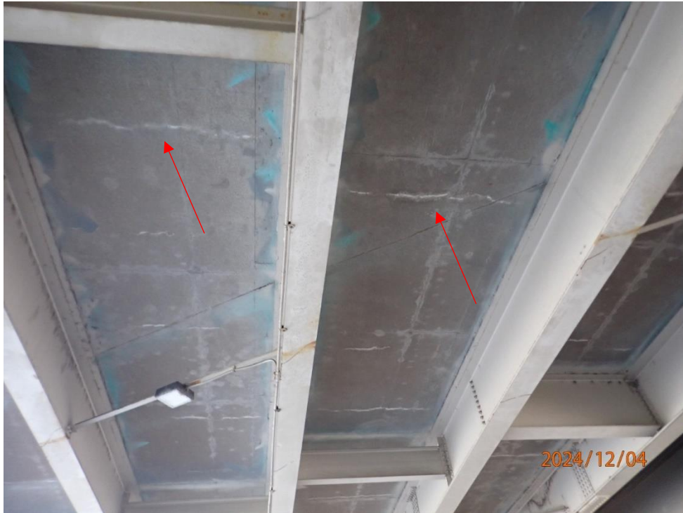
Soffit has transverse cracks, some with efflorescence
