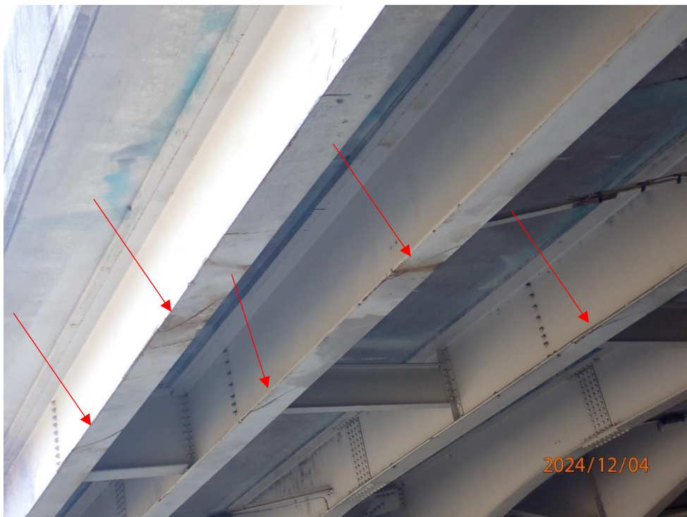
Span 2 Beams 9-14 have shallow scrapes/gouges with surface corrosion (Beams 12-14 pictured)
