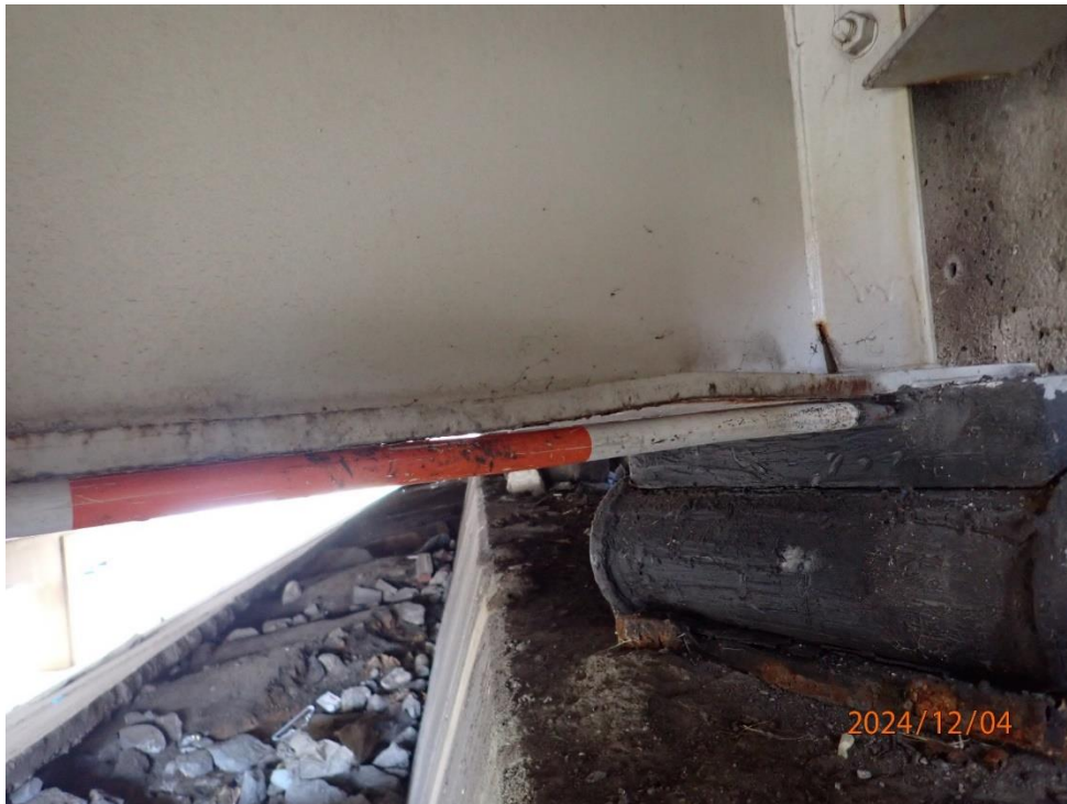
Beam 13 bottom flange has a 1.5'L area of minor distortion at Abutment 4
