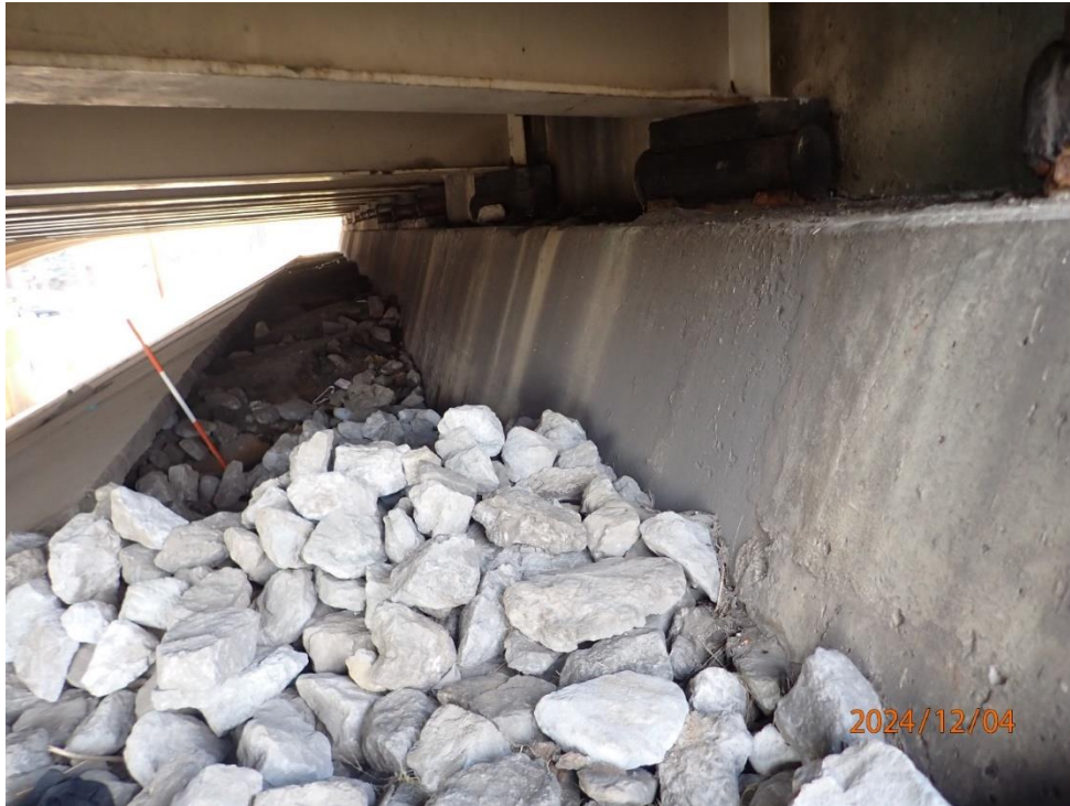
Abutment 4. Note rip rap in place at the NE corner and undermining along the top of Abutment 4 slope protection.
