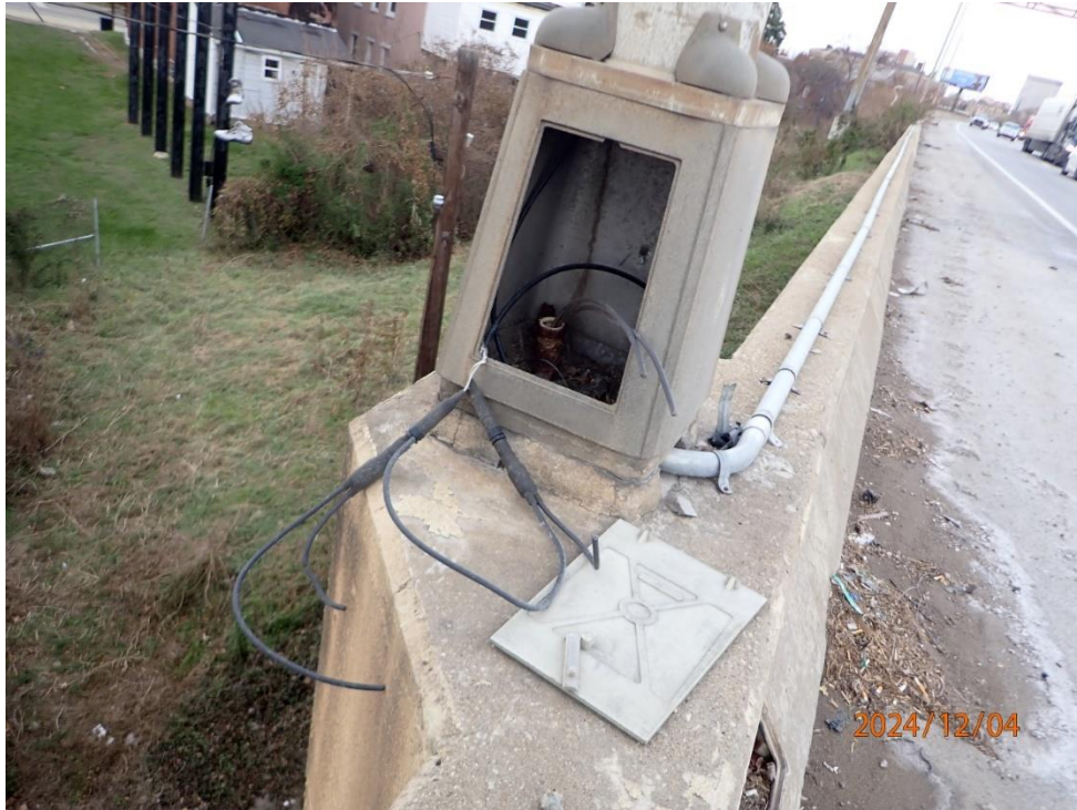
SB west rail has a light fixture with missing cover plate and disconnected wiring near Pier 3
