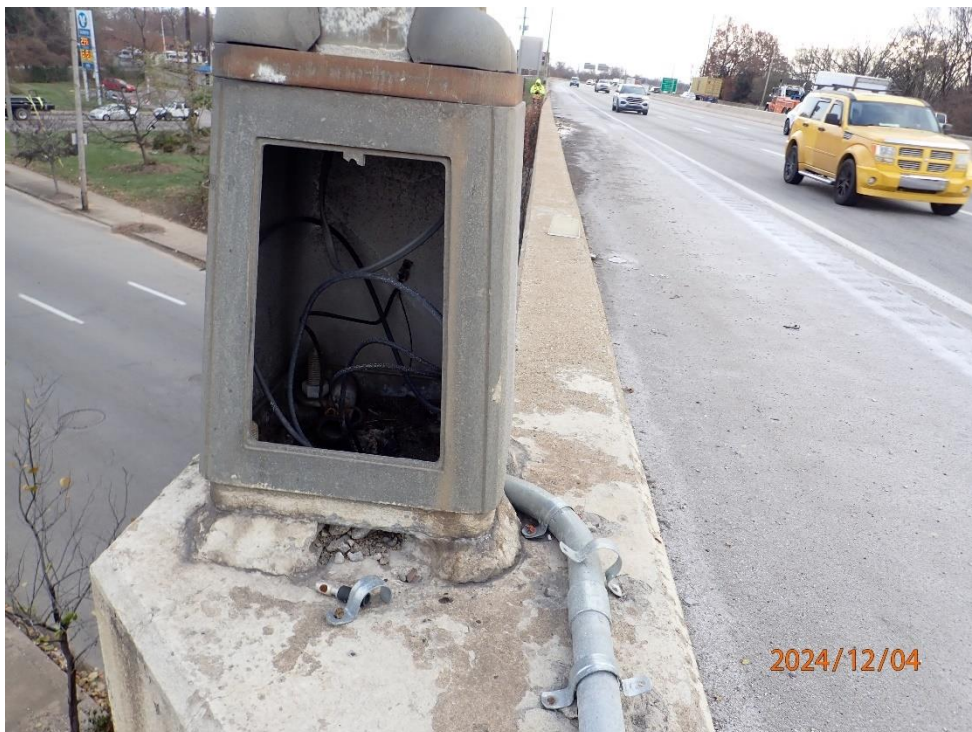
NB east rail has a light fixture with missing cover plate near Pier 3
