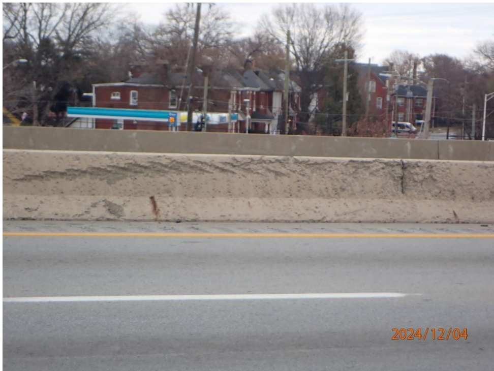
The SB median barrier has a large area of shallow scrapes/spalls near Pier 2
