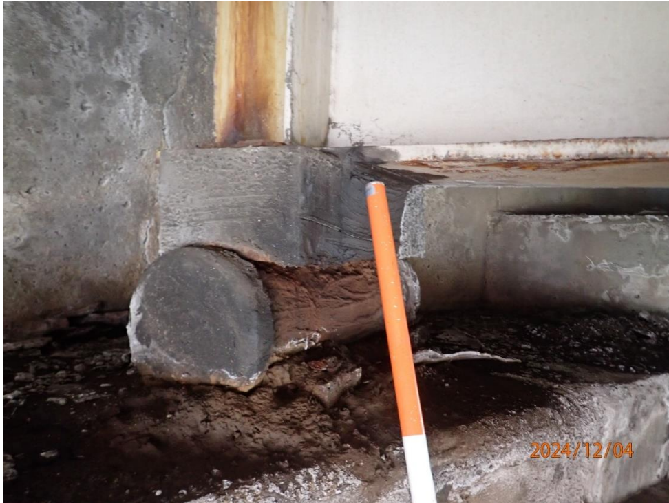
Rollers and masonry plates typically have flaking corrosion, and some areas have section loss (Beam 5 at Abutment 4 pictured)
