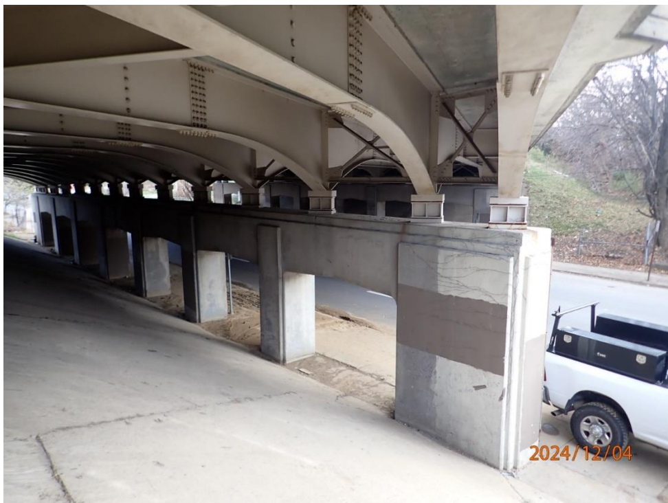
Soffit has transverse cracks, some with efflorescence
