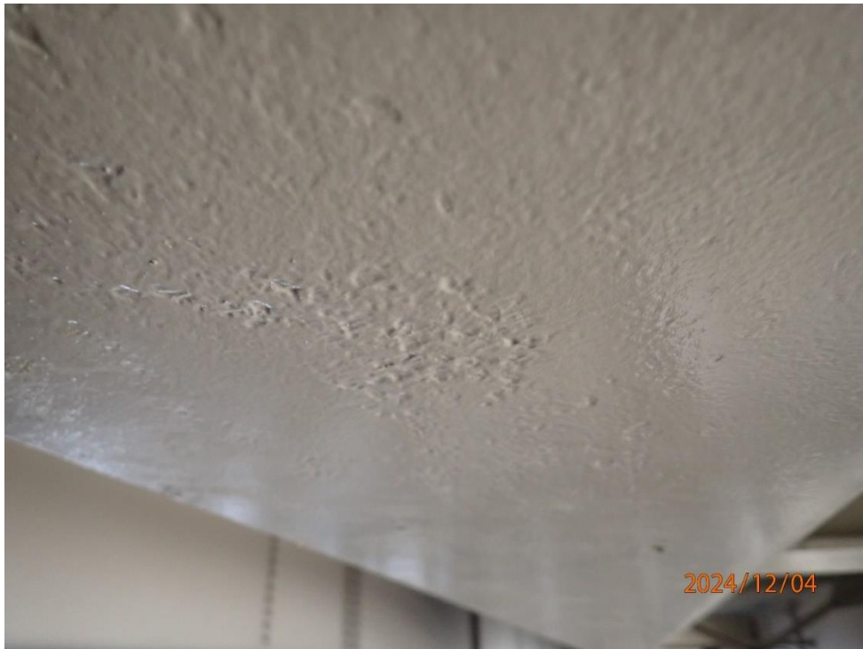
Bottom face of bottom flanges in non-haunch sections typically have paint over minor pitting
