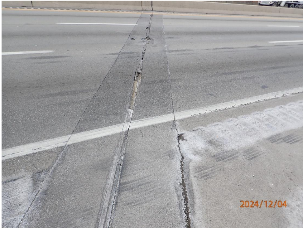
Joint over Abutment 1, NB lanes
