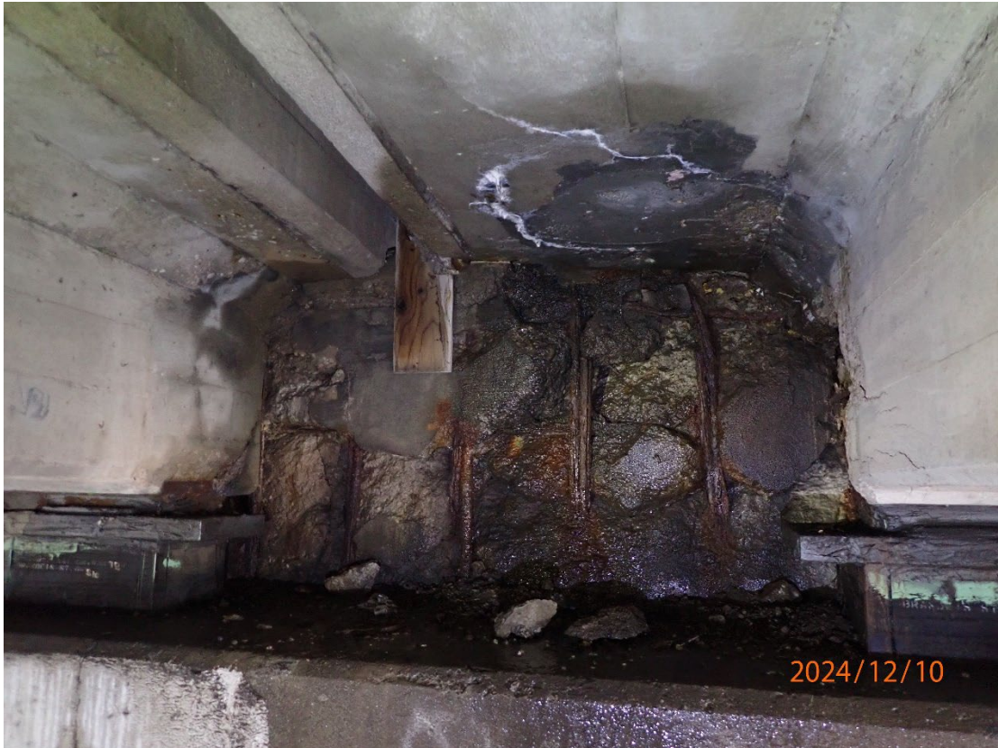
Heavy spalling with exposed rebar in the Abutment 1 backwall under the longitudinal joint in Bay 9
