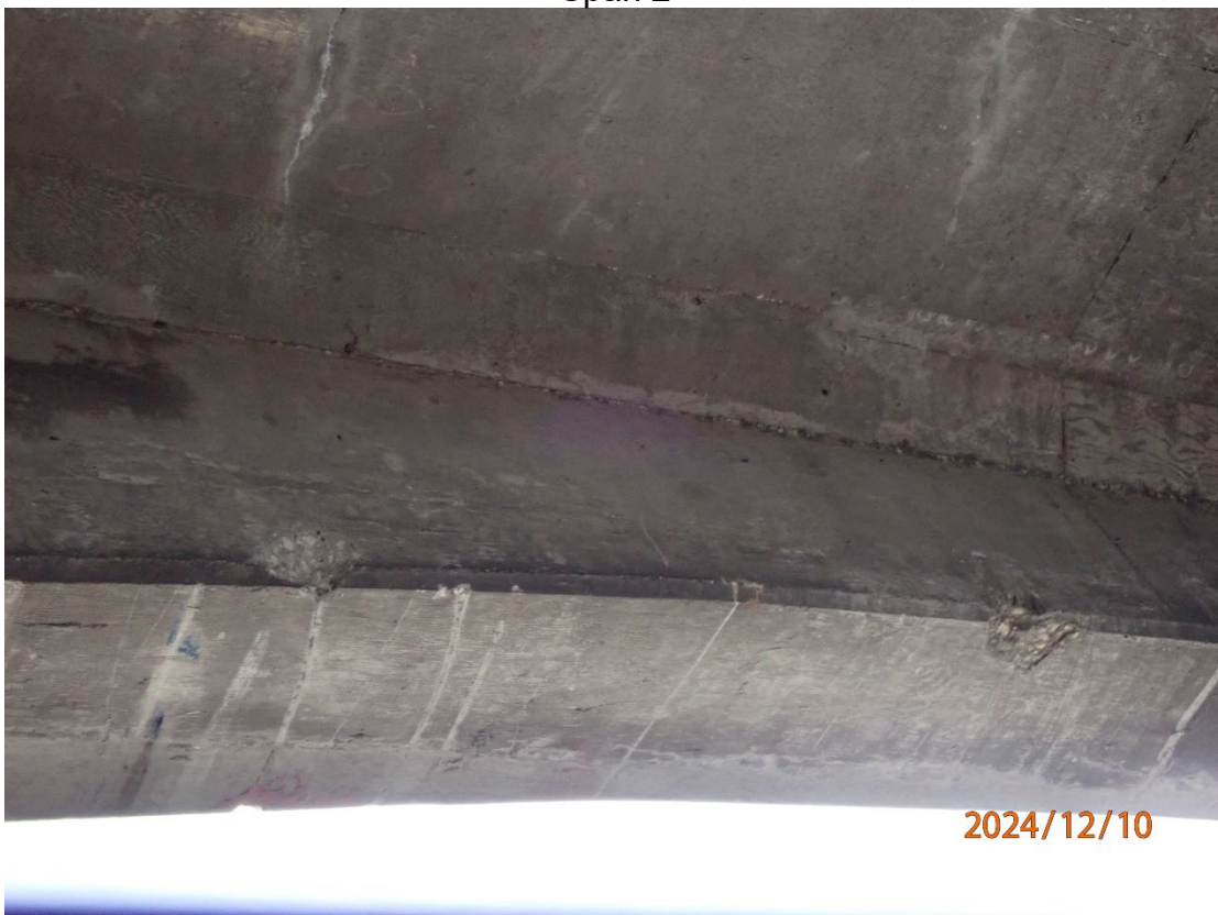
Scraping with edge spalling in the bottom face of Beam 18 near the 3/4 point of Span 2
