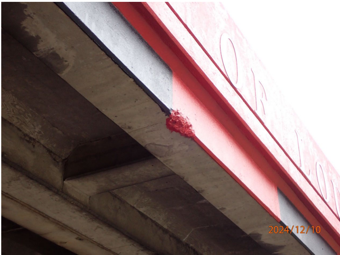
Spall in the bottom north edge of Beam 18 near midspan of Span 2
