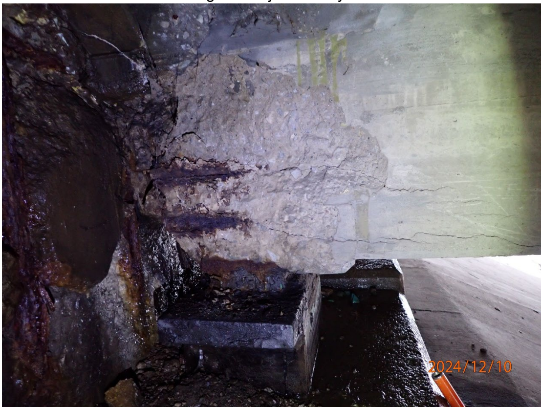
Spalling with exposed rebar and horizontal cracking in the east face of Beam 9 at Abutment 1
