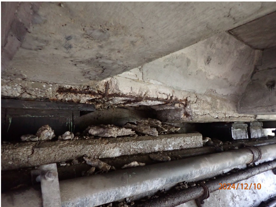
Spalling with exposed steel in the Bay 15 diaphragm at Abutment 4
