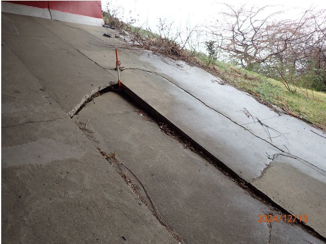
Undermined and settlement concrete slope protection near the west end of Span 1
