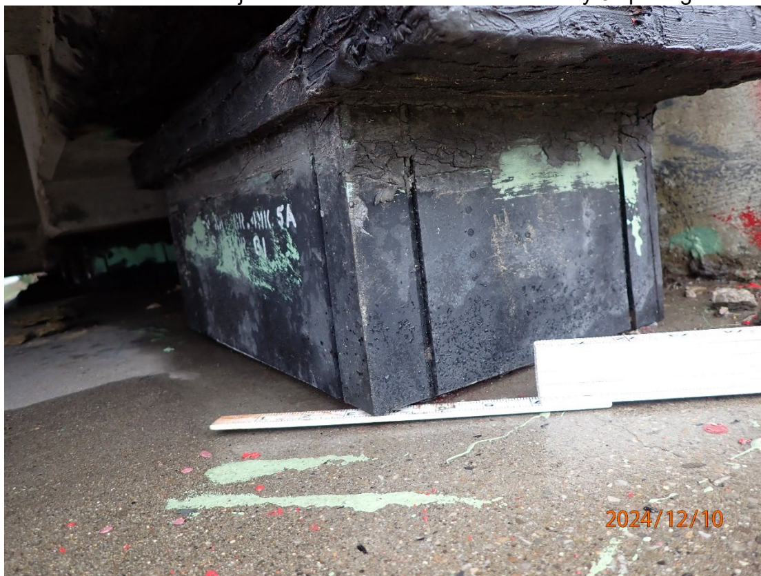
Up to a 1/4" gap under the northwest corner of the Beam 1 bearing pad at Abutment 1
