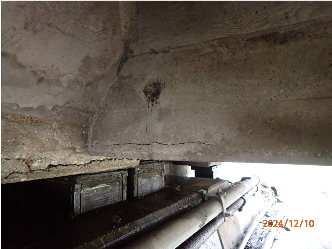
2' wide horizontal crack in the west face of Beam 16 at Abutment 4
