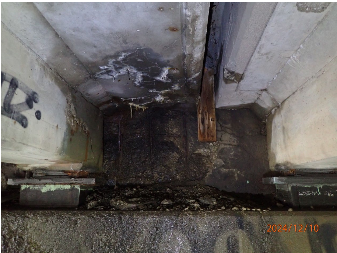
Heavy spalling in the Abutment 4 backwall along with full depth deterioration along the soffit in Bay 9
