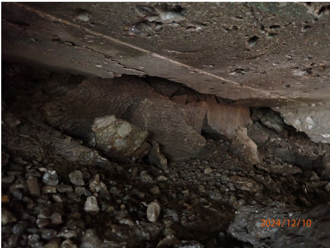
Heavy spalling in the Abutment 4 backwall. Bay 4 shown
