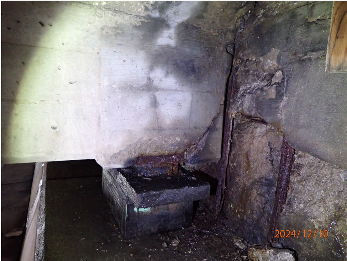
Spalling in the west face of Beam 10 at Abutment 1
