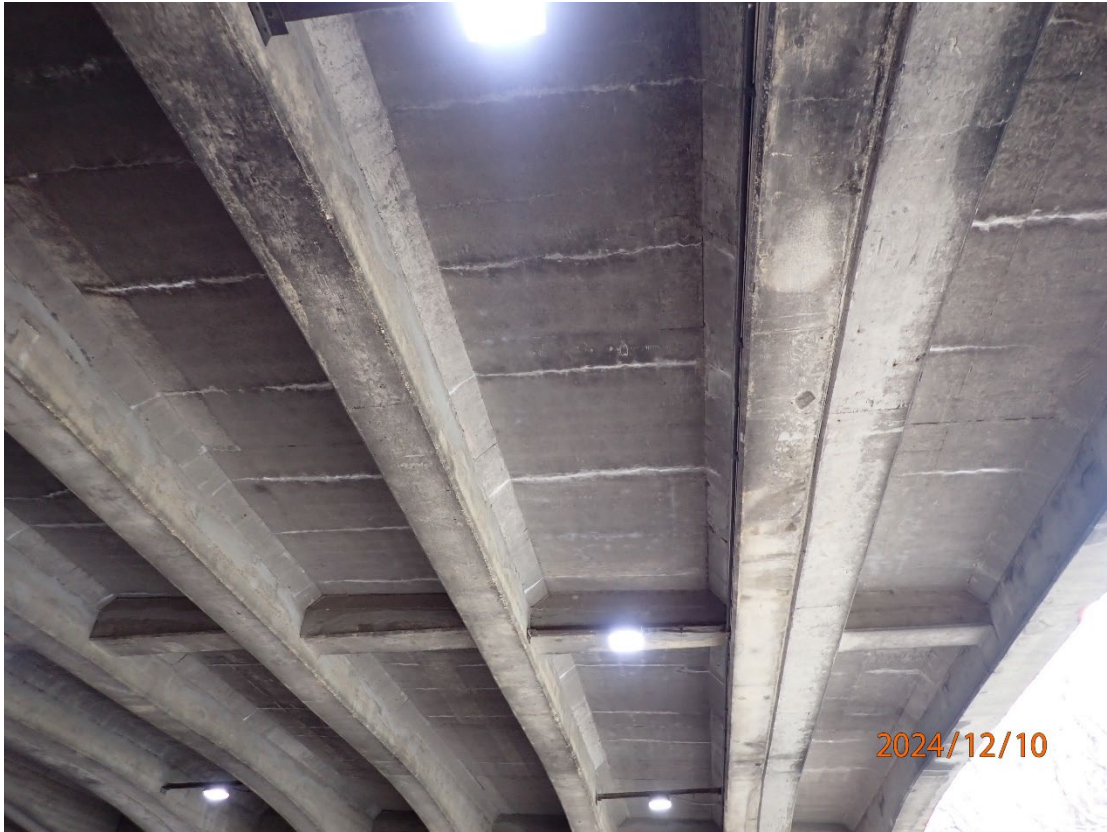
Typical transverse cracking with efflorescence in the Span 2 soffit
