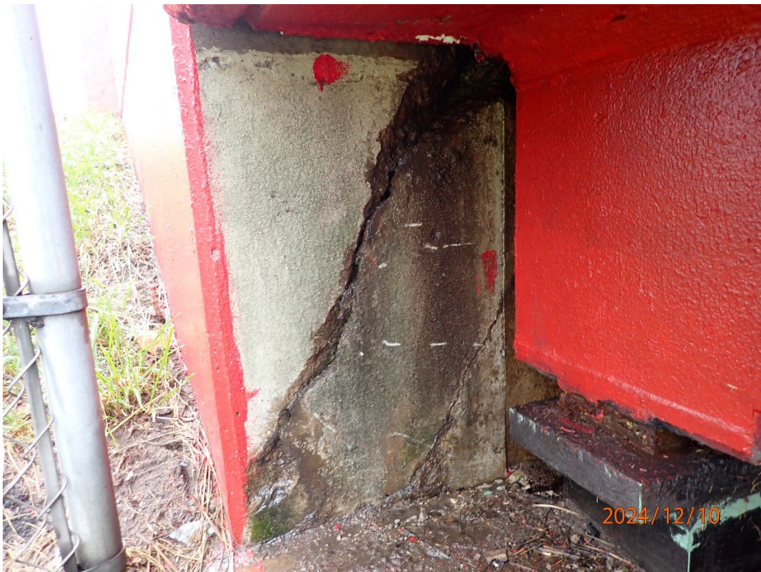
Wide diagonal crack with edge spalling in the east end of the Abutment 1 backwall
