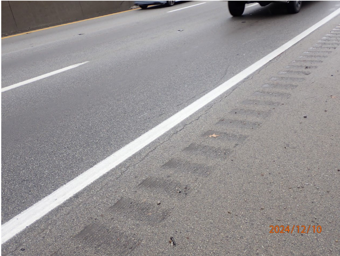
Full length longitudinal crack along the west southbound shoulder edge line. Span 1 shown
