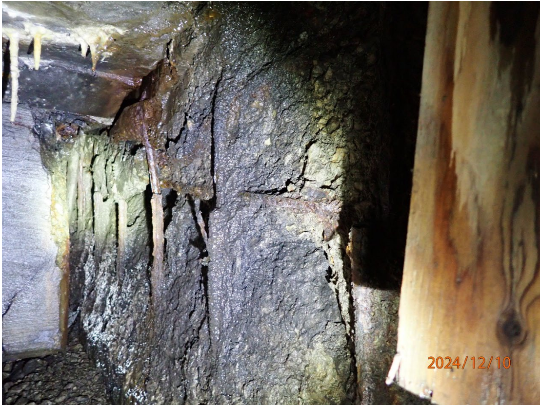
Heavy spalling with exposed and broken rebar in the Abutment 4 backwall. Bay 9 shown
