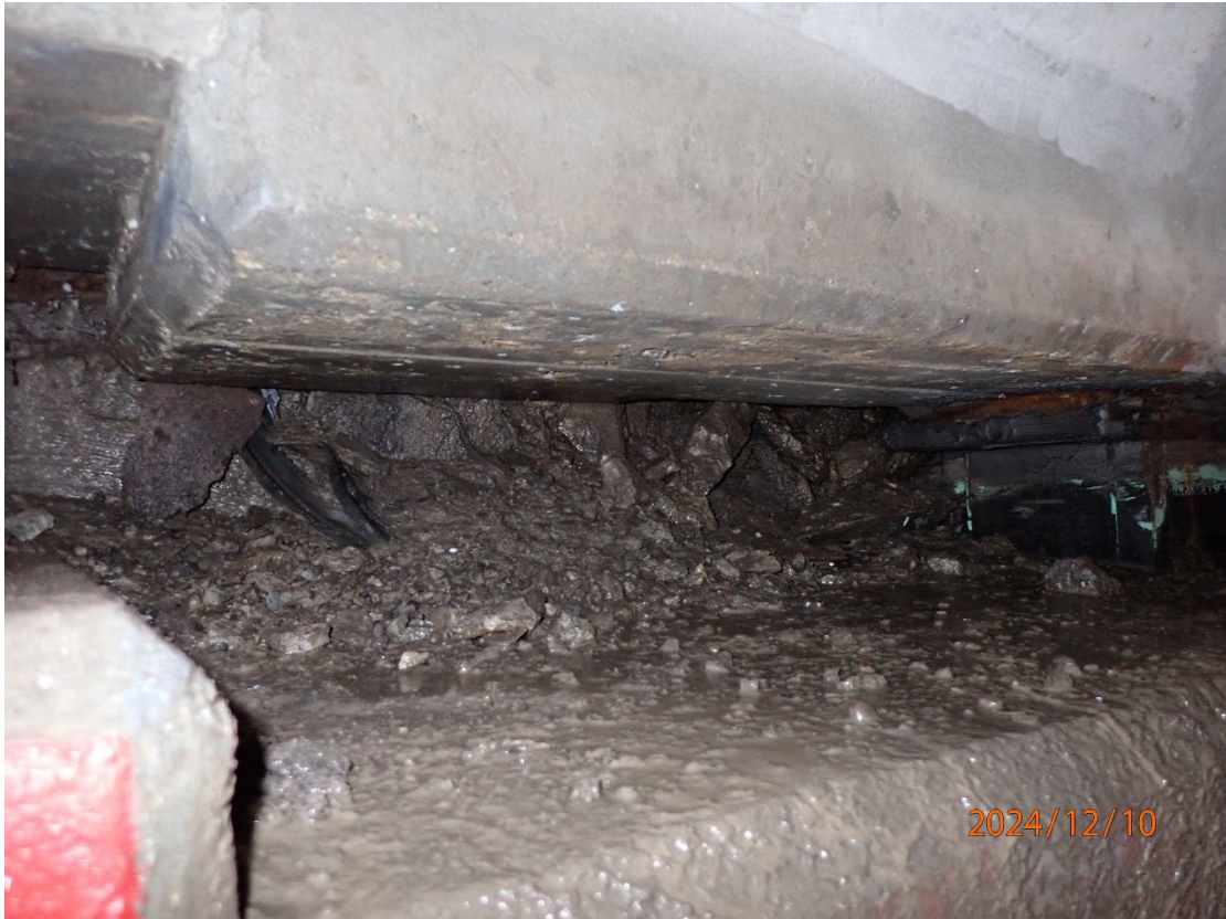
Heavy spalling in the Abutment 4 backwall. Bay 3 shown
