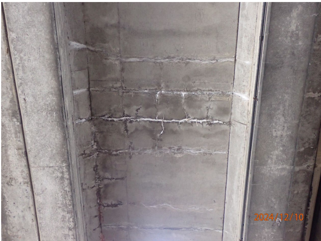
Area of full depth deterioration in Bay 8 of Span 2 near the 3/4 point
