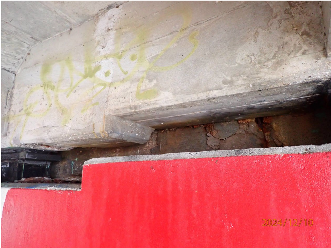
Areas of spalling with exposed rebar in the Abutment 1 backwall. Bay 3 shown
