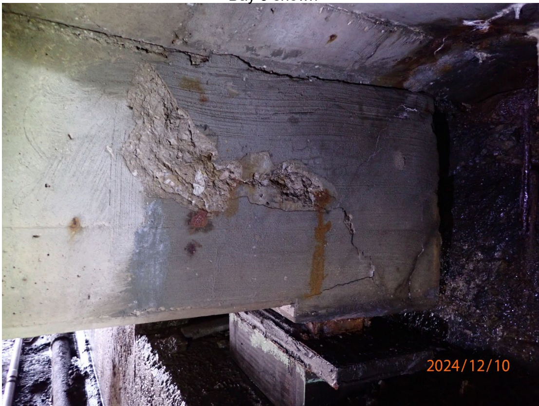
Unsound patching and spalling in the east face of Beam 9 at Abutment 4
