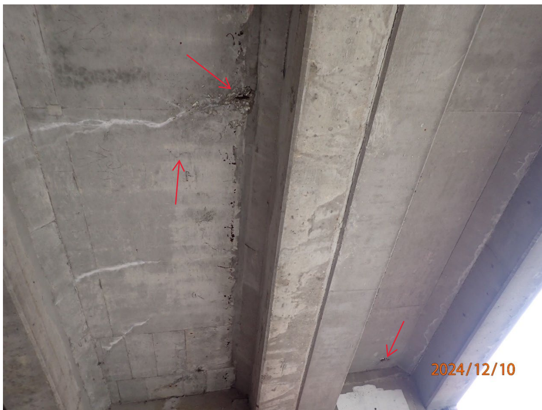
Spalling with exposed rebar in the underside of Bays 1 & 3 near Abutment 1. Note there is adjacent delaminations next to the Bay 3 spalling
