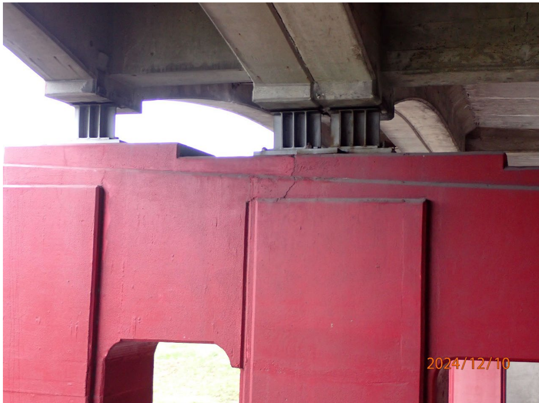
Wide cracking in the south face of the Pier 2 cap under Beam 2
