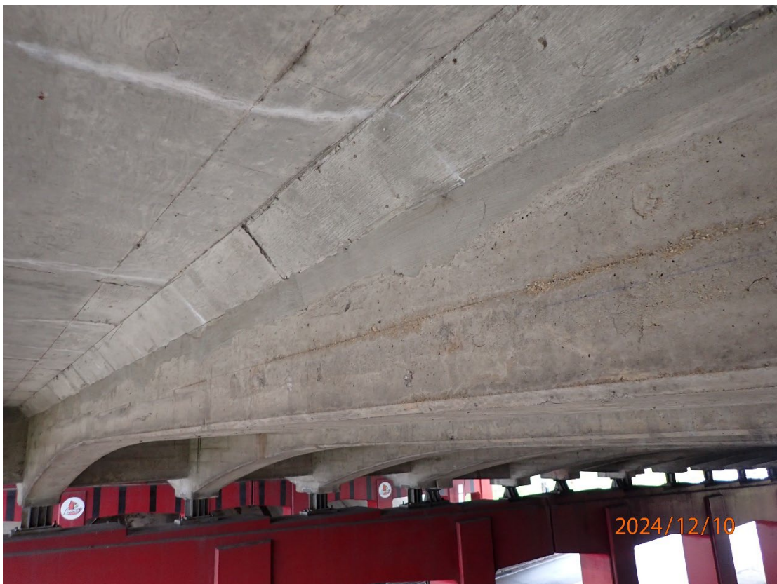
Typical patching along the top of the beams. Beam 4 in Span 1 shown
