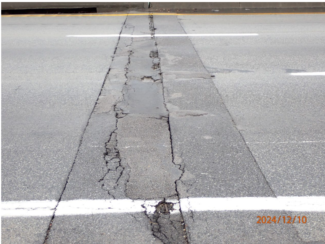
Soundbound joint over Abutment 4. Note the areas of spalling and patching
