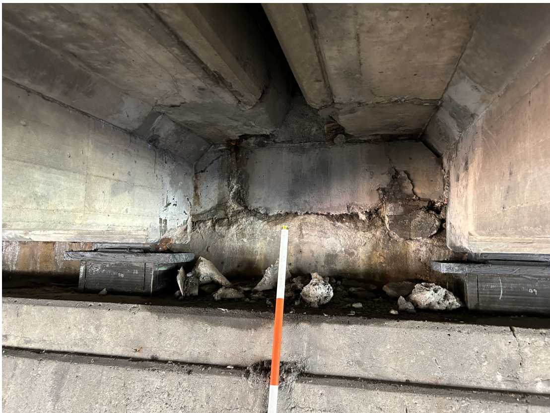
Failing patching in the backwall of Abutment 1 at the I-65 centerline.
