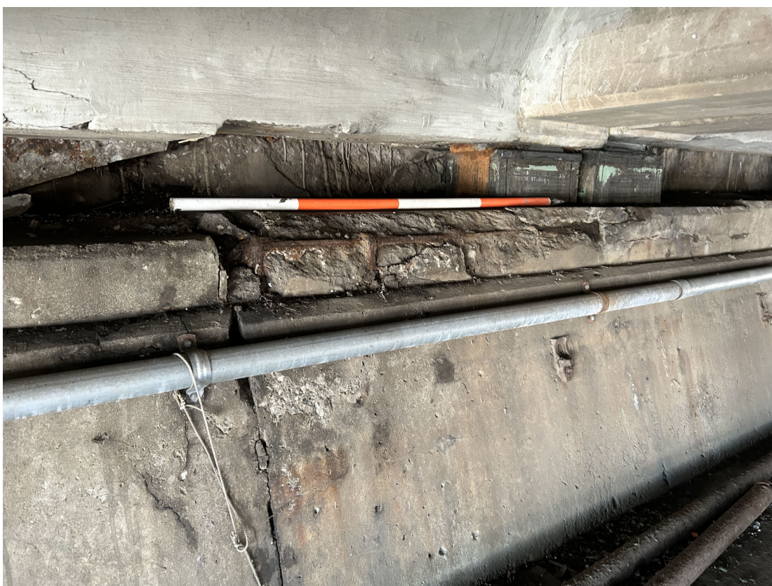
Abutment 4 is spalling at the ends of the original length. Spall between Girders 6 and 7 shown.
