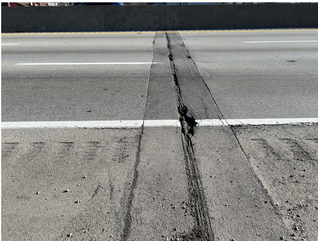
Asphalt plug joint over Abutment 1 SB
