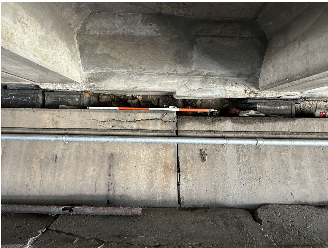
Wide cracking in Abutment 4 seat between Girders 12 and 13.
