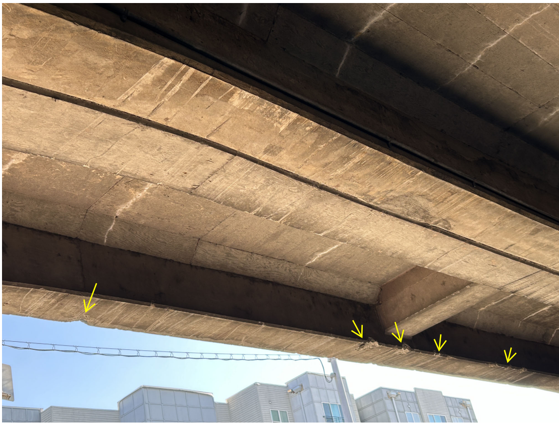
Girder 18 in Span 2 has impact spalls and scrapes.
