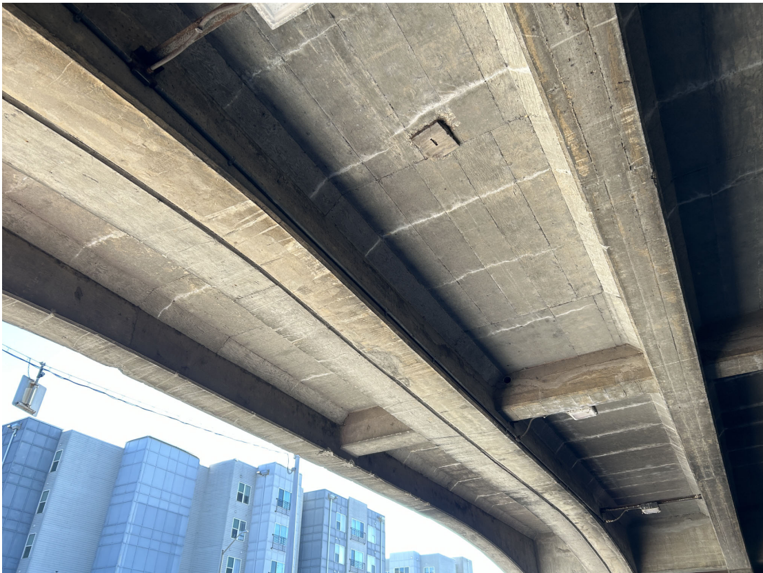
East end of Span 2 soffit showing transverse cracks with efflorescence spaced less than 3 feet apart.
