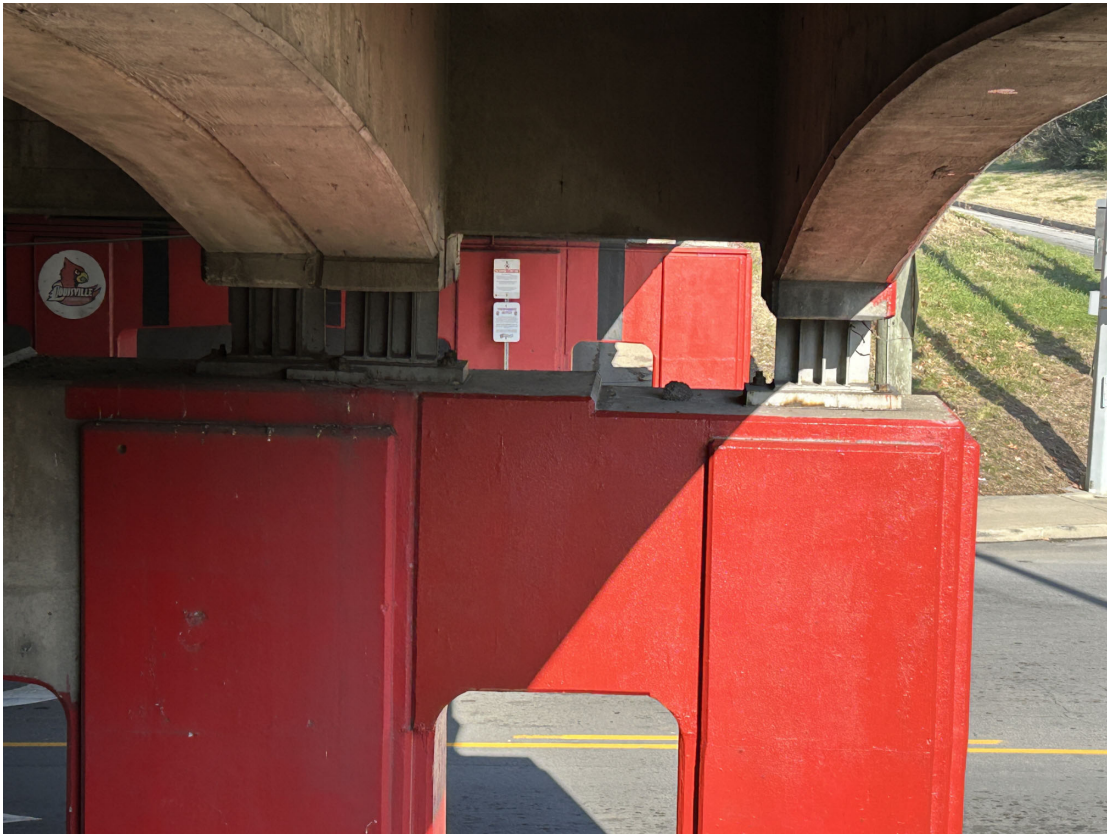
Typical fixed bearing at Pier 2 with some surface corrosion.
