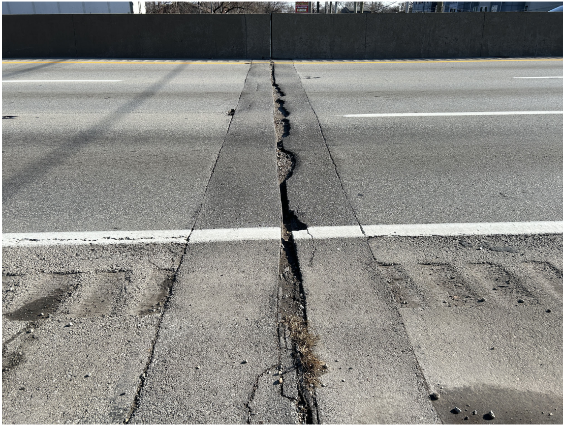
Asphalt plug joint over Abutment 4 SB
