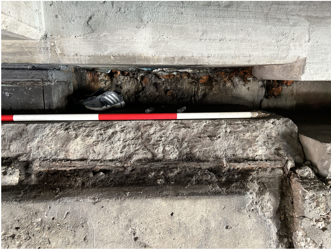
Close-up of deep spalling in Abutment 1 west of Girder 7 at end of original abutment.
