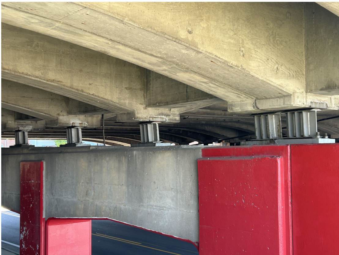
Pier 3 bearings are expanded towards Abutment 4, inconsistent with ~32 degree weather.
