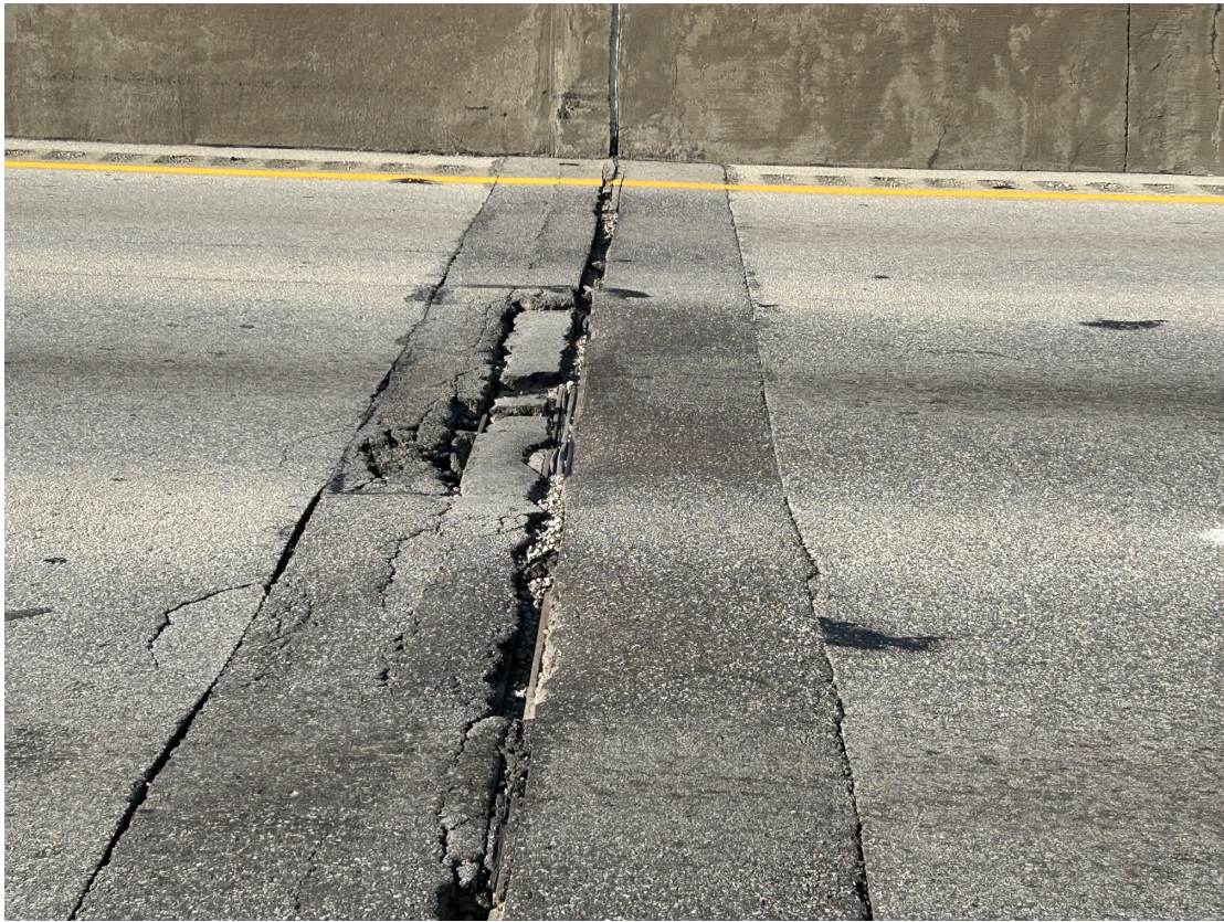
Joint and pavement over the Abutment 1 backwall in the center NB lane is breaking up.
