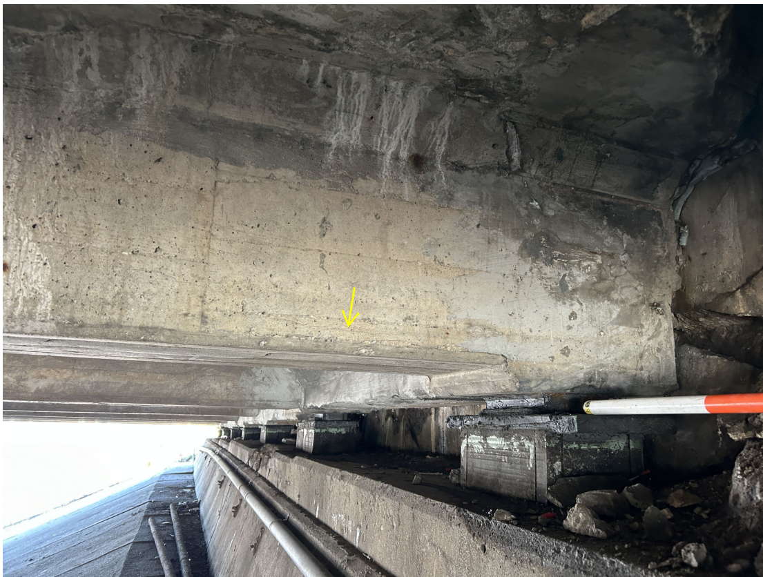
Girder 9 has a longitudinal crack in the east face near Abutment 4.
