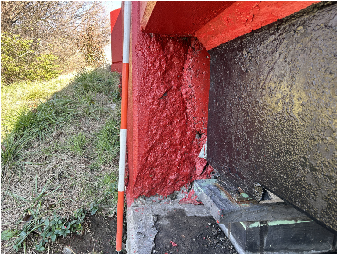
Spalling and cracking at the west end of the Abutment 4 backwall.
