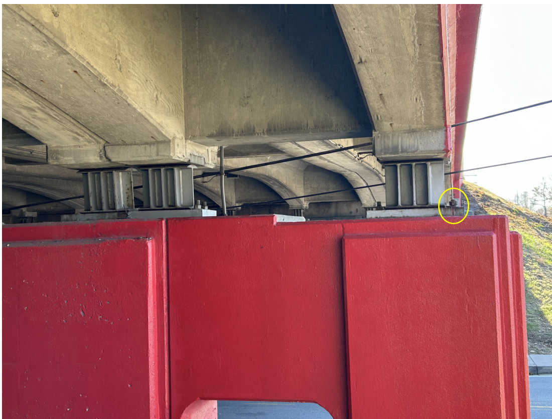
Pier 3-Girder 1 bearing has a loose nut on the NW anchor bolt.
