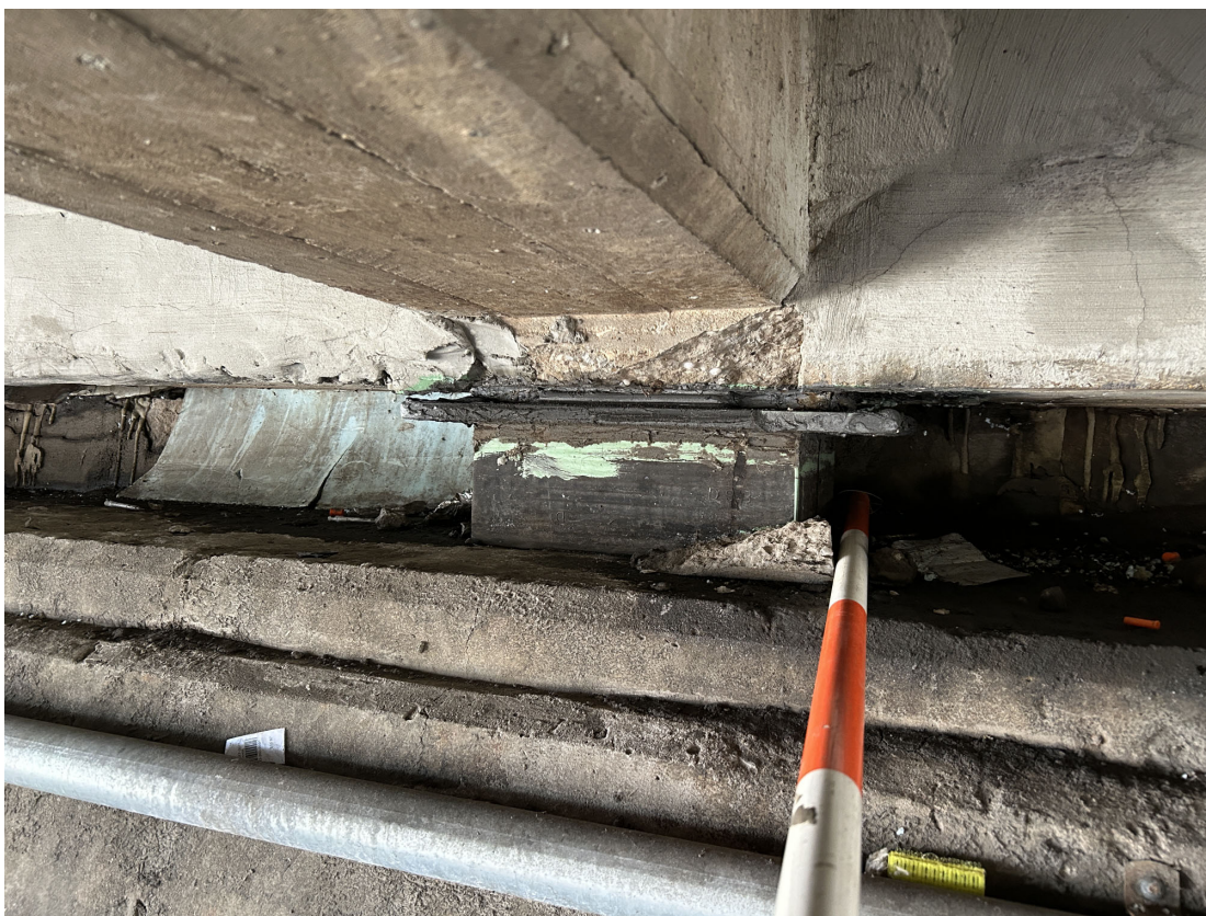
Girder 5 has a spall at the Abutment 4 bearing.
