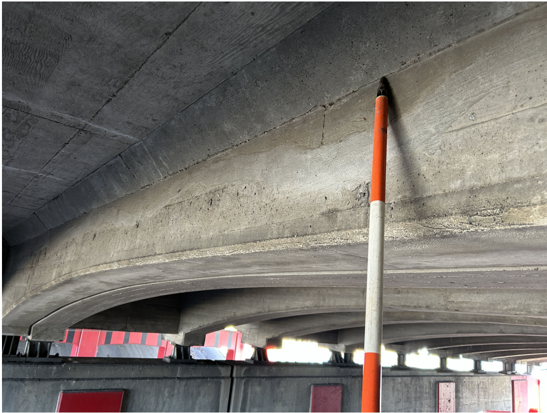
Several girders have sound concrete patching along the top of the webs in all three spans. Example along Girder 7 in Span 1.
