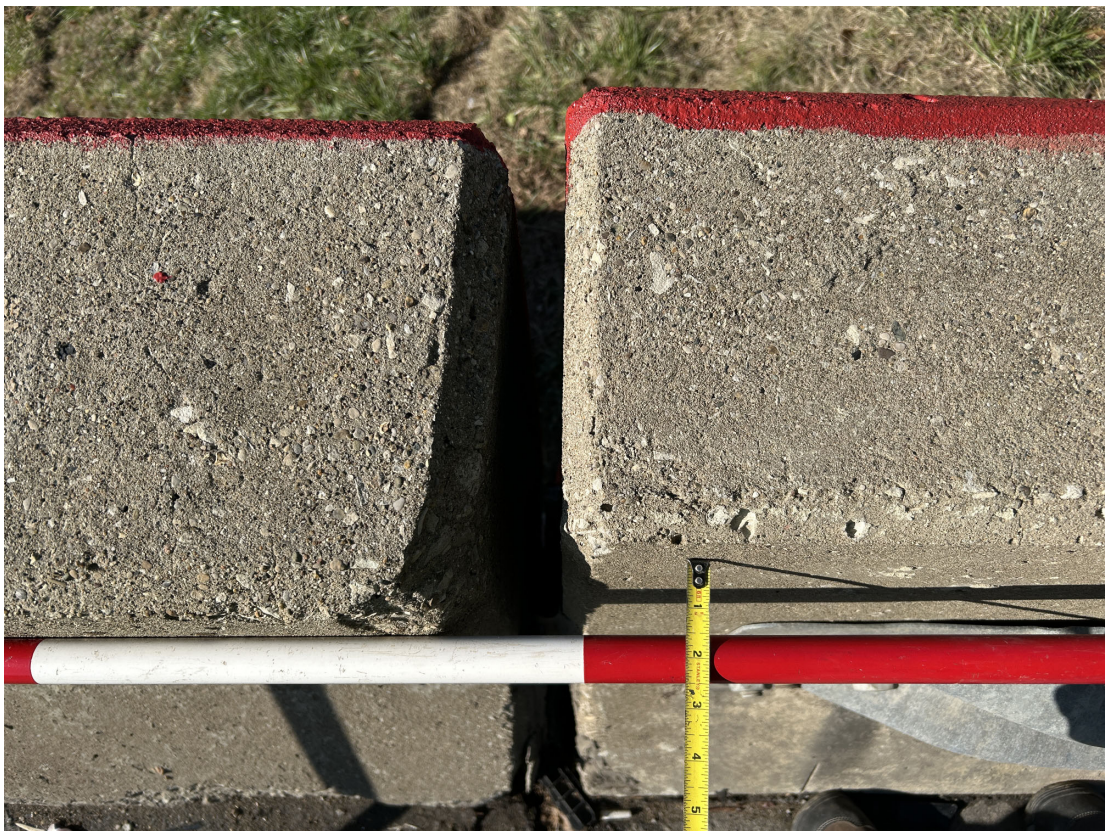
NW wingwall is tilted out 1.5 inches at the top of the rail.
