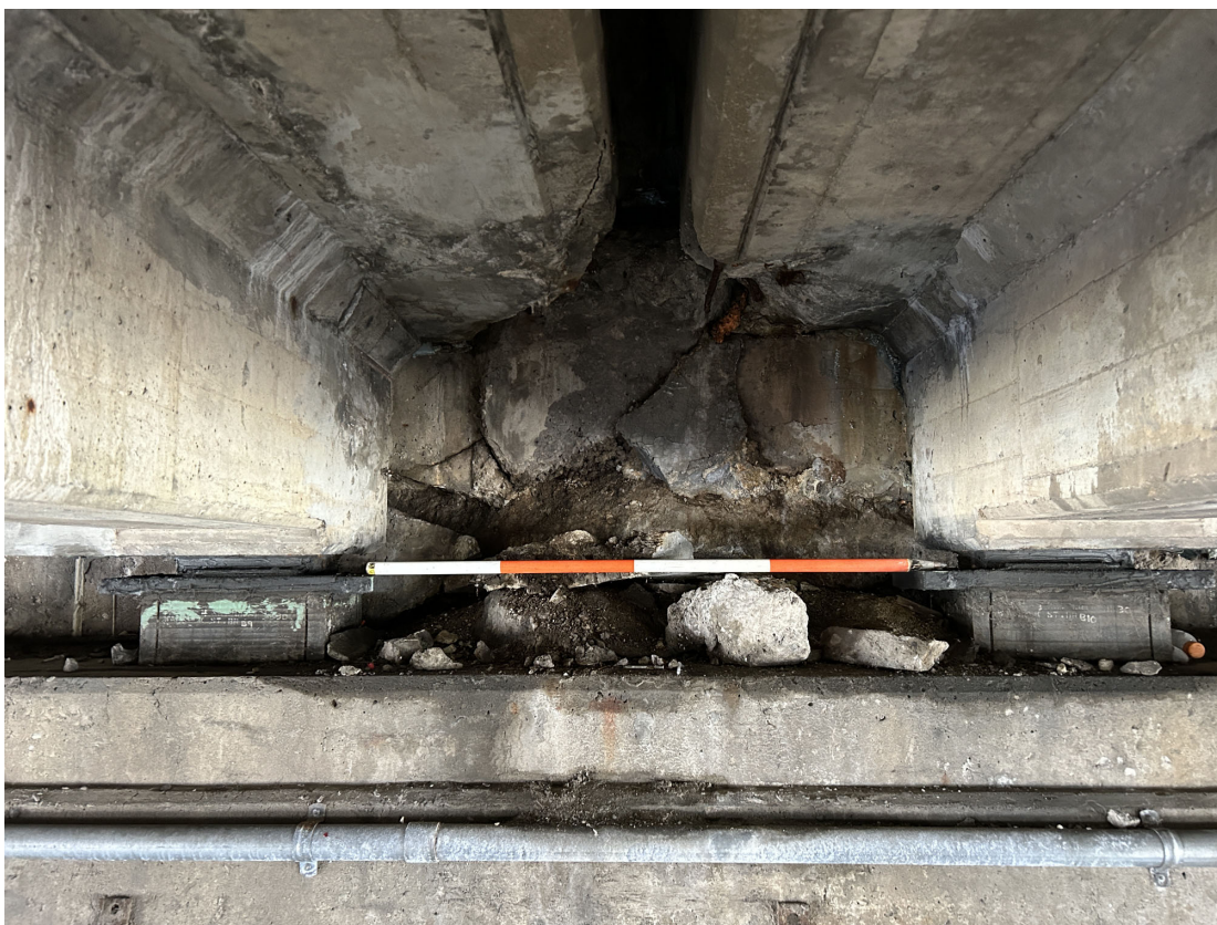
Spalling and failing patch in the Abutment 4 backwall at the I-65 centerline.
