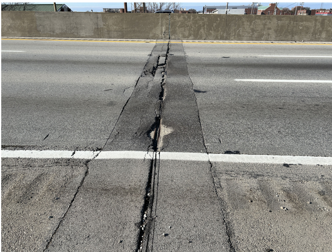
Asphalt plug joint over Abutment 1 NB
