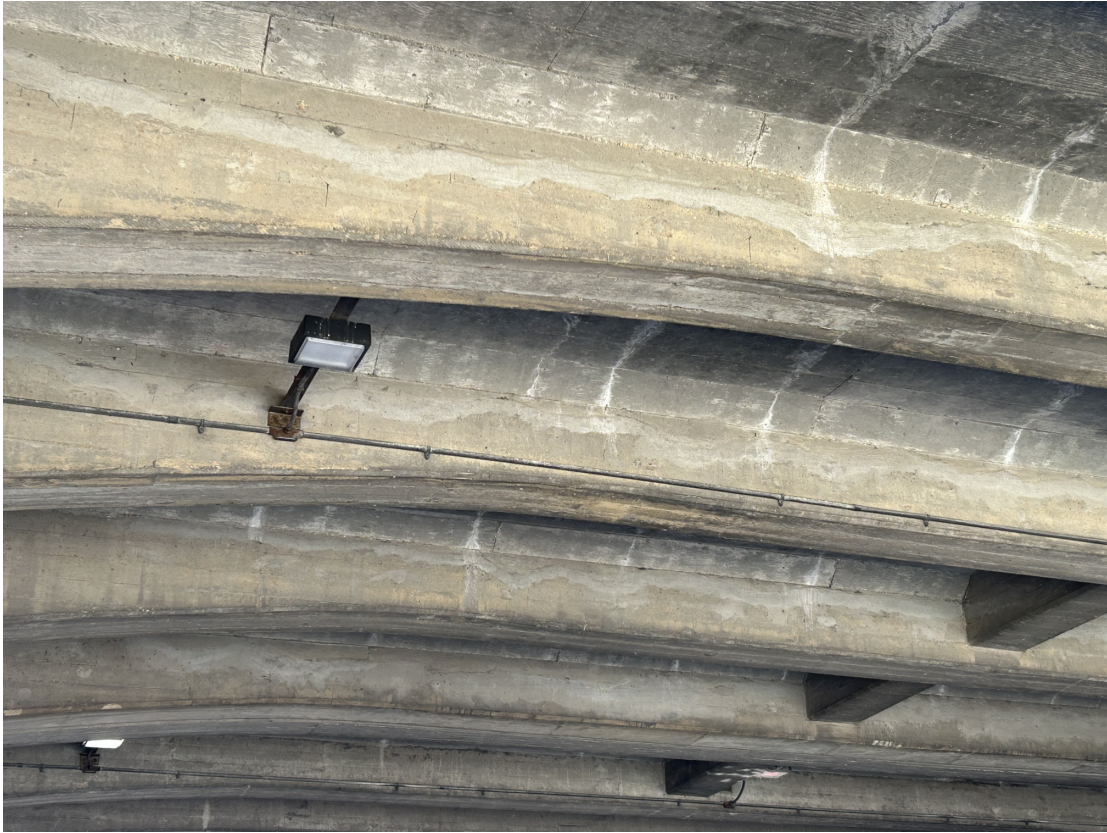
Sound concrete patches along the tops of the girder webs in Span 2, plus transverse cracking in the deck soffit.
