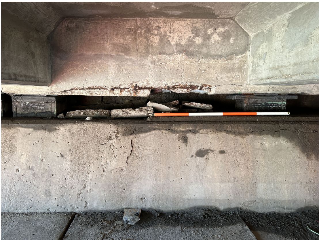
End diaphragms have numerous spalls and cracks. Abutment 1 end diaphragm between Girders 15 and 16 shown.
