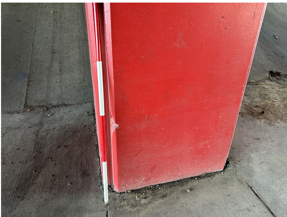
Pier 3-Column 7 has a small spall near the bottom.
