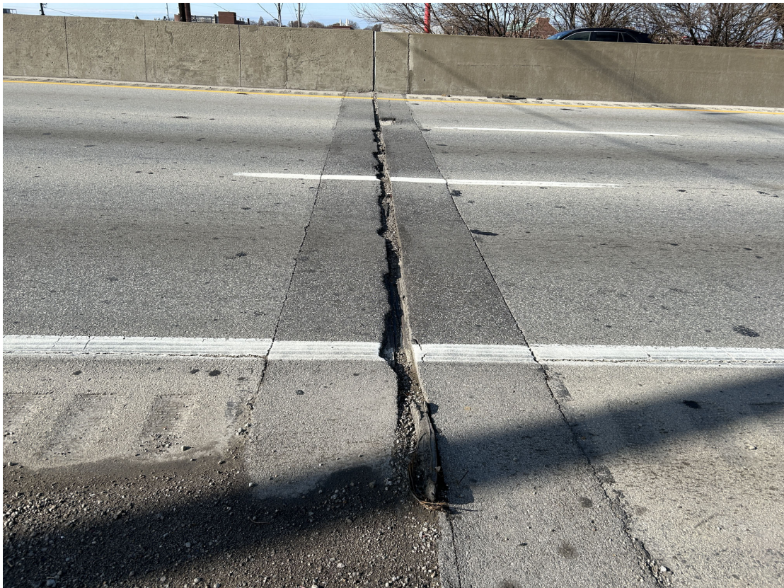
Asphalt plug joint over Abutment 4 NB
