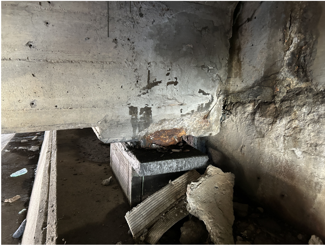
Girder 10 has a spall at the bearing at Abutment 1 end.
