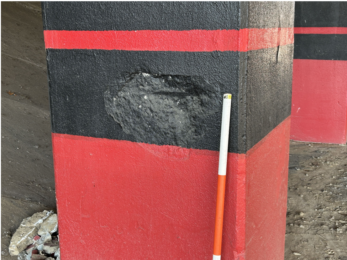
Pier 2-Column 7 painted over spall.
