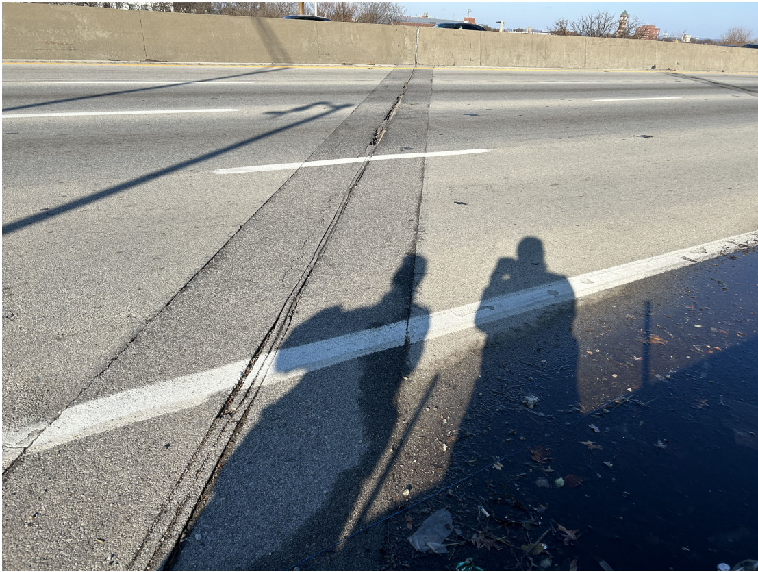
Asphalt plug joint over Abutment 1 NB.
