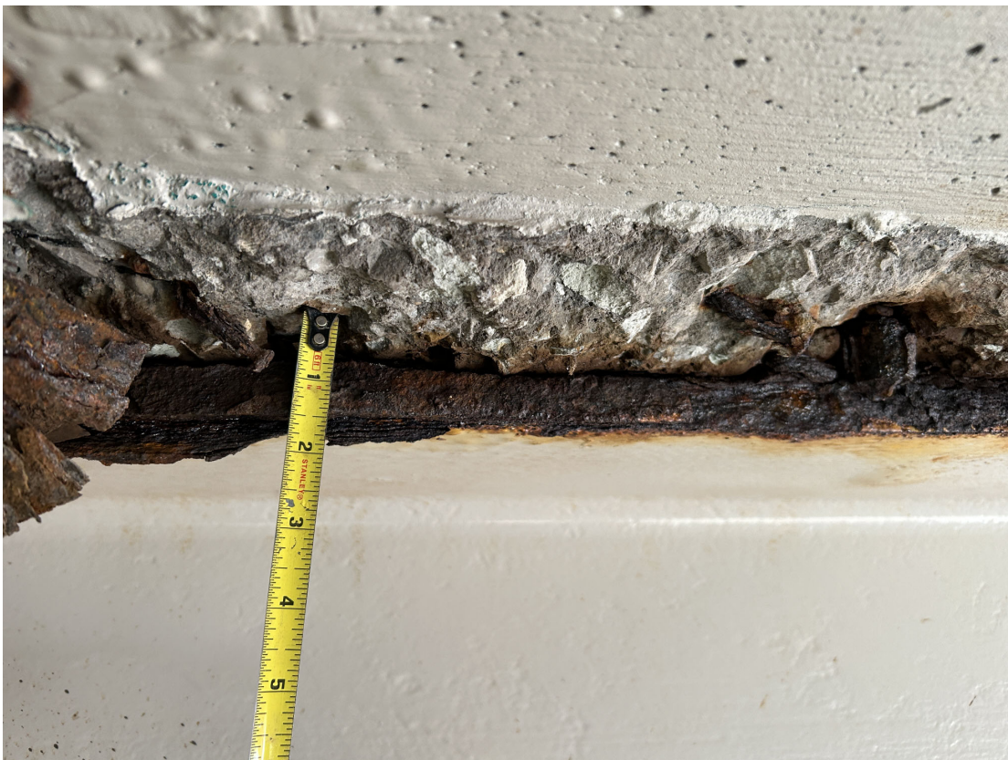
Deck moves independent of girders at several locations along abutments. Gaps between the deck and top flanges, along with haunch spalls are present at these locations. Example at Girder 14 at Abutment 1.
