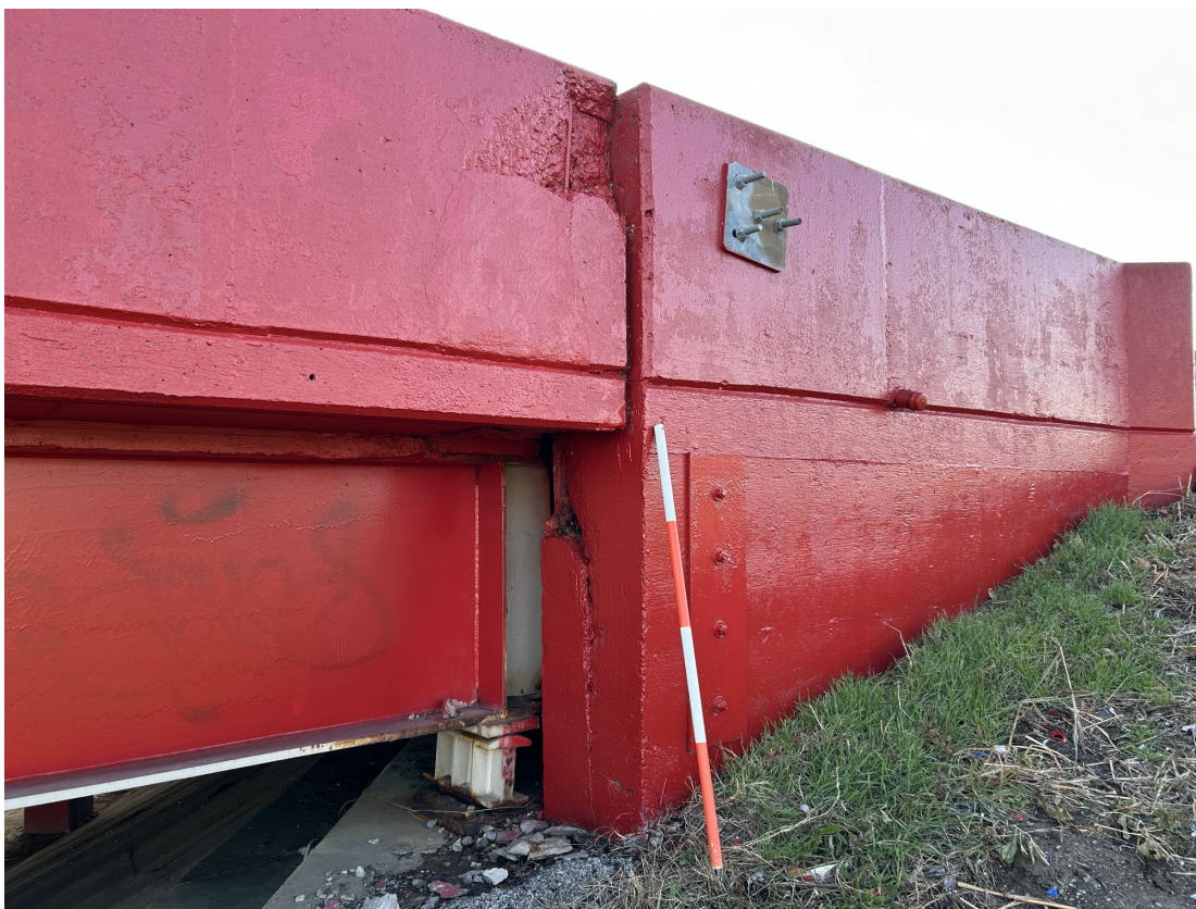
SW wingwall is fractured at the Abutment 1 backwall and is tilting out. There is also a 2-foot long spall with exposed rebar in the west rail at the south end.
