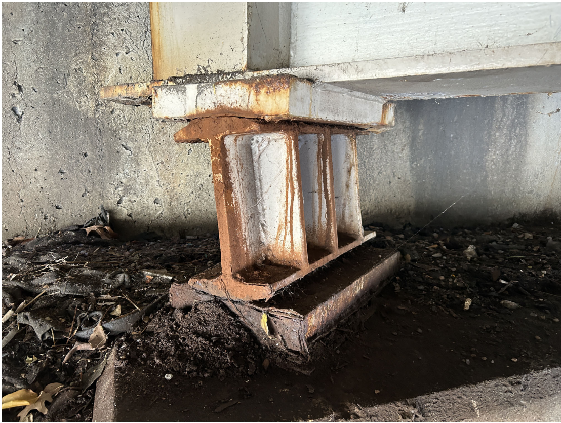
Close-up of Girder 7 bearing with fretting rust. Rocker can be moved slightly by hand.
