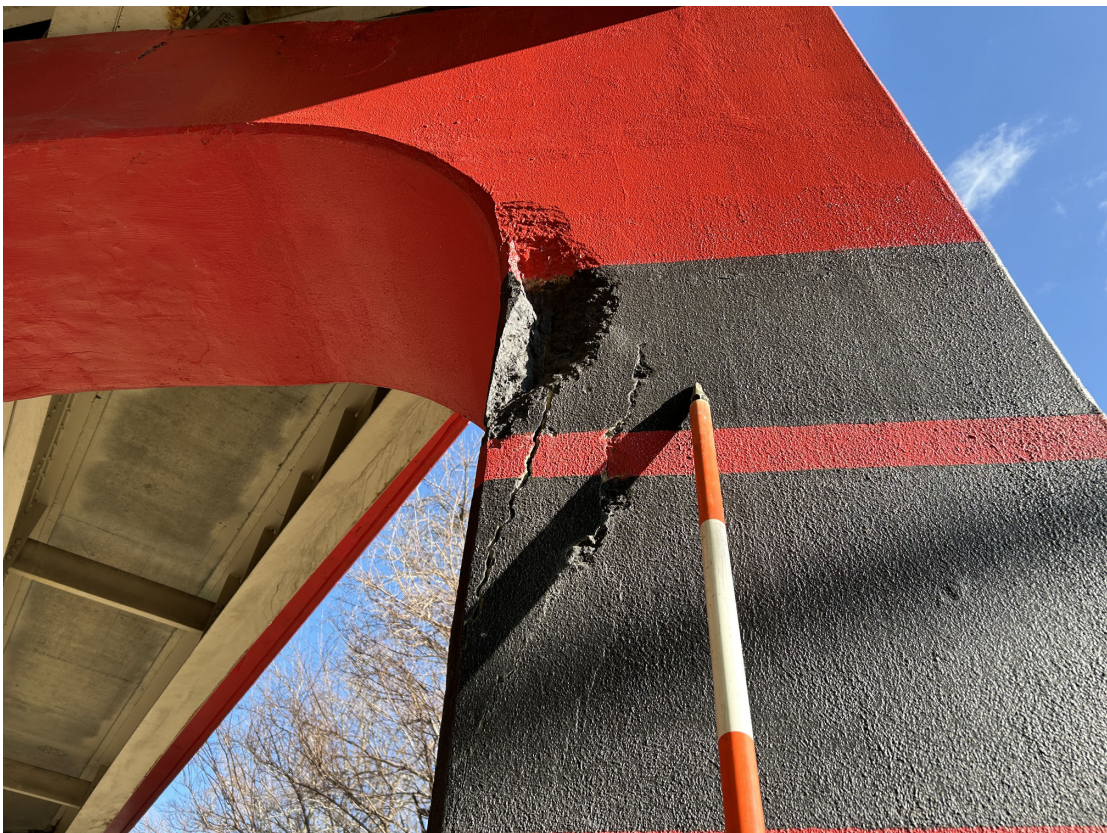
Spall in Pier 3-Column 10
