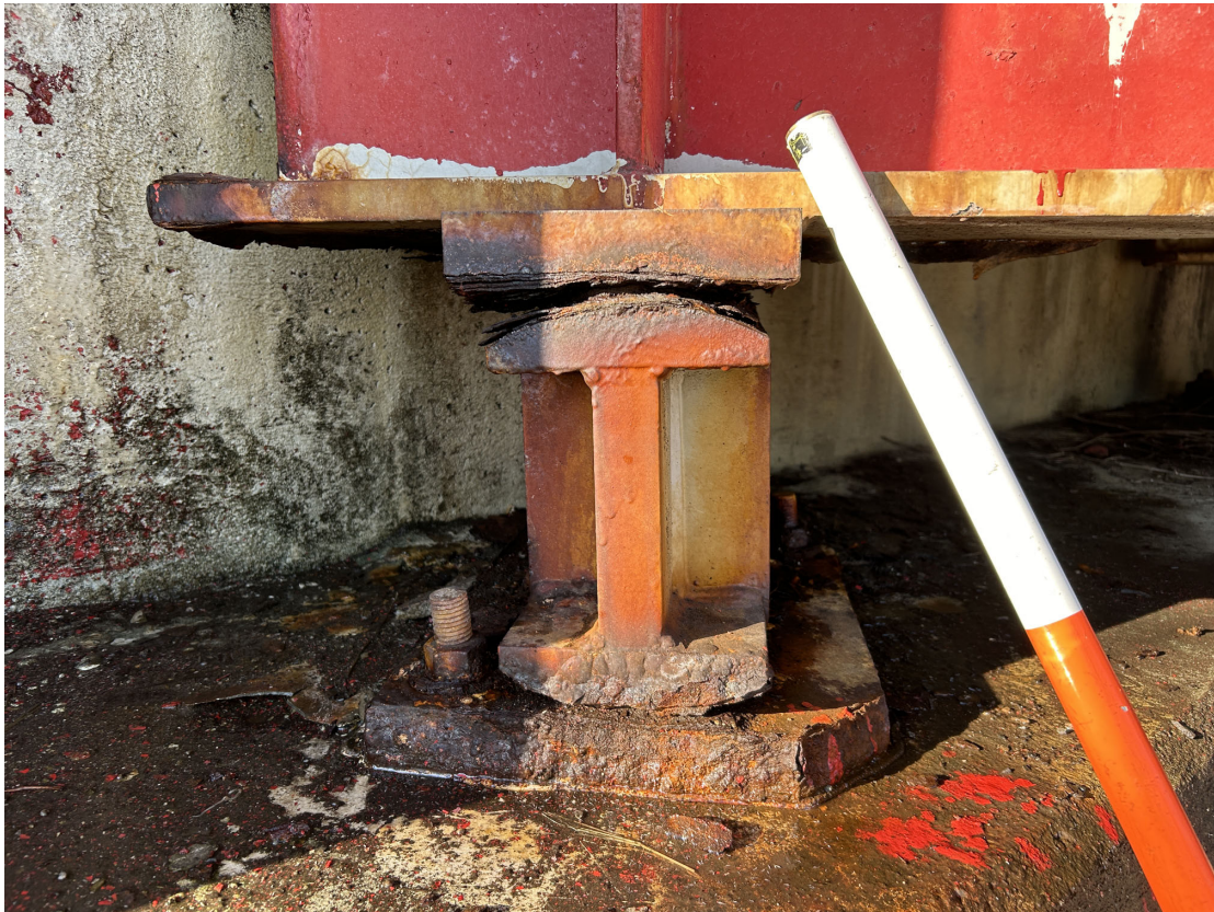
Bearing for Girder 18 at Abutment 1 has pack rust, creating a gap between the top of the rocker and the sole plate.
