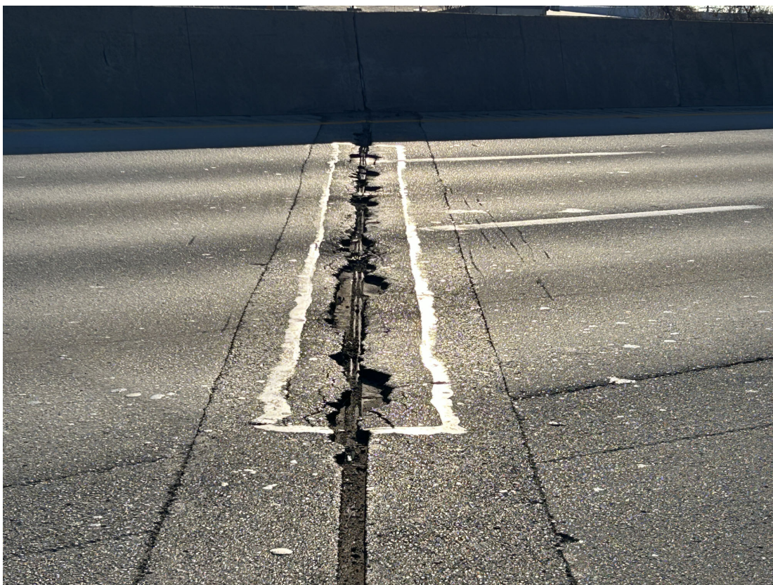
Close-up of typical failing asphalt plug joints.
