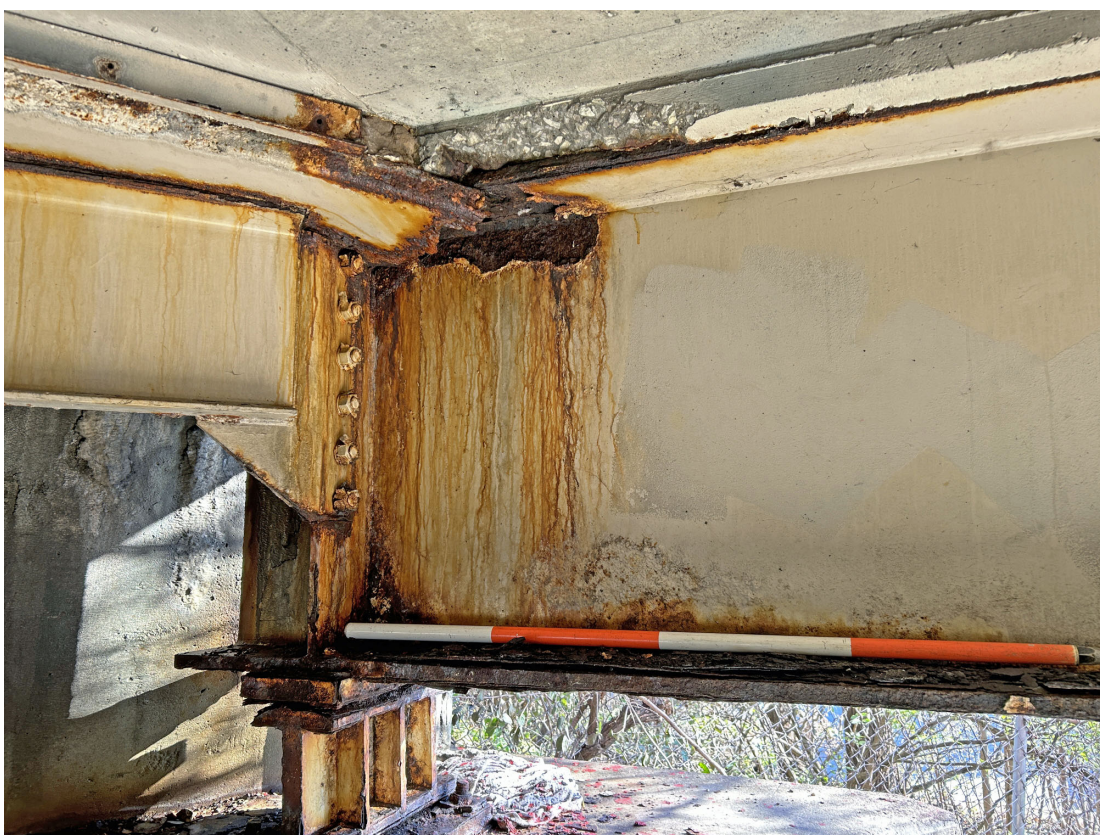
Girder 18 has corrosion with section loss at Abutment 4 end.
