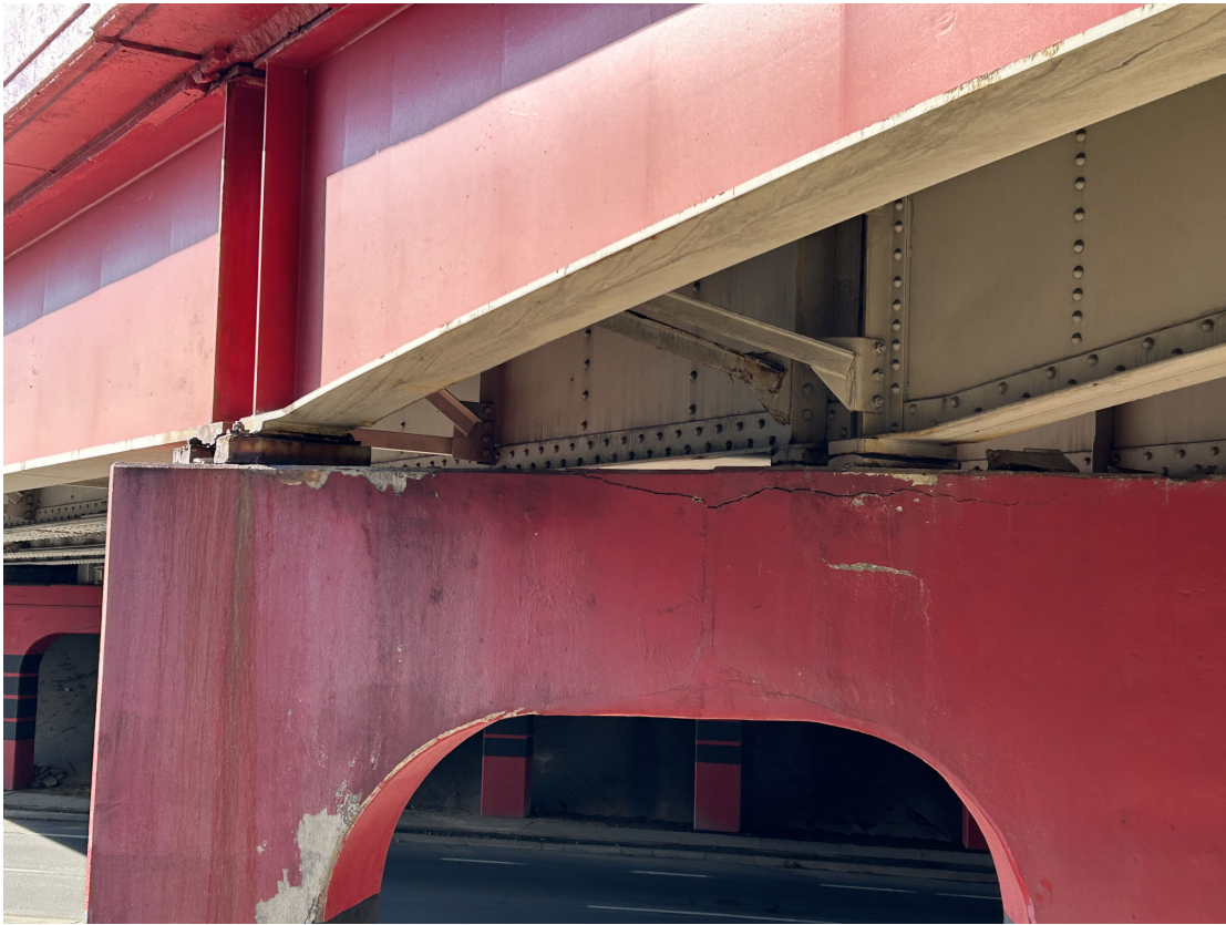
Pier 3 east end of the north face showing wide cracking in the cap plus typical bearings.
