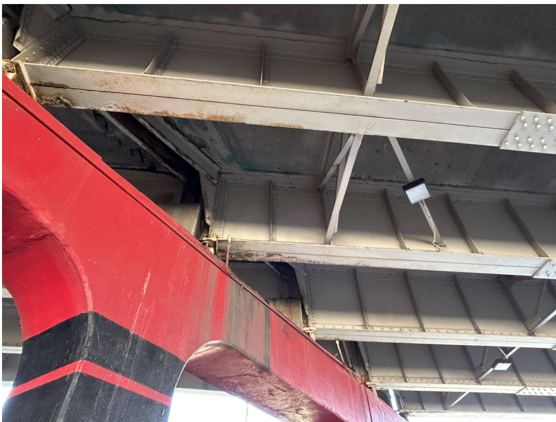
Span 2-Girders 4 and 5 at Pier 2 showing corrosion along bottom flanges.
