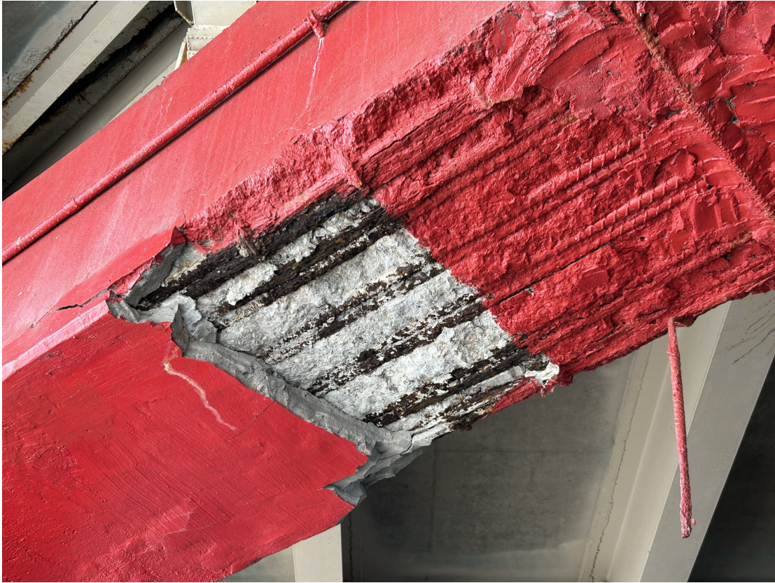
Pier 2 cap has multiple areas of spalling with exposed rebar. Example between Columns 7 and 8.
