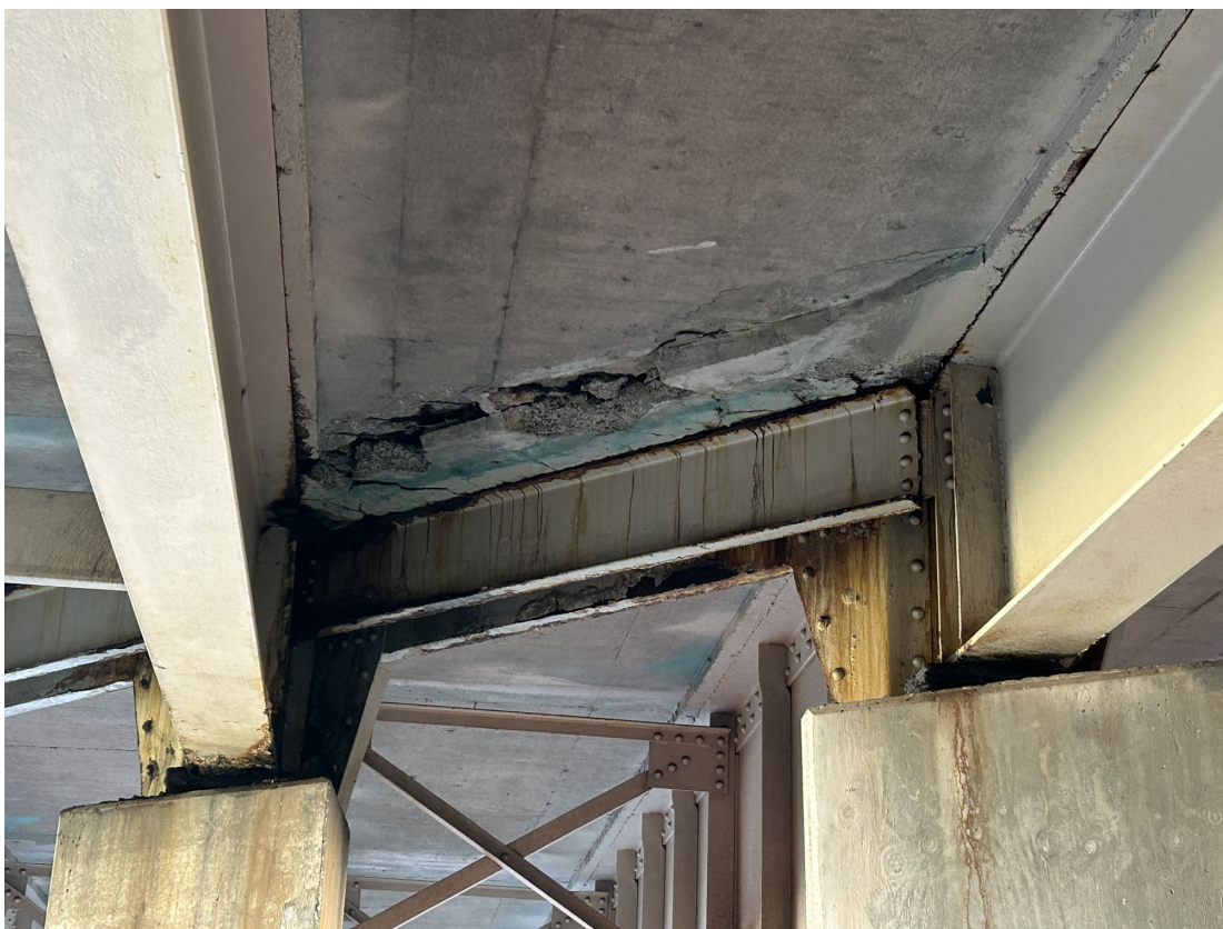
Span 1 soffit has a spall with exposed rebar in Bay 4 at Pier 2.
