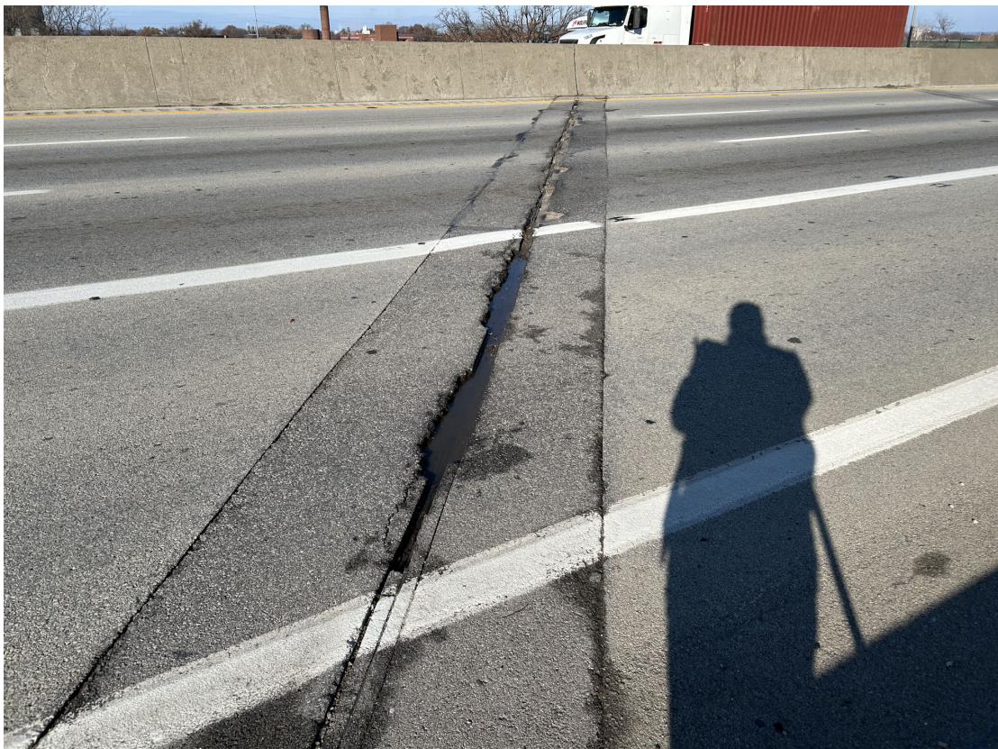
Asphalt plug joint over Pier 3 NB.
