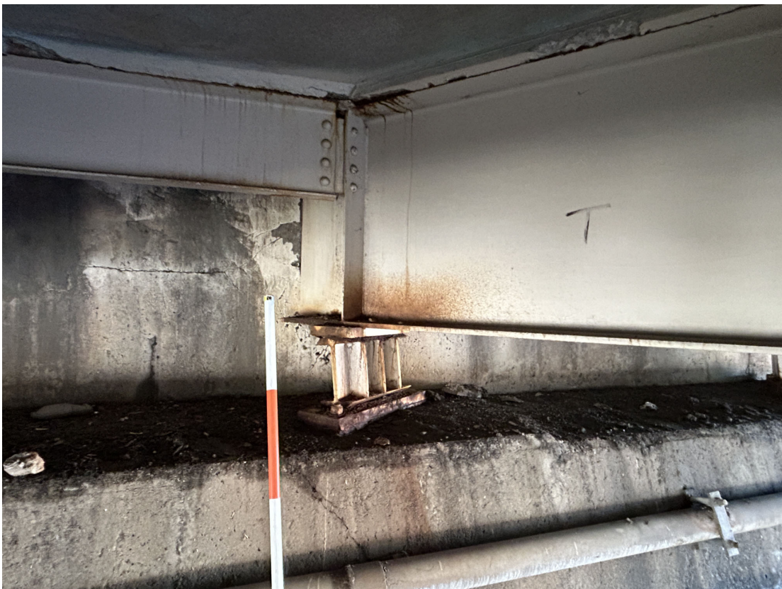
Typical bearing at Abutment 1. Bearings are expanded and have corrosion. Girder 3 shown.
