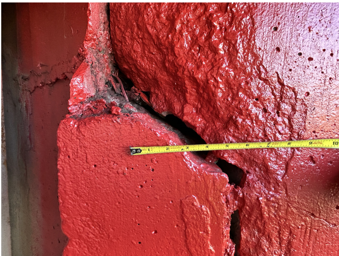
Close-up of fracture width.
