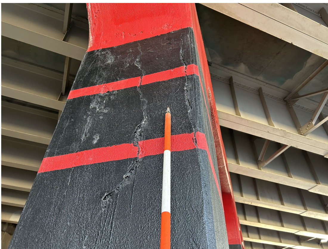
Pier 3-Column 4 with closely spaced wide vertical cracks.
