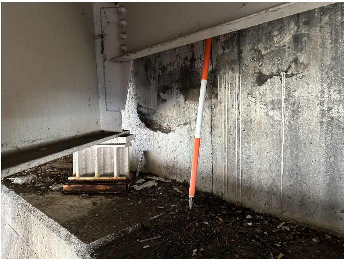
Abutment backwalls have failing patches and spalls. Abutment 1 backwall at Bay 8 shown.
