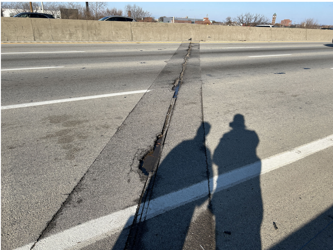
Asphalt plug joint over Pier 2 NB.
