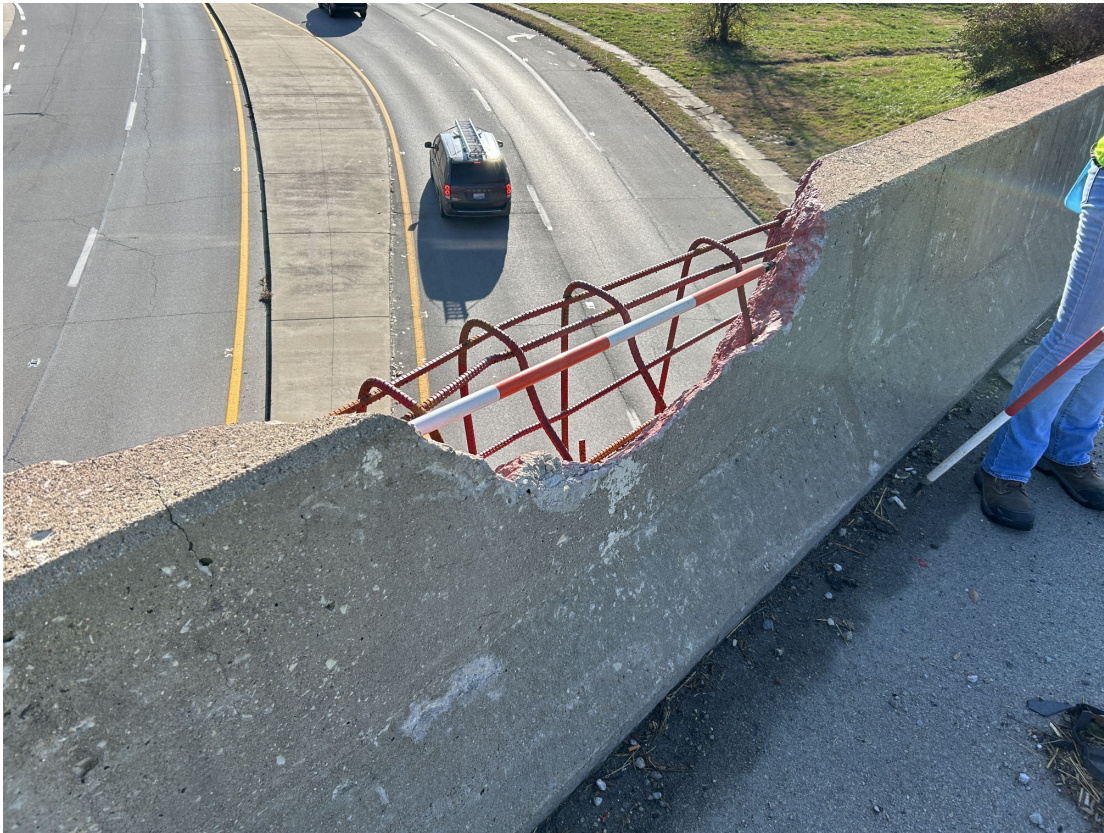
East rail in Span 2 has a full depth spall.
