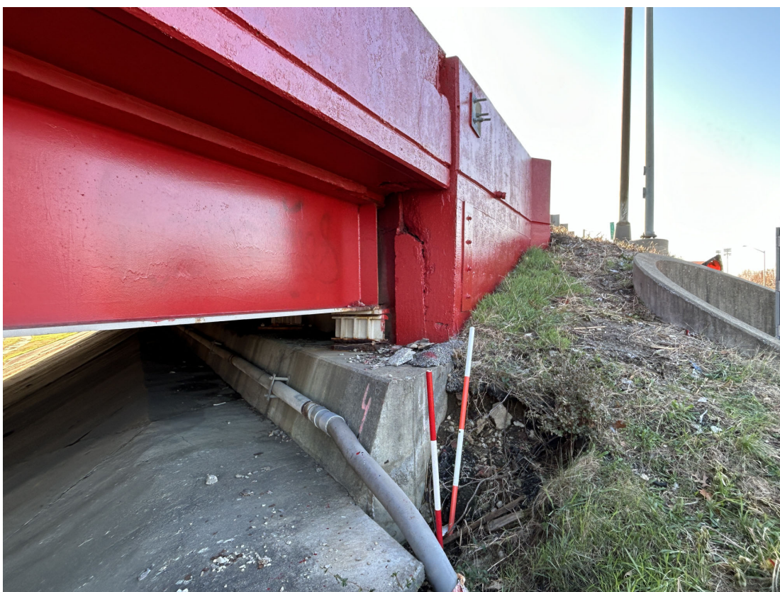
West end of Abutment 1 showing erosion plus damage to SW wingwall.
