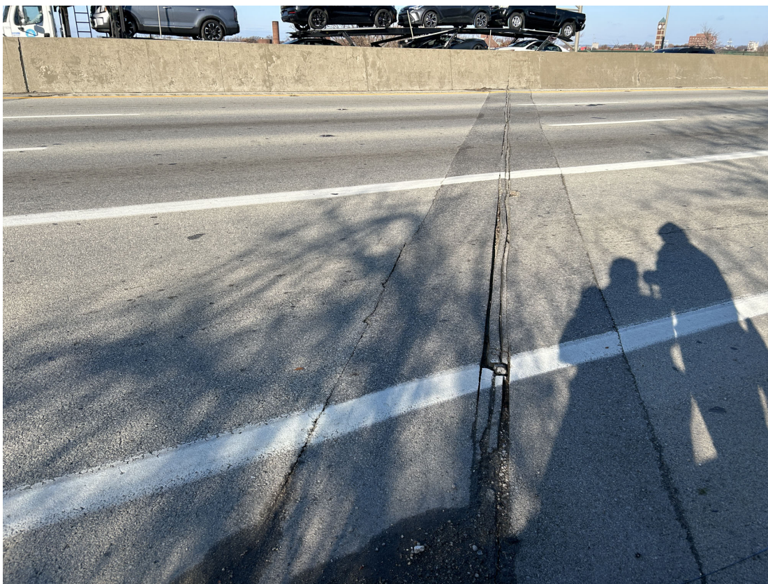
Asphalt plug joint over Abutment 4 NB.
