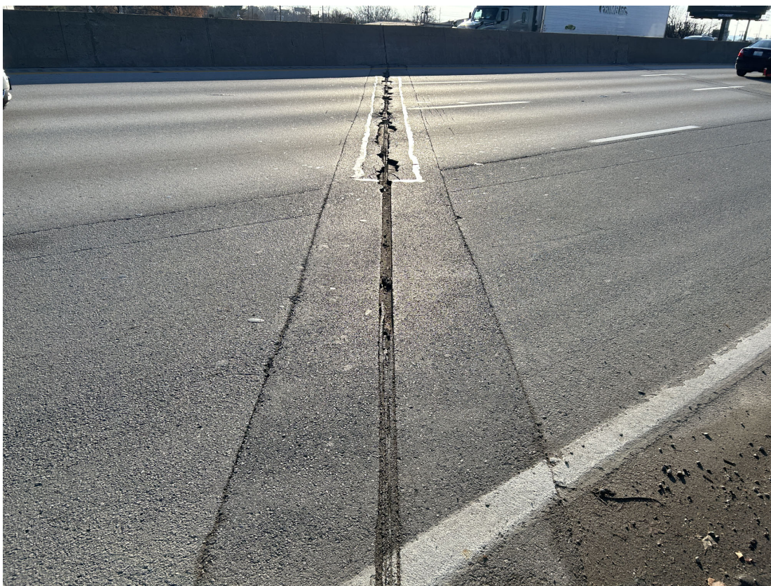
Asphalt plug joint over Pier 2 SB.
