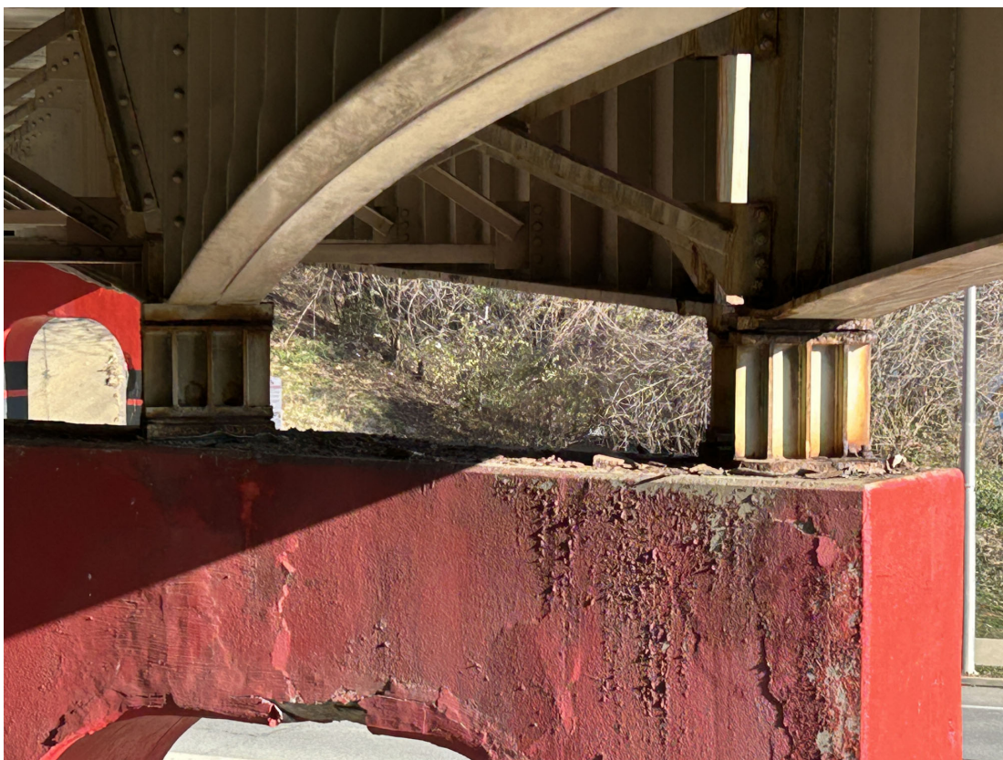
Another view of Pier 2-Girders 17 and 18 showing corrosion on bearings.
