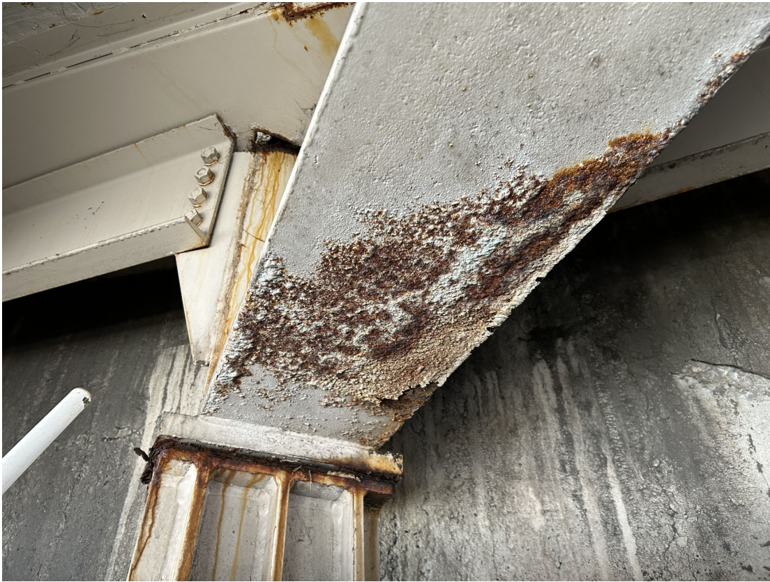
Beams ends have corrosion. Example along Girder 11 at Abutment 1.
