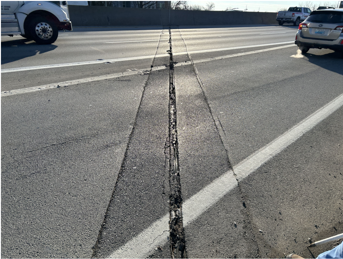
Asphalt plug joint over Abutment 4 SB.
