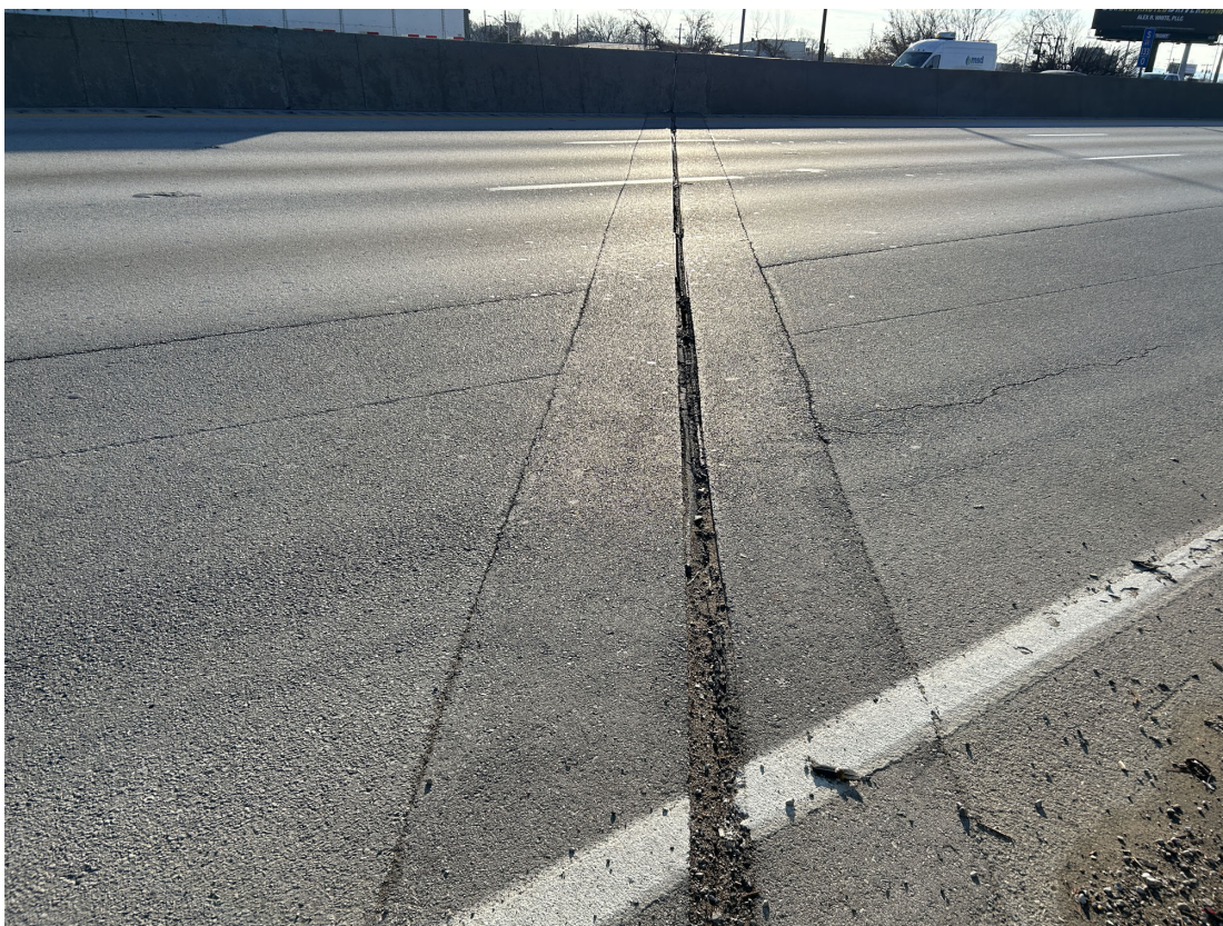
Asphalt plug joint over Abutment 1 SB.
