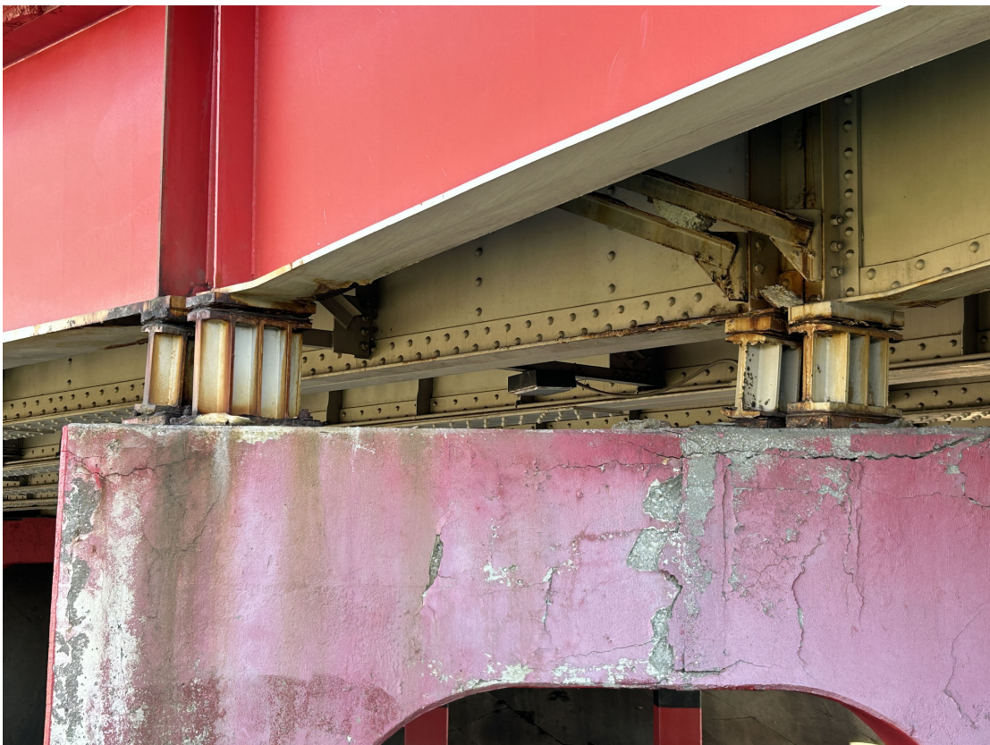
Pier 2-Span 1 fixed bearings at Girders 1 and 2 showing corrosion, plus there is cracking in the pier cap.
