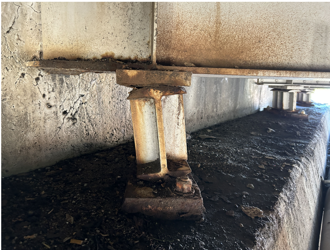
Abutment 1-Girder 3 bearing close-up
