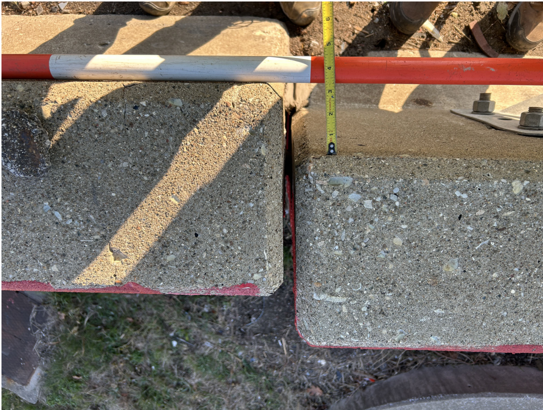
SW wingwall is tilted out roughly 3.25 inches at the top of the rail.
