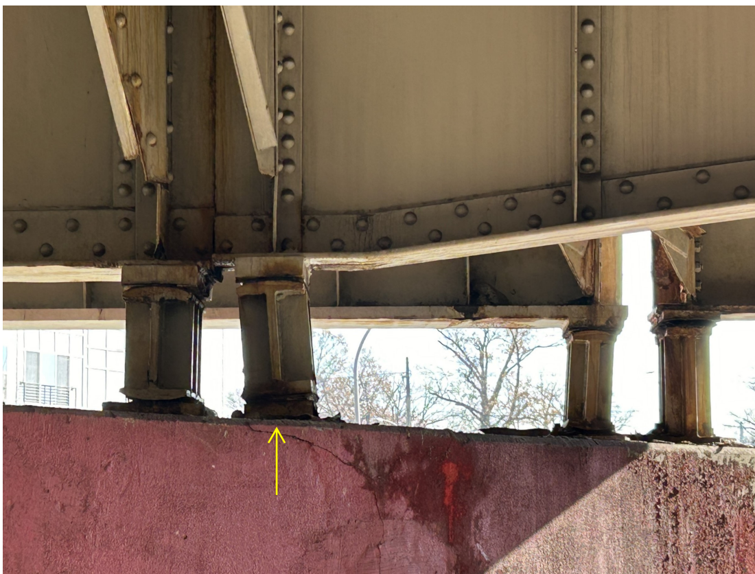
Pier 2 bearings for Girders 17 and 18. Span 1 bearings are fixed. Note Girder 17-Span 1 fixed bearing is tilted to the north due to pack rust.
