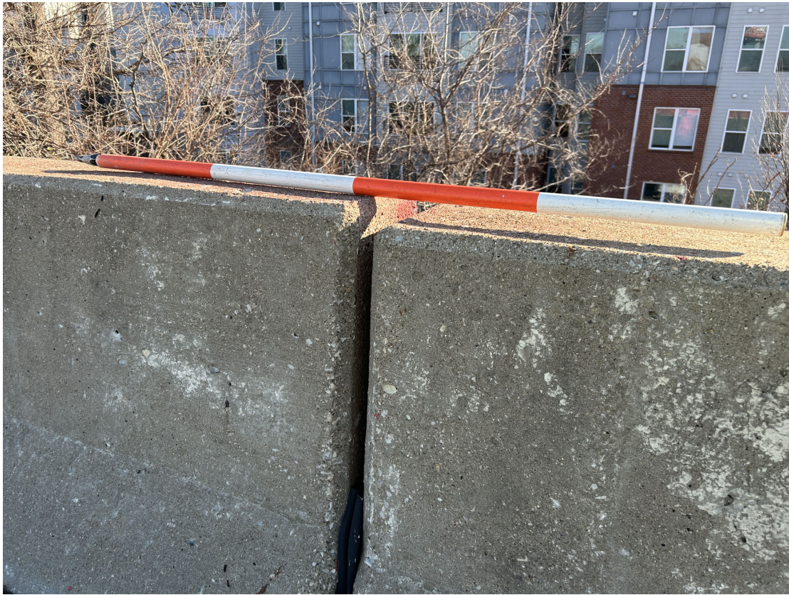
East rail at Pier 3 has a vertical offset. Span 3 is roughly 1 inch higher than Span 2.
