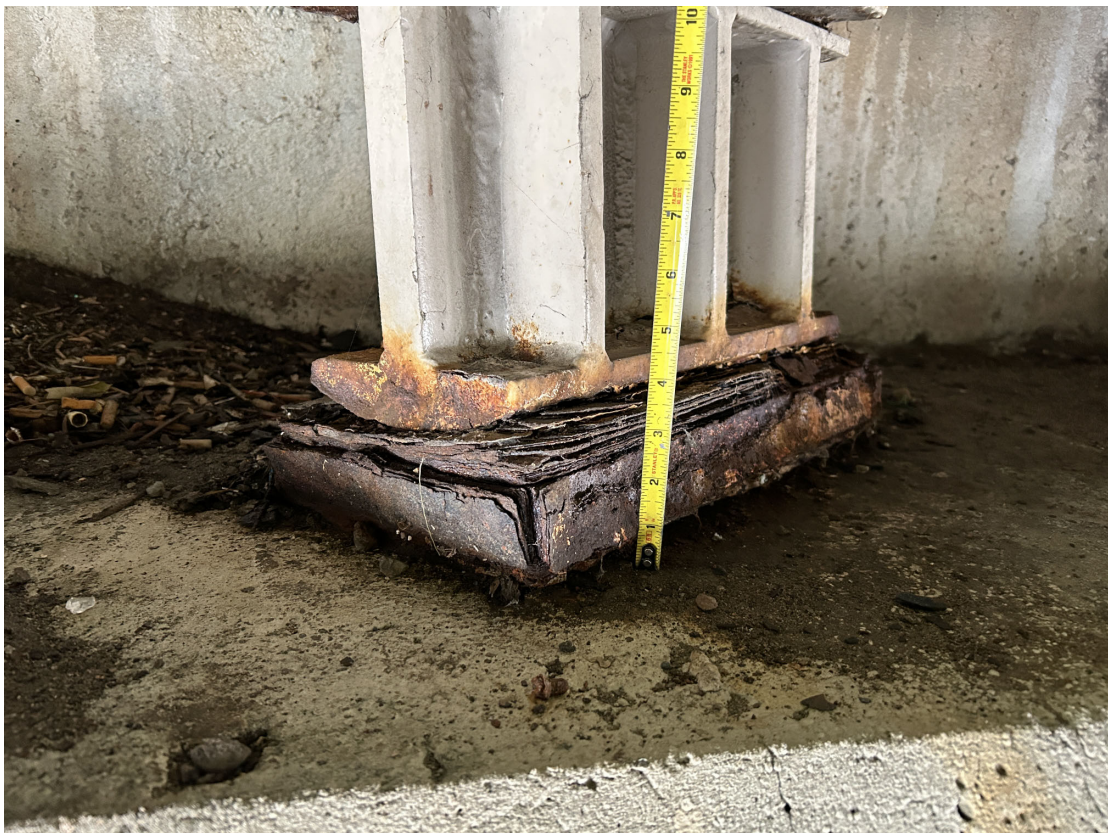
Abutment bearings typically have pack rust and section loss, primarily along the masonry plates. Example at Abutment 4 Girder 10.
