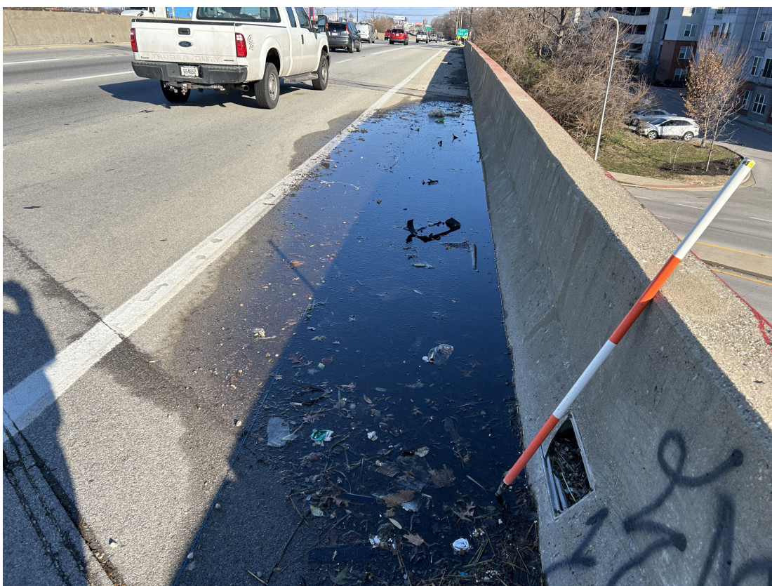
Water is ponding in the SE shoulder.
