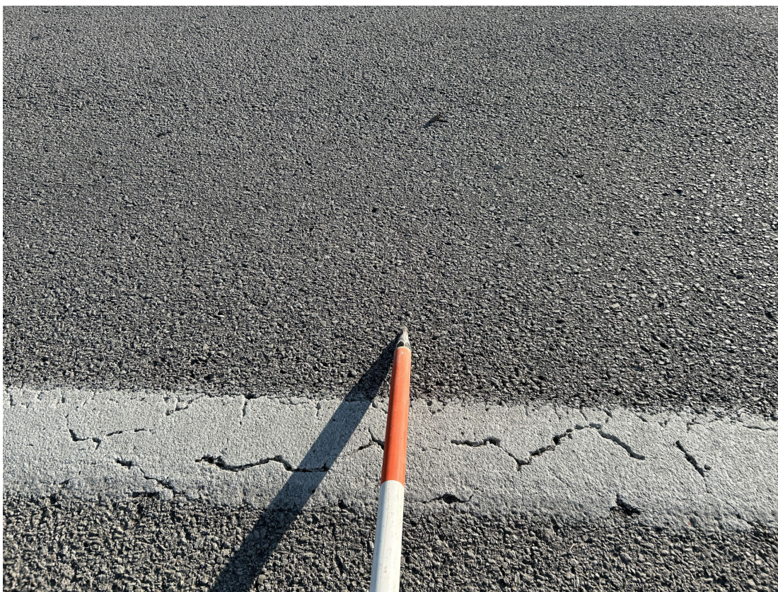
Typical raveling of the asphalt overlay.
