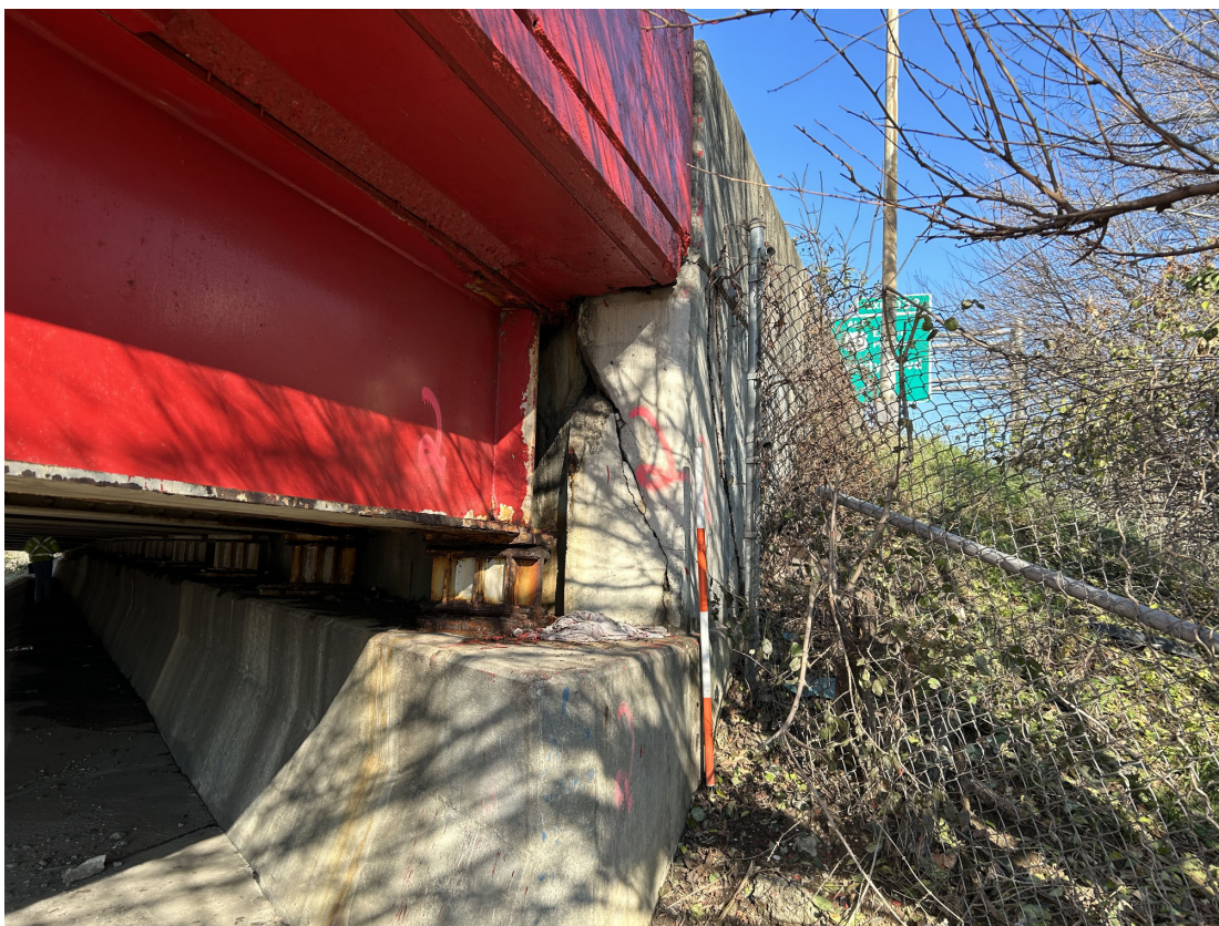
East end of Abutment 4 has a wide crack in the backwall.
