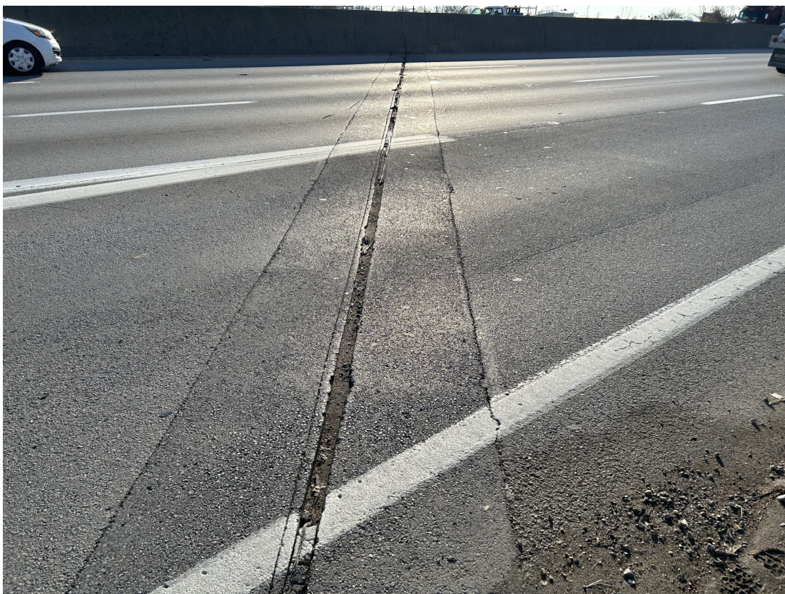
Asphalt plug joint over Pier 3.
