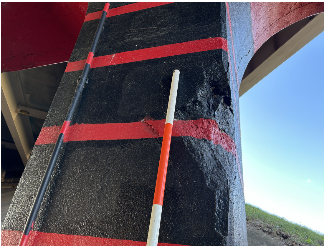
Pier 2-Column 2 - example of painted over spall with exposed rebar.
