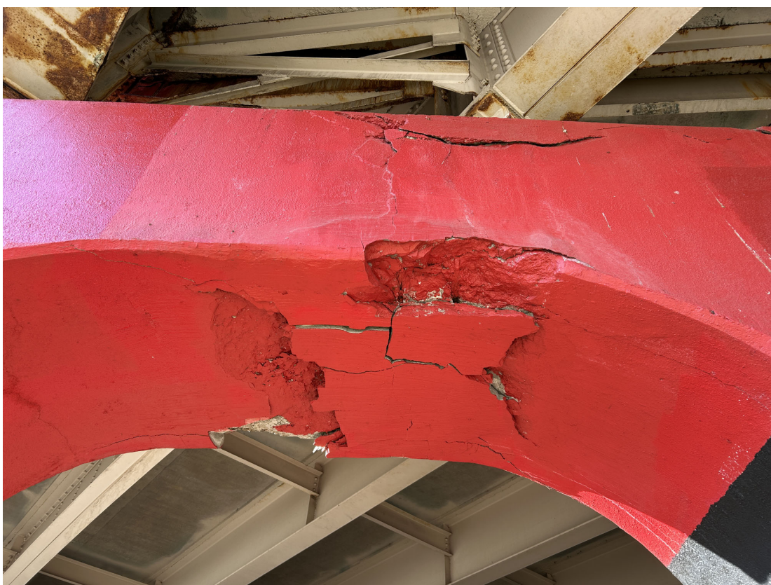
Cracking and spalling in the Pier 2 cap between Columns 9 and 10.
