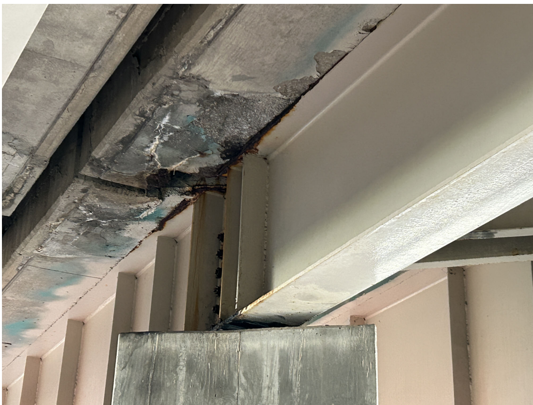
Deterioration in the soffit at the longitudinal joint over Pier 2.
