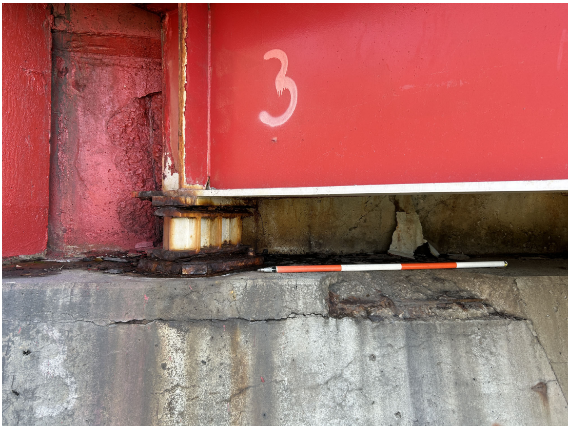
West end of Abutment 4 has spalling with exposed rebar in the backwall and spalling in the beam seat in Bay 1. Also note heavy corrosion of the Girder 1 bearing.
