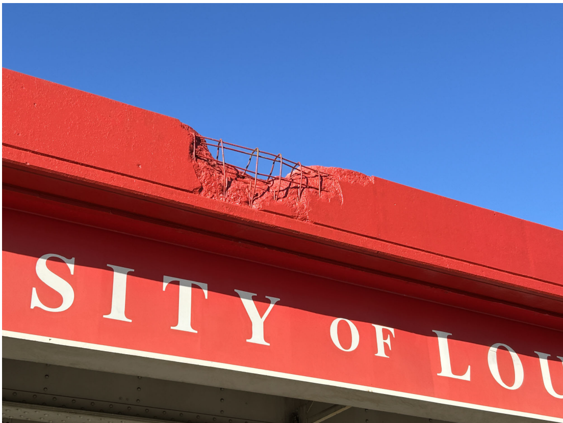
Another view of east rail spall mid-Span 2.
