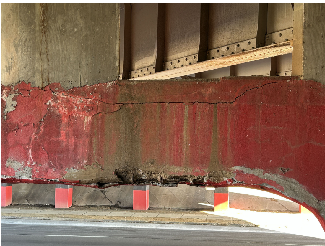
Cracking and spalling in the Pier 2 cap below Girder 5.
