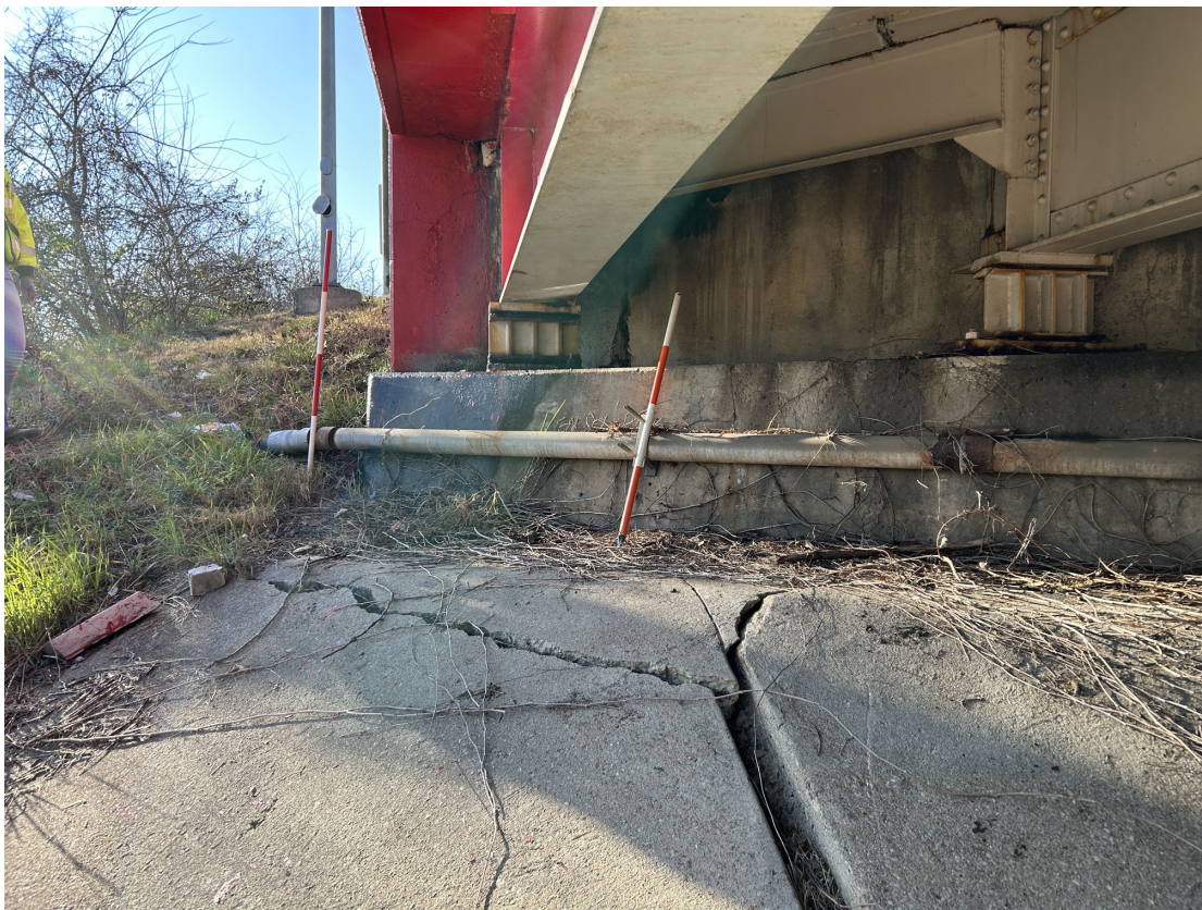
East end of Abutment 1 showing cracking slope protection.
