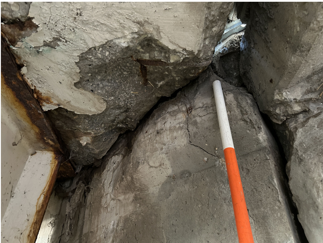
Close-up of deck spalling at the south end at the longitudinal joint.
