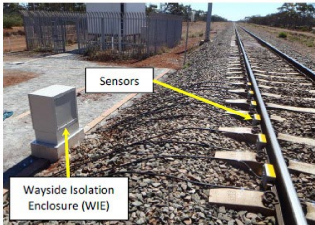
Typical Site Installation
