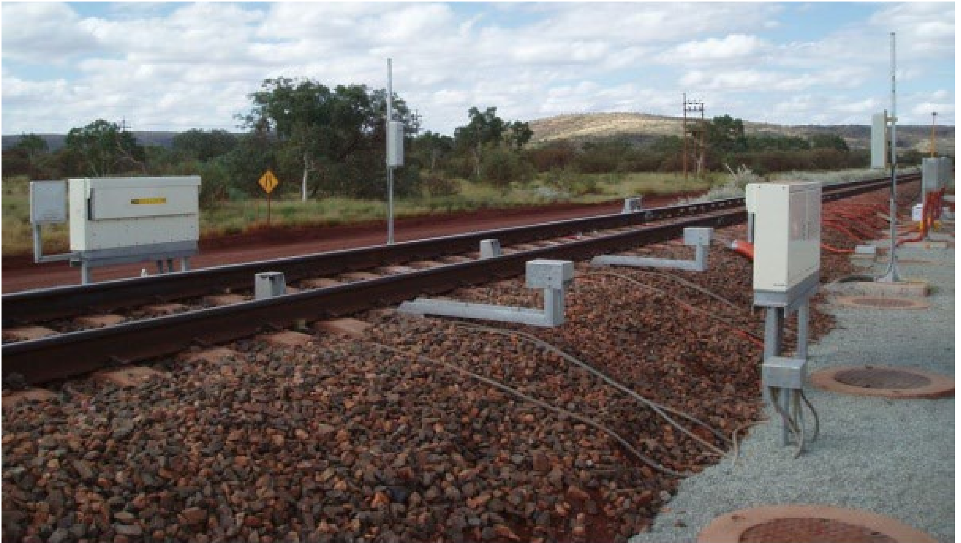
Bearing Acoustic Monitor Installed
