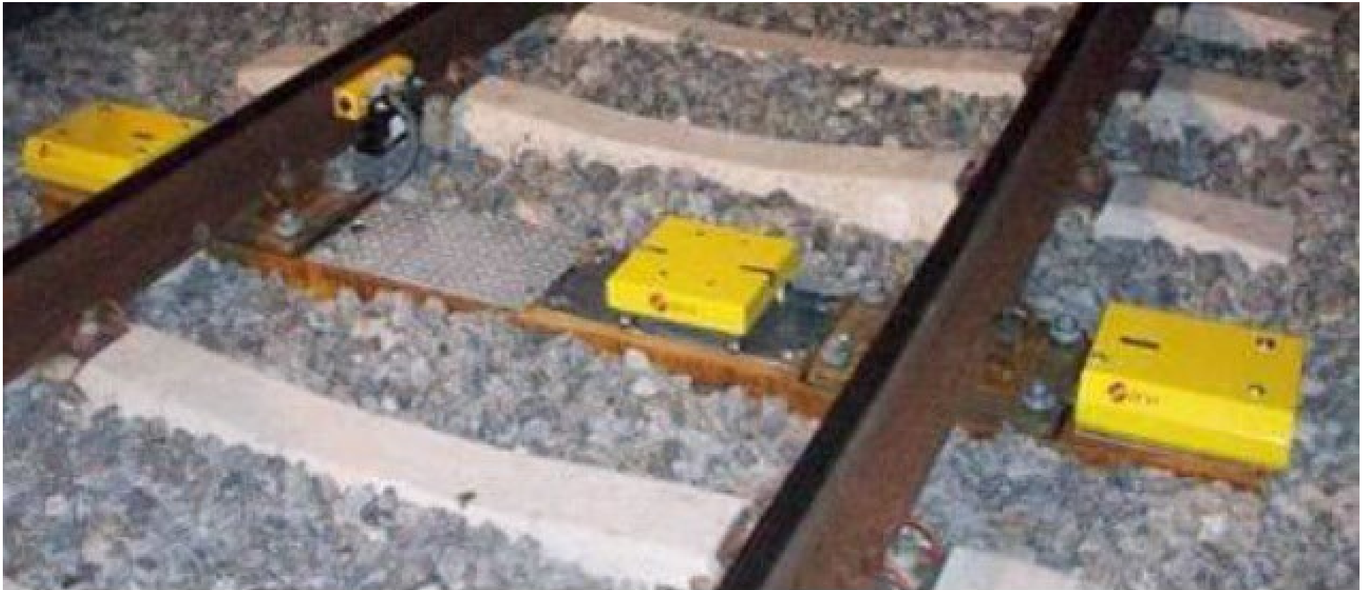
Hot-Bearing & Hot-Wheel Installation
