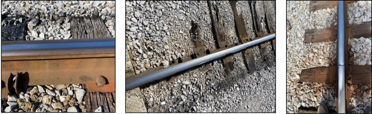
Figure 5: Representative poor mainline track conditions on the RJCM
