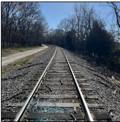
Worn-out rail on the Memphis Line
