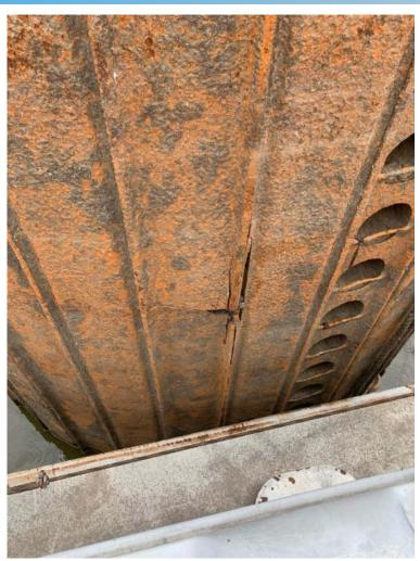
Project would make long term repairs to Mooring Cells 2, 3, and 4. Temporary patches and repairs have been made, but full circumference bands are needed for protection and stability and to prevent loss of internal ballast stone.
