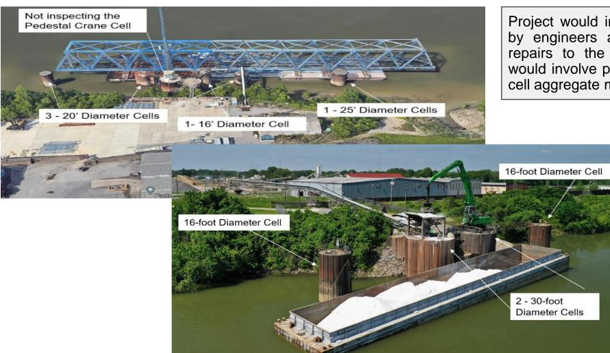
Project would involve inspection of nine barge cells by engineers and divers and then begin making repairs to the most needed barge cells. Repairs would involve patches or full bands and replenishing cell aggregate material.
